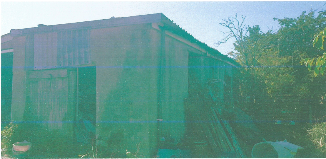
Photo 1 External front and side elevation
