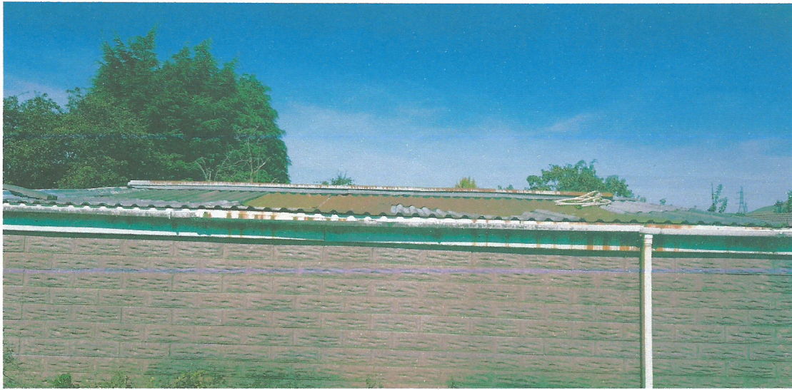
Photo 2 External view rear elevation
