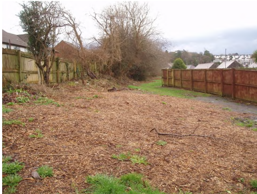
Disturbed ground at the Site entrance from Heol Llwyn Celyn
