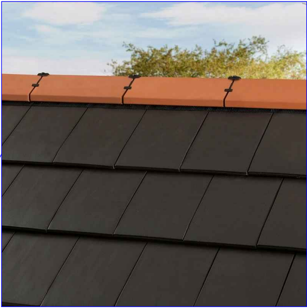
Grey flat tile roof covering with red clay effect ridge tiles.
