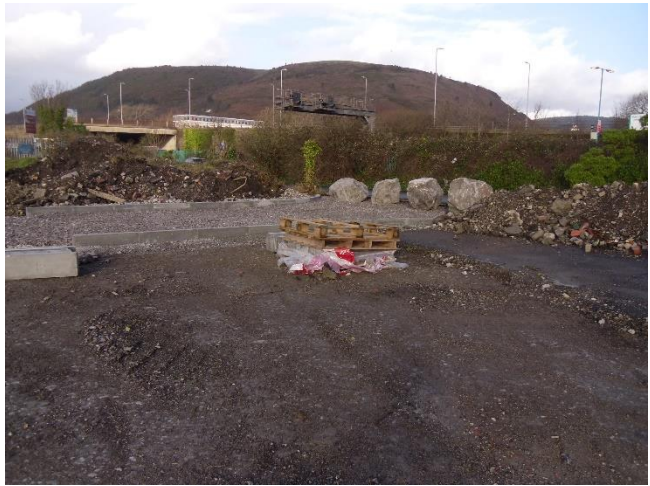
Figure 6: New concrete access road located within the north eastern corner of the site.
