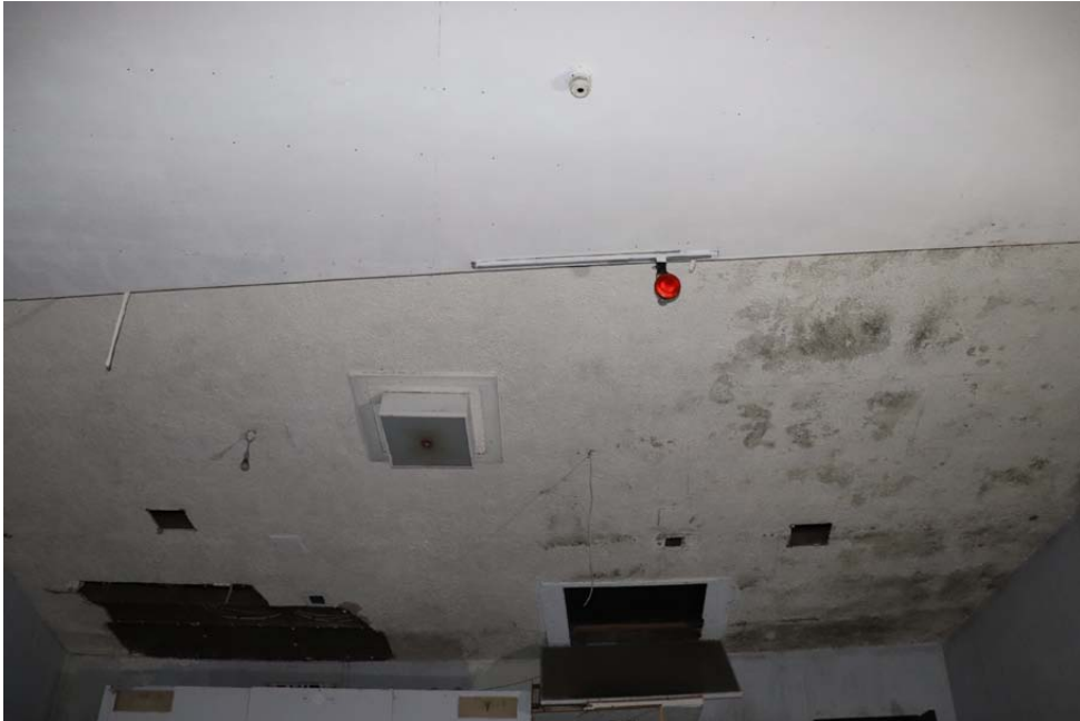
View of ceiling to soffit underneath main auditorium balcony
