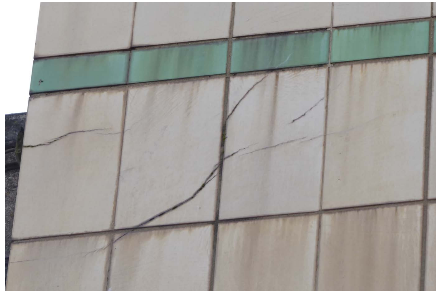
View of one of the cracks running through a series of faience tiles near the top
