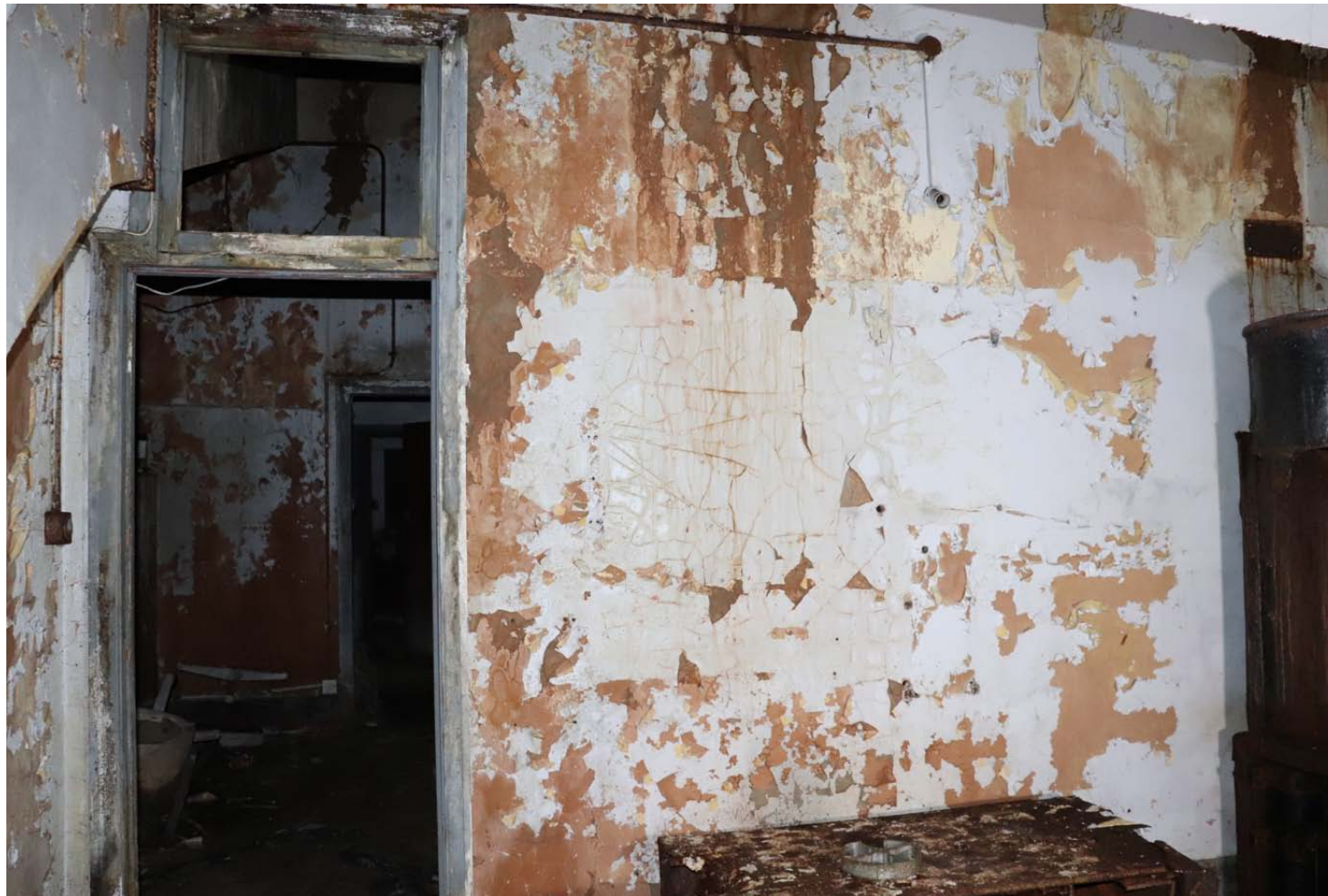
View of north wall with entrance to space
