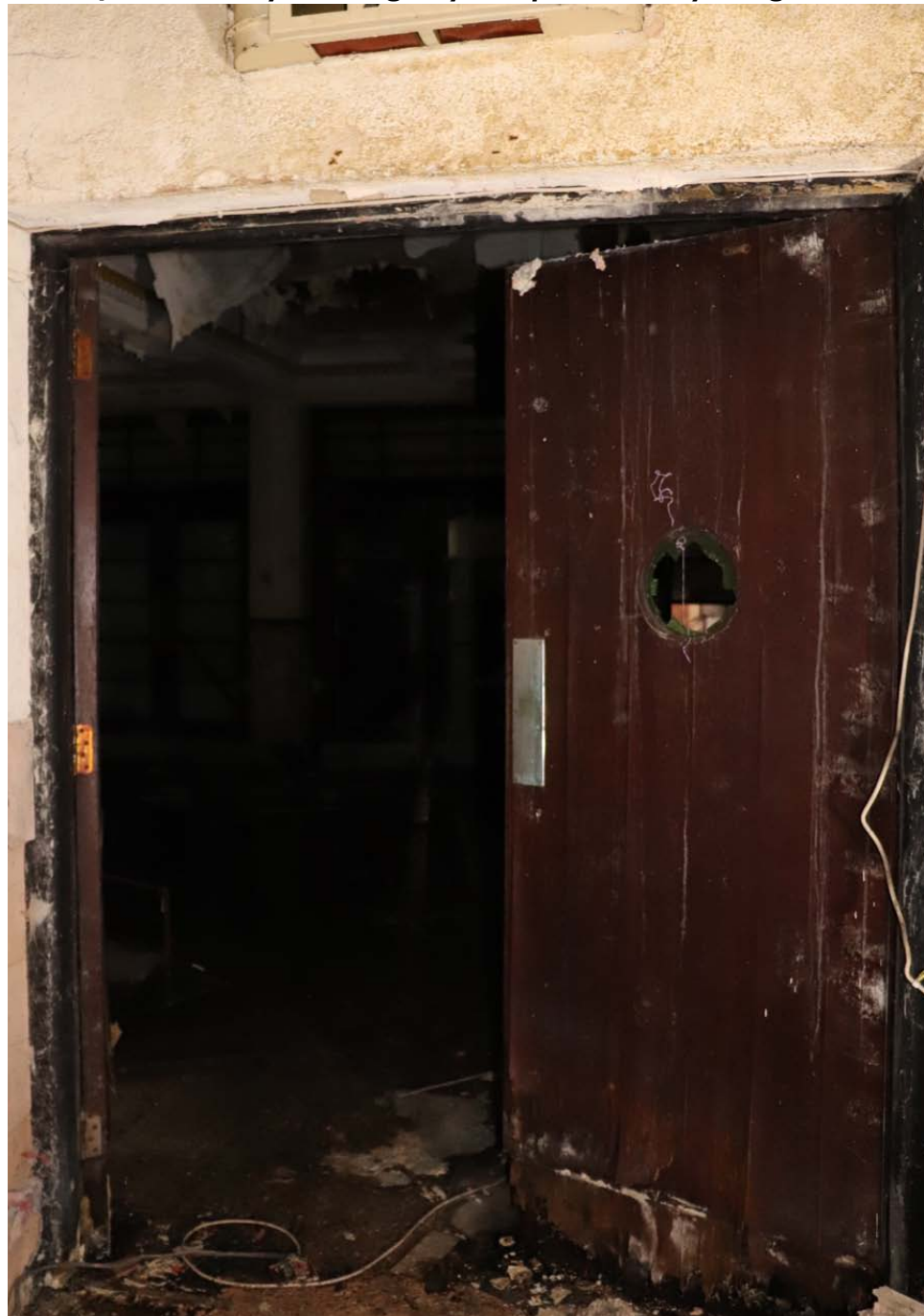
View of double doors leading from Foyer into central Corridor
