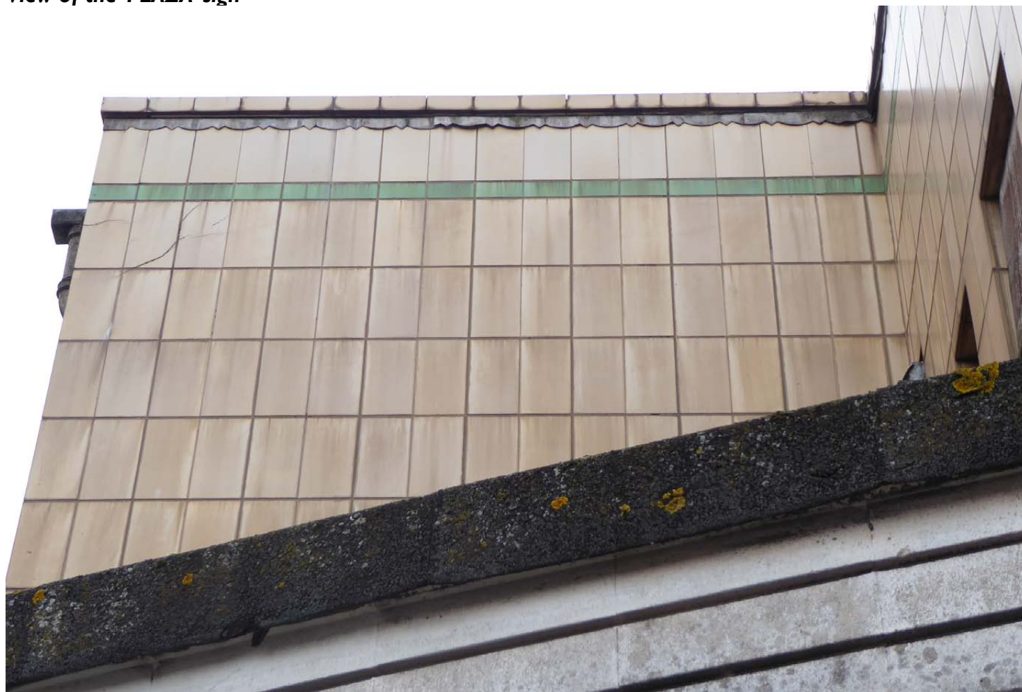
View of the left hand side of the front elevation
