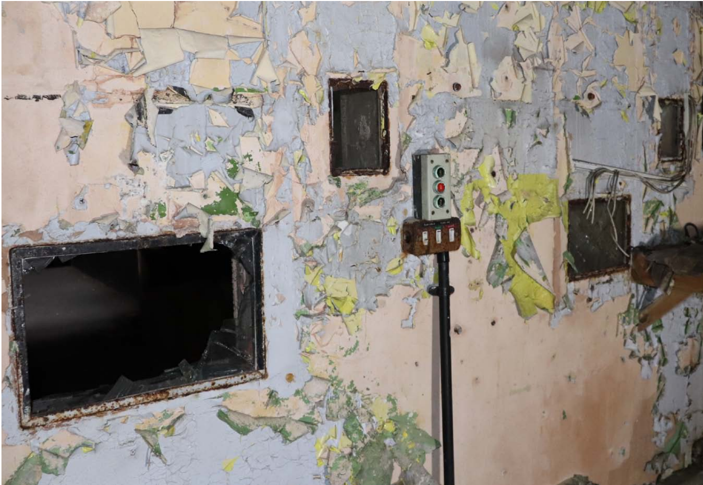
View of glazed projection openings as seen from the left
