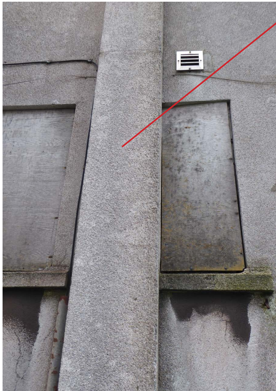
View of boarded up windows to ground floor to Male Toilets
