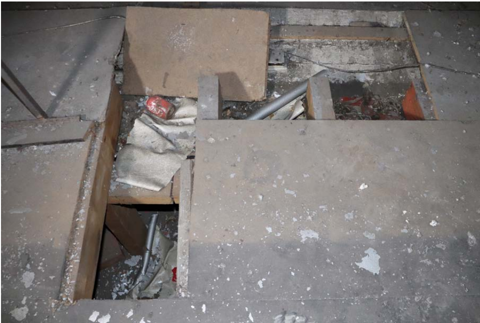
View of dip troughs within stage showing timber raised construction
