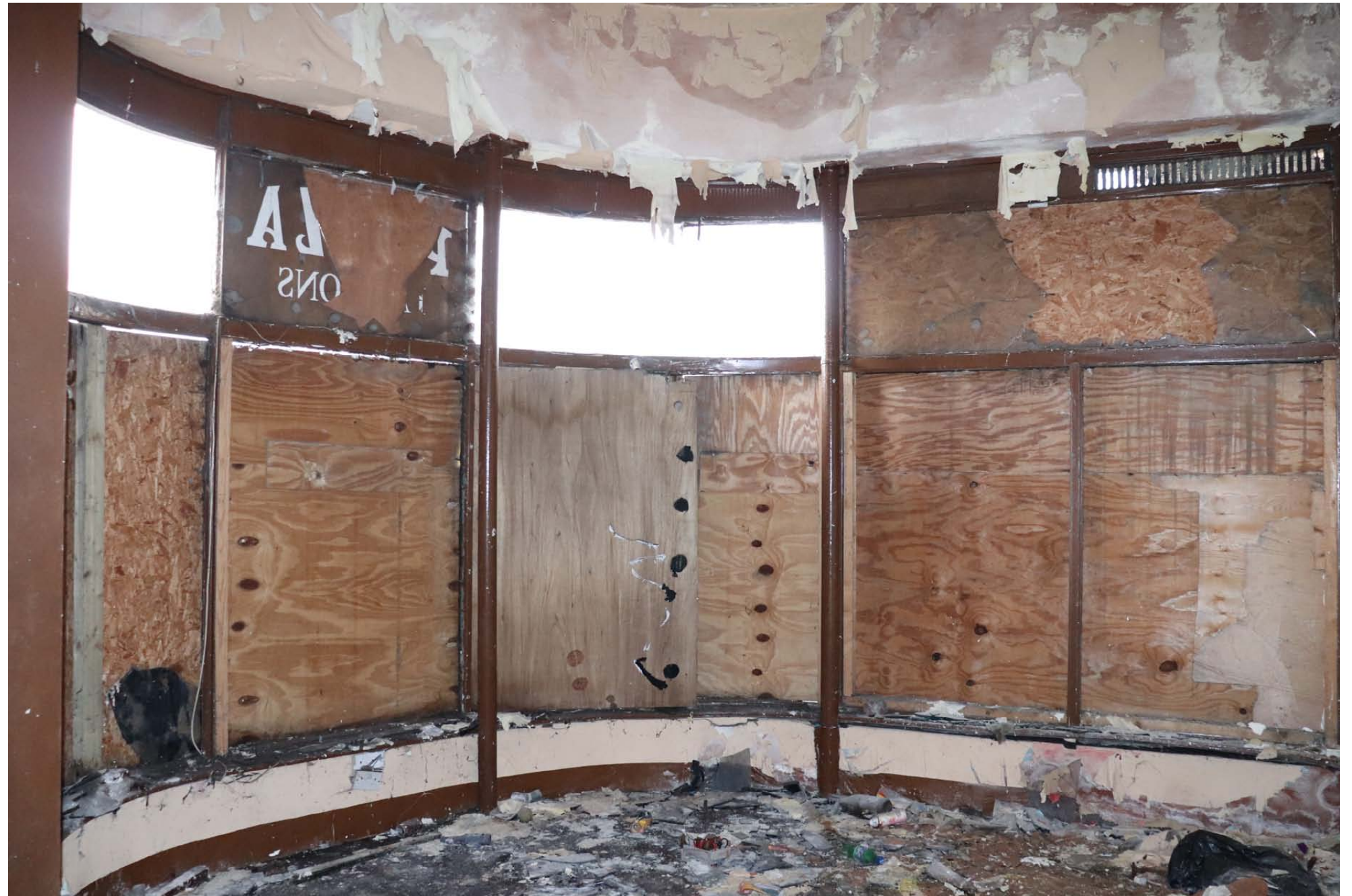
View of Glazing with Curved End and two Steel Columns and full extent of boarded up glazing panes, timber cill & vented strip to top
