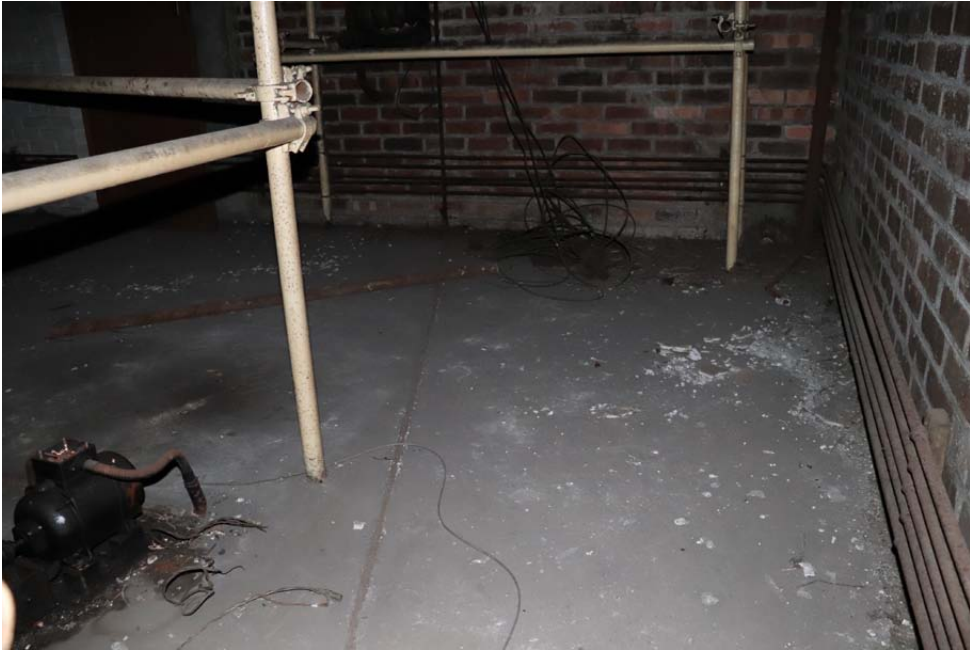
View of concrete floor to raised section
