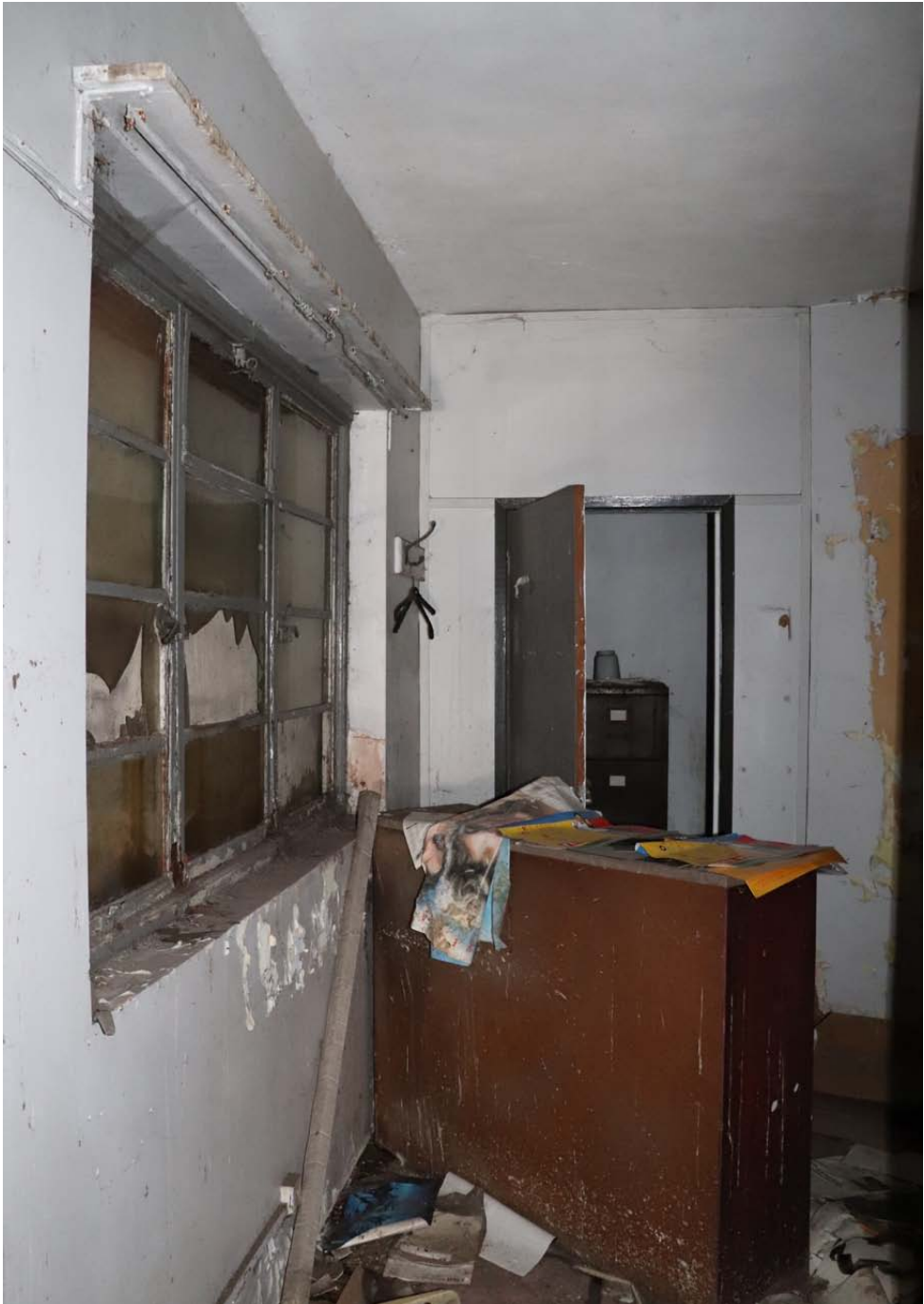
View of room from entrance door with apse-like space at end
