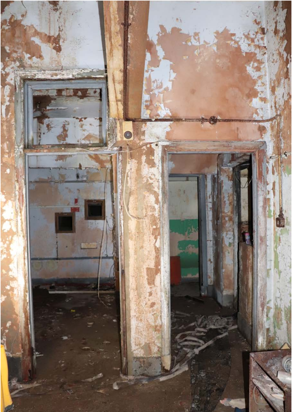
View of south wall with doors into projection room & stair area
