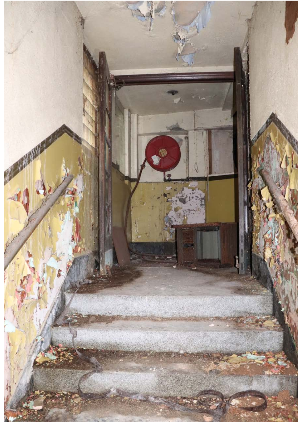
View at top of staircase towards timber-framed door
