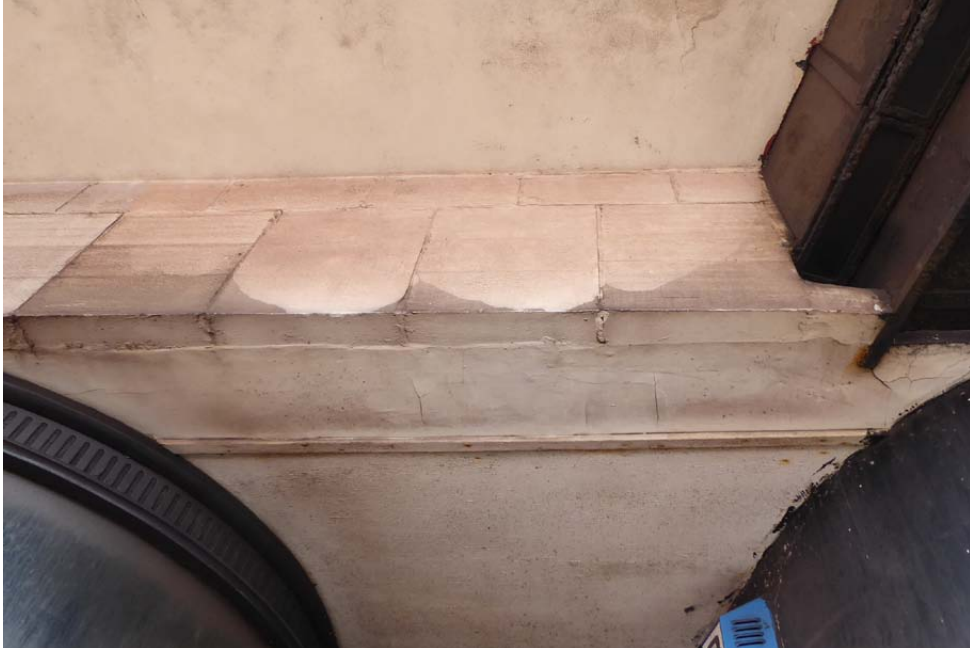
M Stone Cladding above openings
