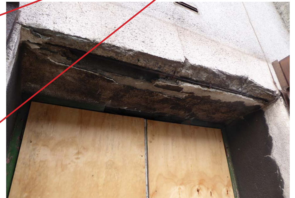
View of top of exit door
