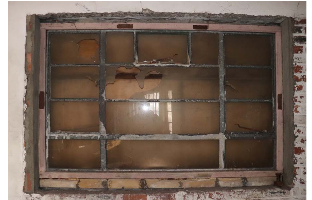
View of right hand window to east elevation
