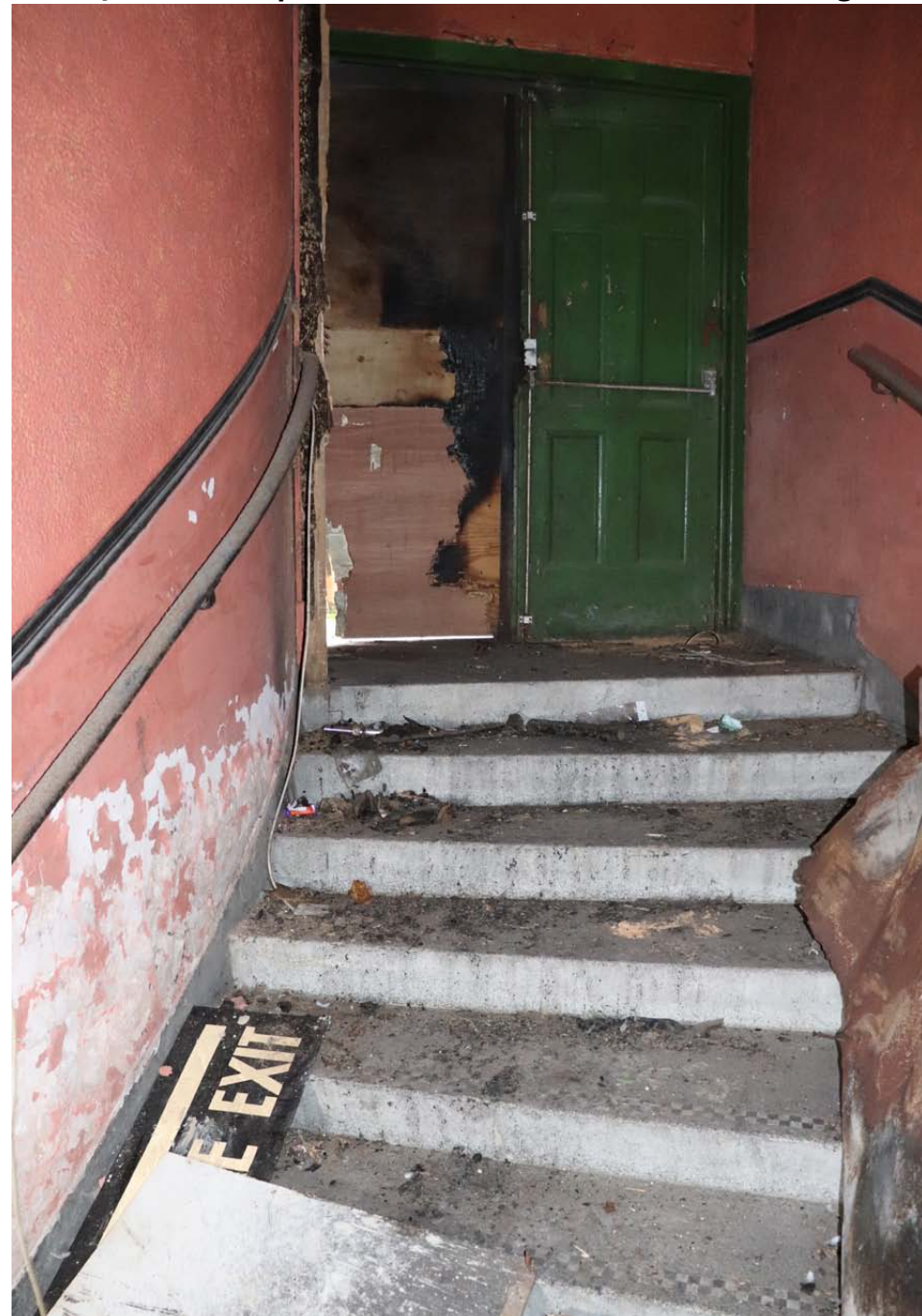
View of the Steps leading up to the final exit doors
