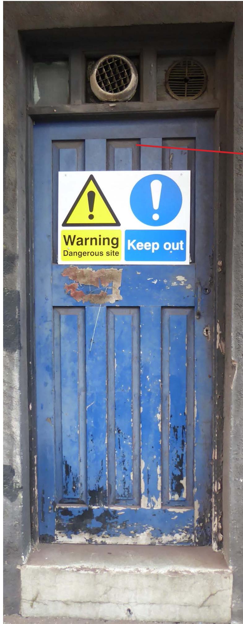
View of external door to rear of Retail unit
