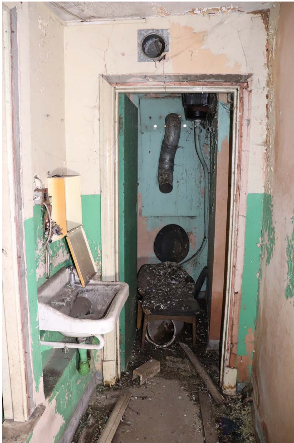
View of Toilet at top of staircase
