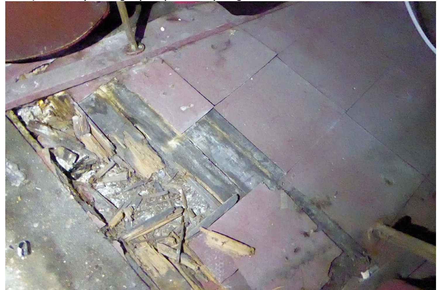
View of vinyl tile floor covering on timber boarded sloping floor
