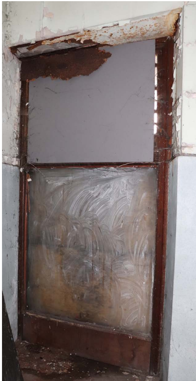
View of east wide timber-frame glazed screen
