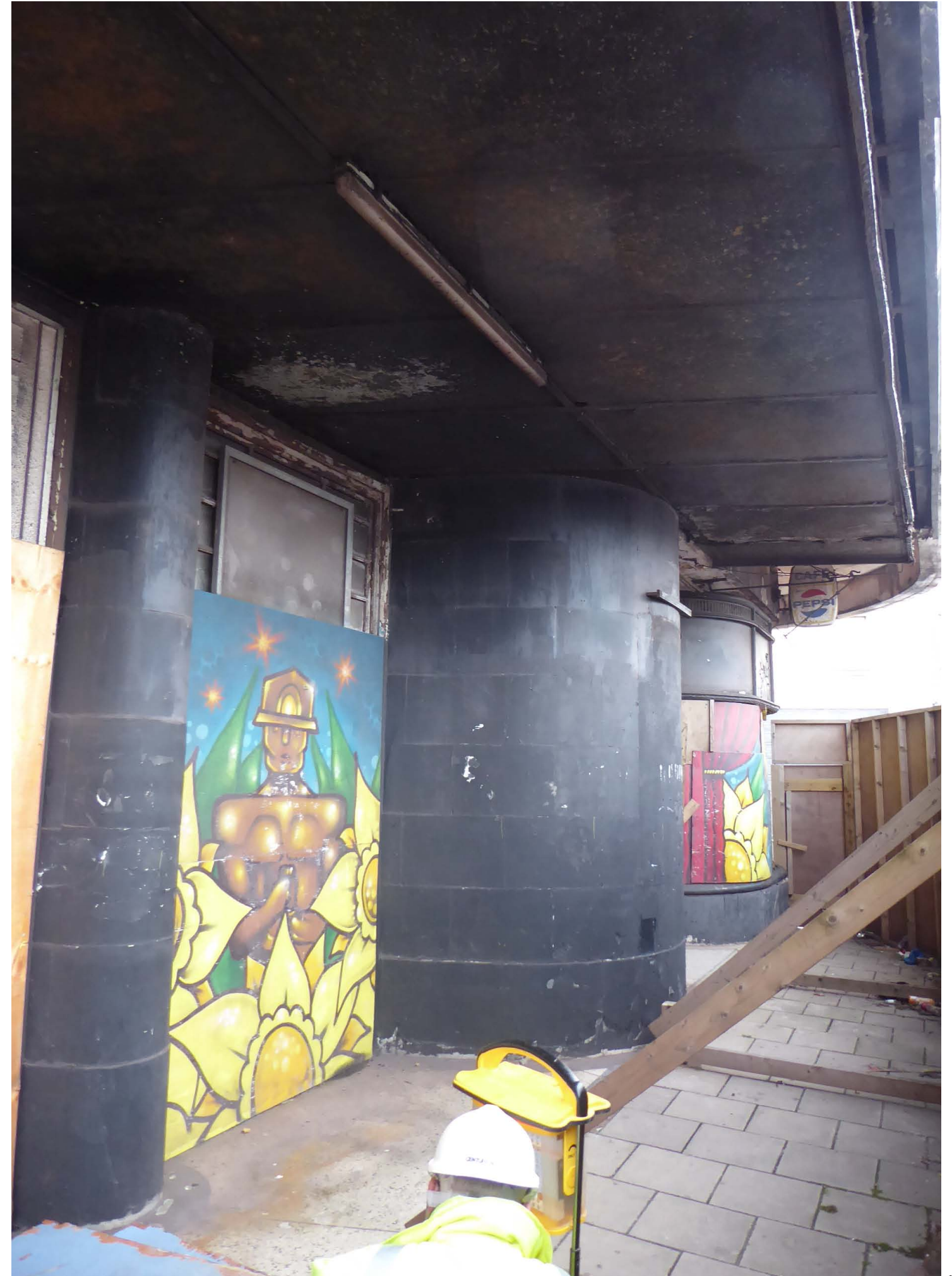
View of the right hand side of the Plaza lower frontage with the metal canopy overhead
