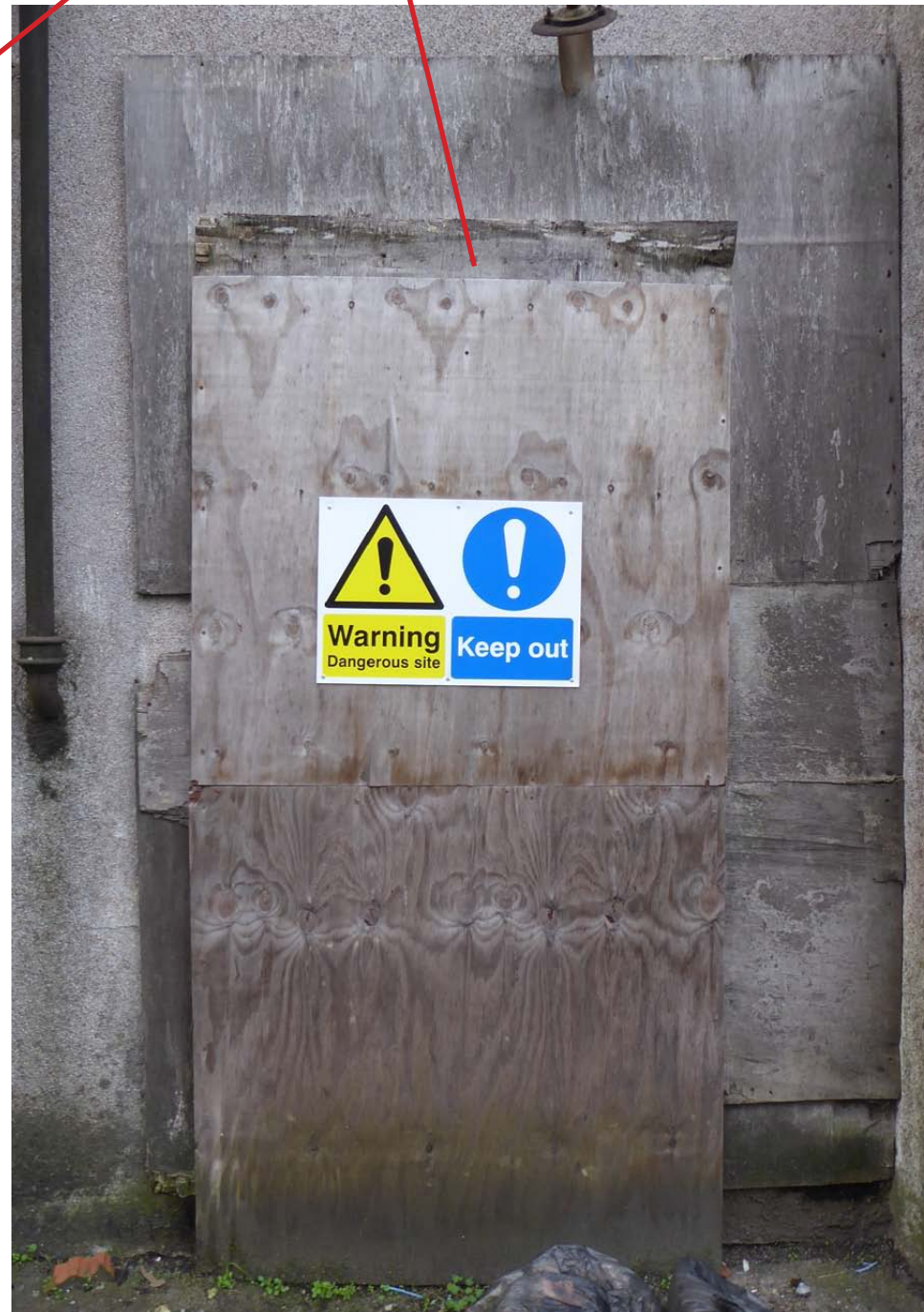
View of boarded up door to ground floor emergency exit from foyer
