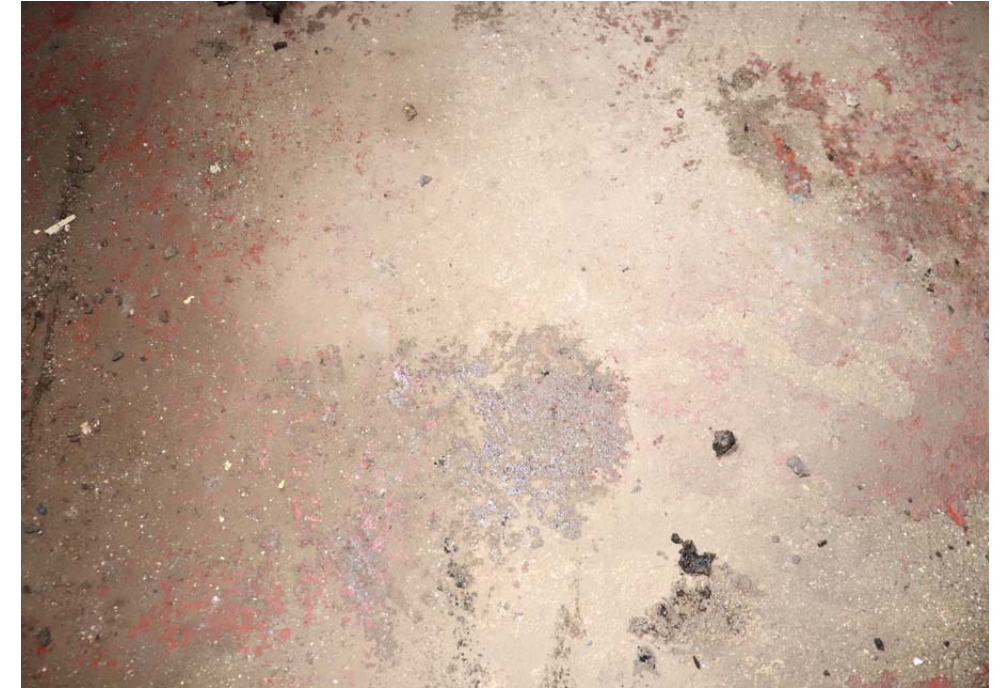
View of painted concrete floor
