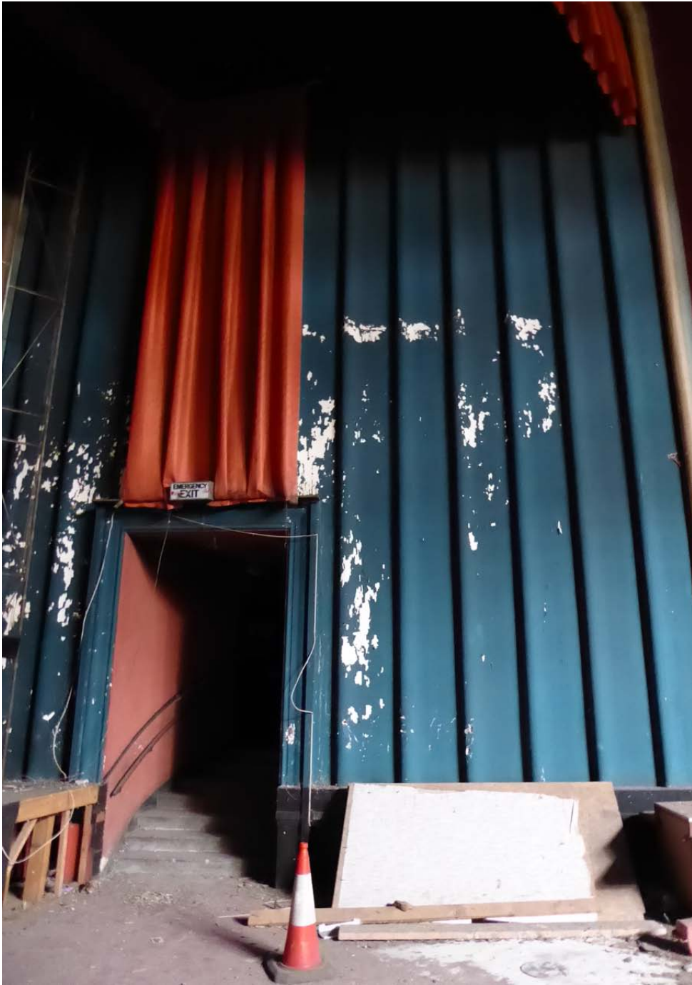
View of profiled acoustic reflector side panelling to stage left
