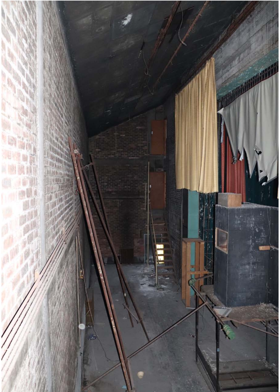
View looking across stage towards east end
