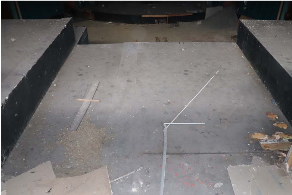
View of timber construction over the top of the central corridor below
