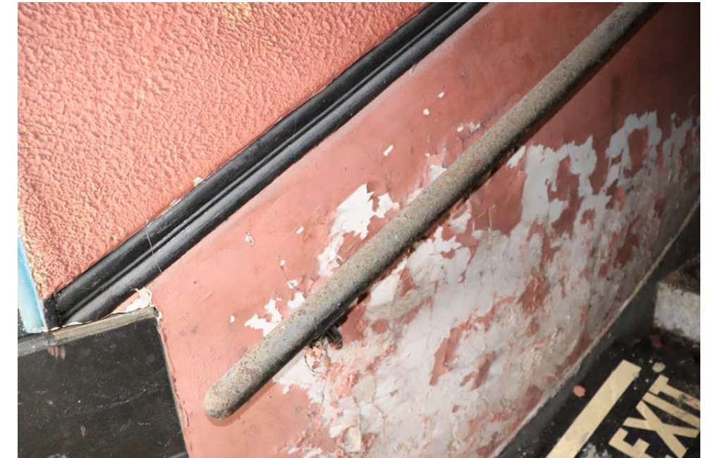
View of round metal handrail & profiled dado above
