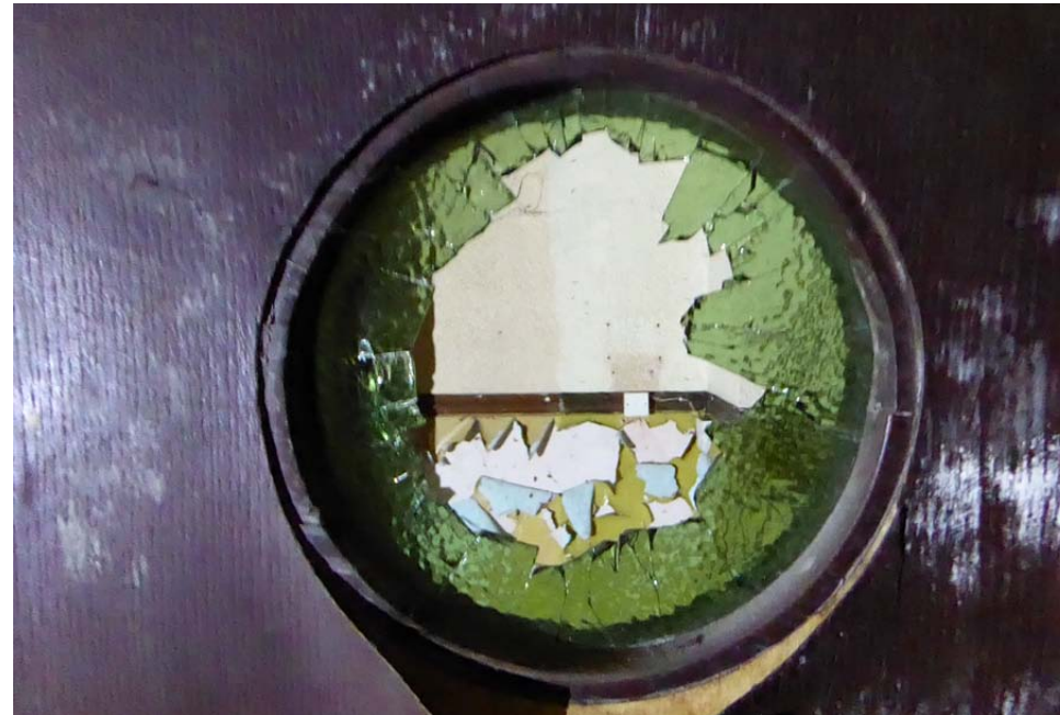
View green glazed circular vision panel to one door
