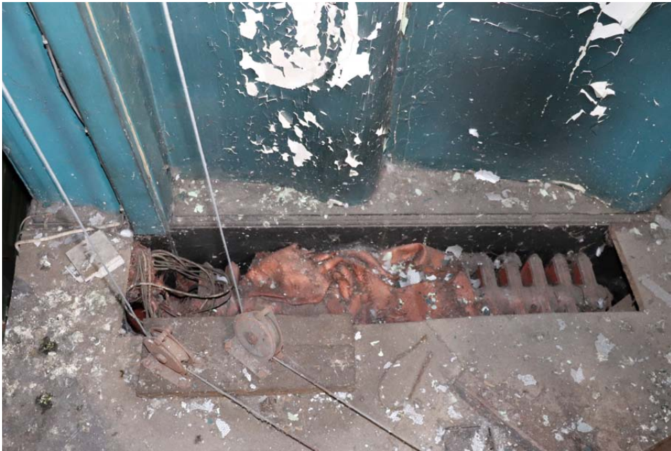
View of recess in stage with cat iron radiator dripped below stage
