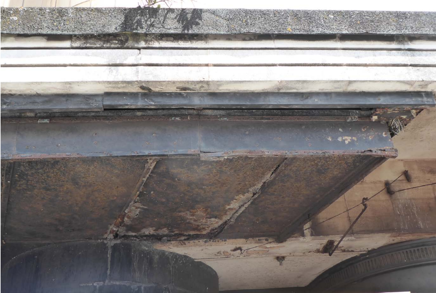
View of edging to metal dropped section to canopy with edging set back from canopy edge
