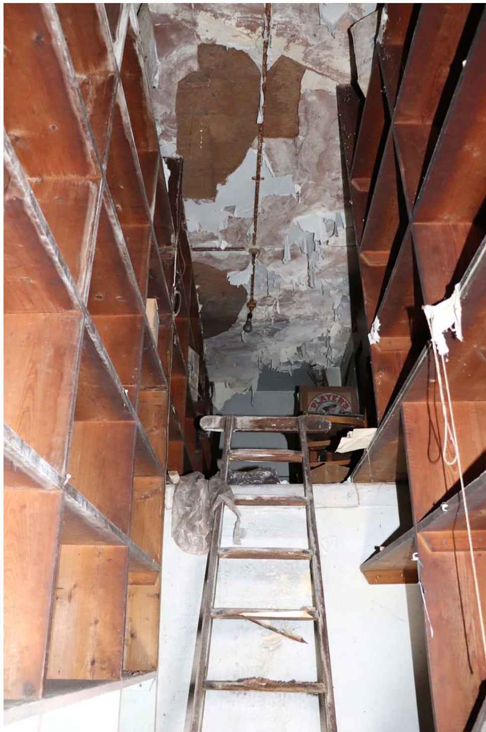
View to east end of Store, over Toilet, with Shelving to both sides
