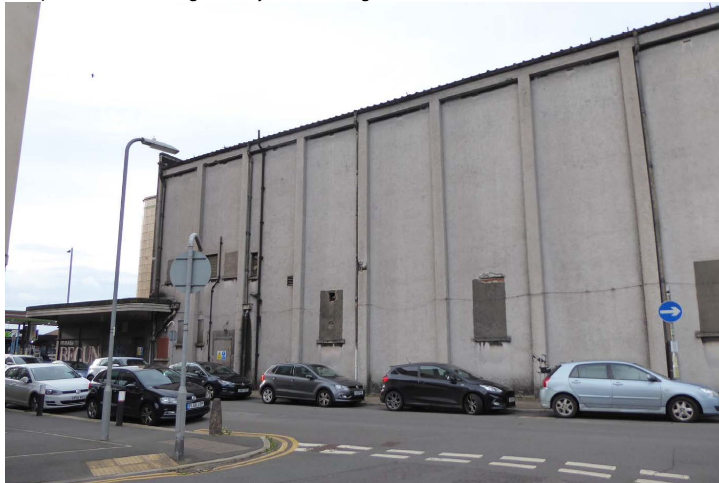
View of left-hand side of Eagle Street (east-facing) Elevation
