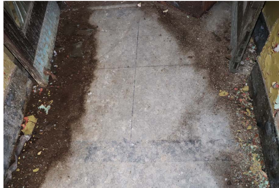
View of terrazzo flooring at top of staircase
