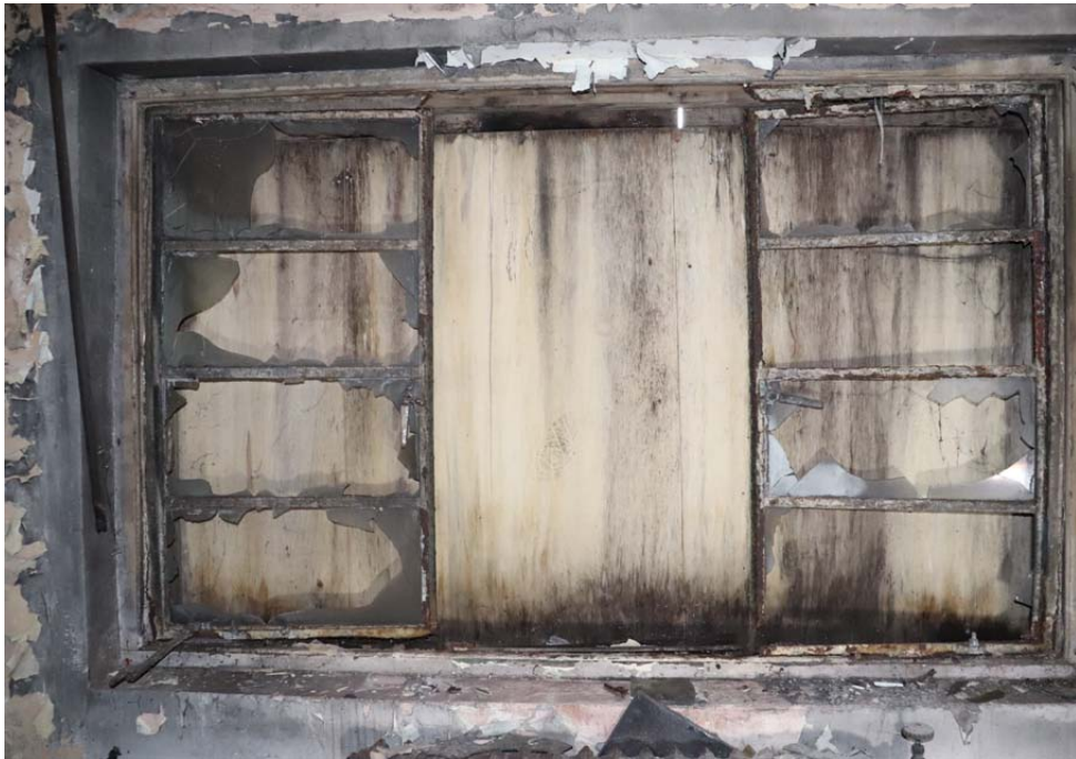
View of window in west wall
