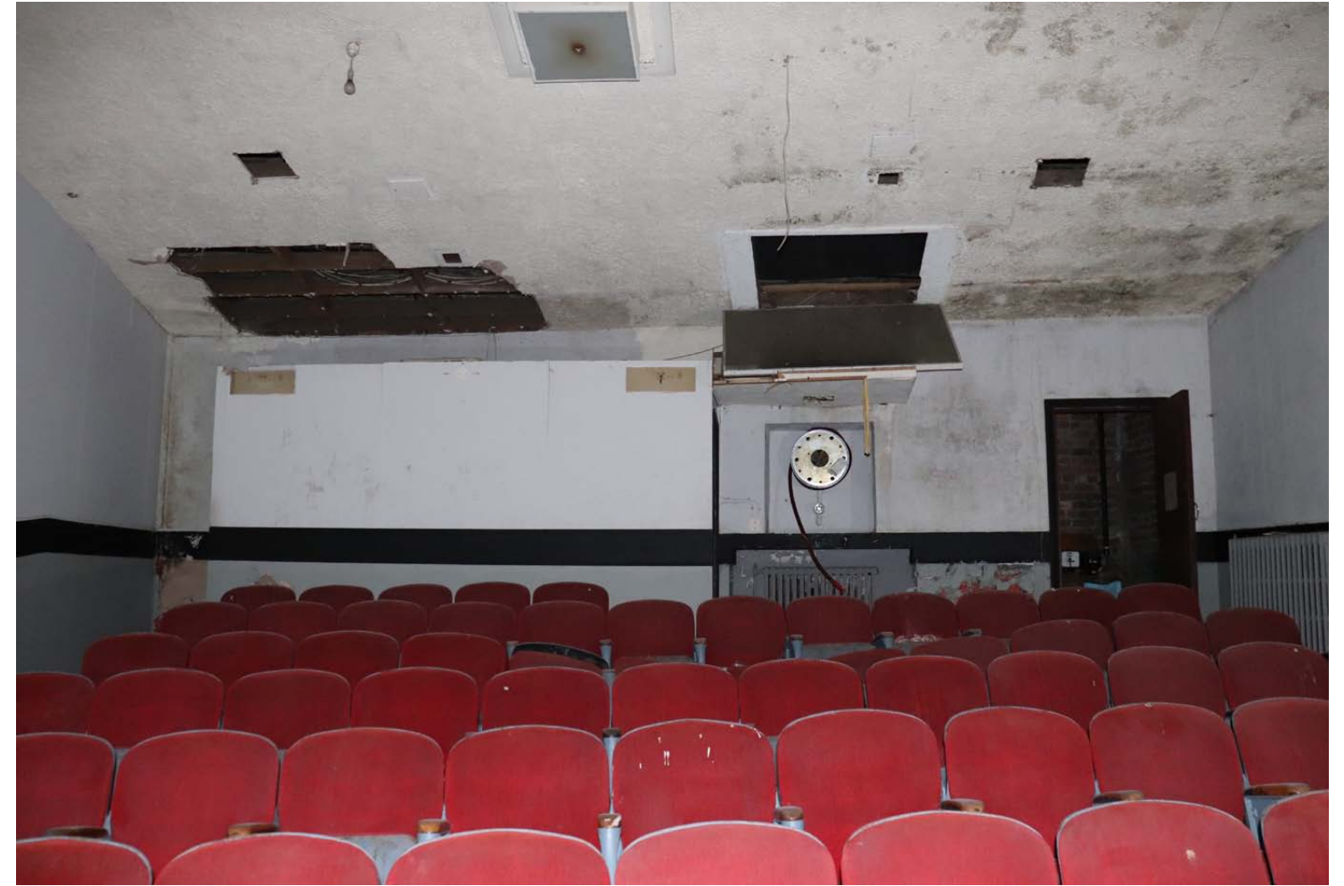
View of Cinema looking south
