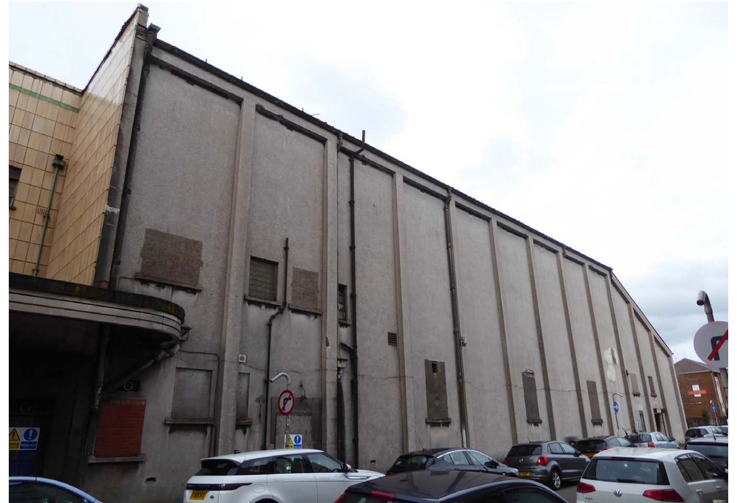
View of Eagle Street (east-facing) Elevation
