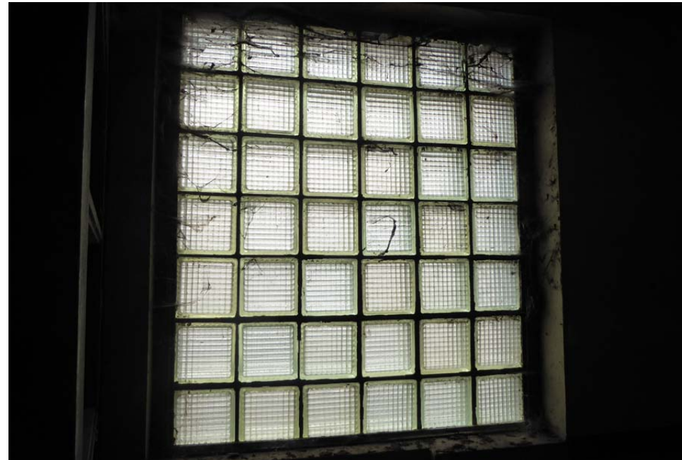
View of glass block window to stair landing
