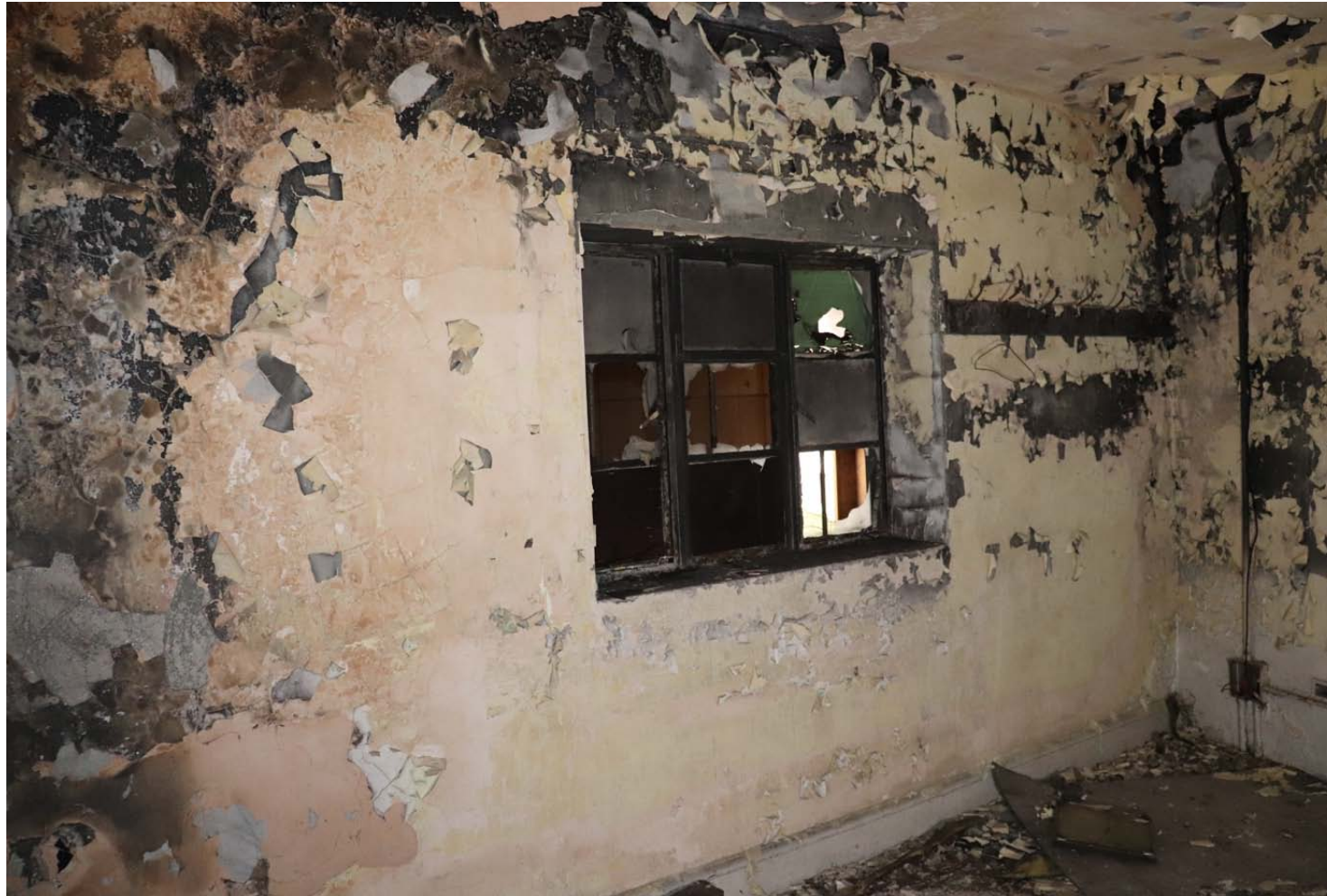
View of east wall with window looking out to recessed roof area
