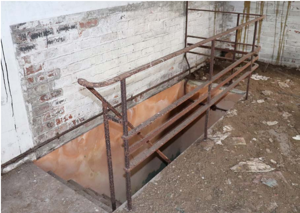
View of steel guardrail around stair void, which is Art Deco in style
