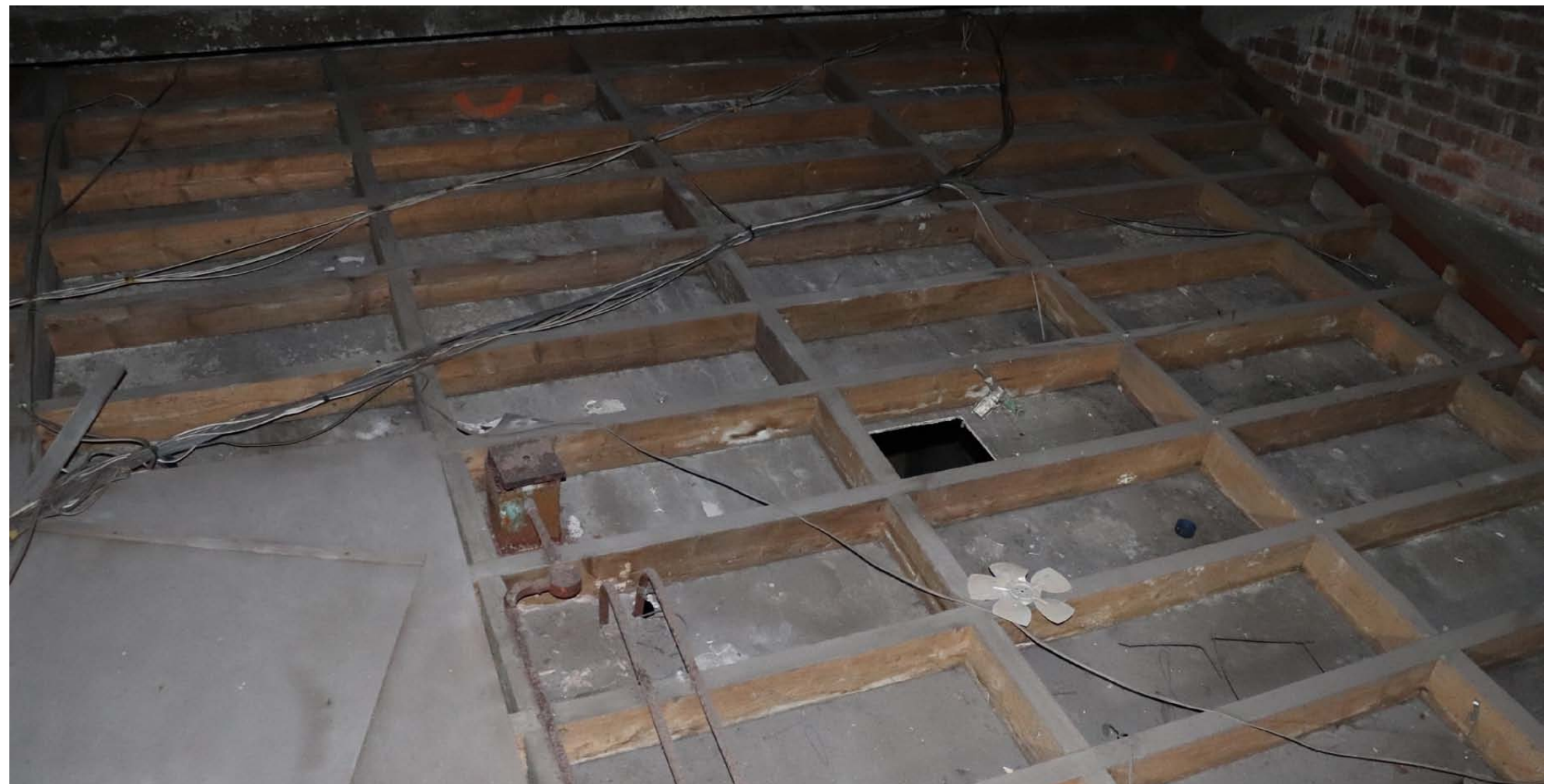
View to void underneath the concrete auditorium balcony seating showing the timber-framed ceiling over the cinema below
