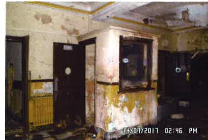
Foyer area ticket booth, July 2017
