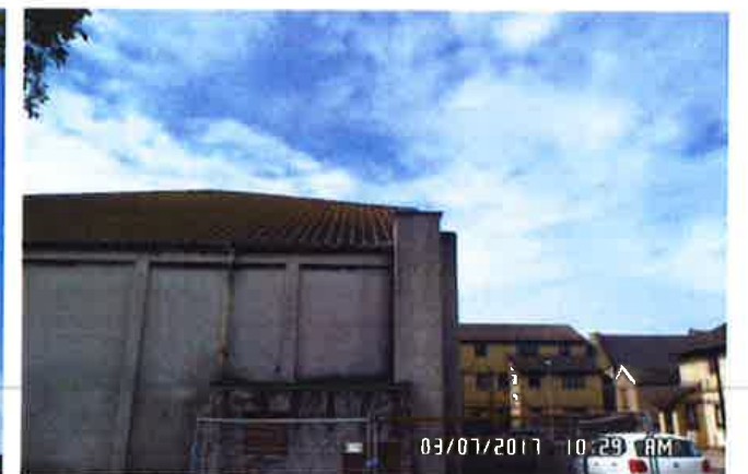
Rear Chimney cracked and leaning (June 2017) Top portion of chimney removed (July 2017)
