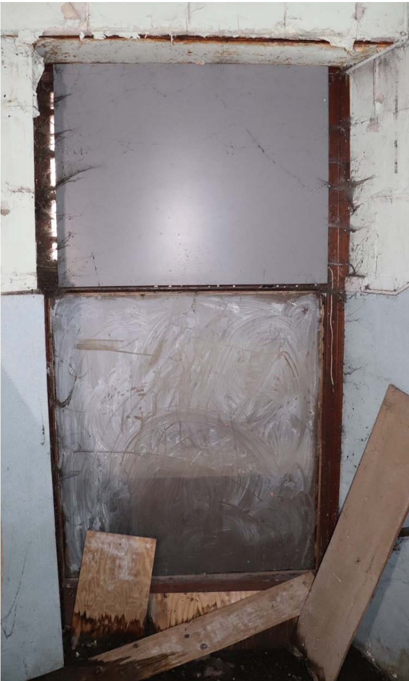
View of west wide timber-frame glazed screen
