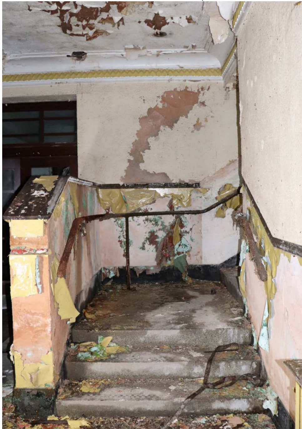
View of bottom flight of staircase with low wall to left
