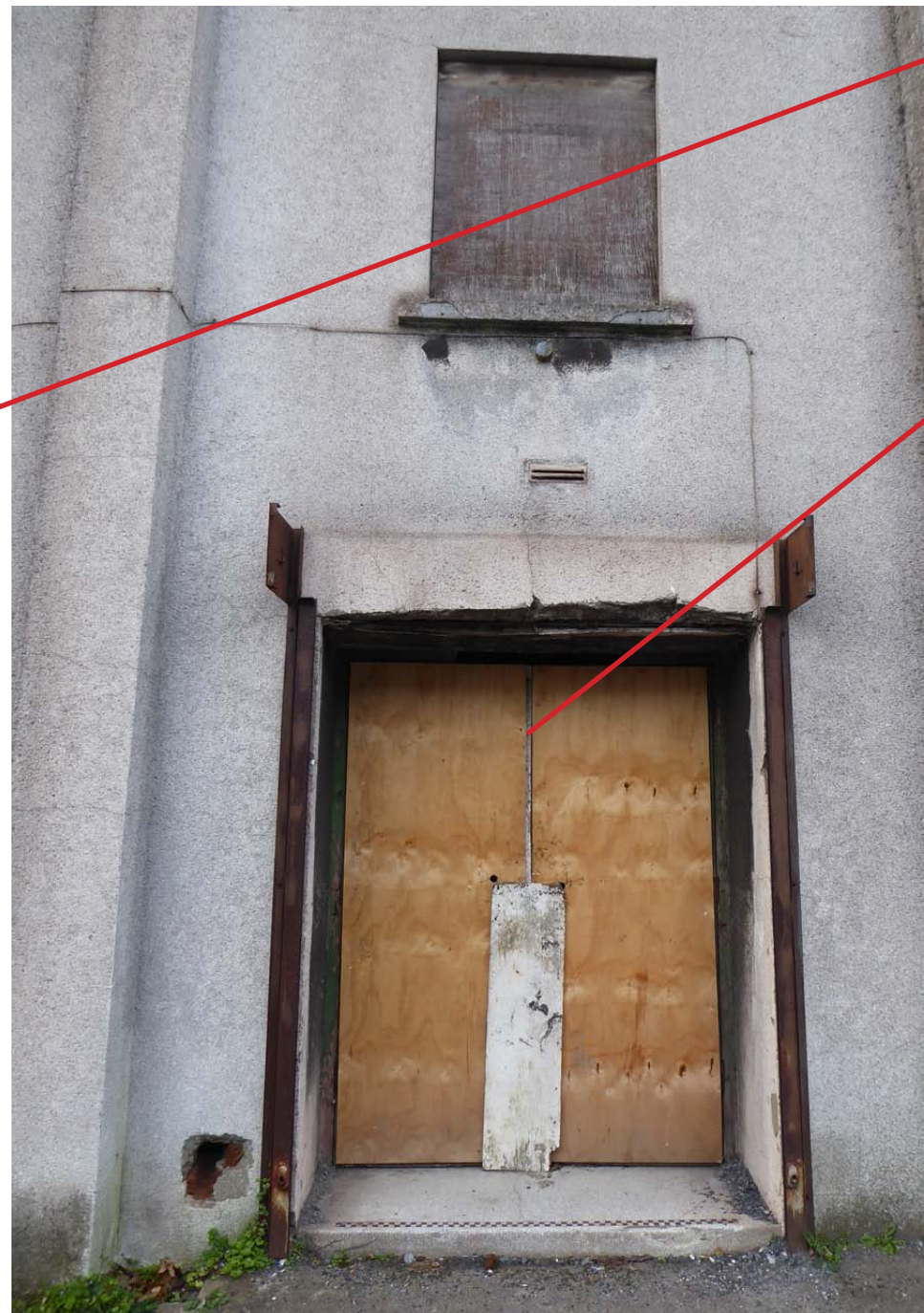
View of boarded up emergency exit door from auditorium
