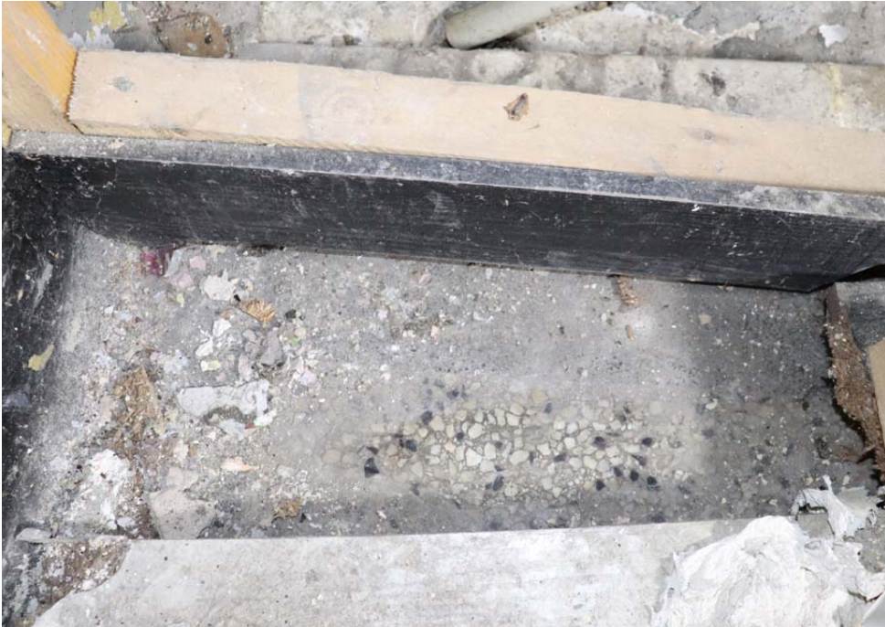
View of grey insitu terrazzo to the toilets
