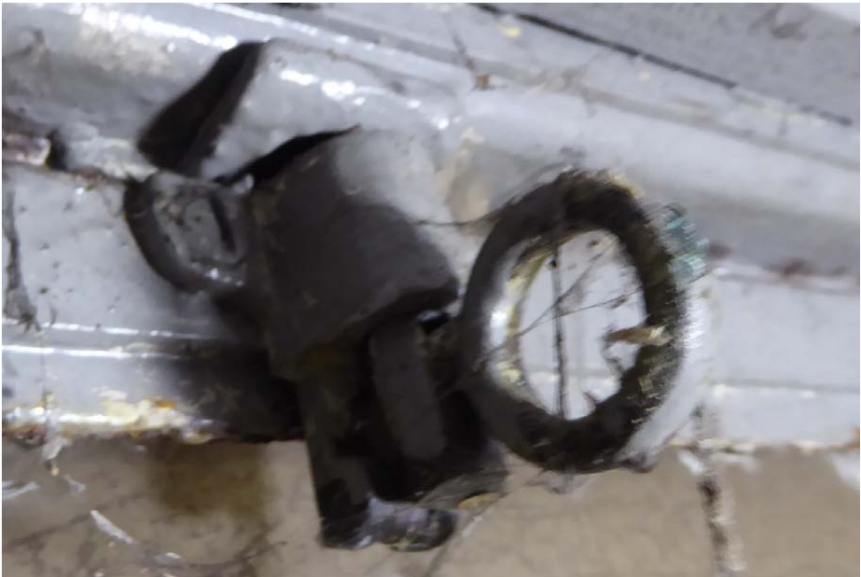
View of finger-pull latch to top bottom-hung opening light
