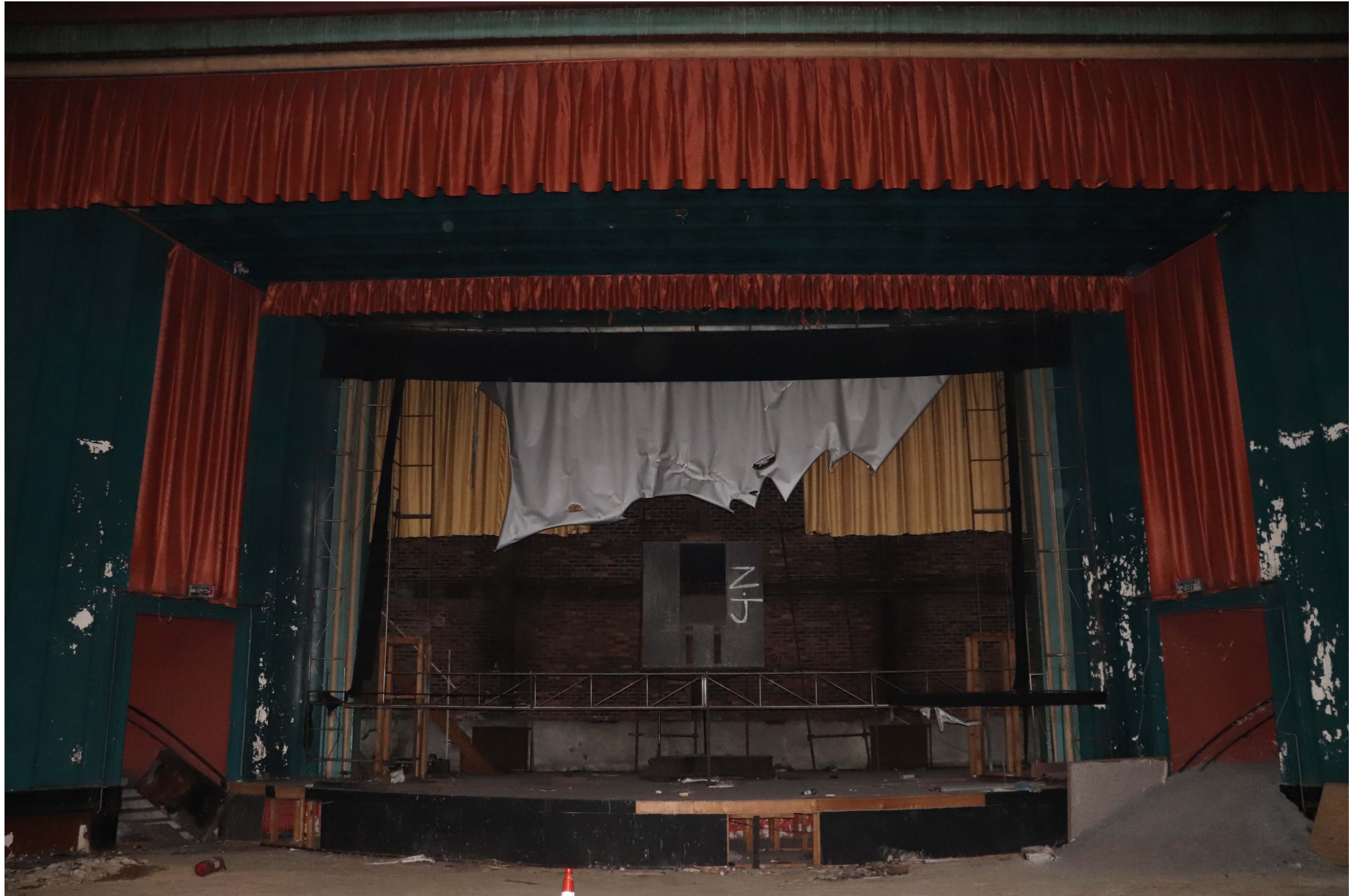
G17 - Auditorium - View looking from auditorium space towards Stage with curve fronted timber raised stage and series of drapes in front of proscenium arch
