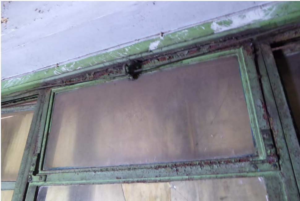
View of top bottom-hung opening light
