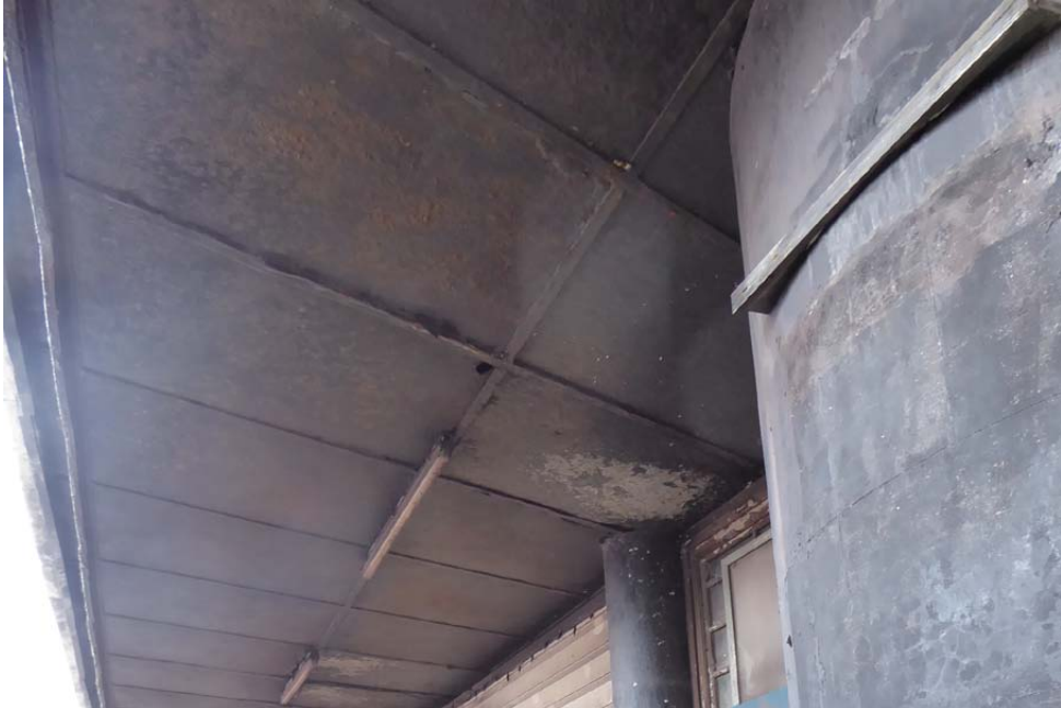
U Metal Downstand to Canopy to be Replicated
