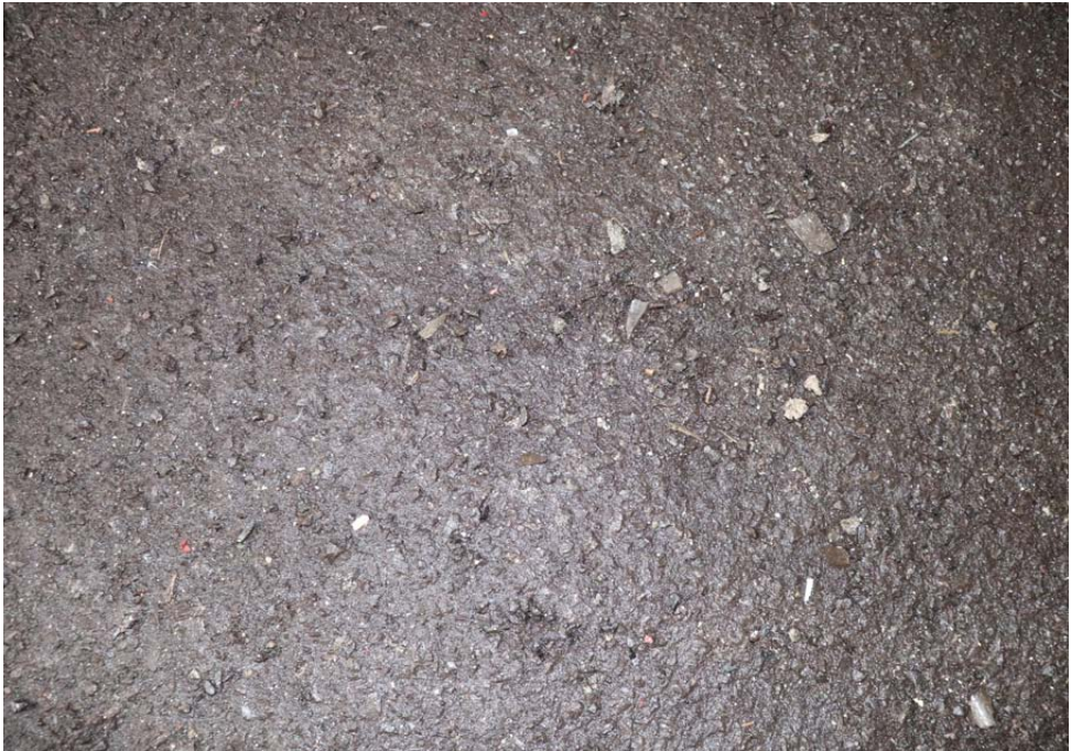
View of the asphalt roof
