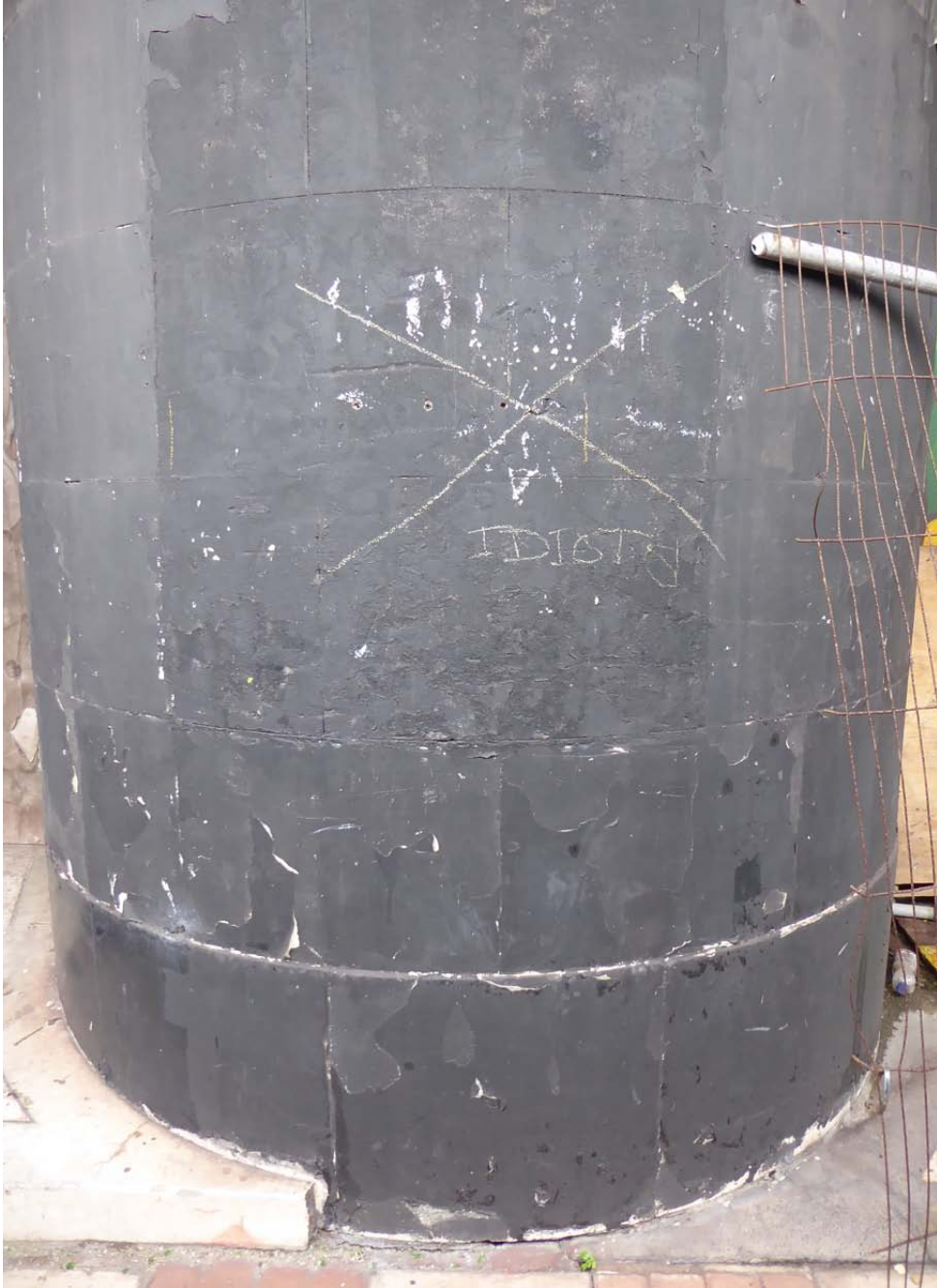
L Black painted Masonry Stall riser & Curved bay
