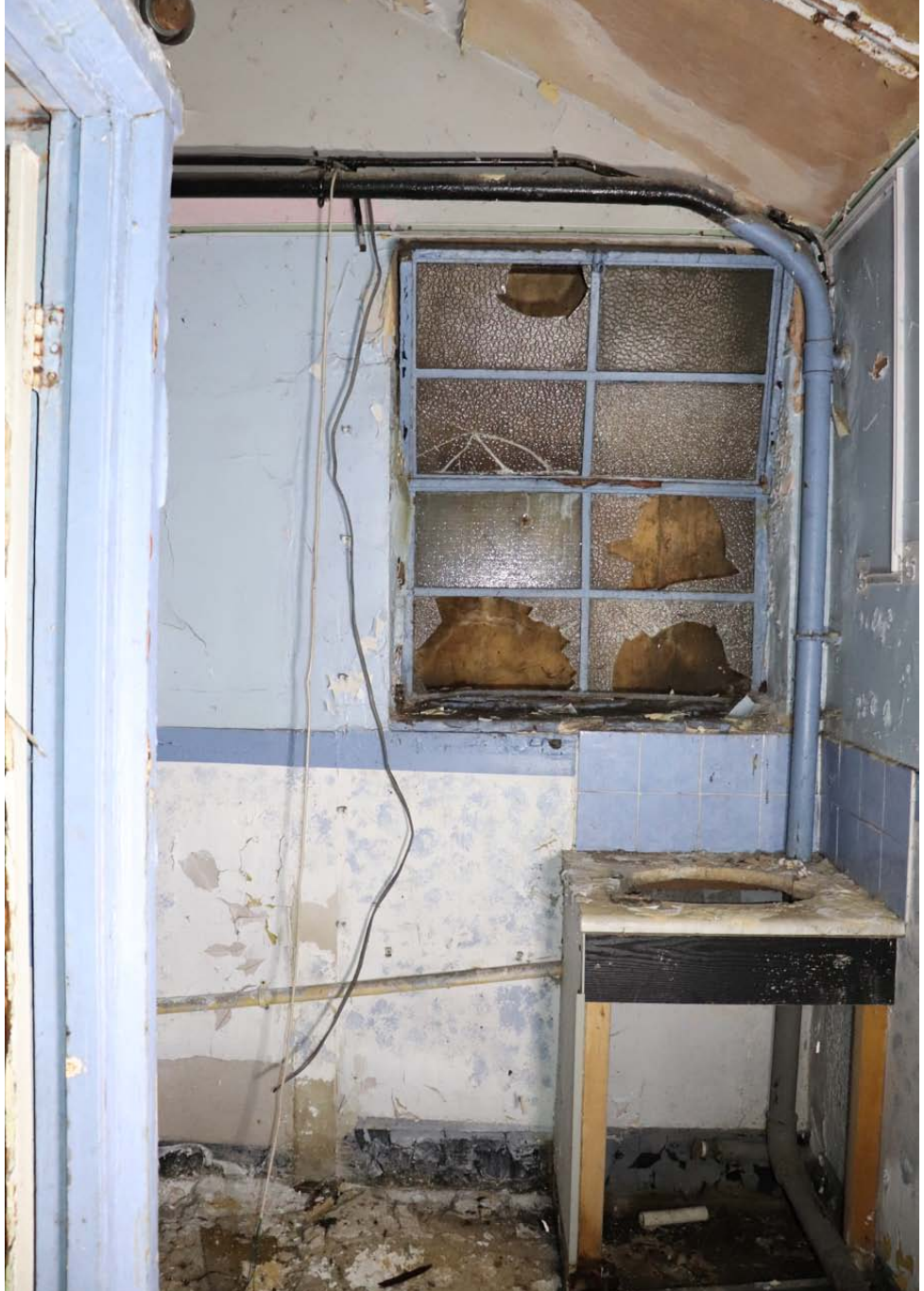
View of the larger window to the east elevation
