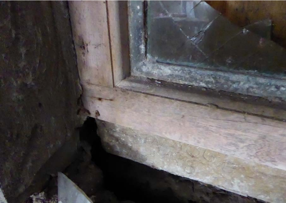
View of example of timber sub-frame to windows
