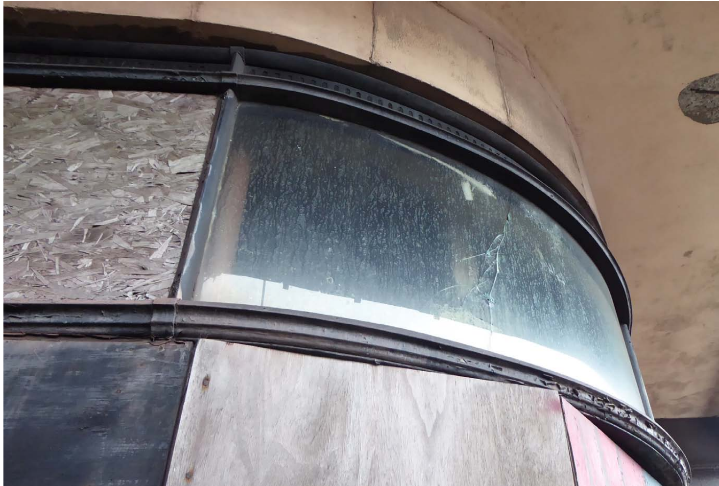
Views of top of curved frontage to timber-framed glazing to the larger (right-hand) Retail unit, showing profile to timber head section and lower transom section and vertical glazing bar with aerofoil profile
