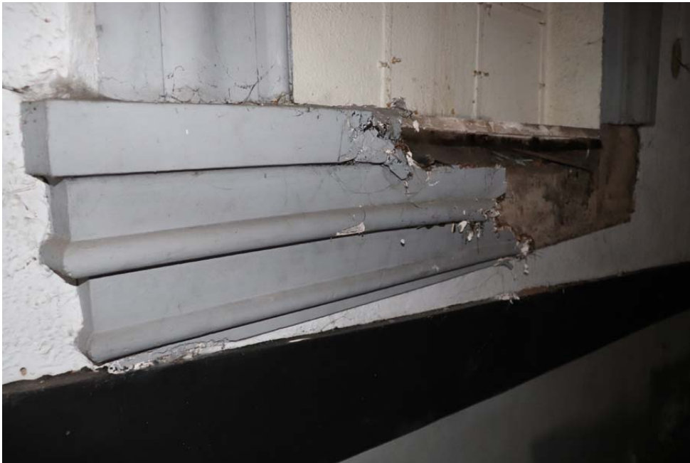
View of plaster profile to front face of window cill
