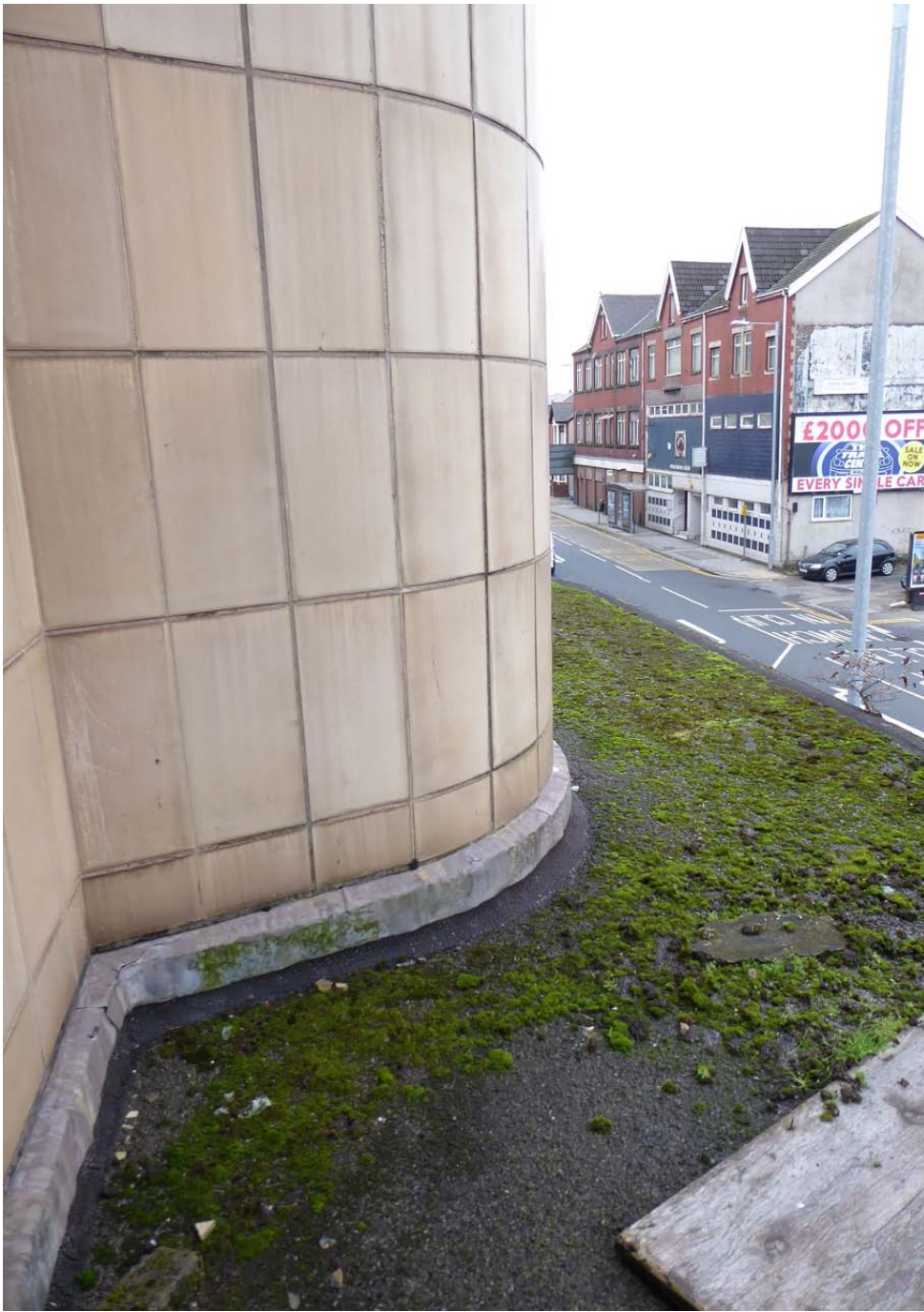
View looking eastwards
