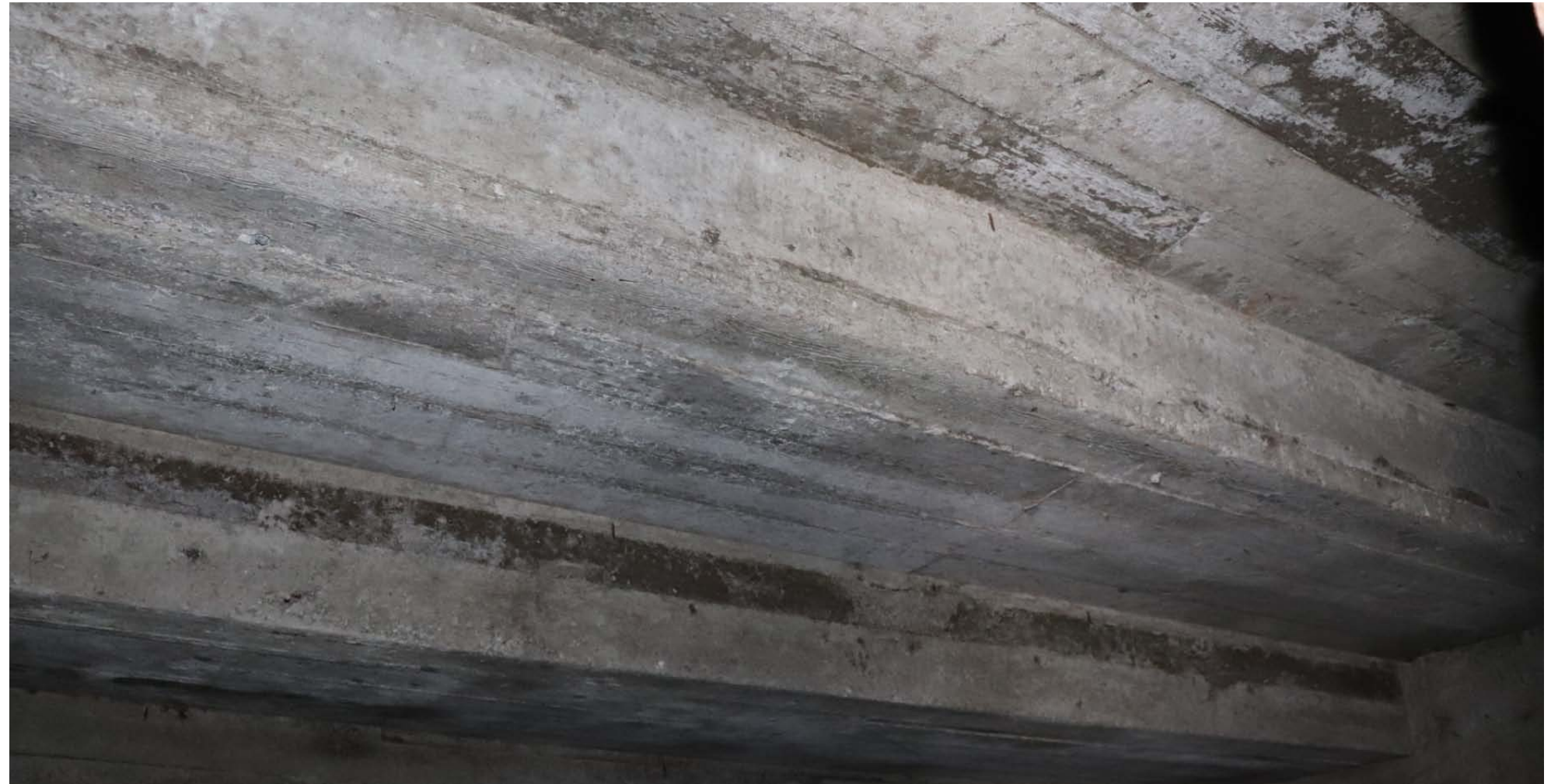
View to void underneath the concrete auditorium balcony seating
