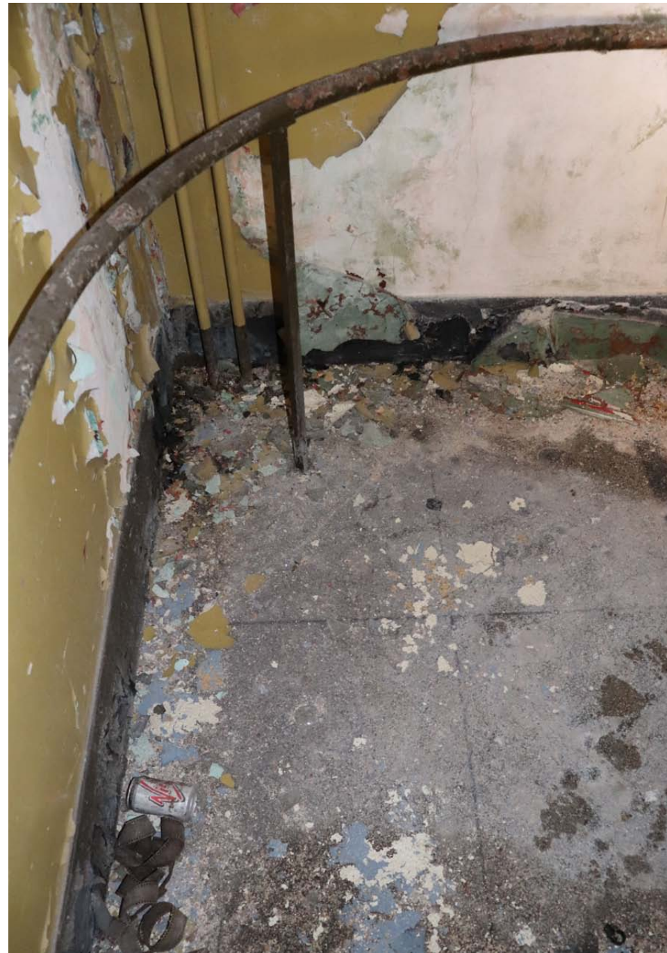
Simple round steel handrail curving inside the square corner
