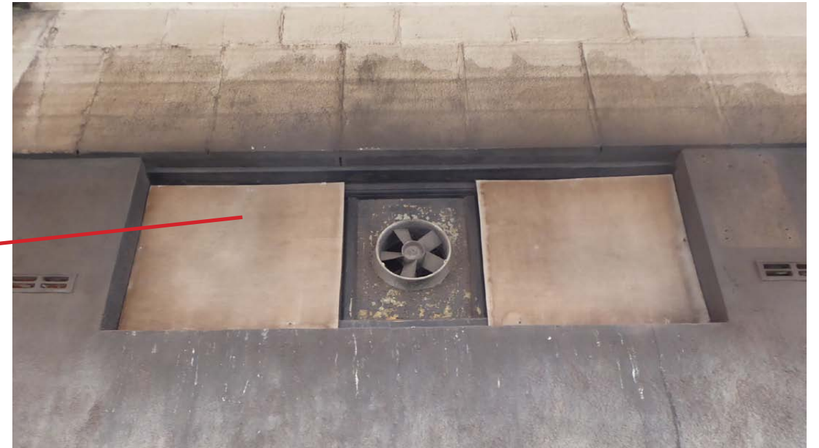
View of part-boarded vent to rear of ground floor to Retail unit
