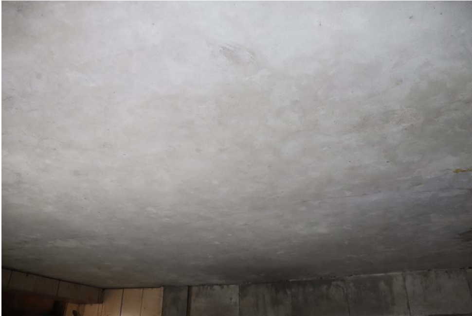
View of plastered ceiling / soffit
