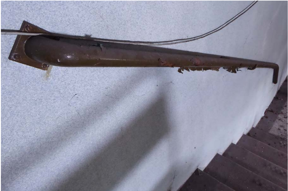
View of the painted steel round handrail on the east side wall
