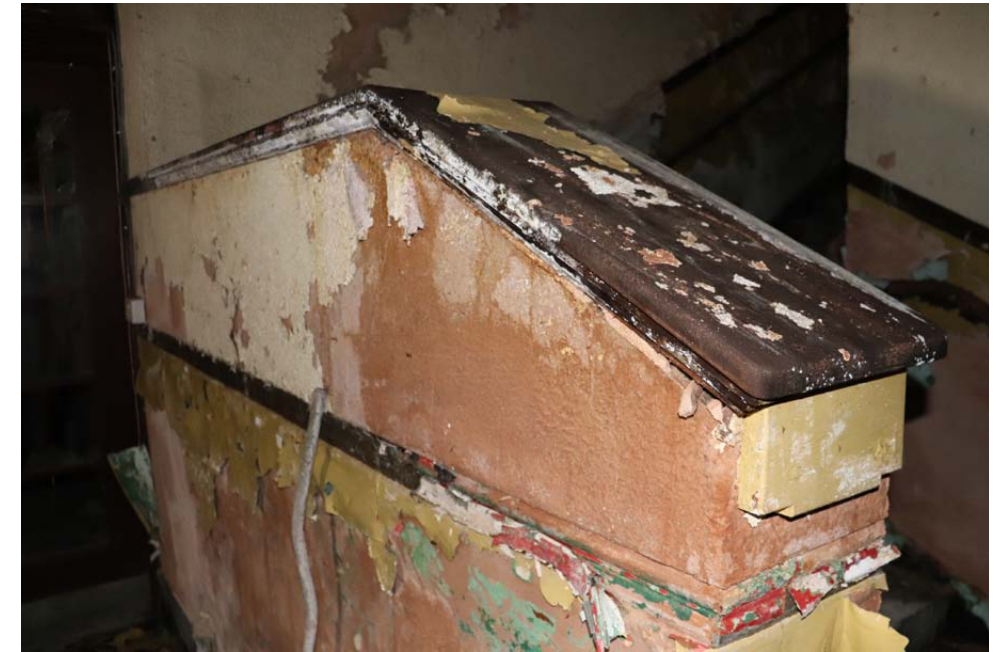
View of low wall with timber oversailing capping.
