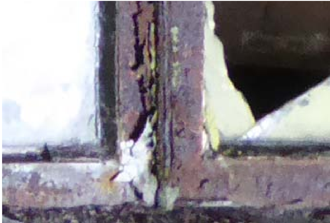
View of corrosion to steel frame sections at mullion
