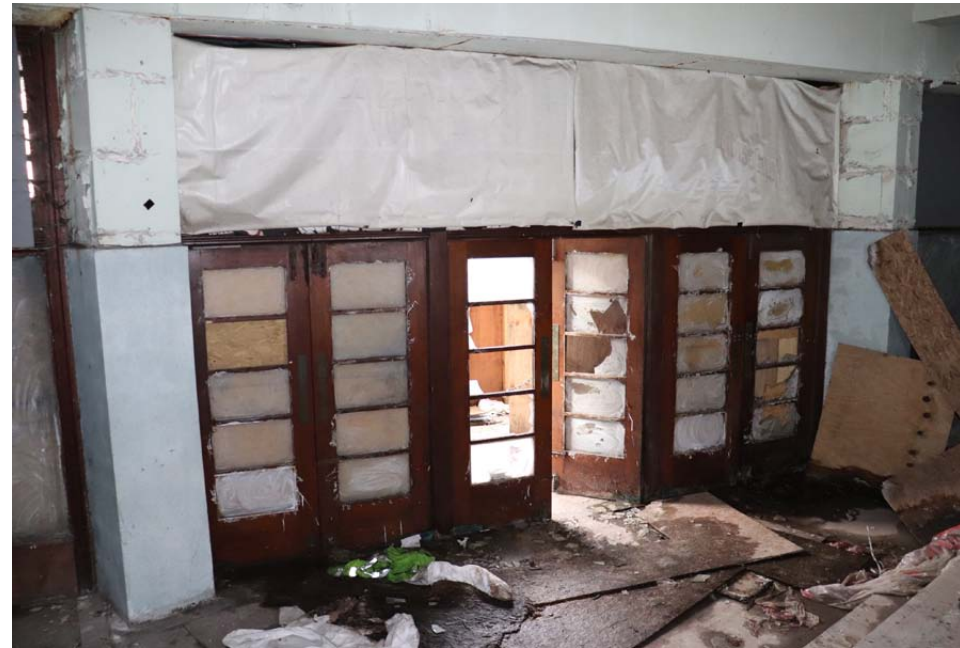
View of Central Bank of 3no. Double Doors
