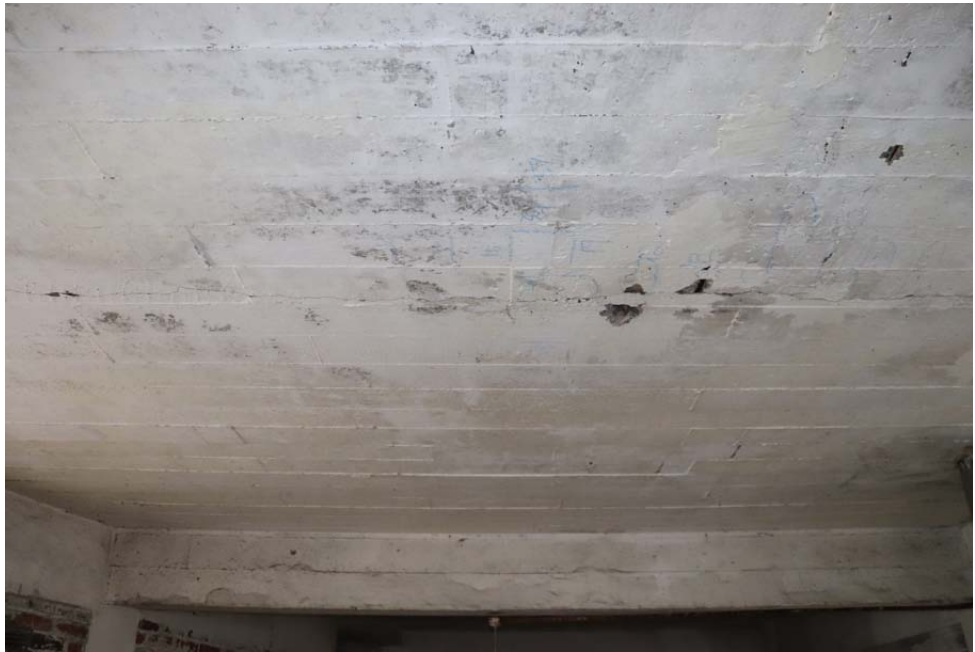
View of slim precast concrete units to soffit, painted white
