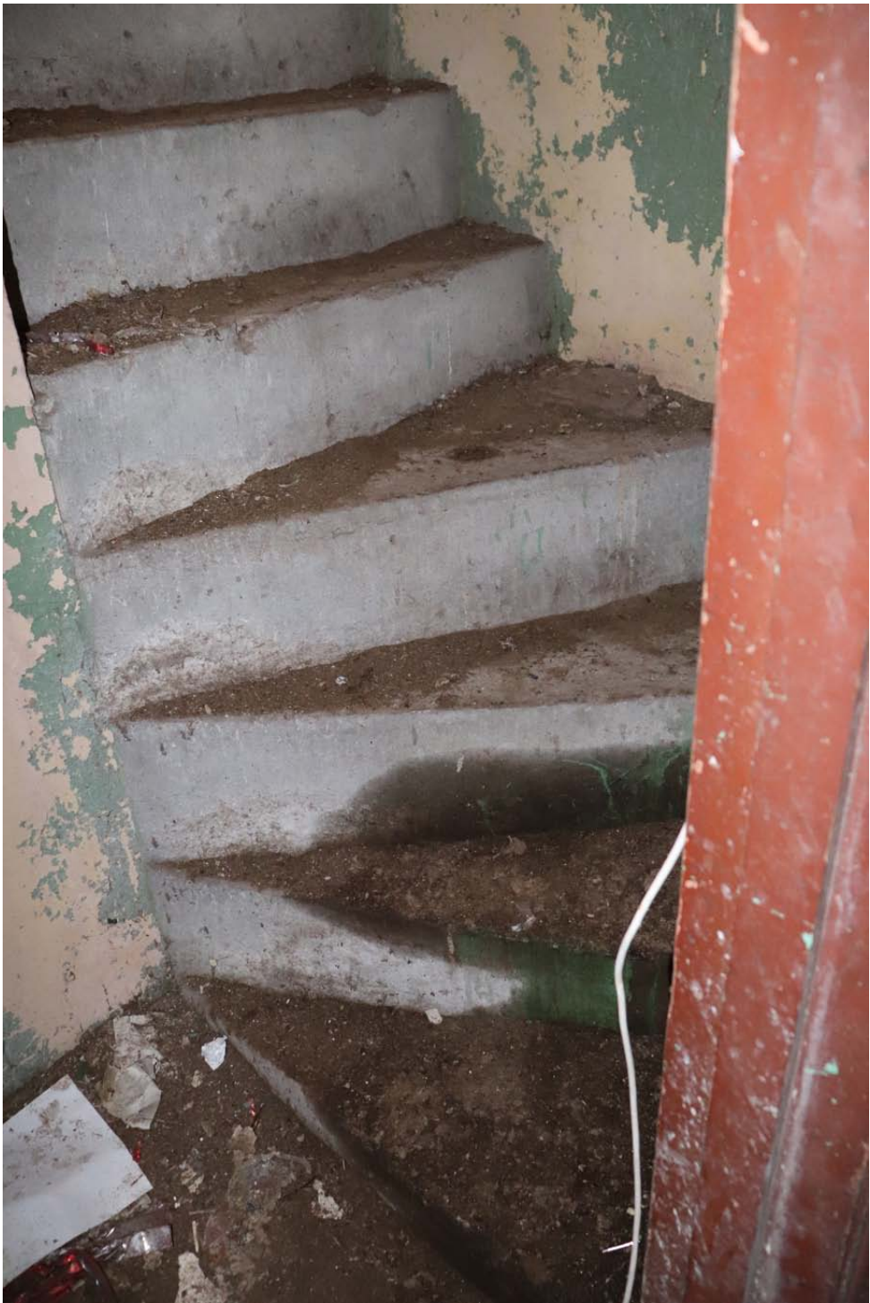
Spiral concrete staircase leading from first floor to second floor
