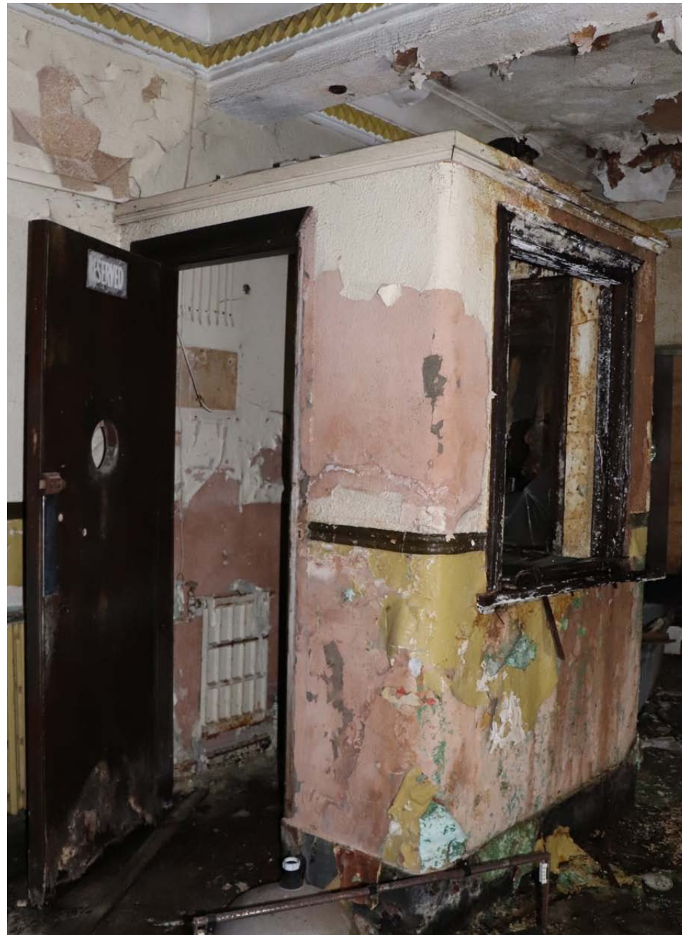
View of the box office enclosure from the west
