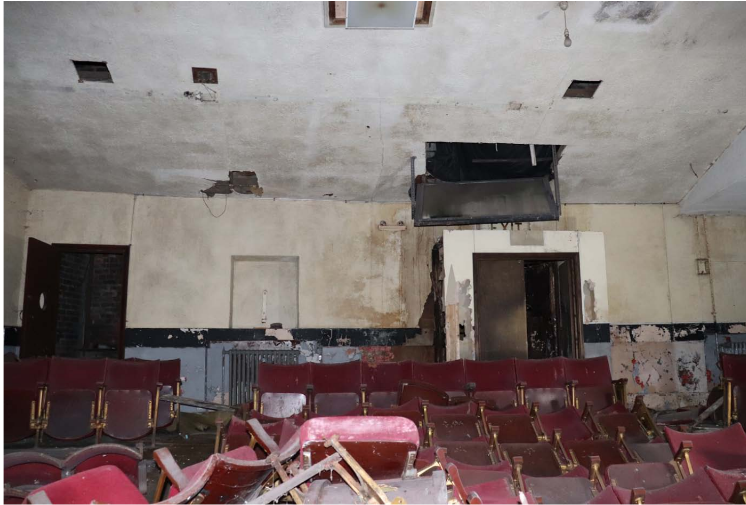
View of Cinema looking south
