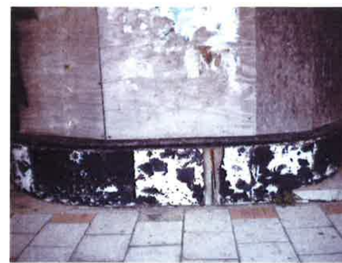
Cladding panels below window 2012
