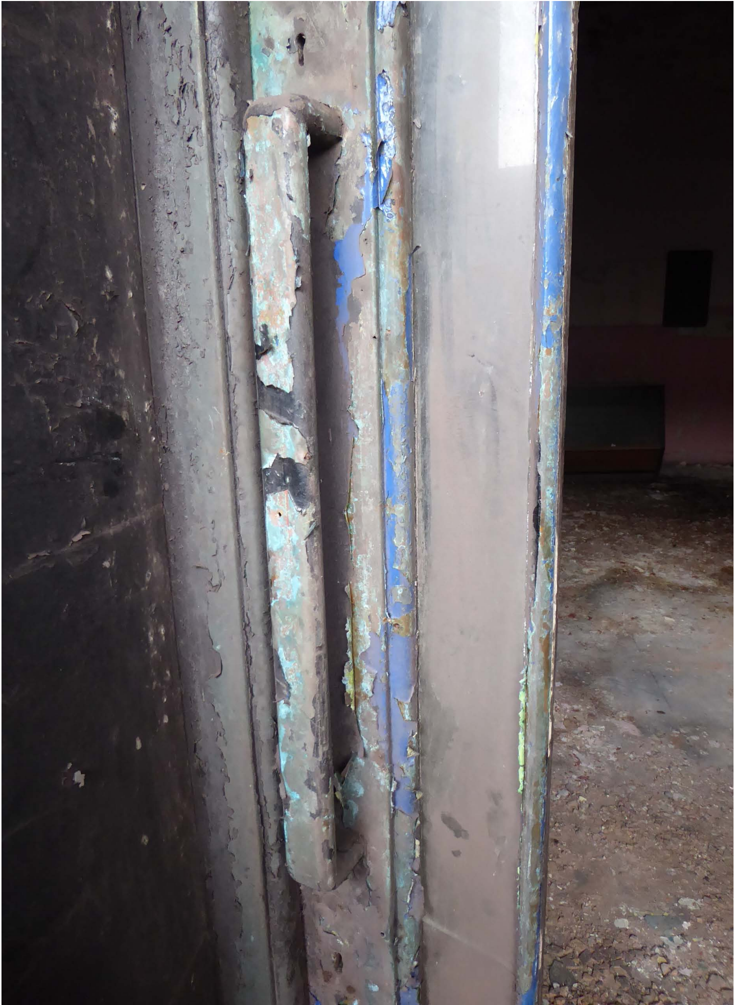
View of side of steel-framed glazed door to right hand retail unit with pull handle & perimeter glazing
