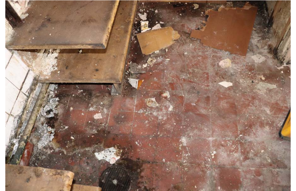
View of Terracotta-coloured small unit Quarry Floor Tiles
