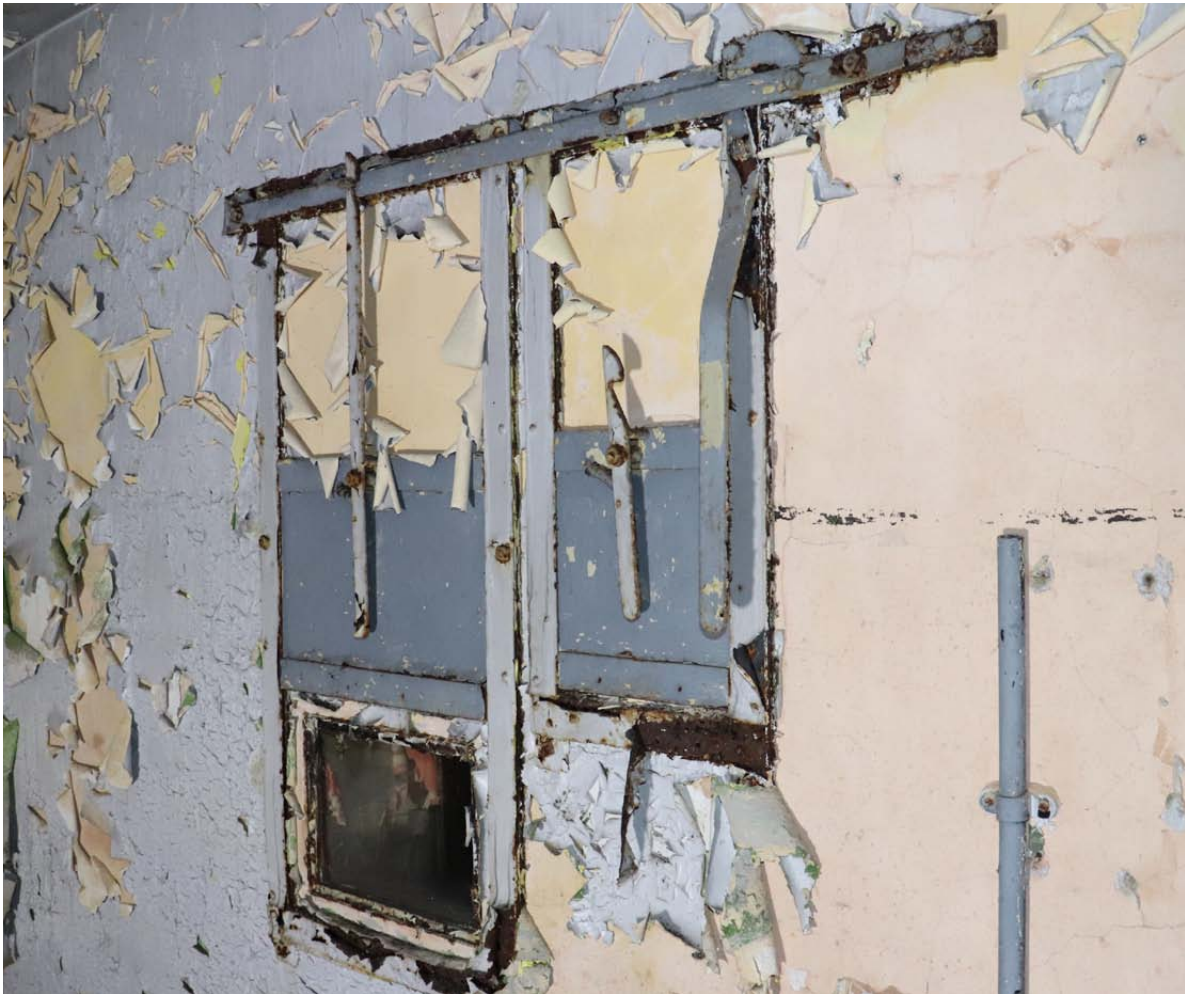
View of left hand openings with sliding covers
