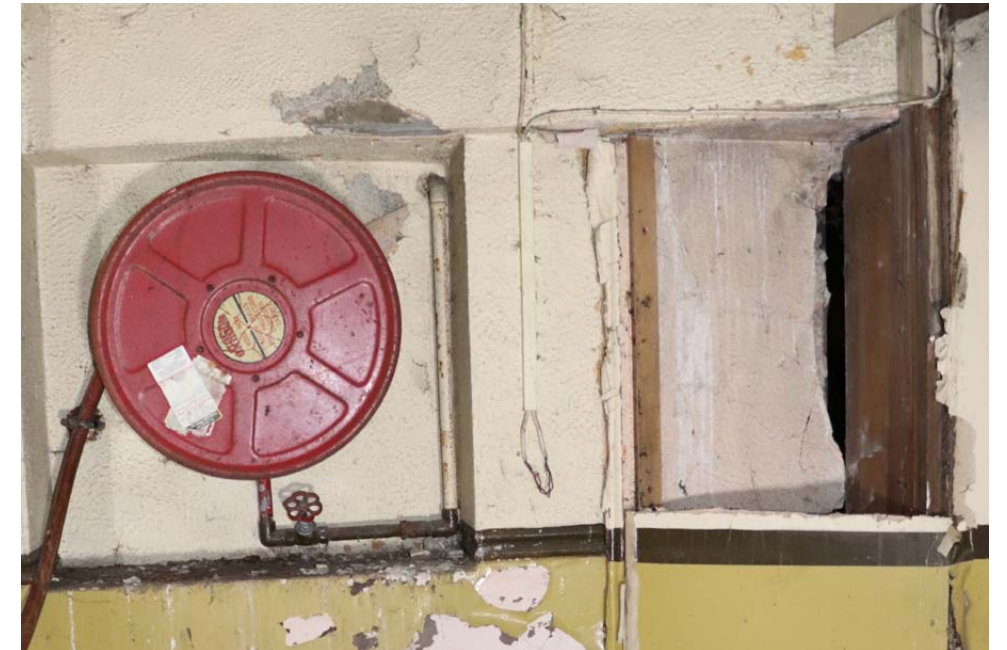
View of end wall at top of staircase with recess for hose reel
