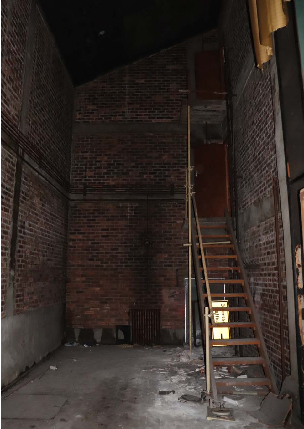
View across stage towards east end with steps to lighting position
