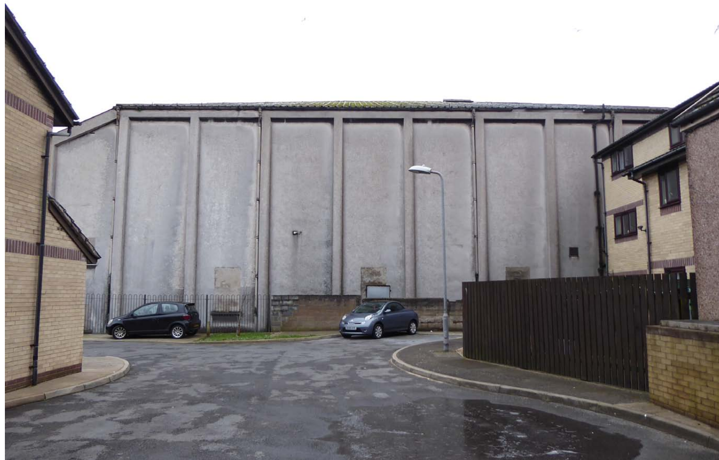
View of central section of west elevation looking from Eagle Mews
