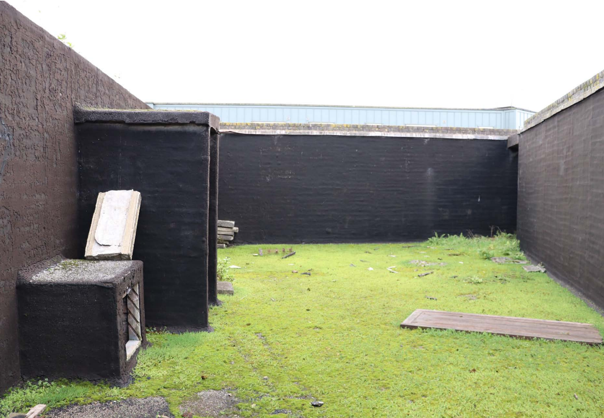
View looking eastwards
