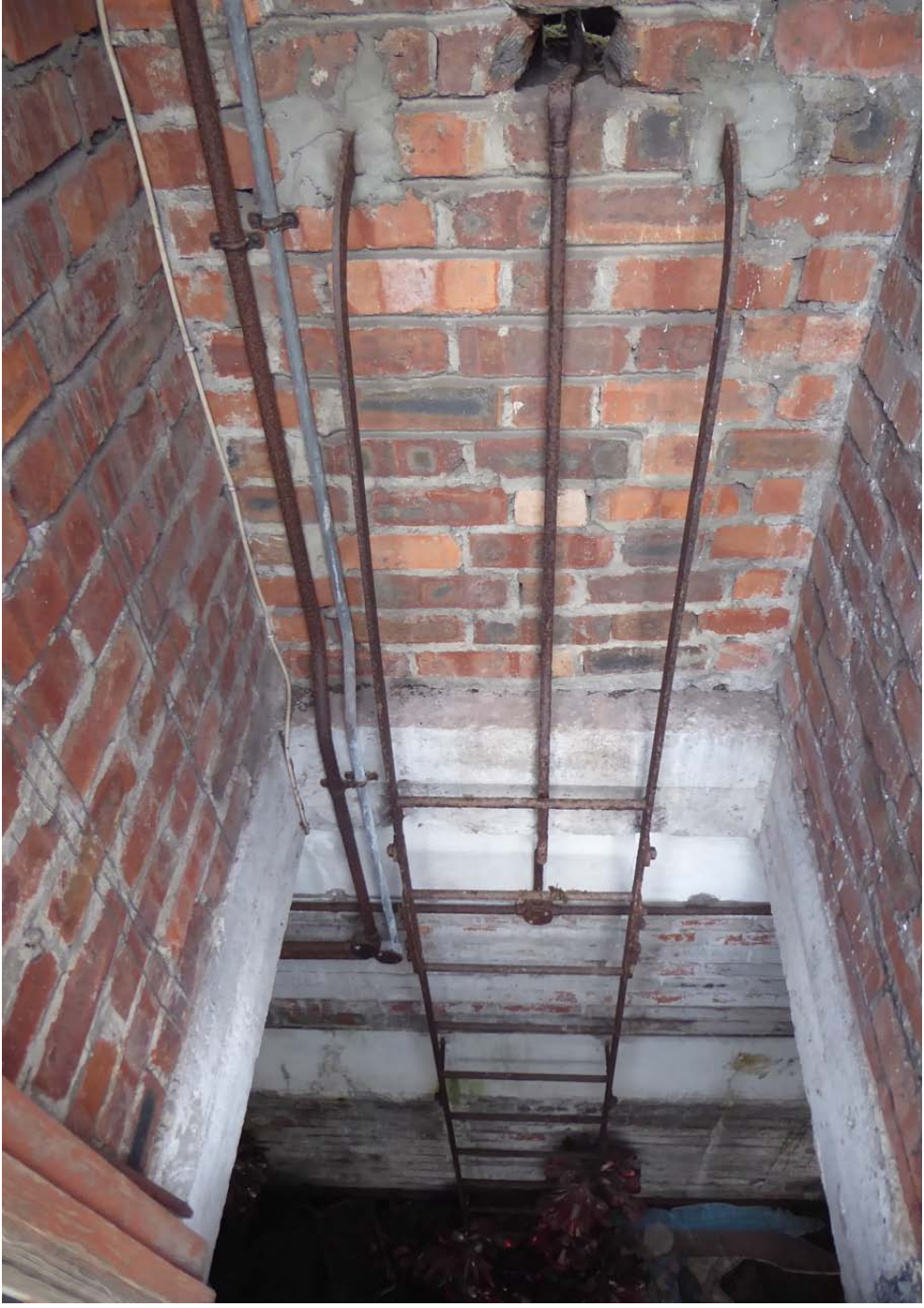
View of interior of box construction to ladder access, looking down
