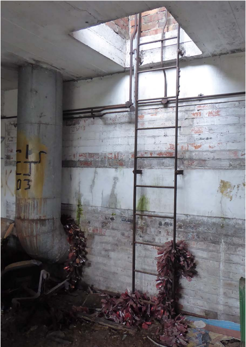
View of steel ladder to access roof & galvanised steel duct
