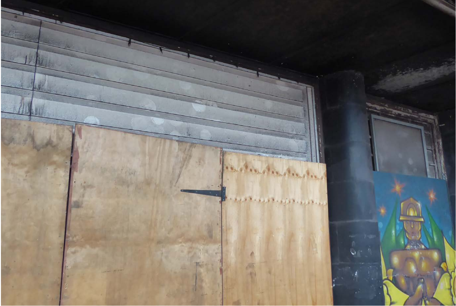
View of right hand side of louvres & overhead panel over the top of the bank of main entrance doors & screen
