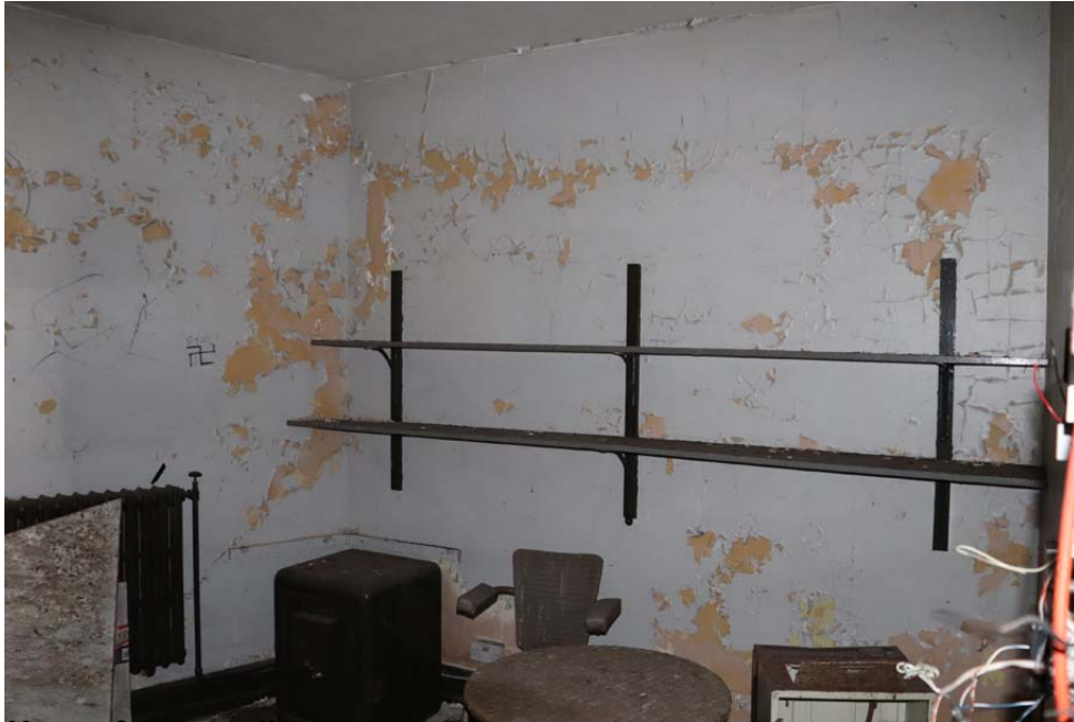
View of west wall
