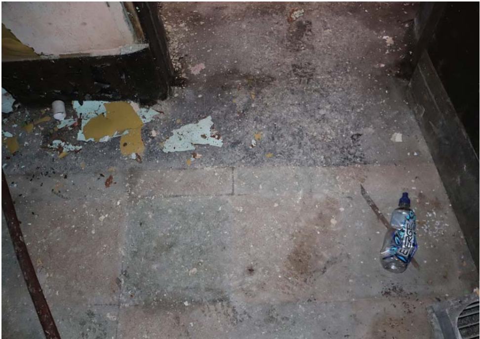
Views of green and yellow terrazzo tiling leading into an grey insitu terrazzo to the toilet lobby
