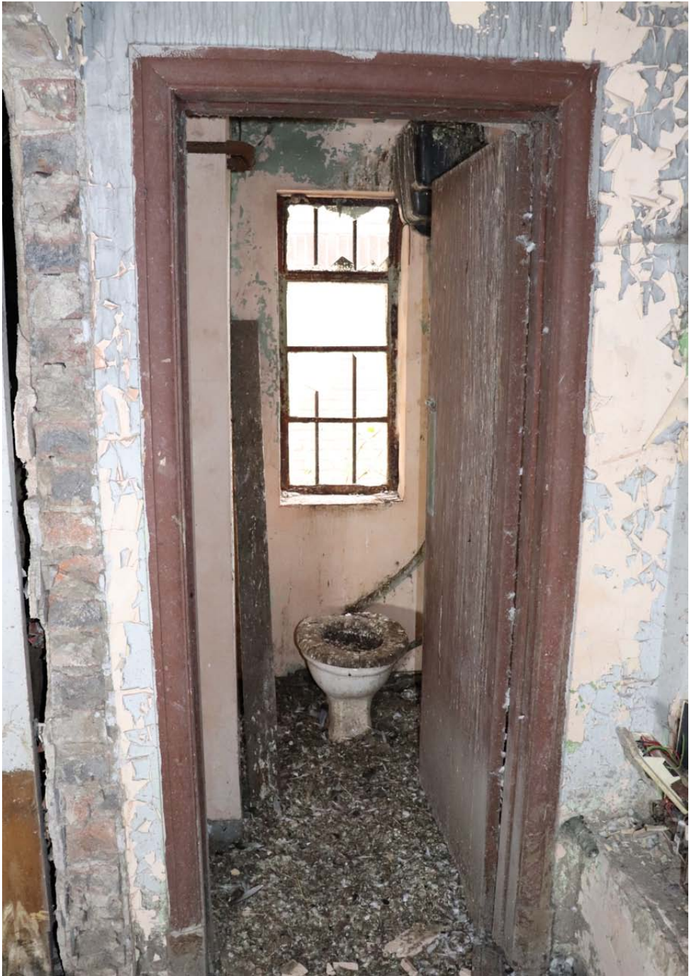
View of Toilet at top of staircase
