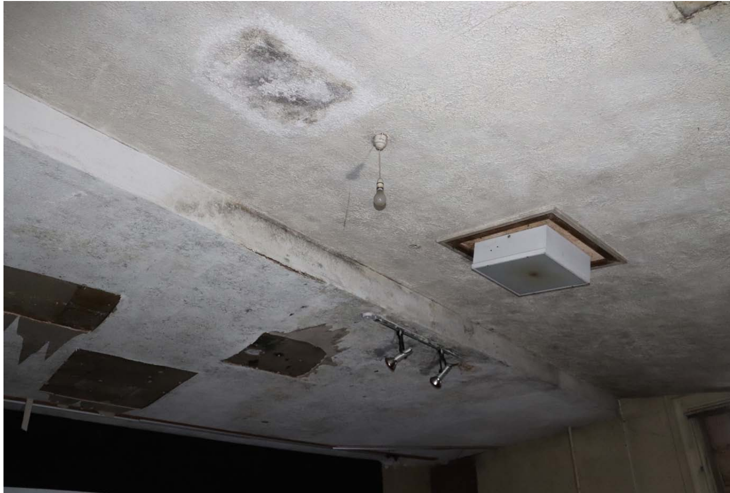
View of ceiling to soffit underneath main auditorium balcony with dropped section for service zone
