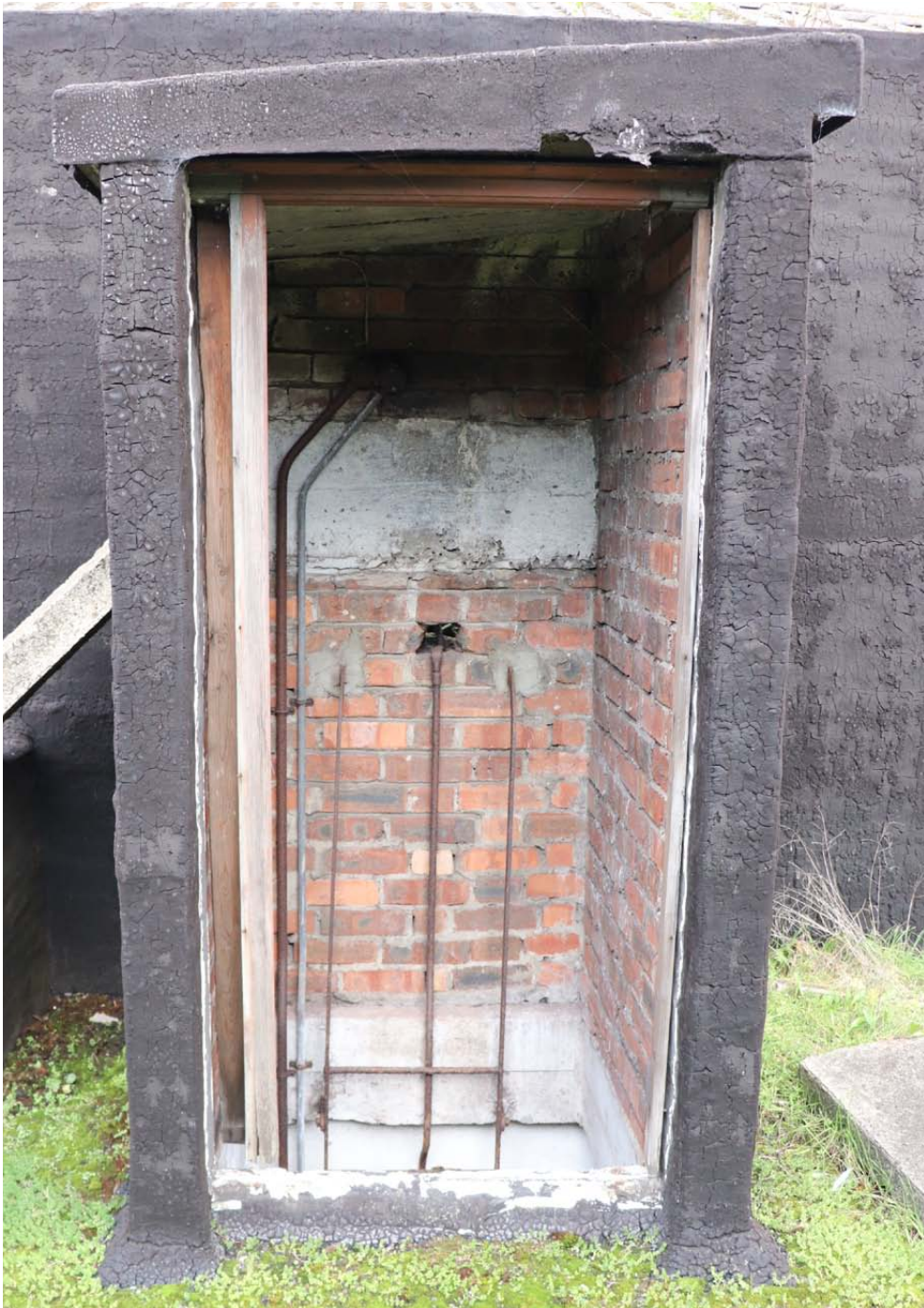
View of box construction to ladder access - straight on
