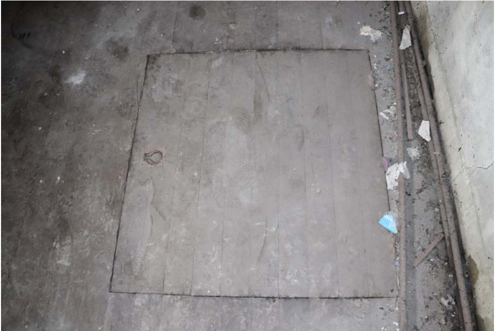
View of access hatch within stage at rear
