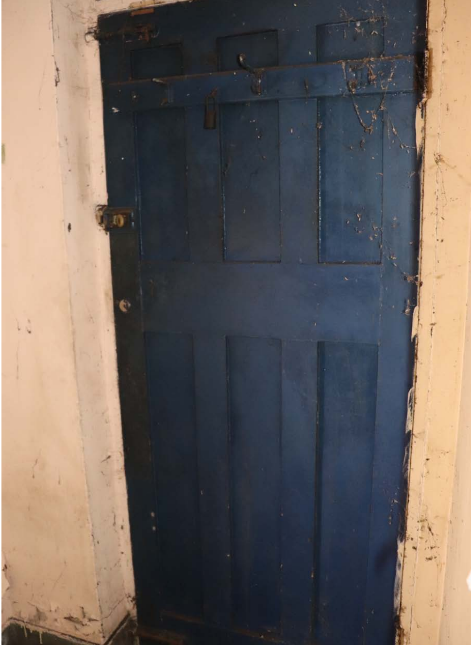
Framed and Panelled Blue-painted External Existing Door
