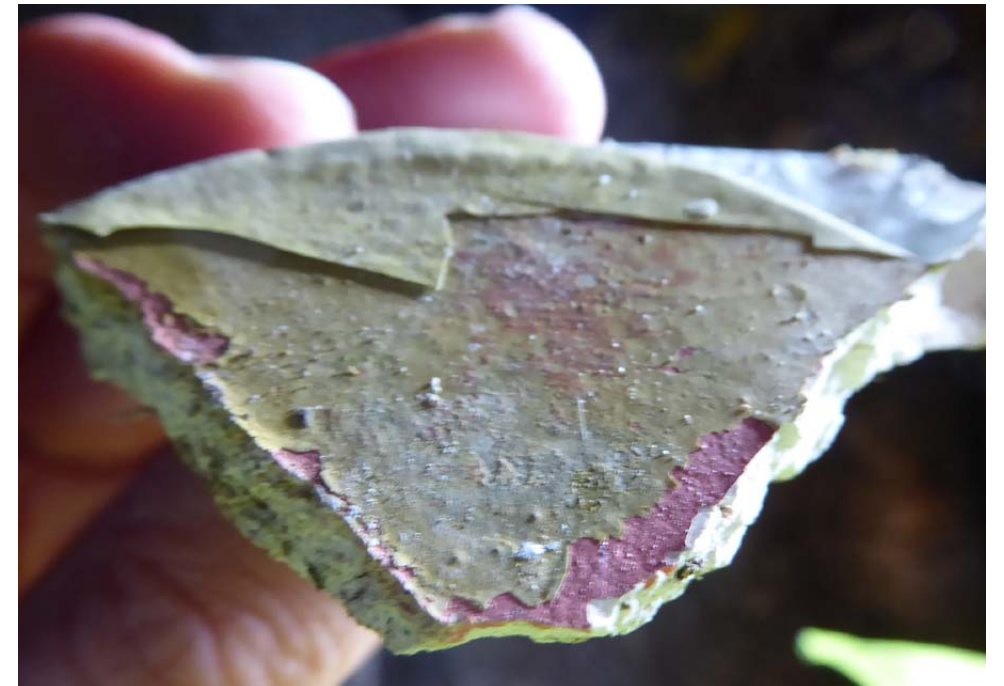
Section of chevron plaster with gold / yellow paint preceded by red
