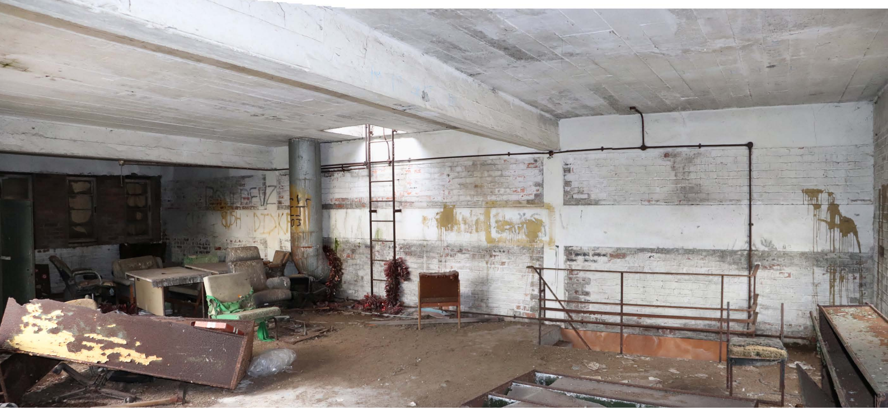
View of north wall showing concrete framed wall with brick infill and slim precast concrete units to soffit, all painted white
