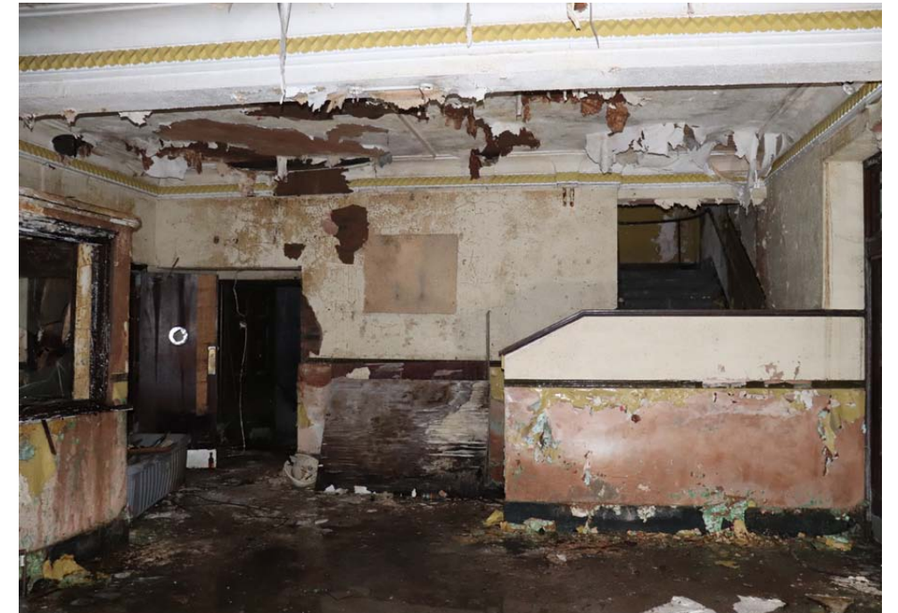
View of the Foyer looking towards the east staircase and toilets
