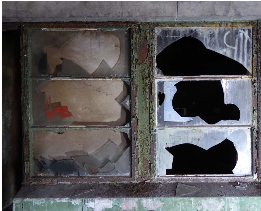
View of corrosion to steel frame sections at mullion
