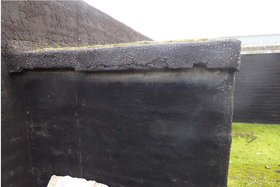
View of asphalt capping to box construction to ladder access
