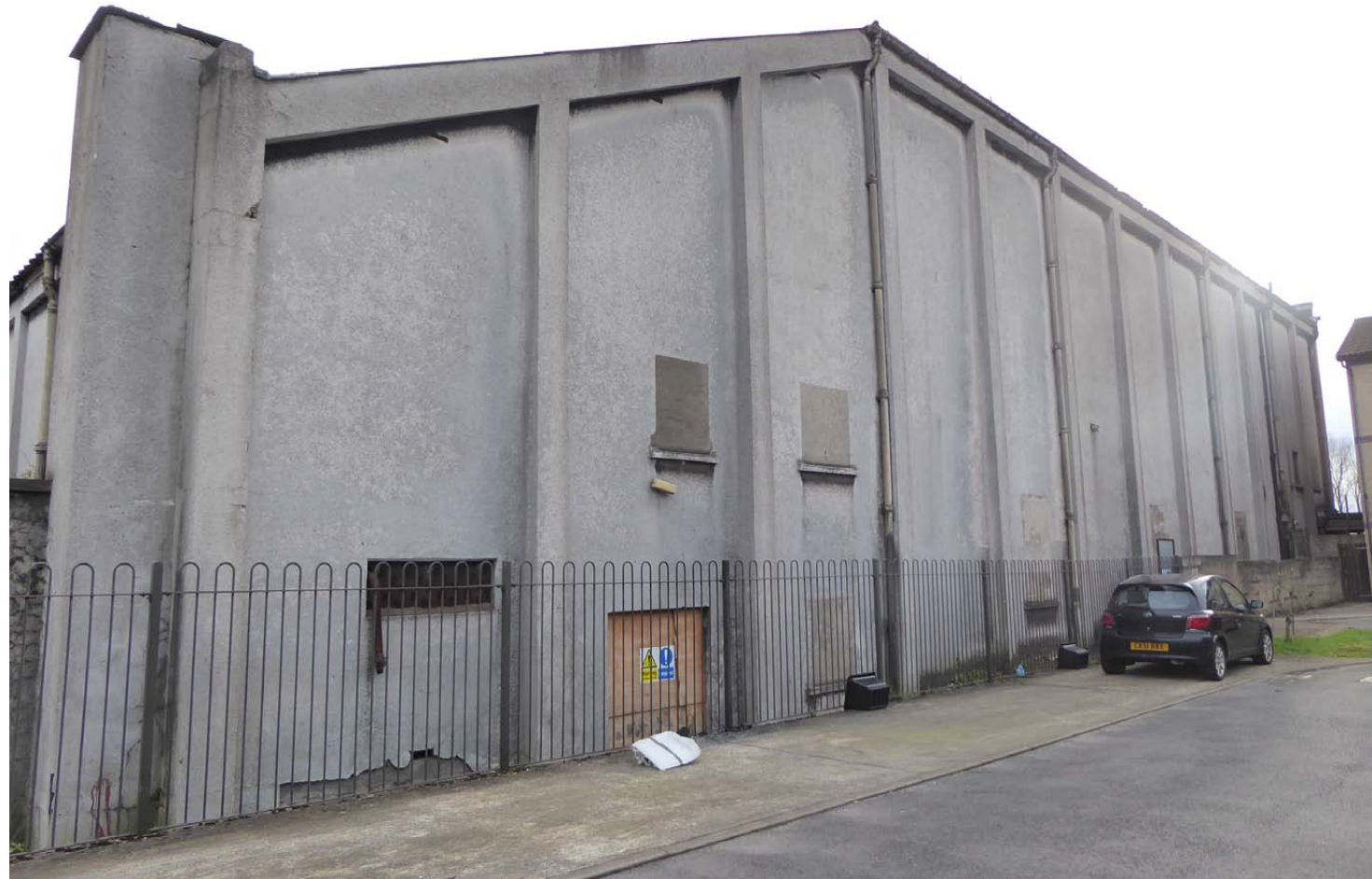
View of west elevation
