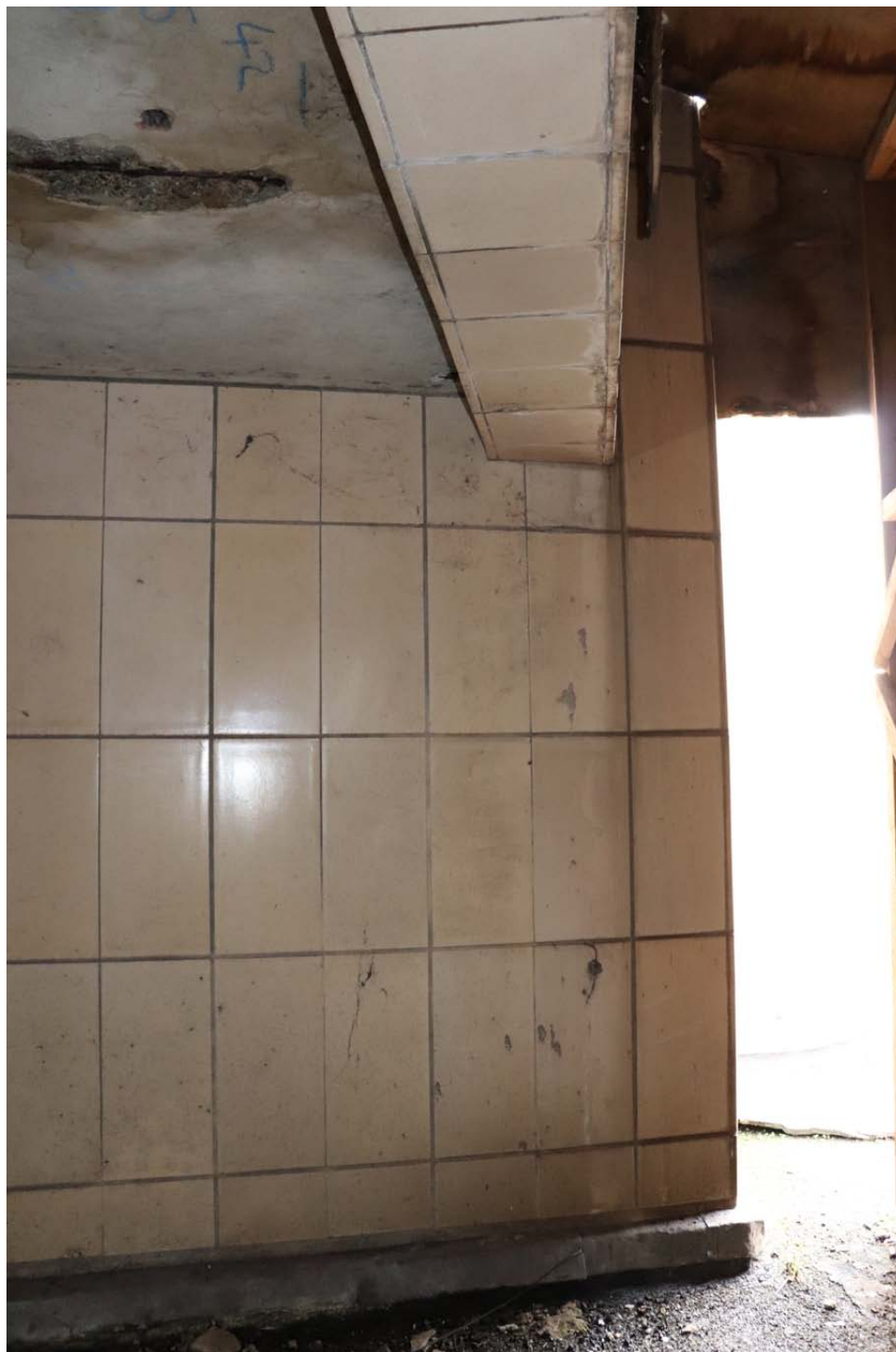
The faience-clad beam to the opening & the faience to the side
