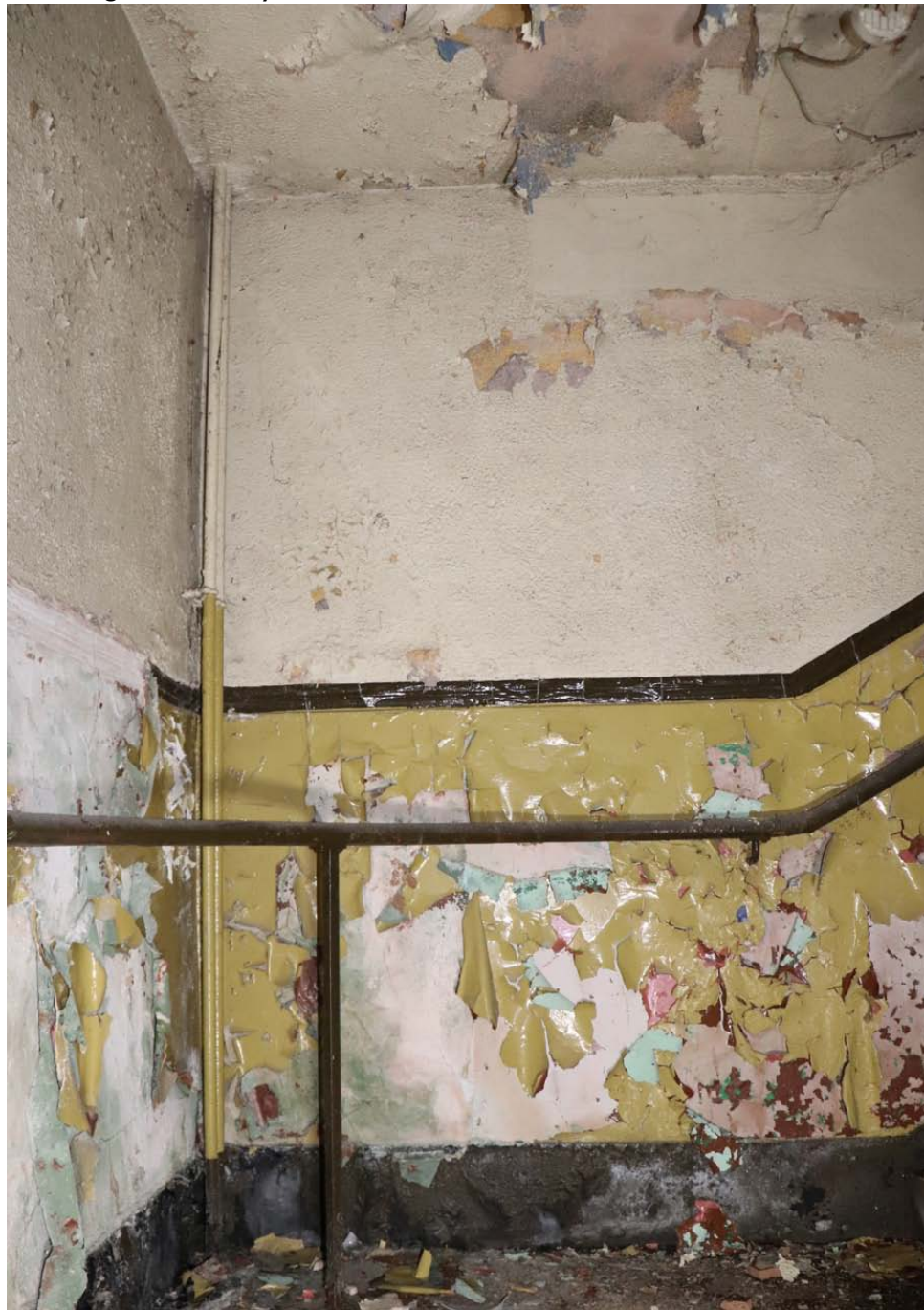
Quarter landing to staircase with curved simple round steel handrail
