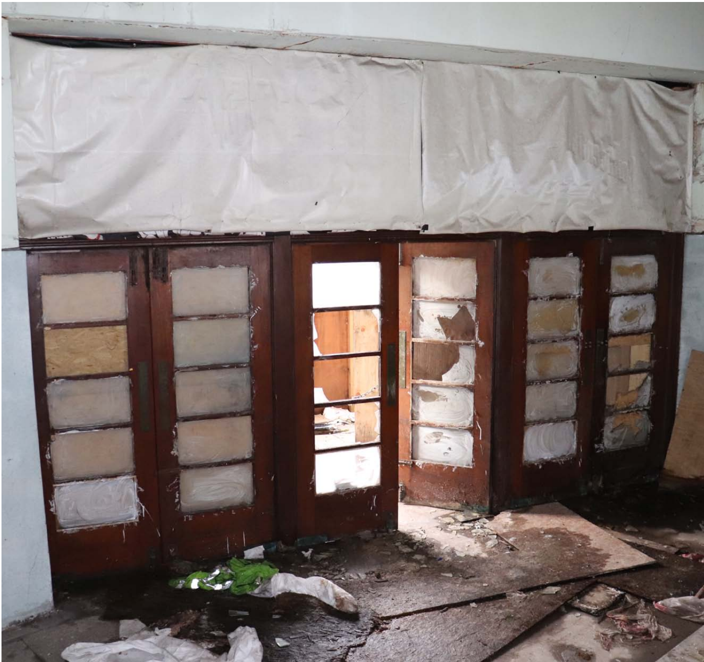
View of bank of 3no. sets of double doors in centre
