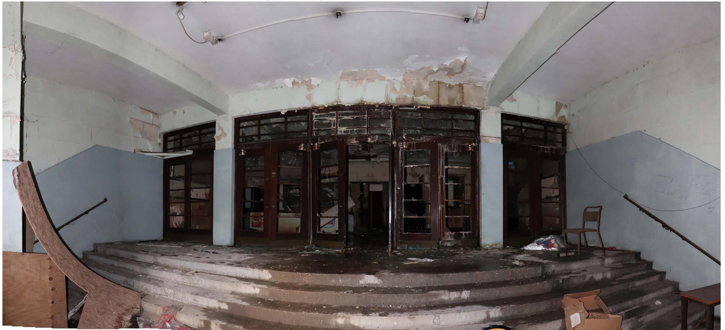
View of bank of timber-framed double doors between lower entrance lobby and upper entrance foyer, with terrazzo steps in foreground
