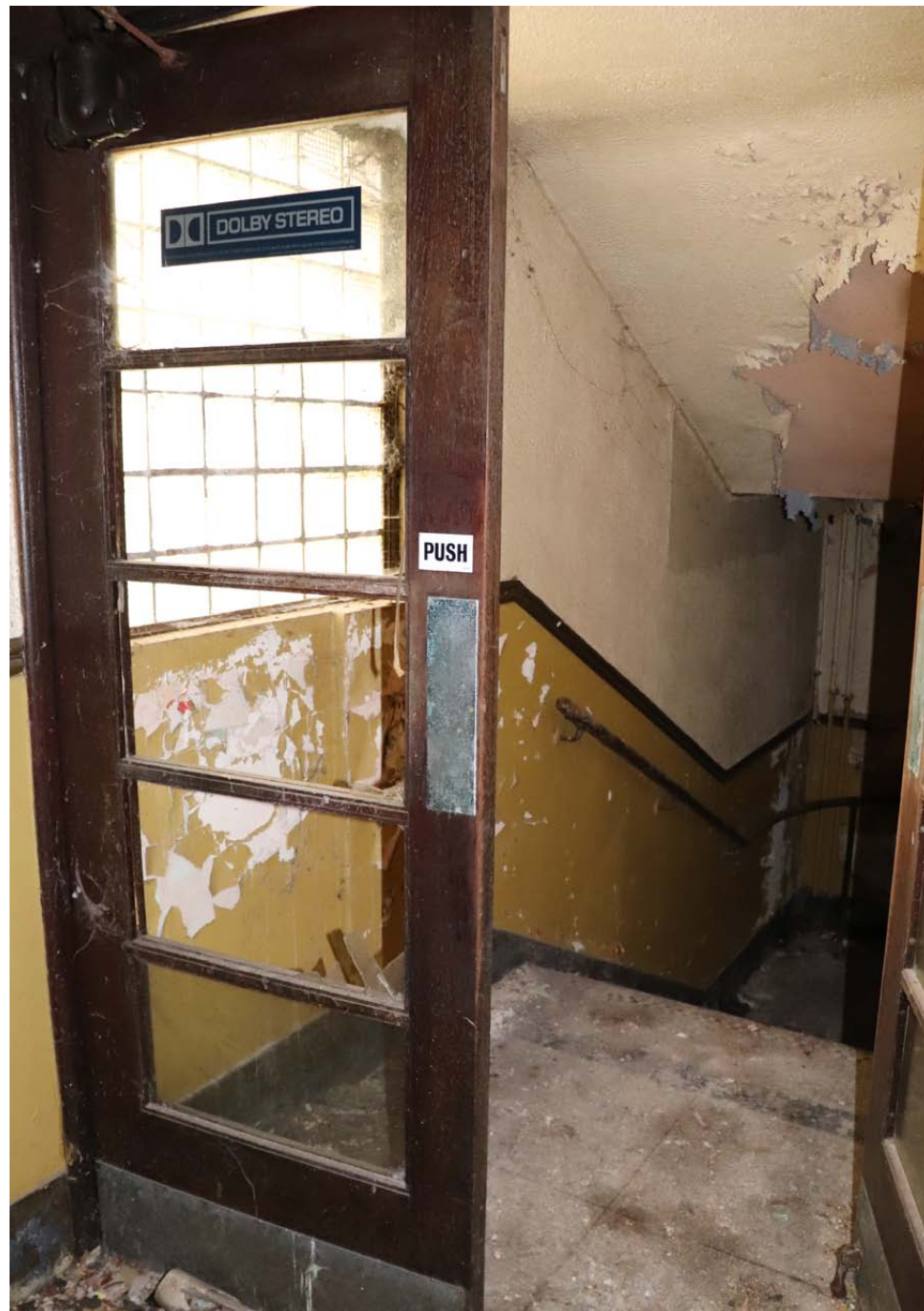
Looking down stairs to blocked up window where timber stairs pass
