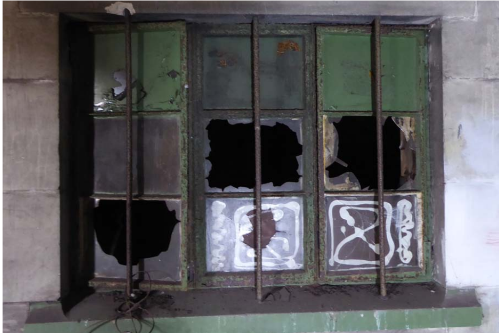
View the metal-framed window with steel bars in front in this case
