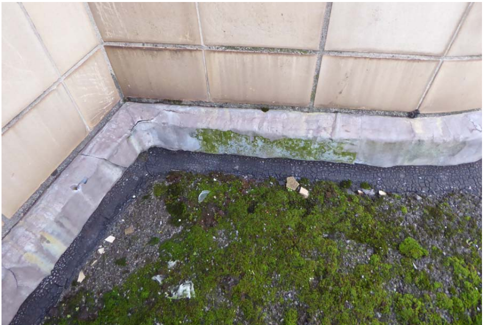
View of the lead flashing at junction between faience & asphalt roof
