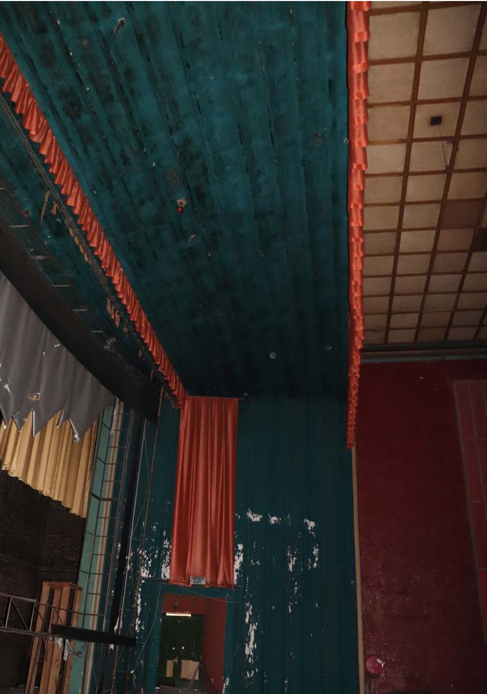
View of stage / auditorium connection on stage left
