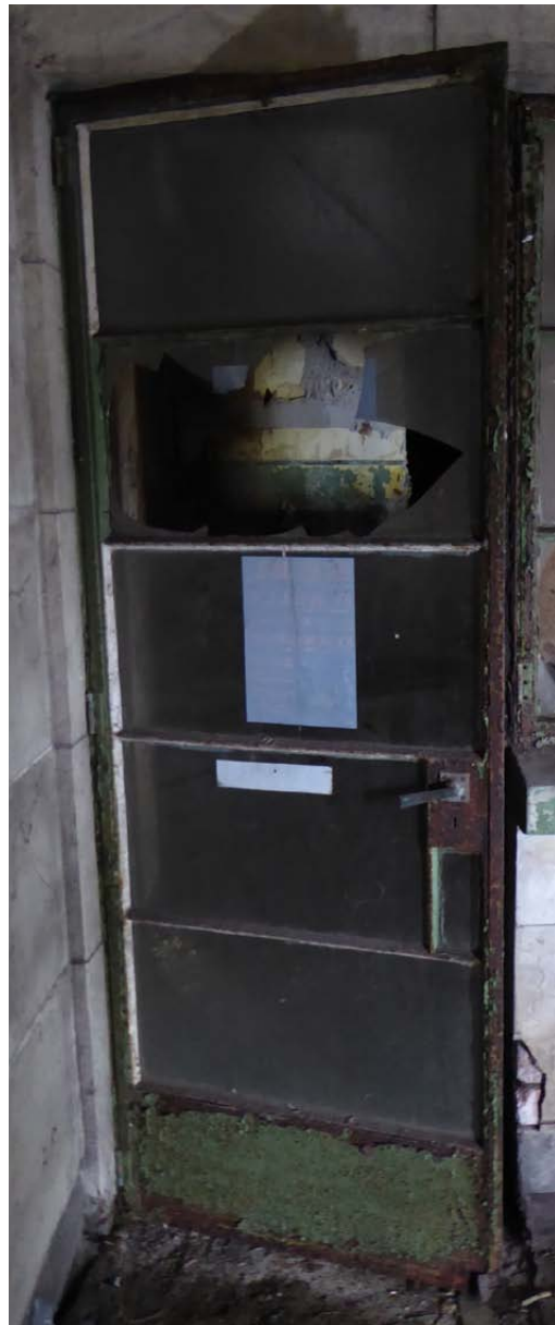
View of corrosion to steel frame sections at mullion
