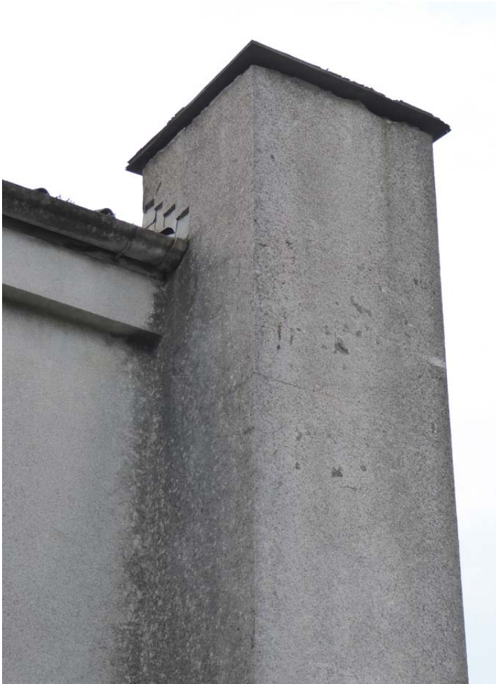
View of vent tower to the north west corner
