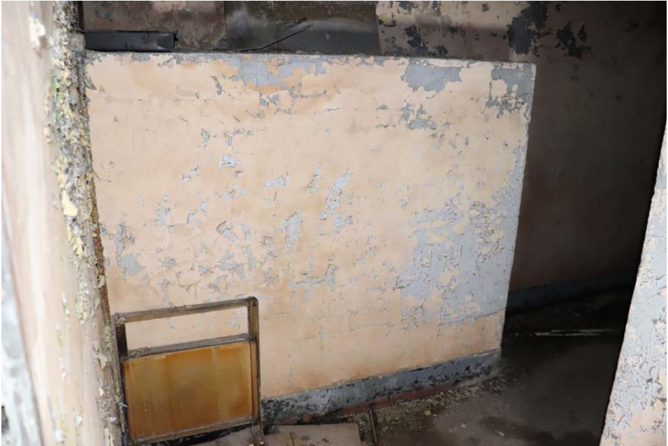
View of masonry construction providing headroom to the staircase
