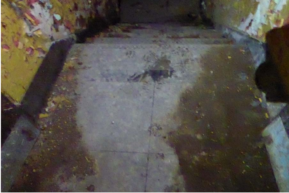
V Existing Steps to be Repaired
