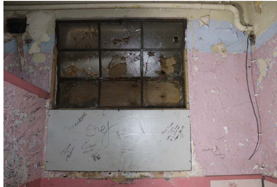
View of the Window to the west elevation
