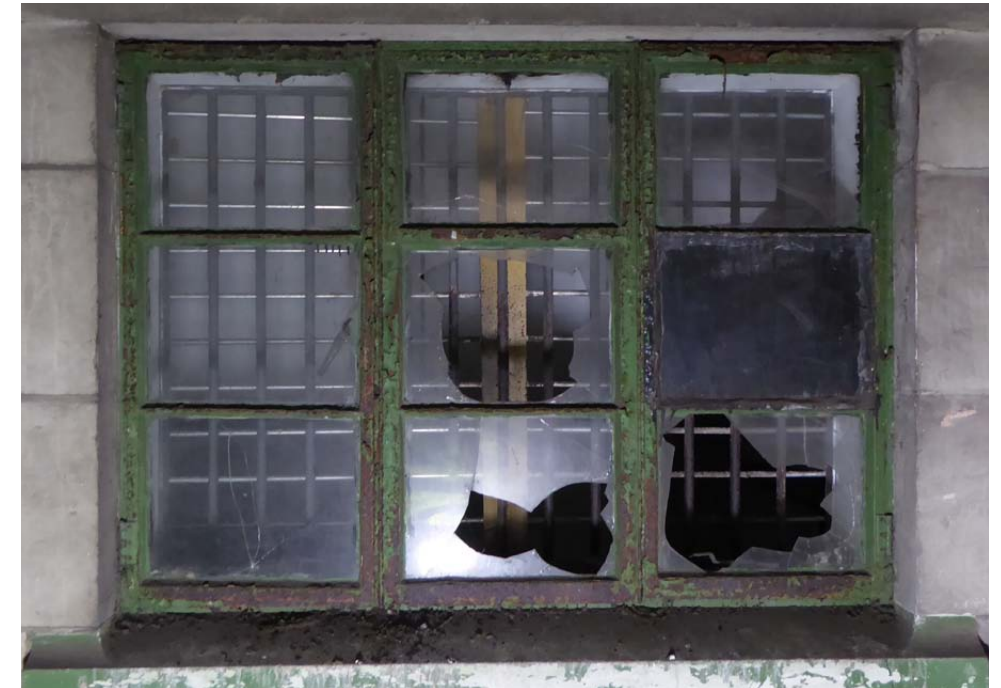
View the metal-framed window with steel bars behind
