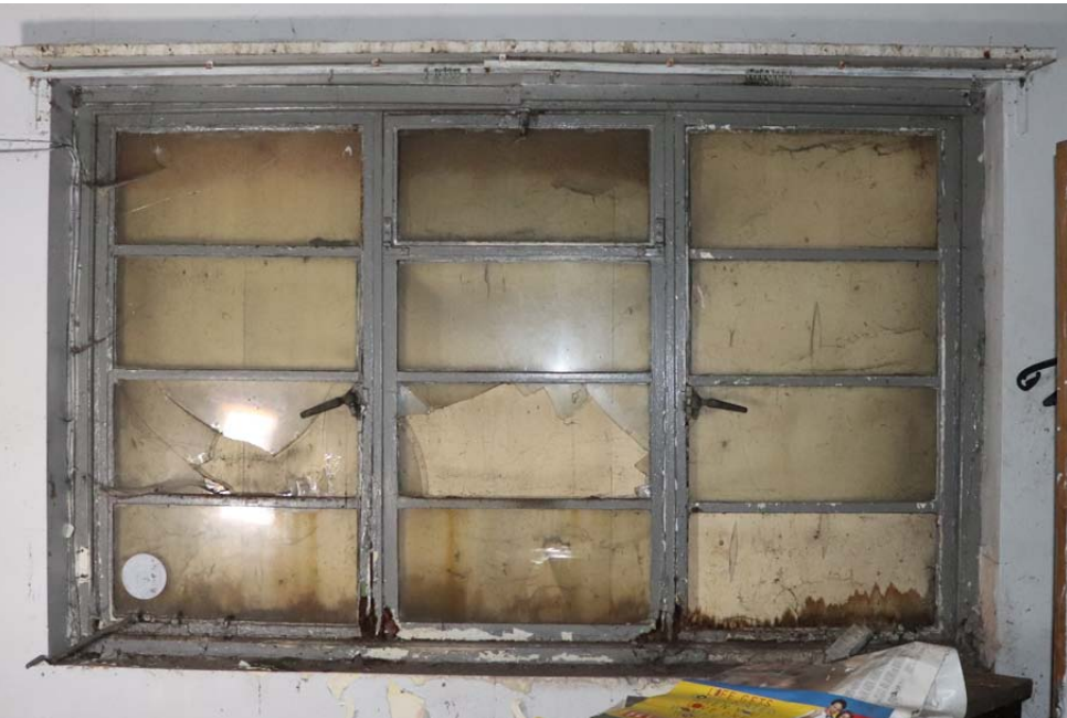
View of window to lobby to office
