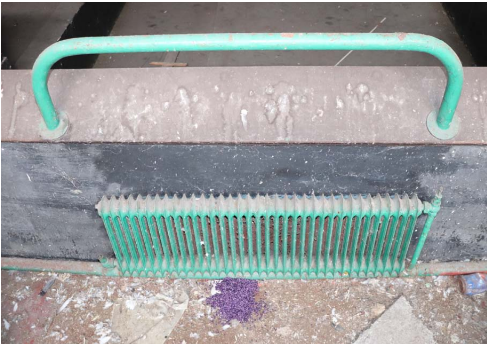
View of railing at bottom of aisle with radiator below it
