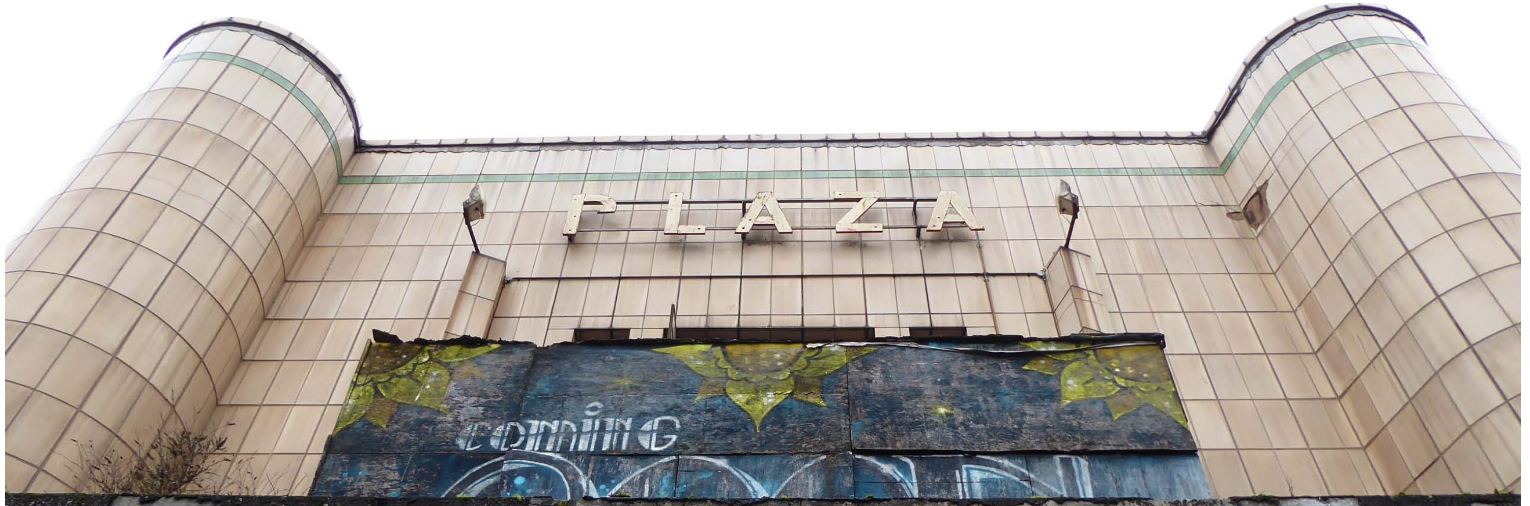
View of the top (faience) section of the front elevation
