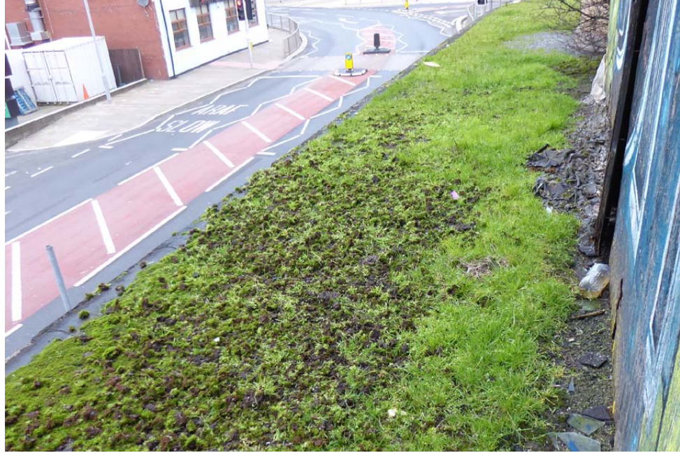
S Canopy Bitumen Roof to be Replaced
