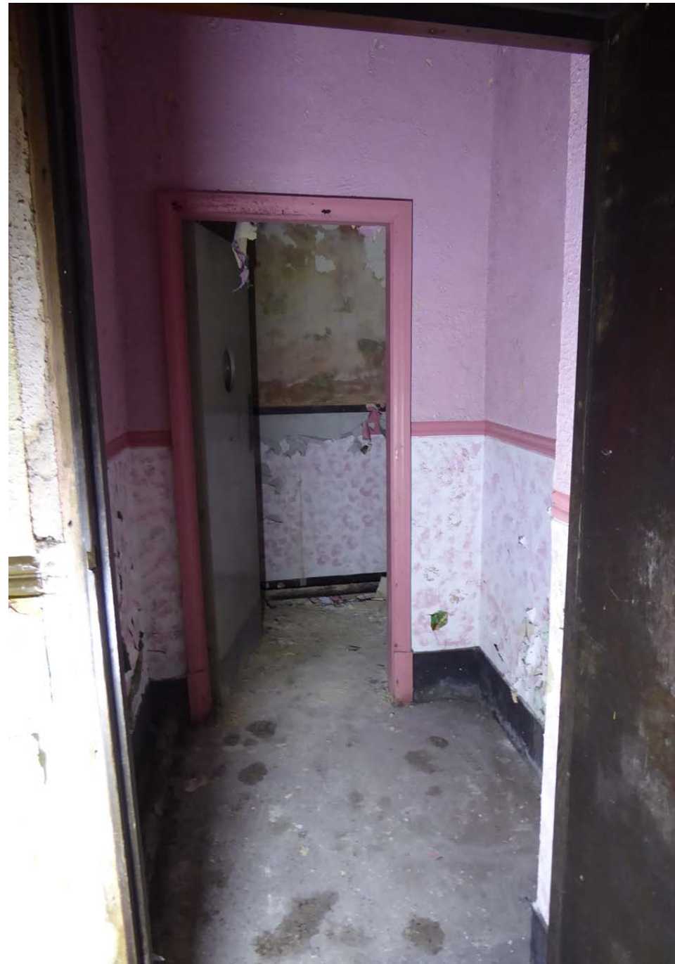
View from the Lobby looking in towards the toilets
