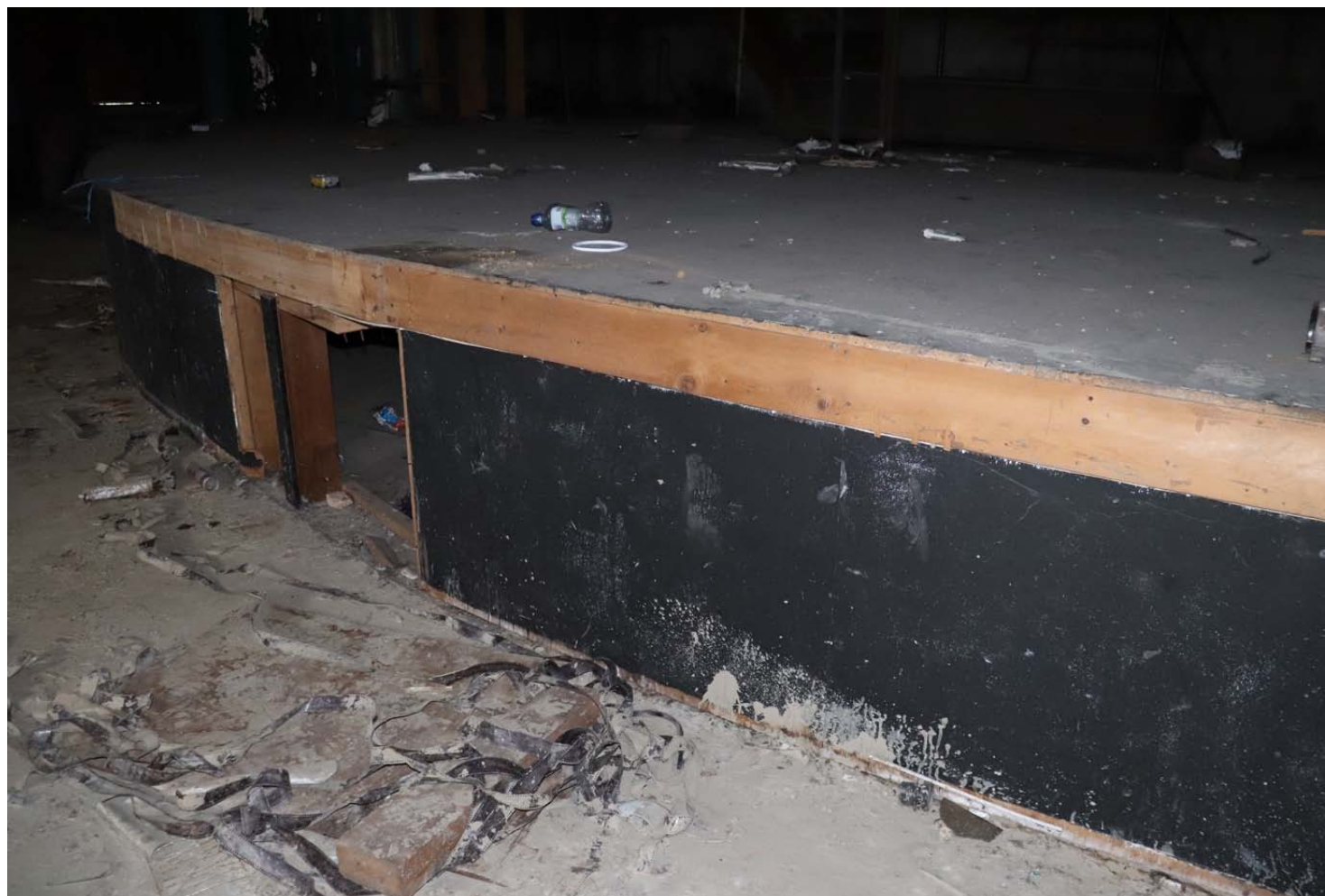
View of the timber framed construction of the curve fronted stage
