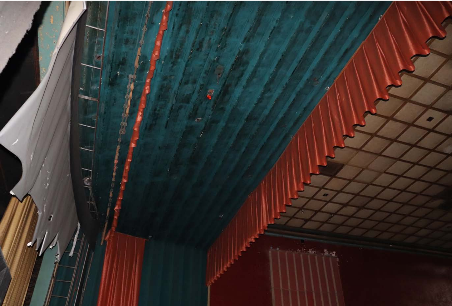
View of ceiling over Forestage running into ceiling over Auditorium with drapes in between
