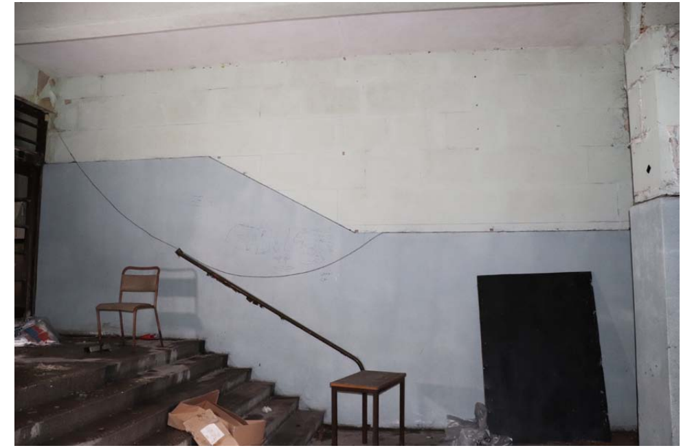
View of east side wall
