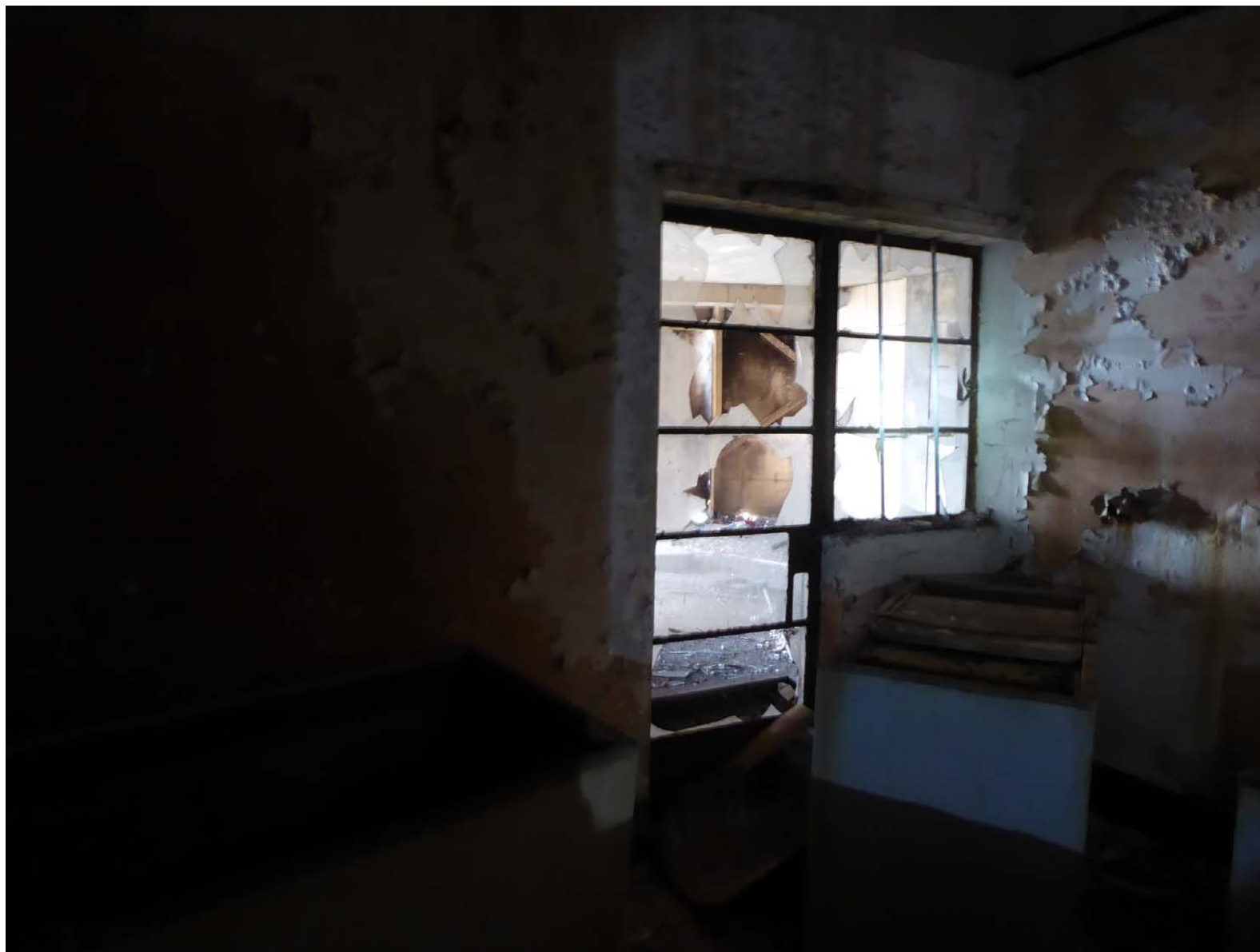
View of room looking towards one door and one window of the glazing looking out onto the recess roof area
