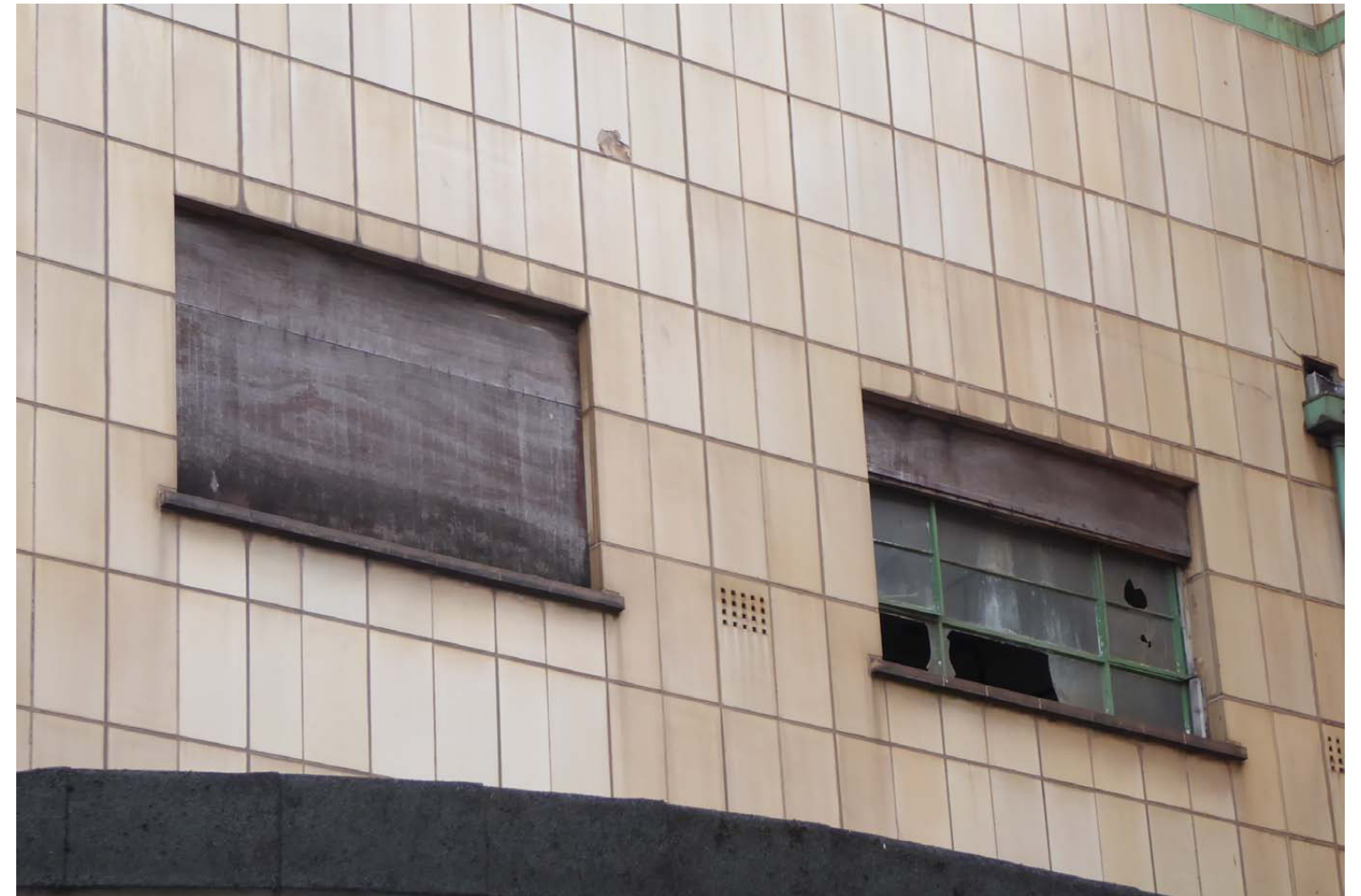
View of the two higher windows on the east facing section of the frontage
