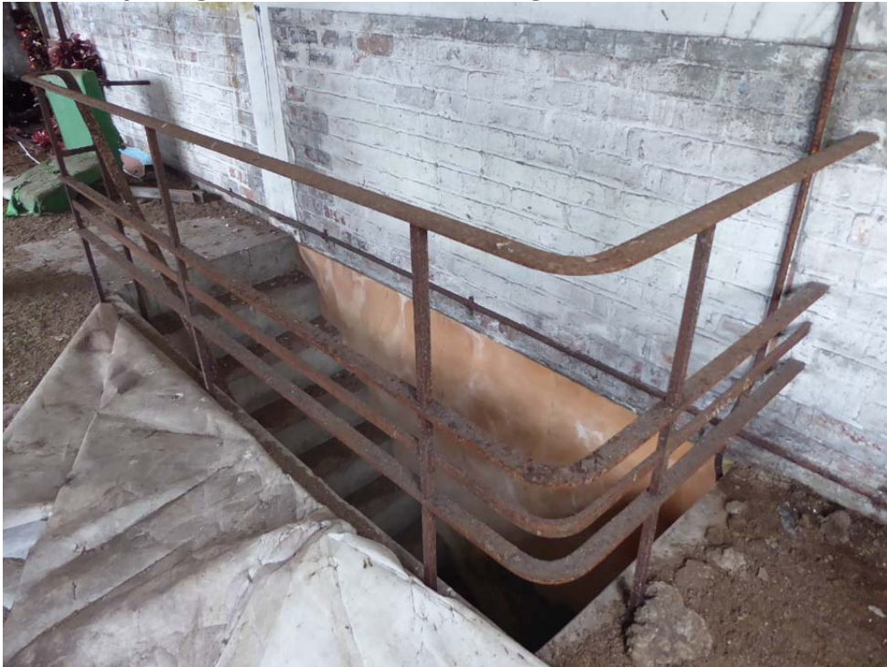
View of steel guardrail around stair void, which is Art Deco in style
