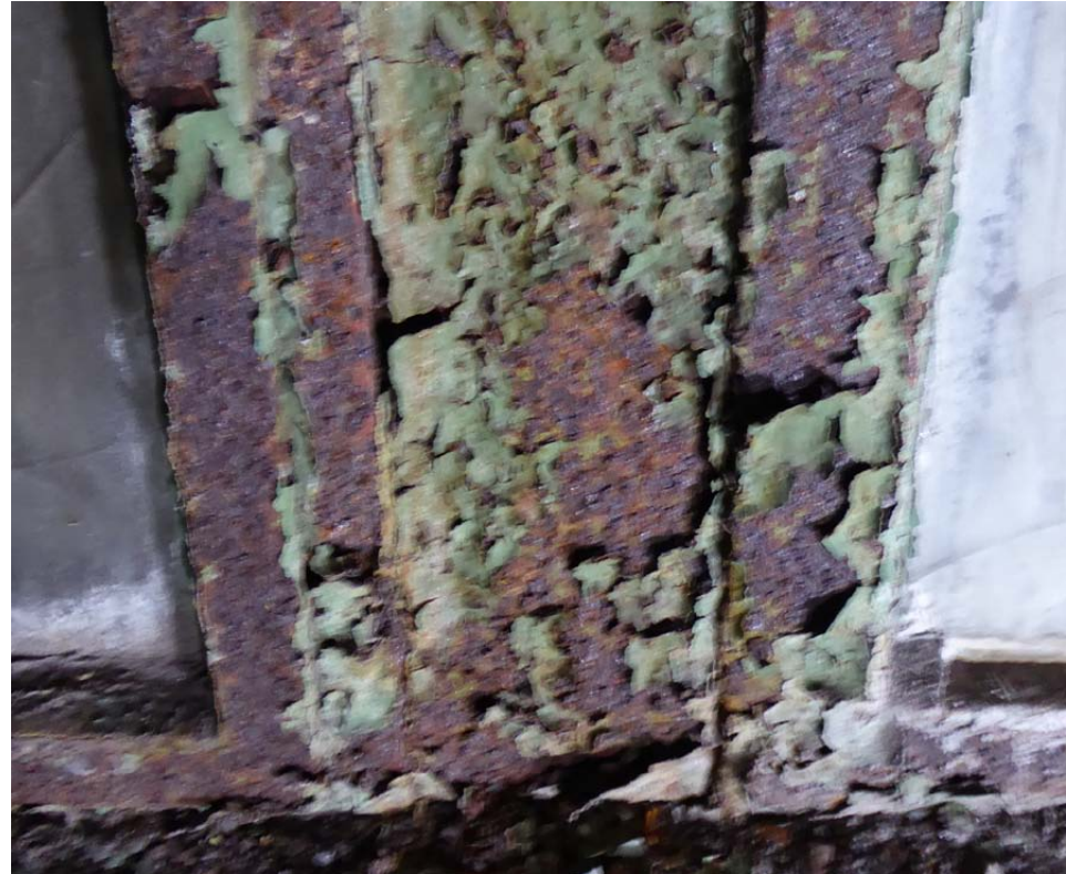
View of corrosion to steel frame sections at mullion
