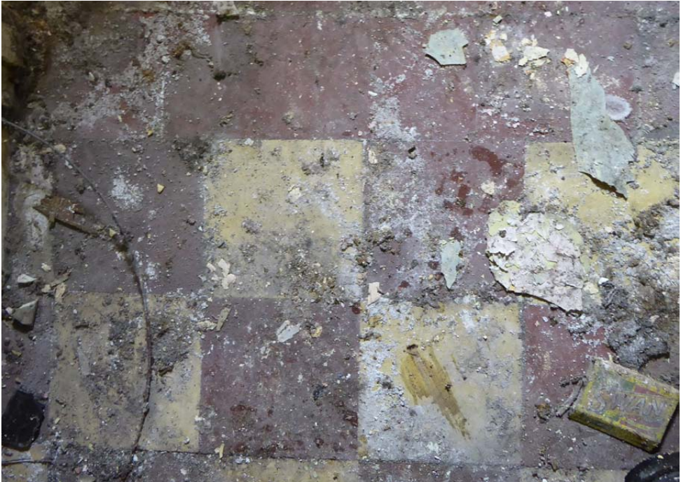
Quarry Tile Flooring in chequer-board pattern, of terracotta & cream
