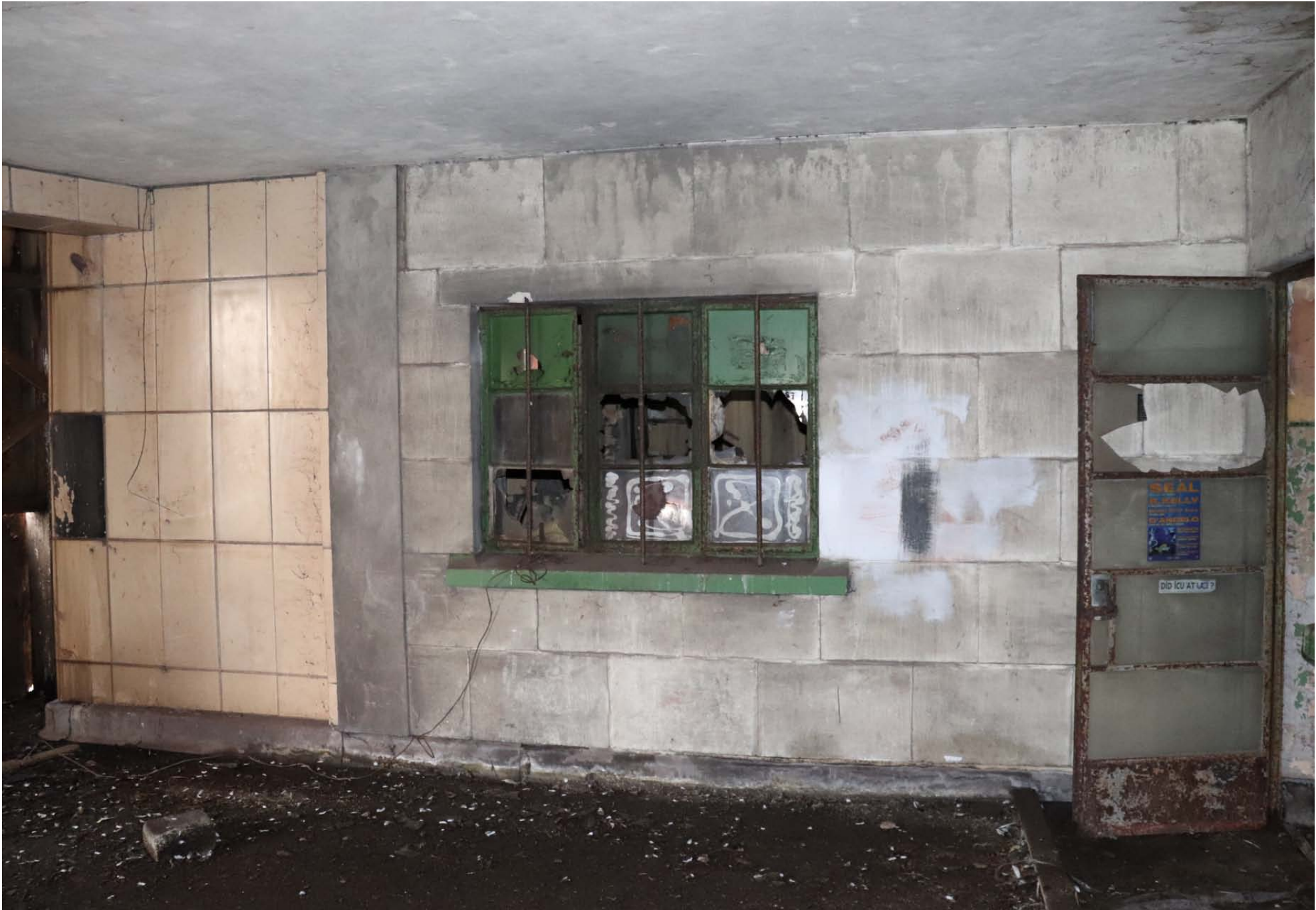
View of east elevation to open space with the masonry block facade, with its metal-framed window, leading to faience cladding
