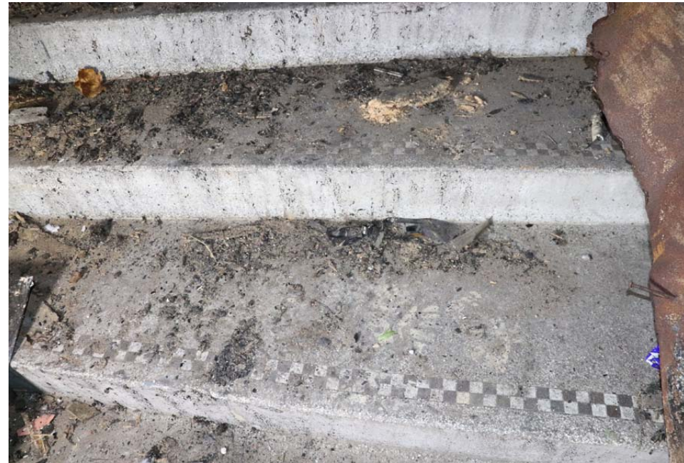
View of terrazzo steps with black & white chequerboard nosings
