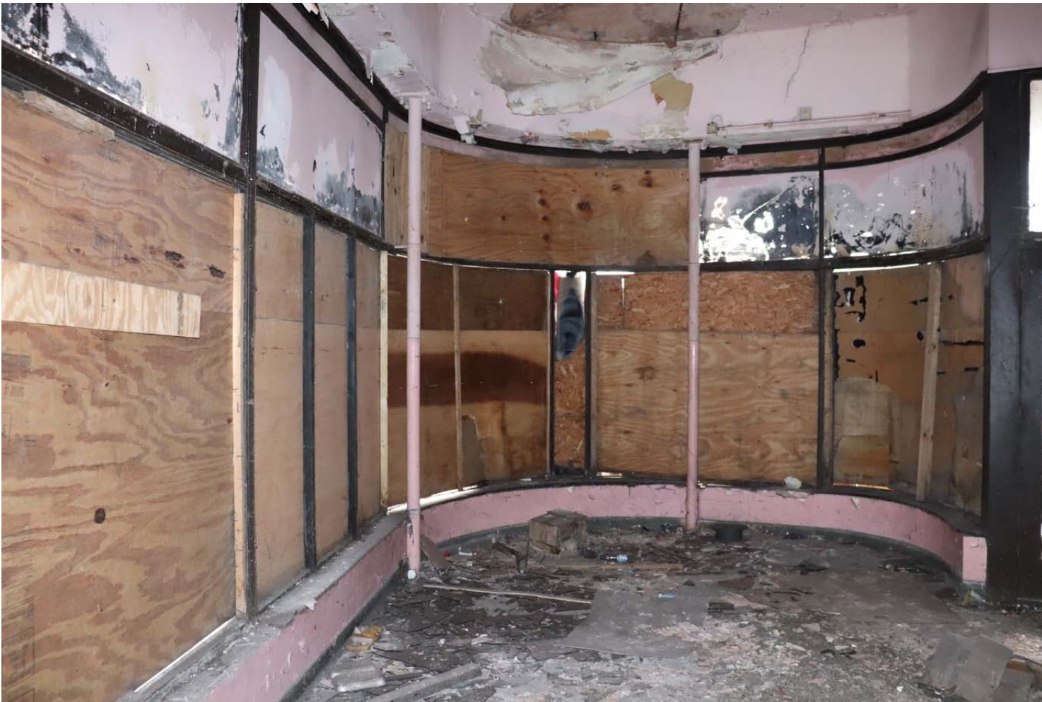
View of Glazing with Curved End and two Steel Columns
