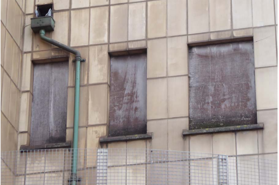
X Existing Rainwater Goods to be Retained & Restored
