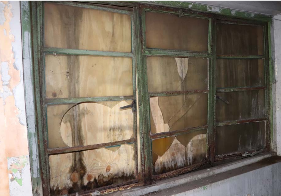
View of window within office
