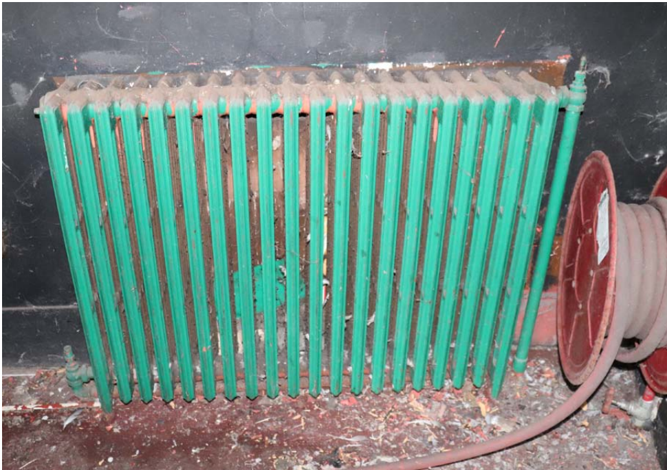
View of radiator at the rear of the space
