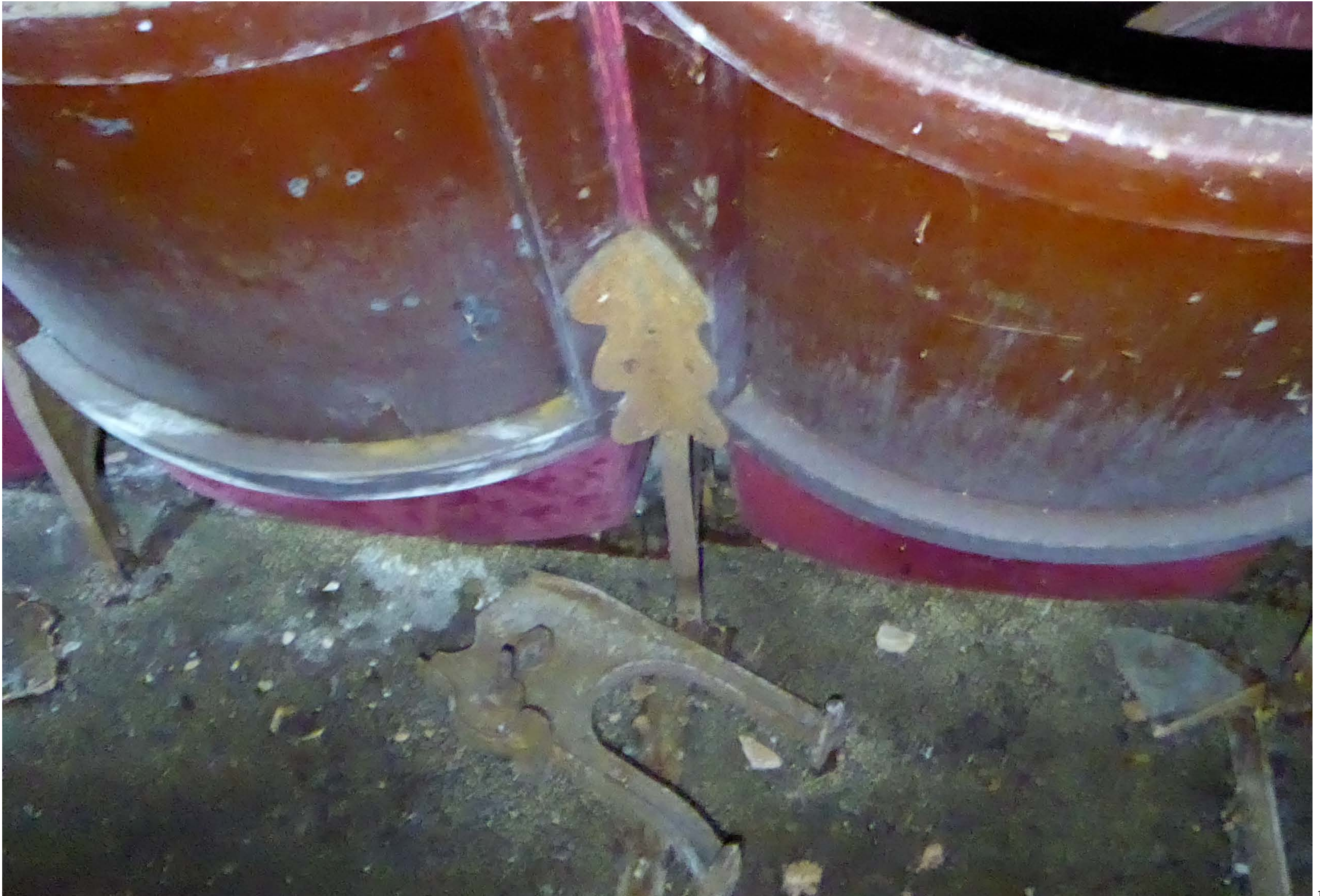
View of the rear of the seats with their timber curved backs and the metal support in between each seat. The metal stand lying on the floor is a broken version of the stand visible between the seats
