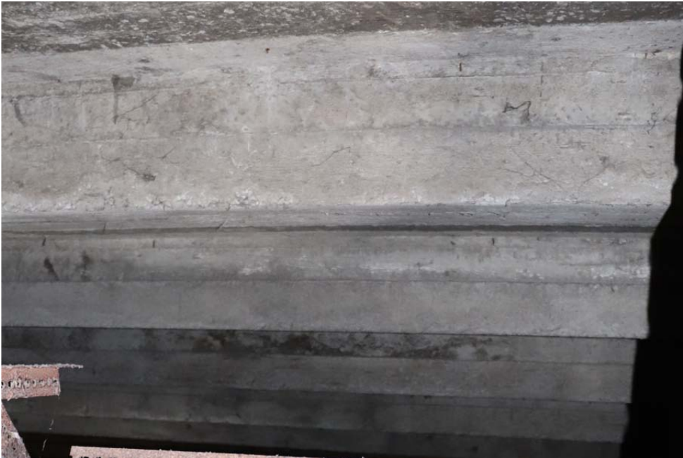
View to void underneath the concrete auditorium balcony seating
