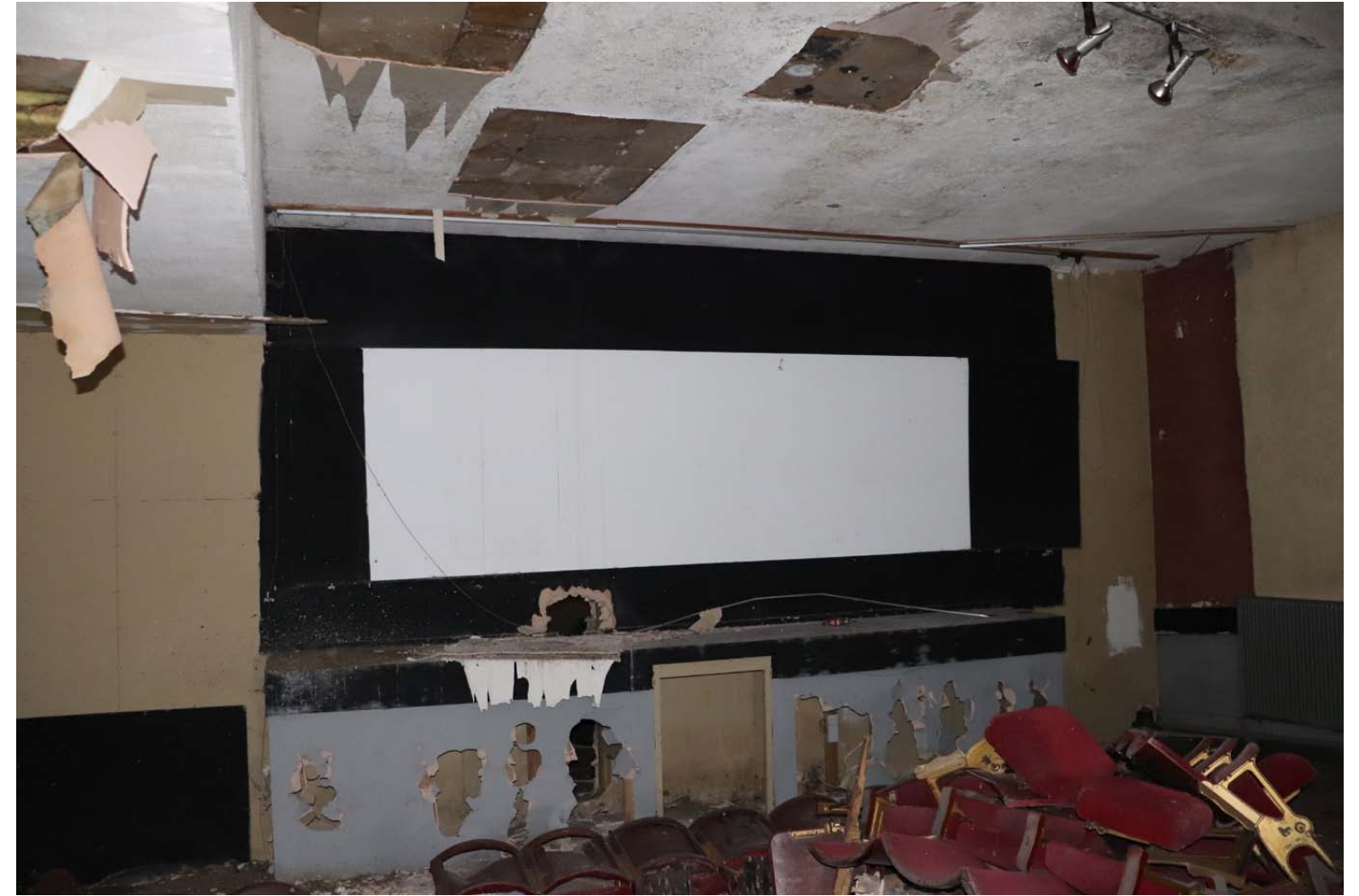
View of Cinema looking north
