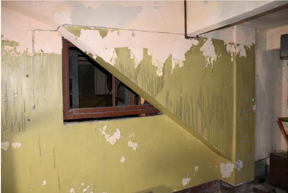
West wall to space showing raking concrete ‘beam’ to seating above
