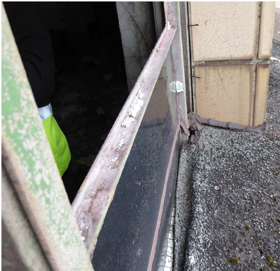
Detail of the south window, showing the mullion and transom bar
