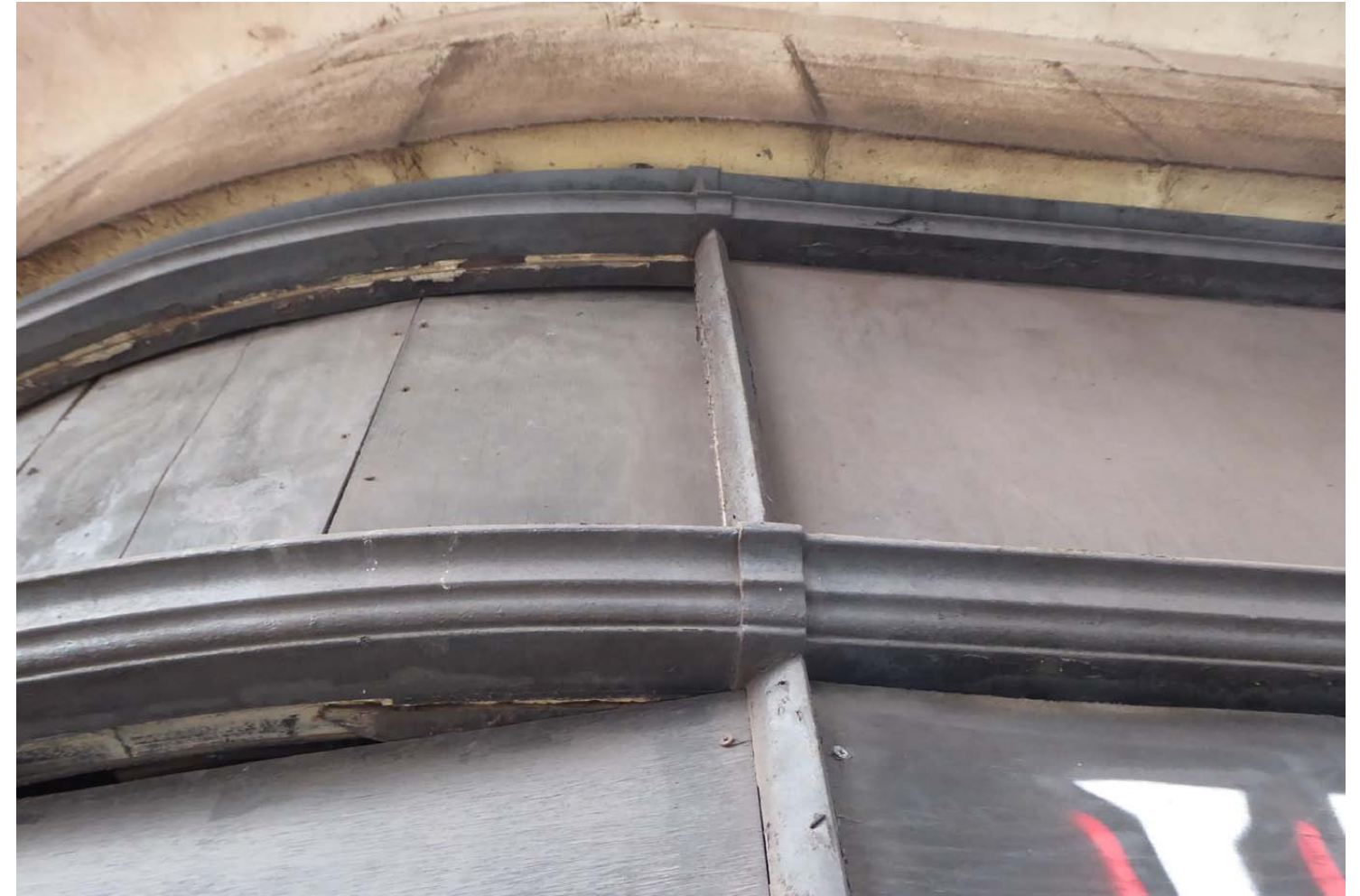
Views of top of curved frontage to timber-framed glazing to the larger (right-hand) Retail unit, showing profile to timber head section and lower transom section and vertical glazing bar with aerofoil profile
