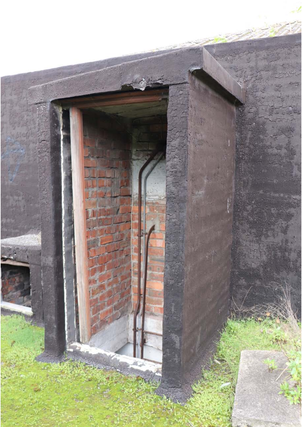
View of box construction to ladder access - from side
