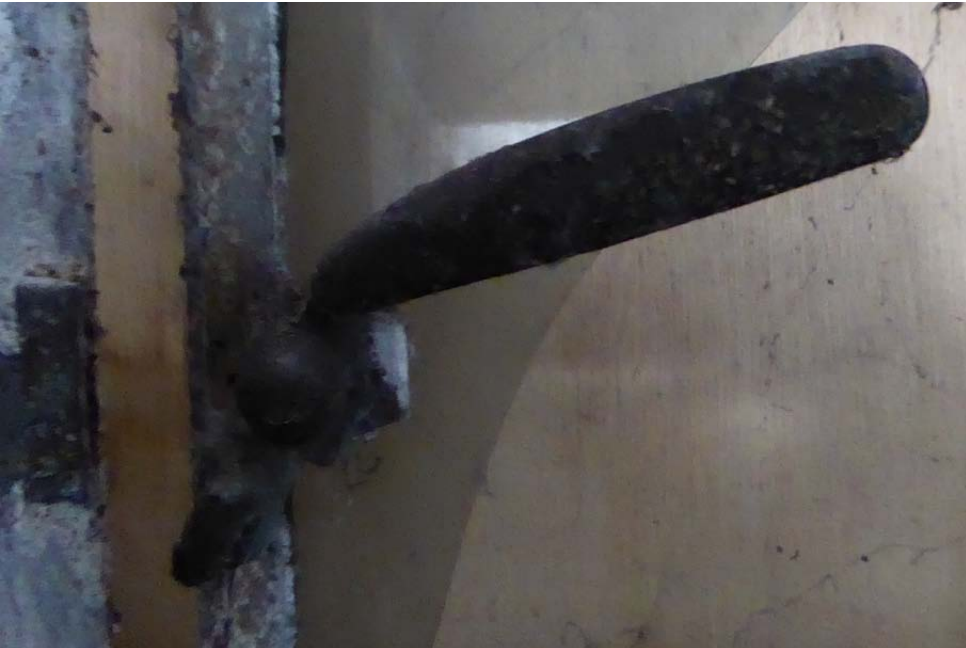
View of example of cockspur fastener to windows
