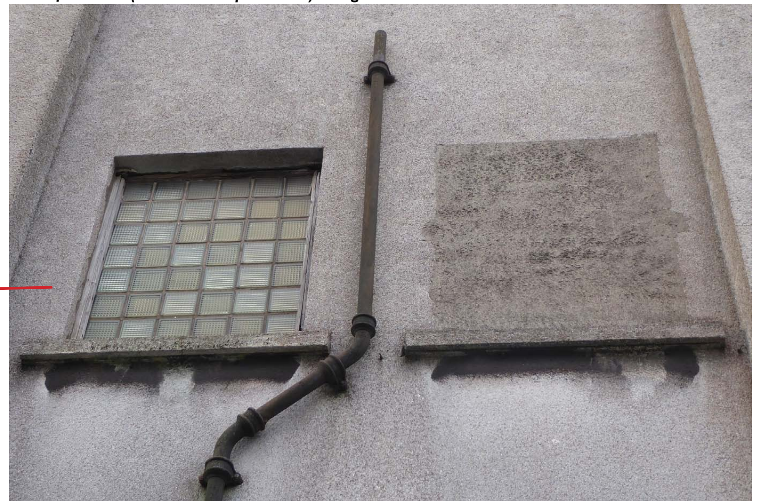
Detailed view of glass block window and one blocked up windows at high level
