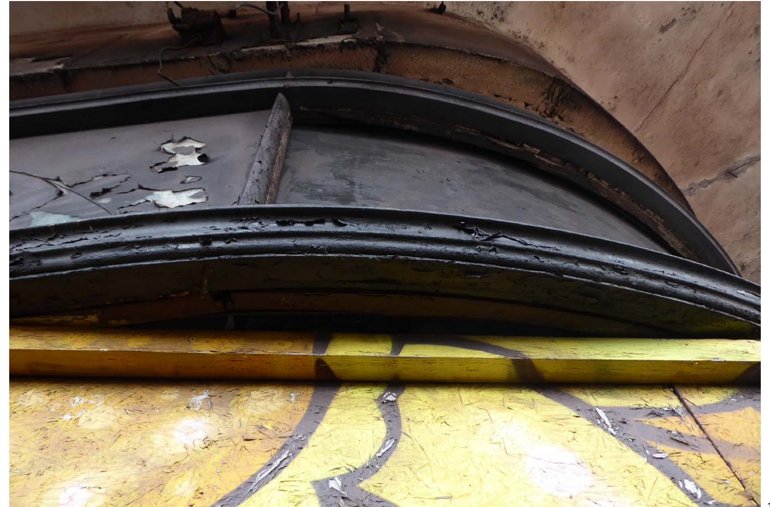
Views of top of curved frontage to timber-framed glazing to the smaller (left-hand) Retail unit, showing profile to timber head section and lower transom section and vertical glazing bar with aerofoil profile
