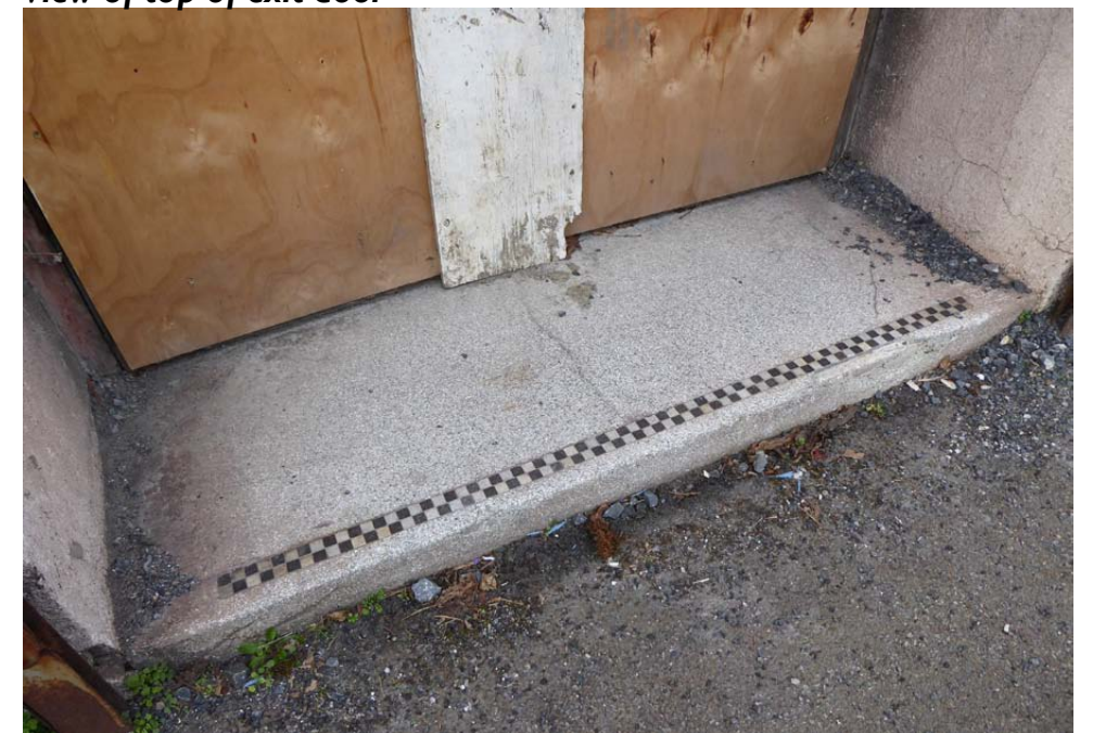
View of threshold of exit door (note terrazzo & chequerboard nosing)
