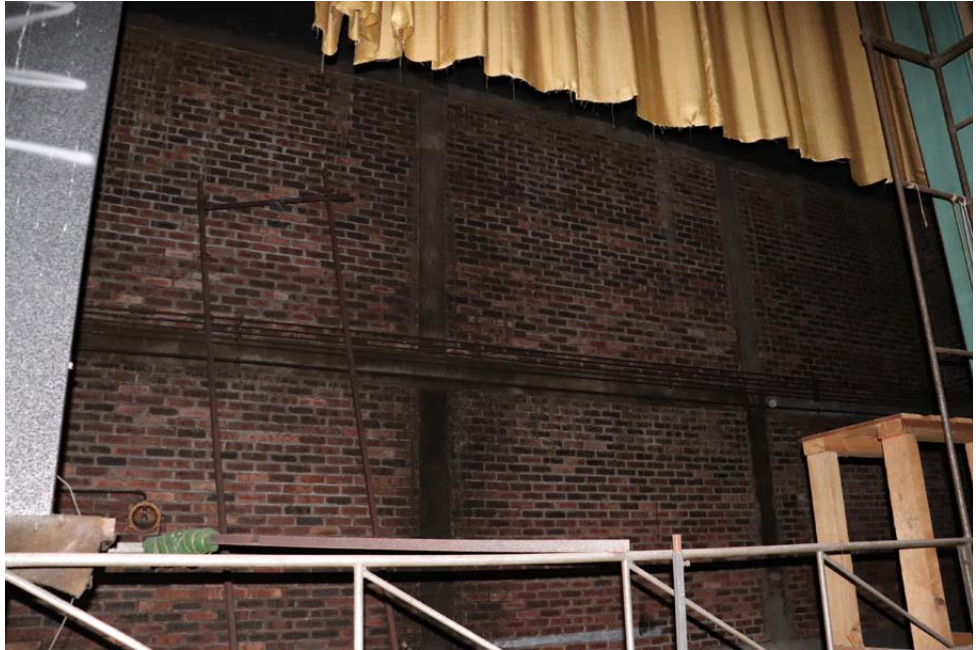
View of brick rear wall to stage within a concrete frame
