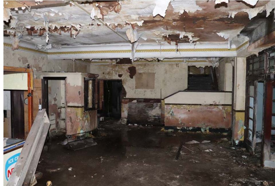
View of the Foyer looking towards the east
