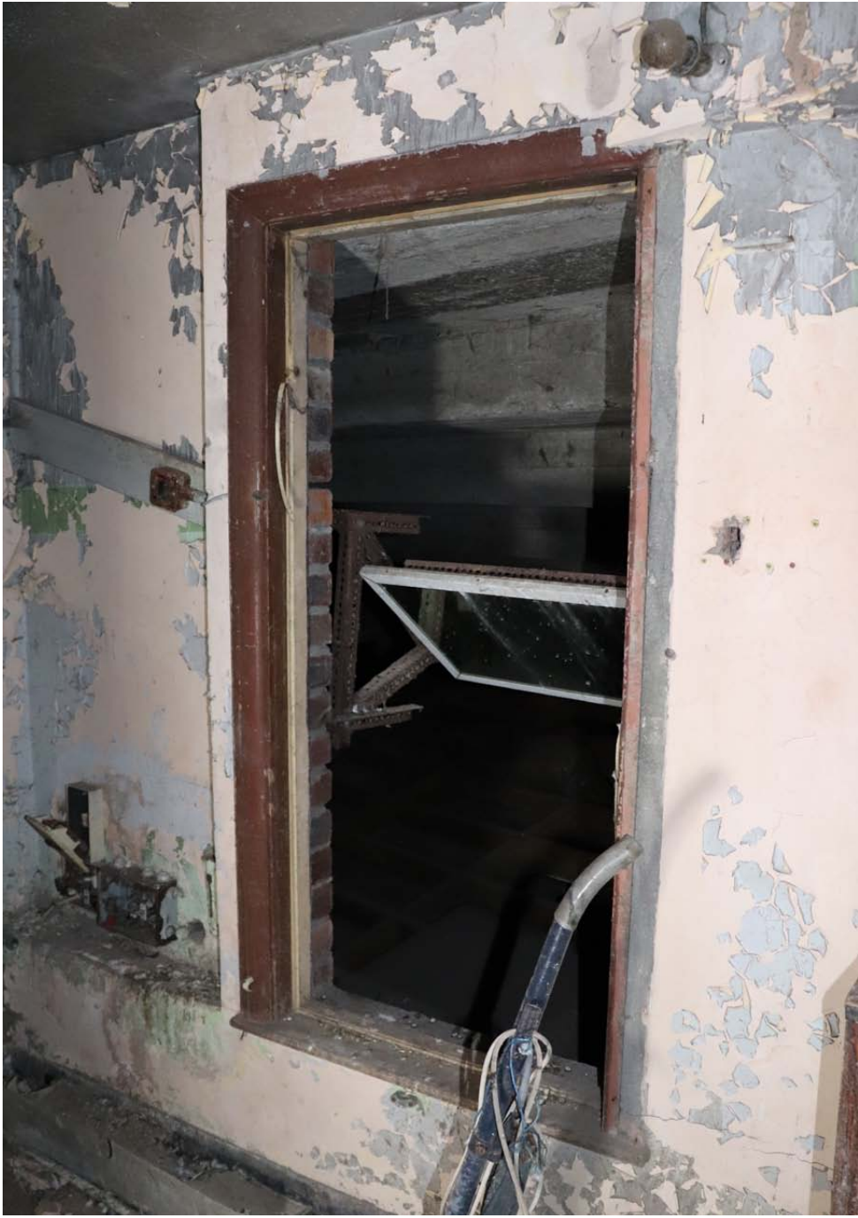
View of opening to underside of auditorium balcony seating
