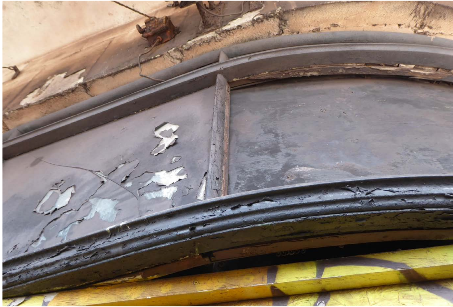
Views of top of curved frontage to timber-framed glazing to the smaller (left-hand) Retail unit, showing profile to timber head section and lower transom section and vertical glazing bar with aerofoil profile
