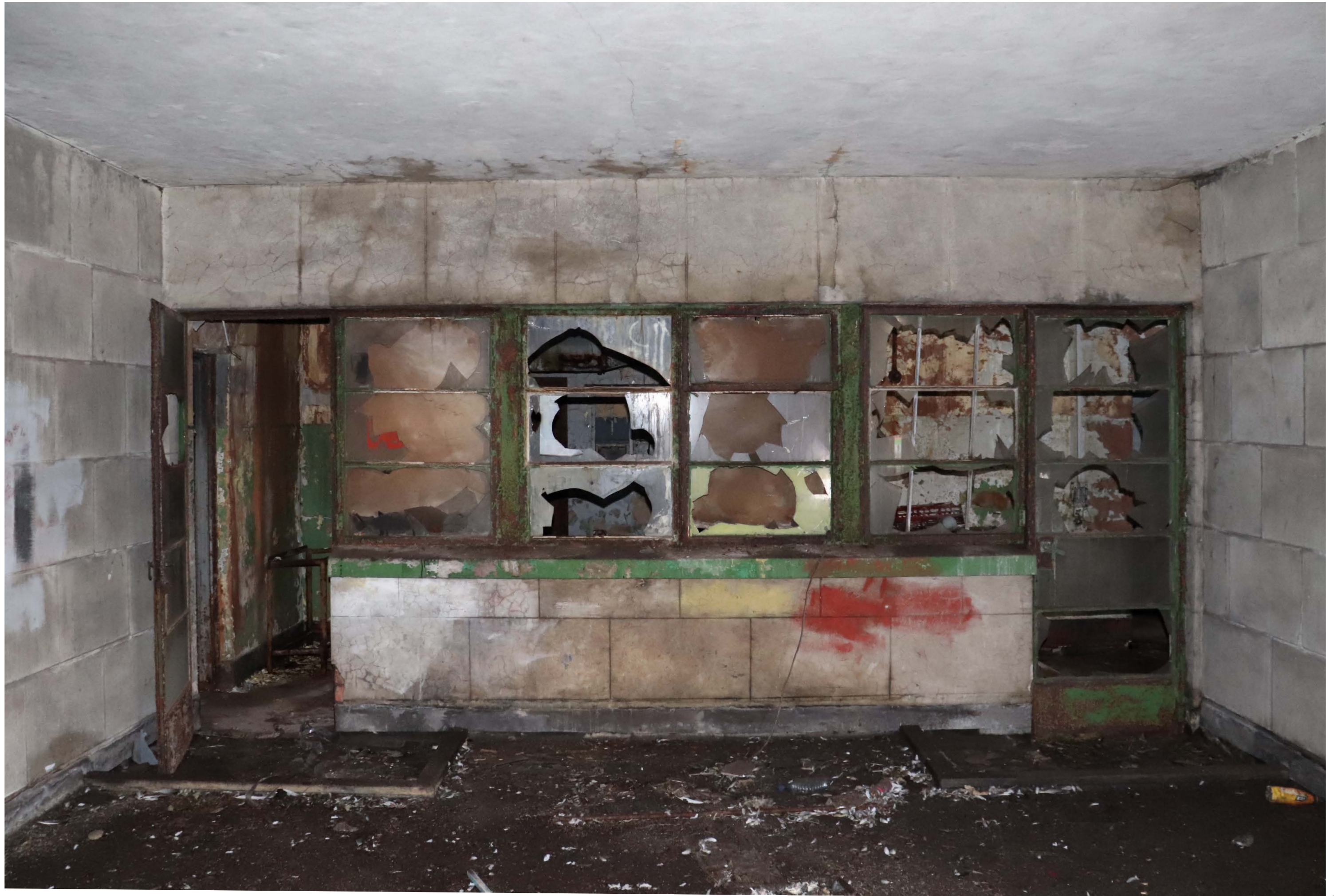
F13 - Central Roofed Recess - View of north elevation to space with run of flat steel-section slender framed windows with doors at either end, manufactured by Crittall or similar, synonymous with the Art Deco style
