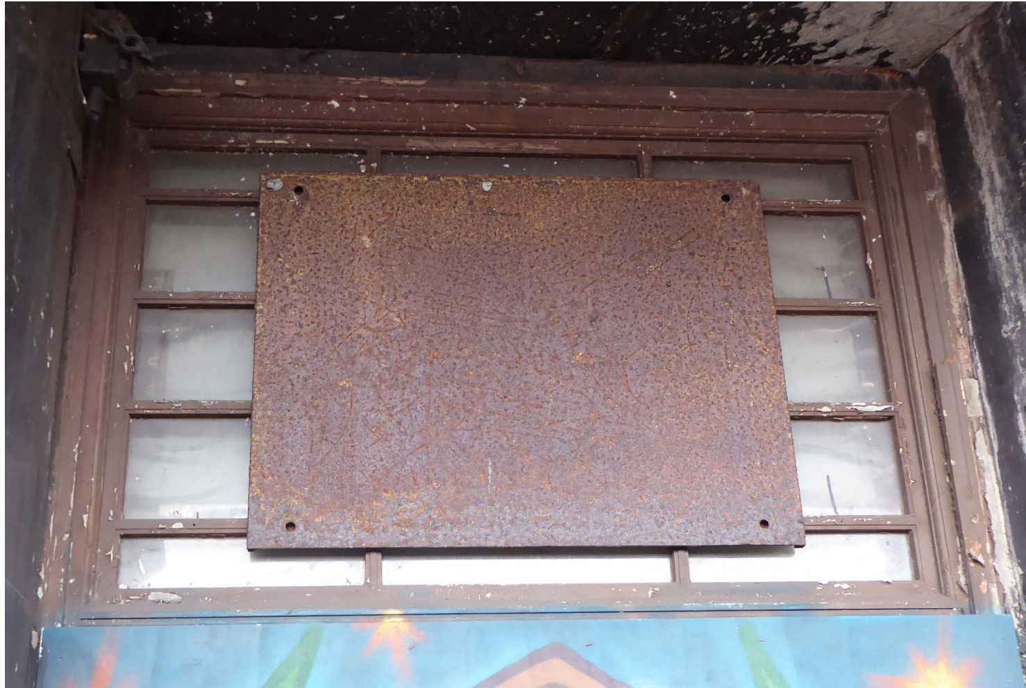
View of glazed overhead panel above side glazed panel, with metal plate affixed
