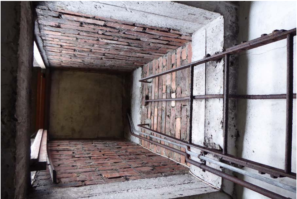
View of box construction to ladder access - from below
