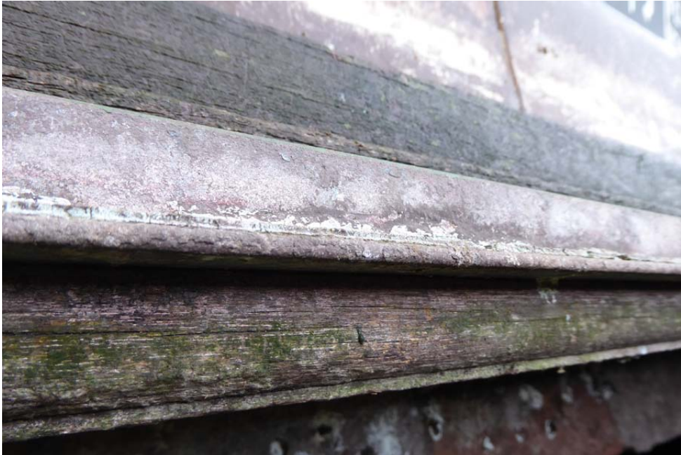
View of example of stay to windows
