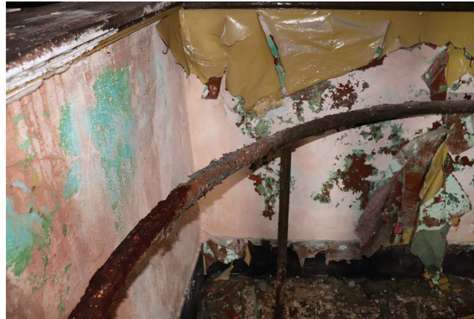
Simple round steel handrail curving inside the square corner
