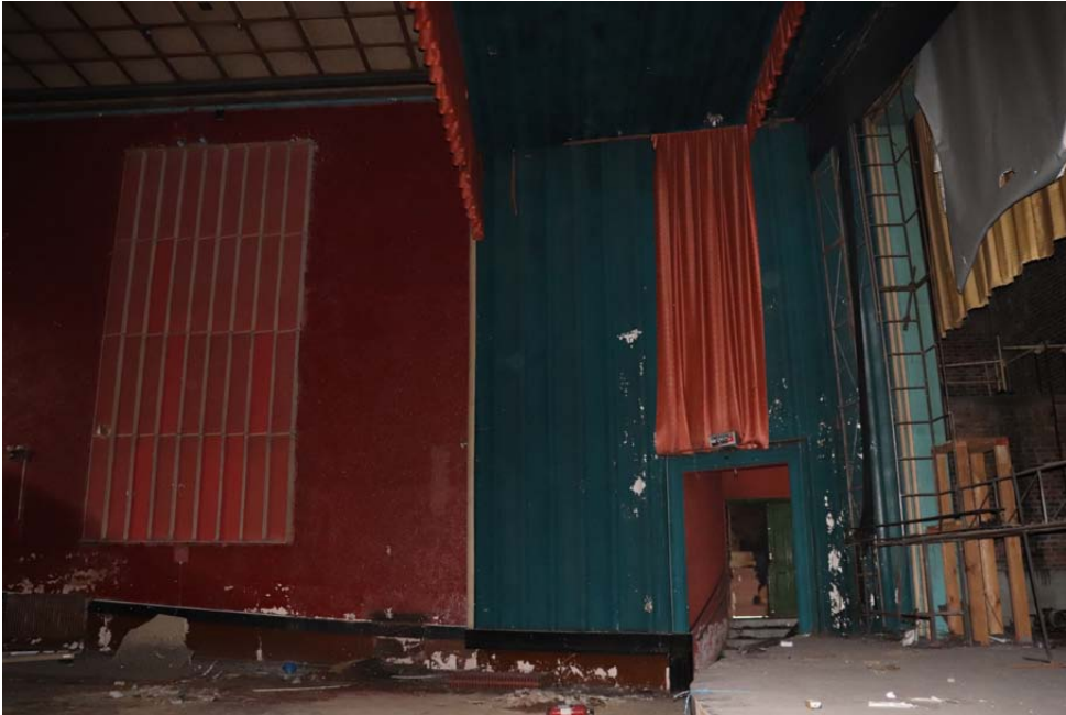
View looking across length of stage to stage right (west) end
