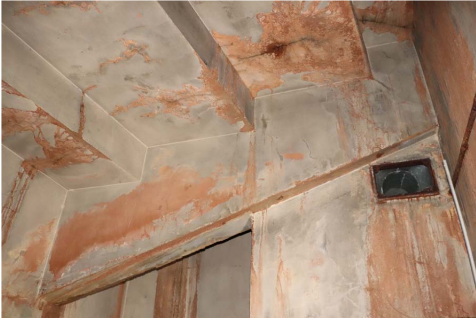
View of soffit showing raking concrete 'beam' and flat seating above
