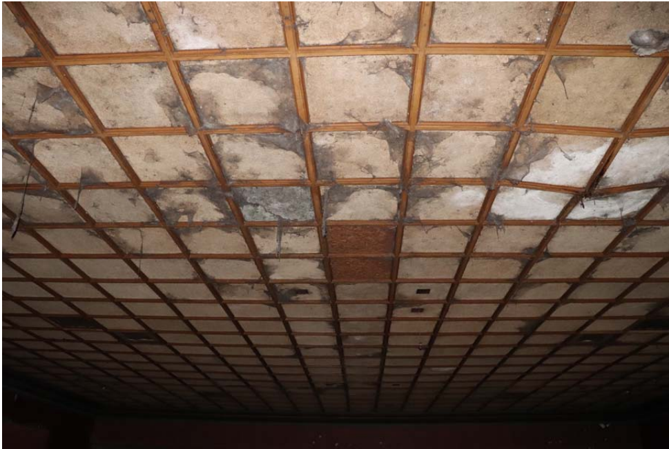
View of the ceiling looking northwards
