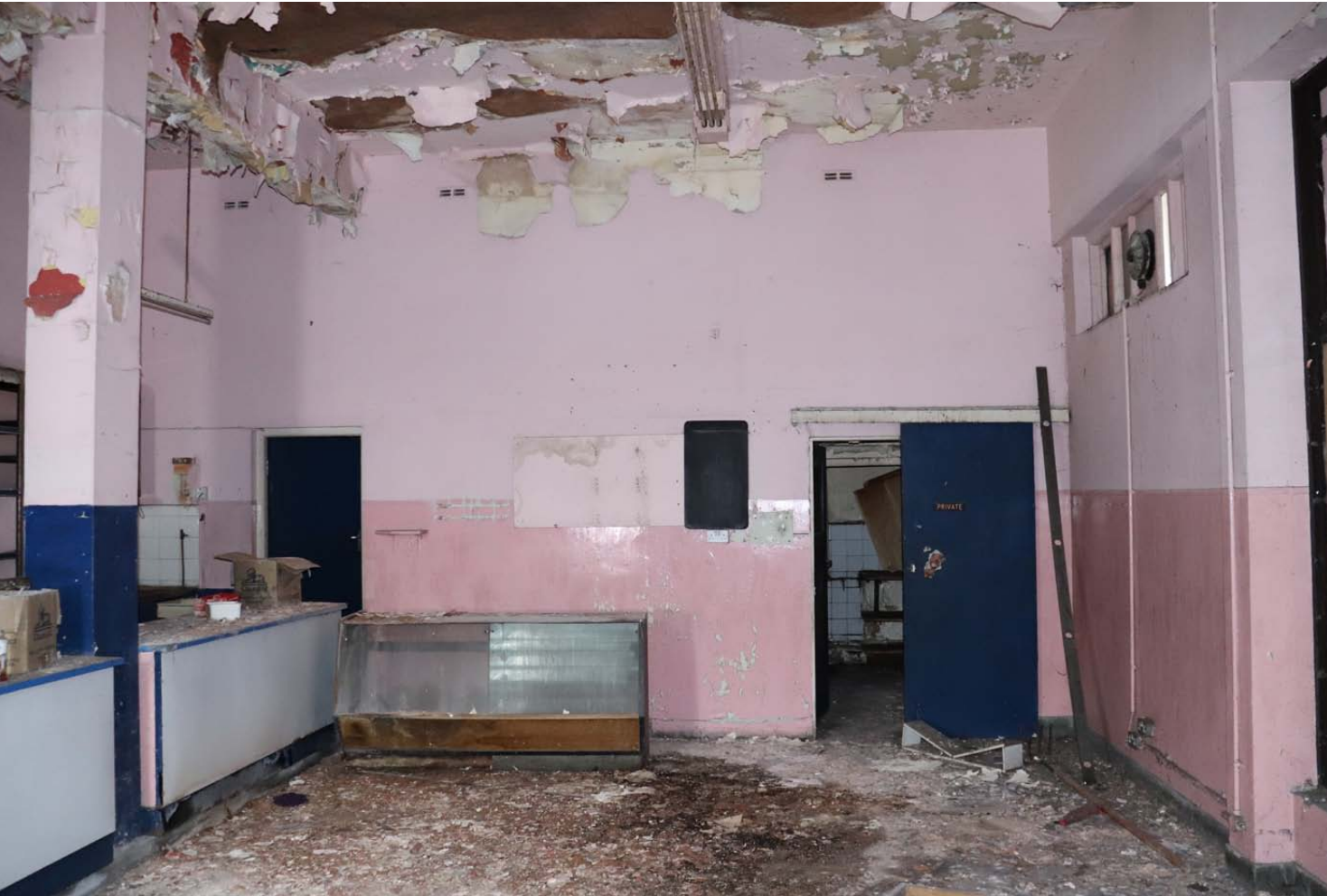
View of Rear of the unit with the Toilet & Kitchenette accessed to the right and the Store to the left
