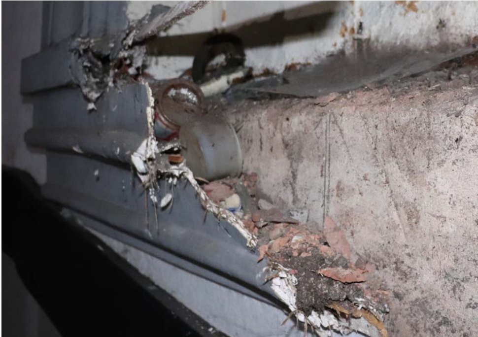
View of plaster profile to front face of window cill
