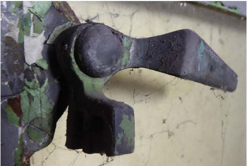
View of two-point cockspur fastener to casements
