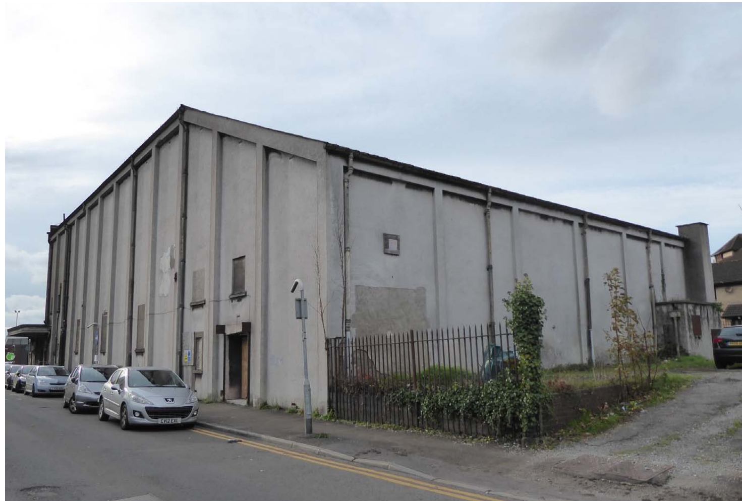
View from the north east corner
