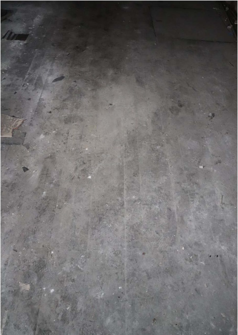
View of timber boarded Flooring to stage
