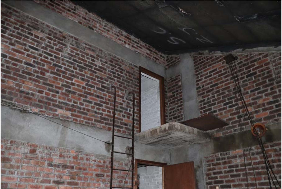
View of brickwork within concrete frame to raised section
