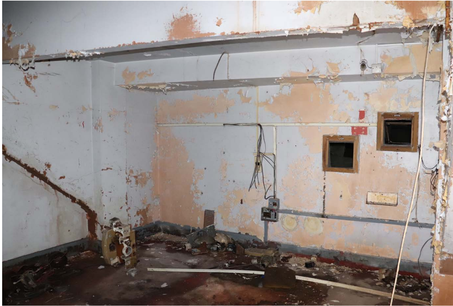
View of north Projection Wall with 2no. projection openings
