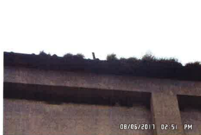
Overgrowth in high level gutters (June 2017) Overgrowth removed via MEWP (July 2017)
