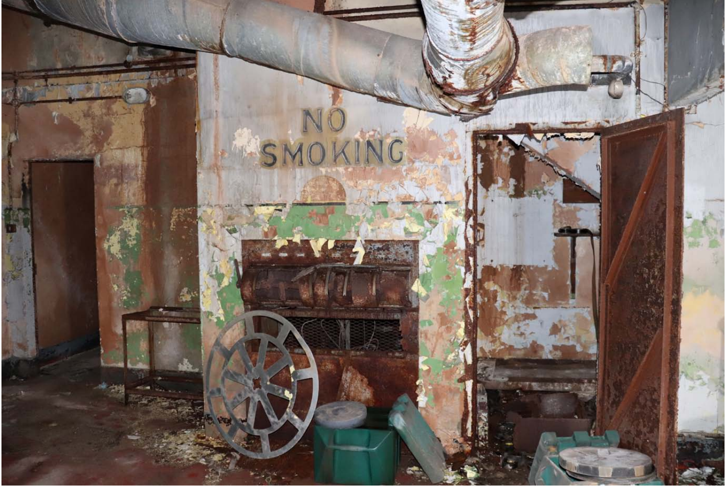
View of west wall with small store room beyond
