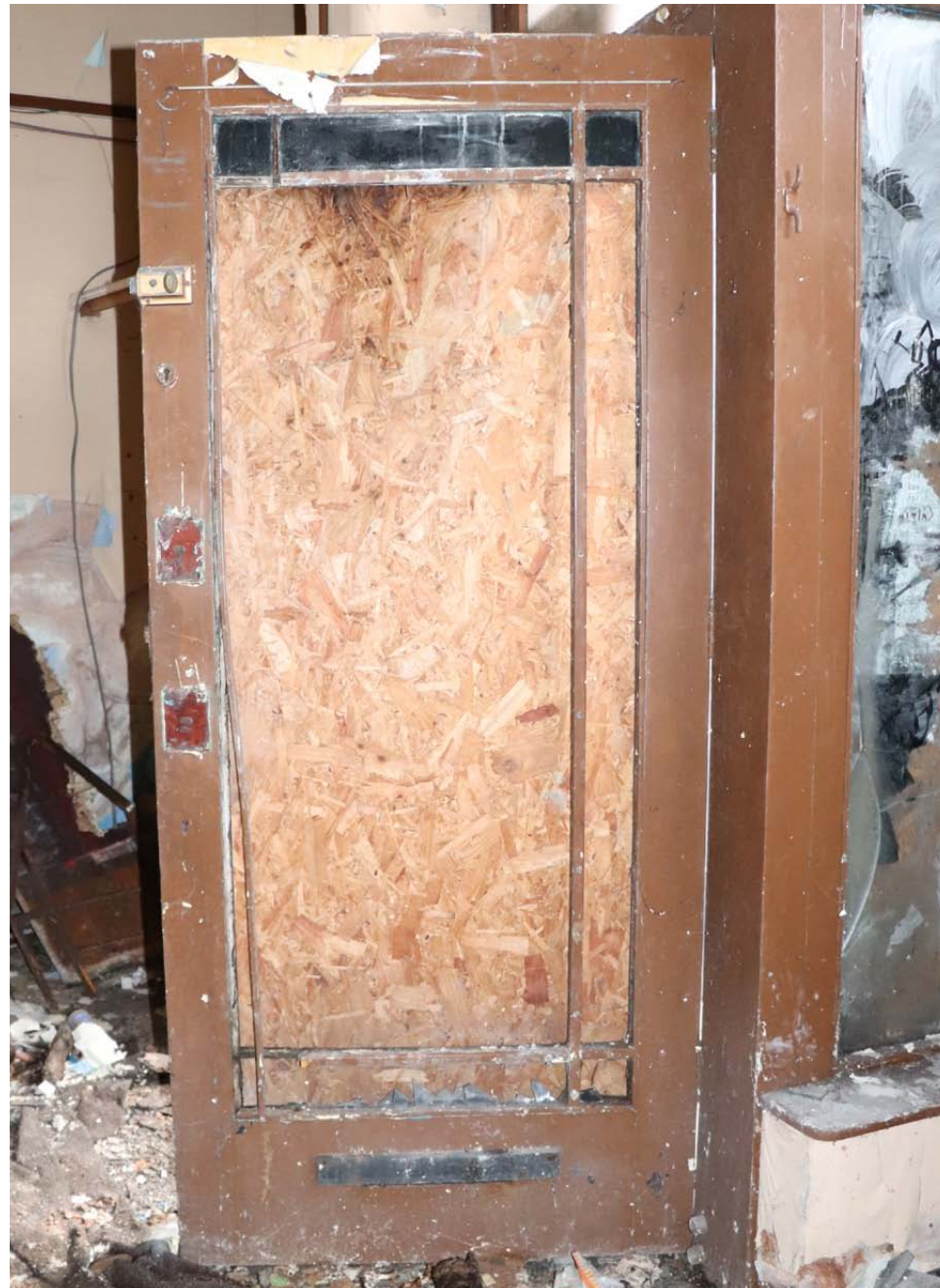
Timber-framed Glazed External Door with perimeter glazed panes
