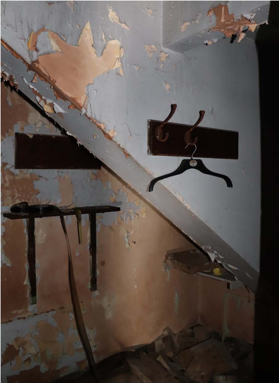
View of Store room showing raking concrete 'beam' to seating above
