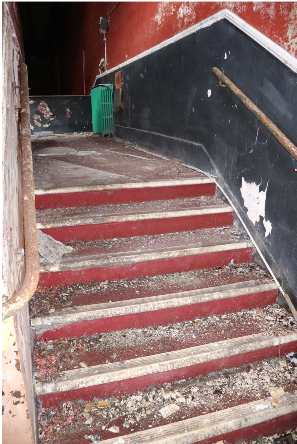
View of last flight of stairs leading into auditorium balcony
