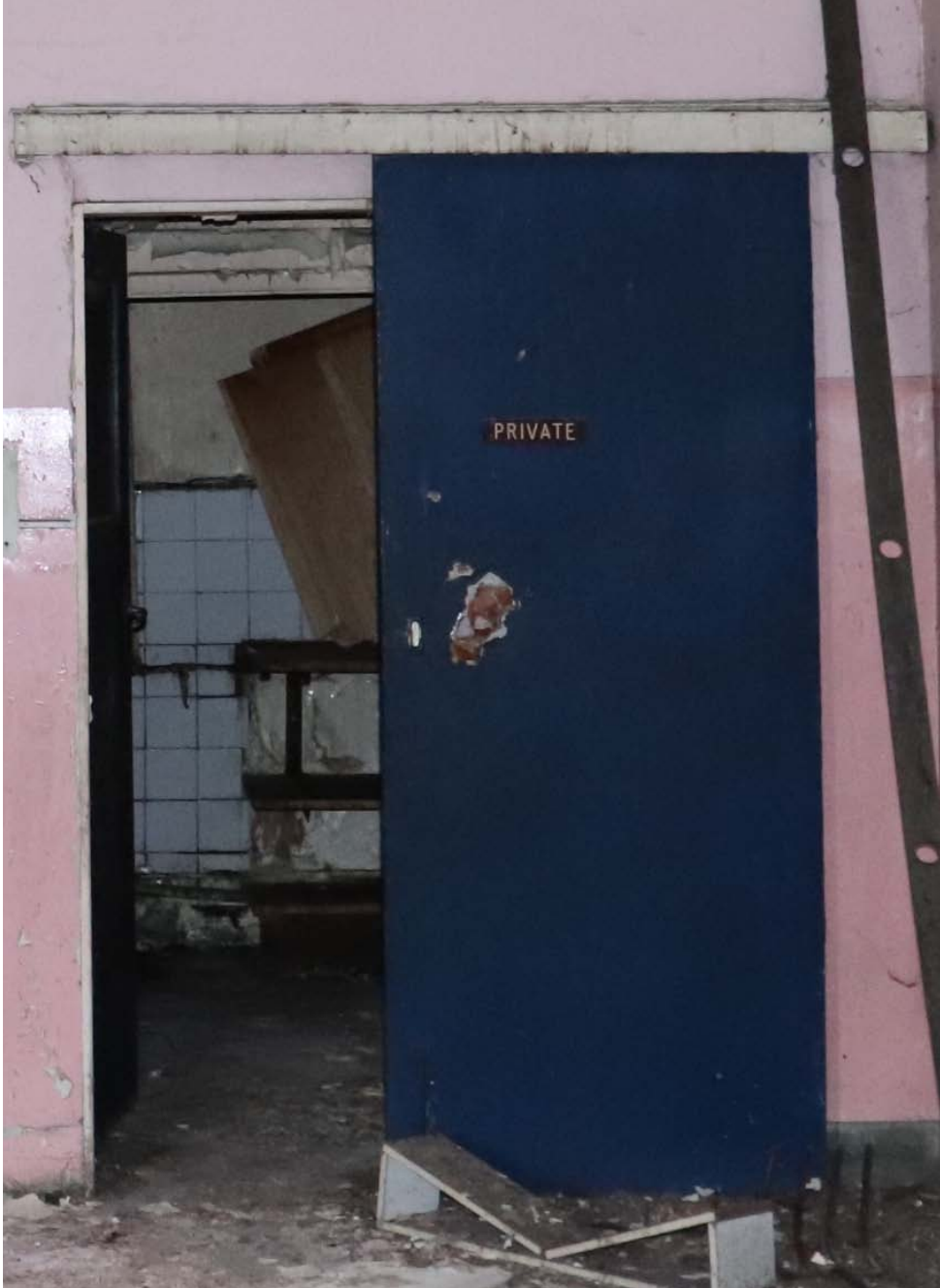
View of Sliding Door from Retail space to rear spaces
