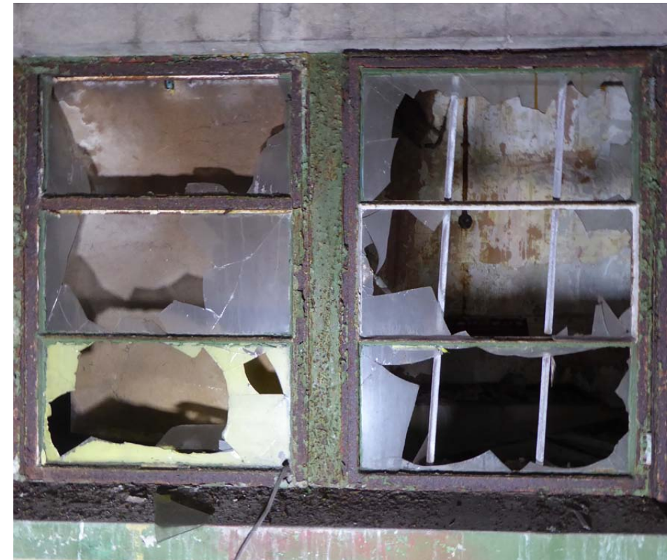
View of corrosion to steel frame sections at mullion
