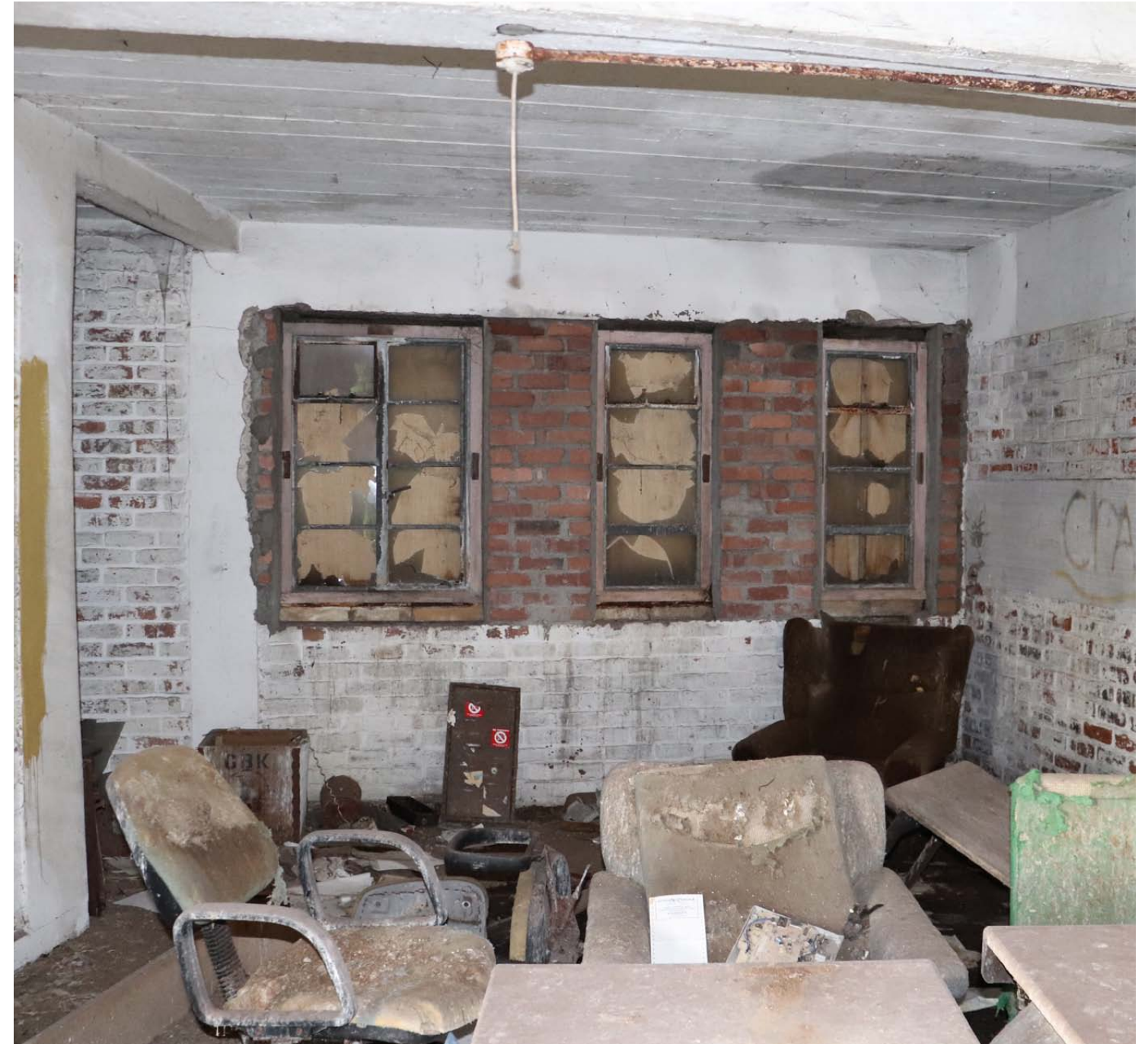
View of the west elevation of the room
