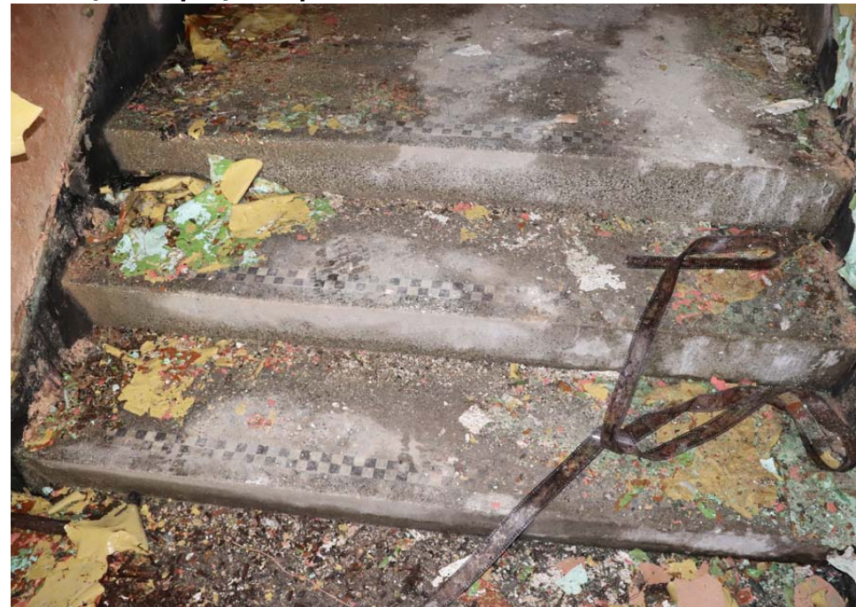
View of detail of treads with black and white chequerboard nosing
