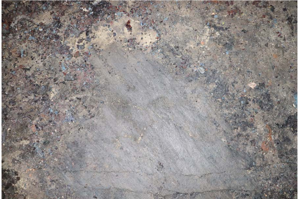
View of painted concrete floor
