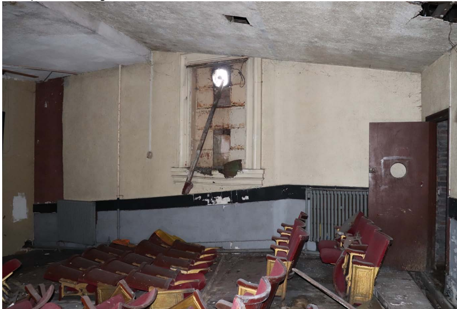
View of Cinema looking east
