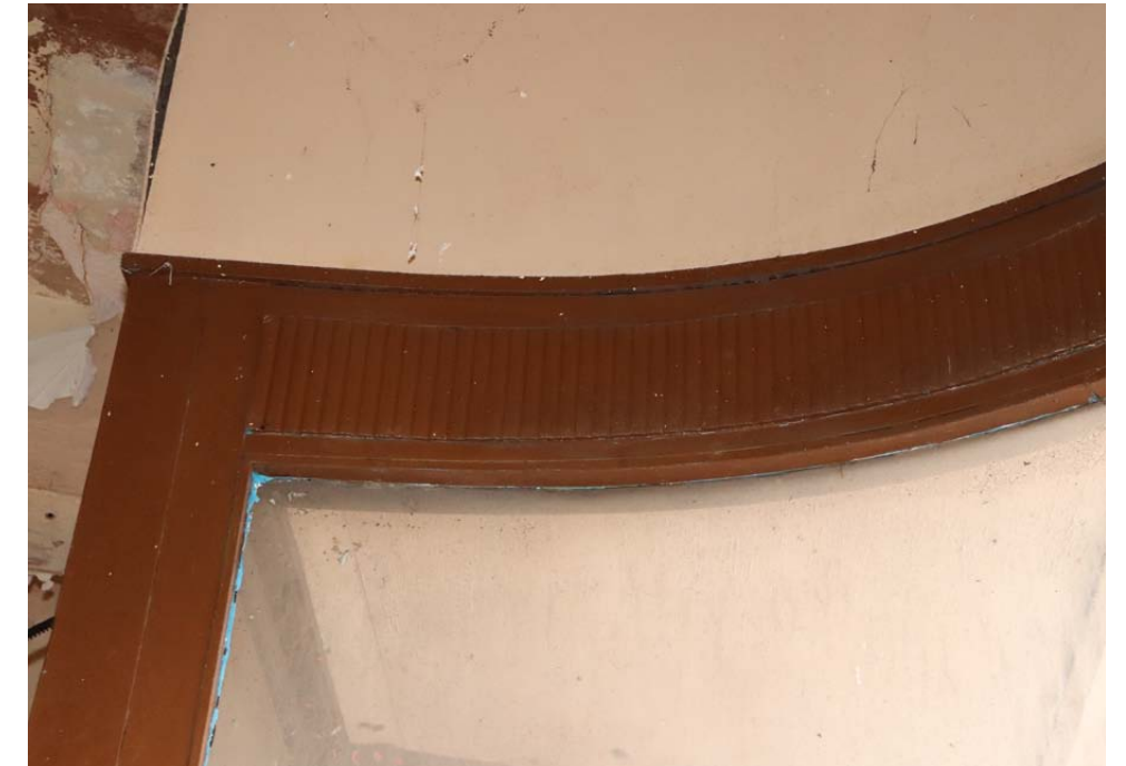
View of Vented Strip to top of Glazing - in this area, the vent is closed
