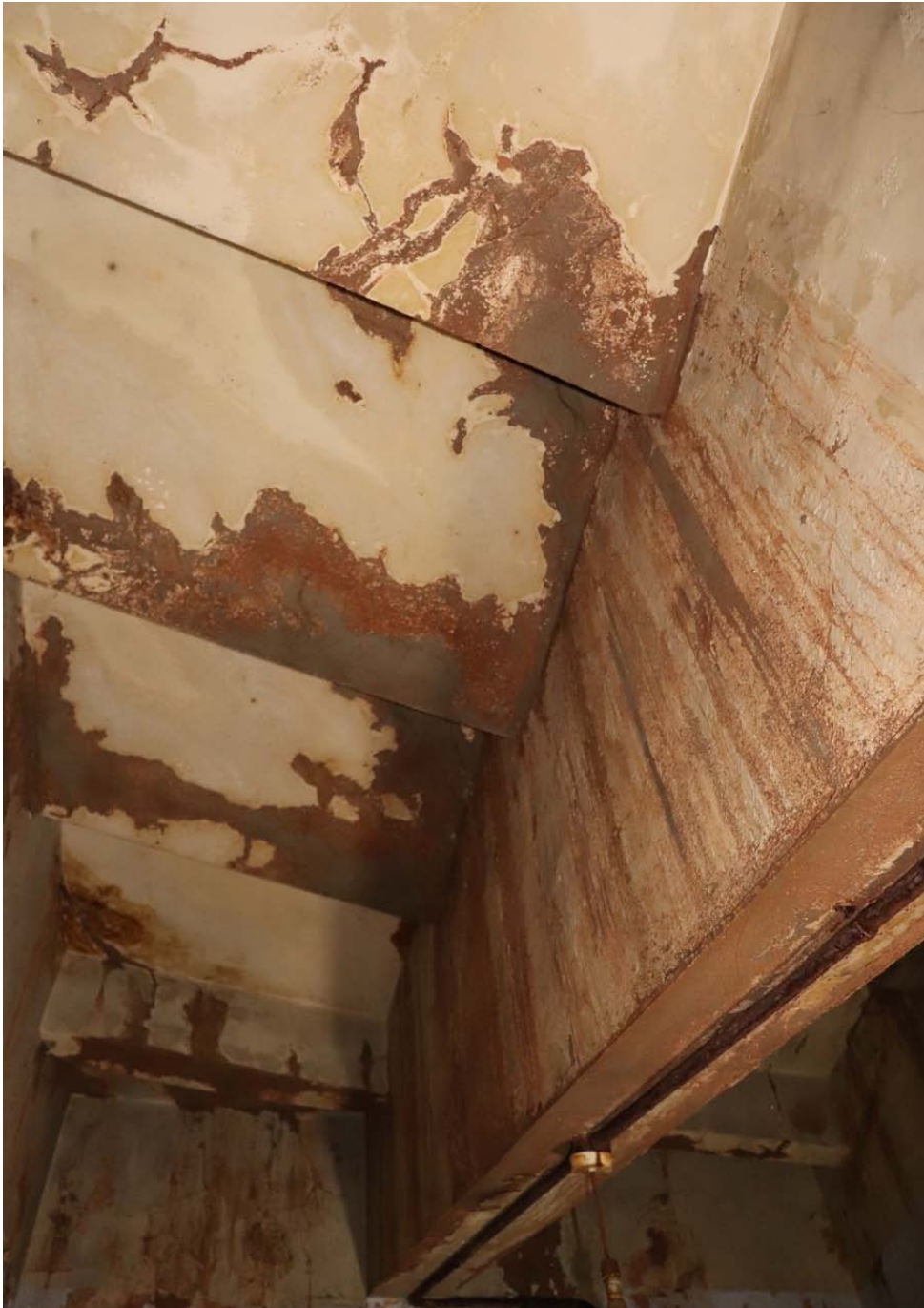
View of soffit showing raking concrete 'beam' and flat seating above
