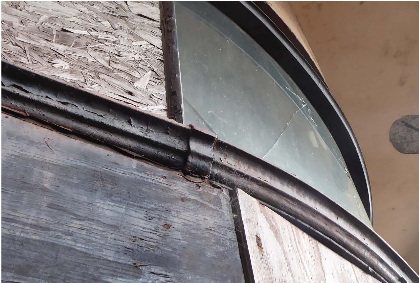
Views of top of curved frontage to timber-framed glazing to the larger (right-hand) Retail unit, showing profile to timber head section and lower transom section and vertical glazing bar with aerofoil profile
