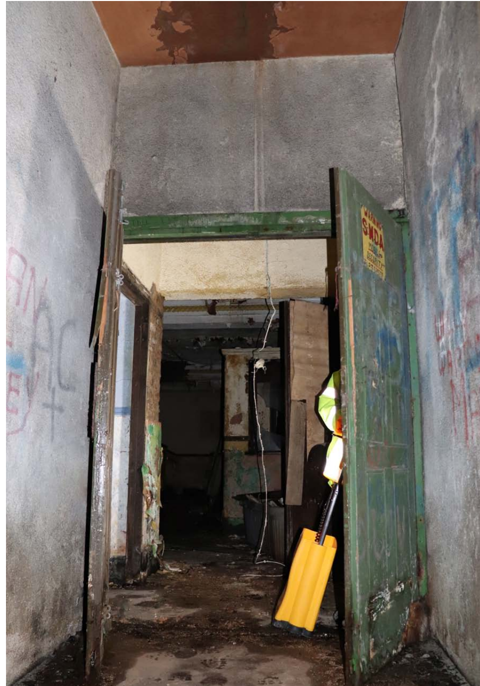
View of internal door at top of steps
