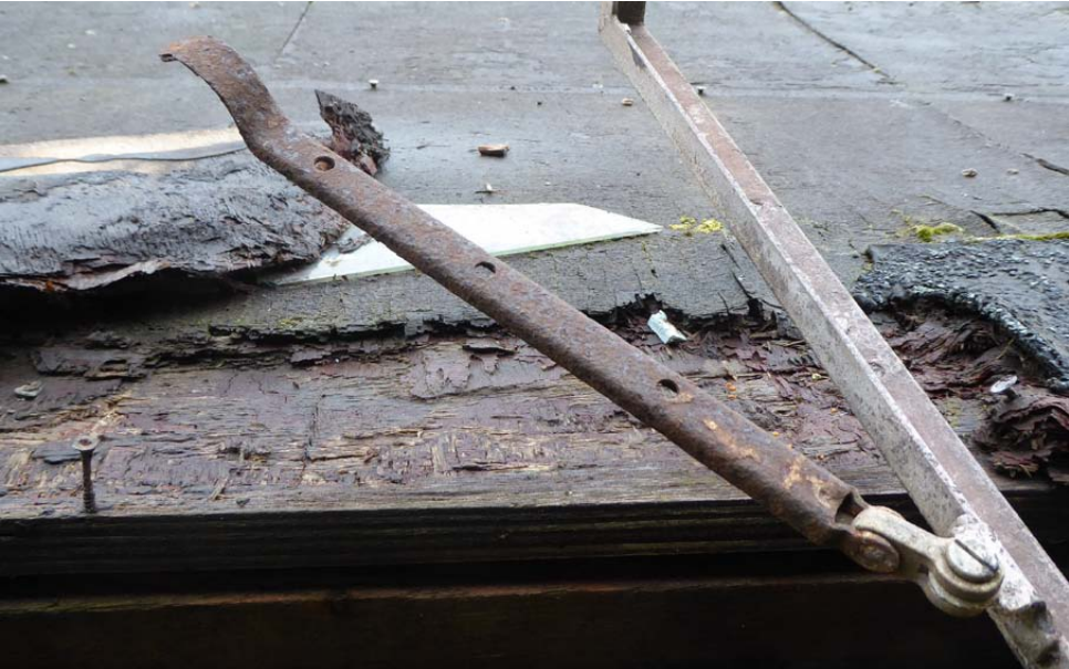
View of example of stay to windows
