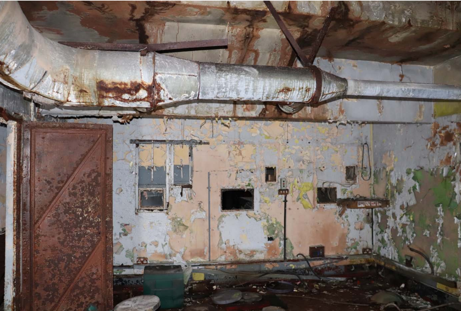
View of north Projection Wall with series of projection openings
