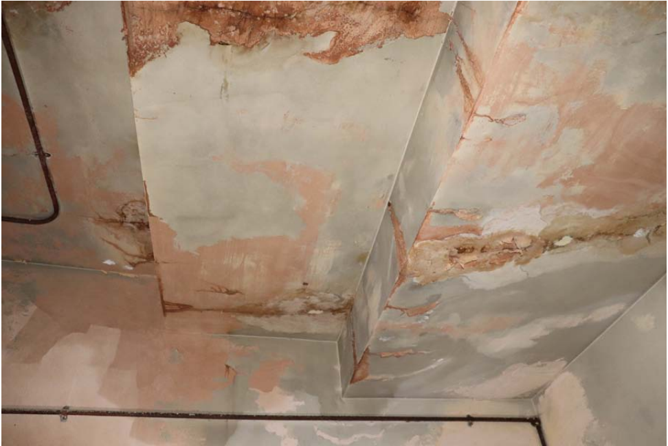
Further view of soffit showing flat concrete seating above
