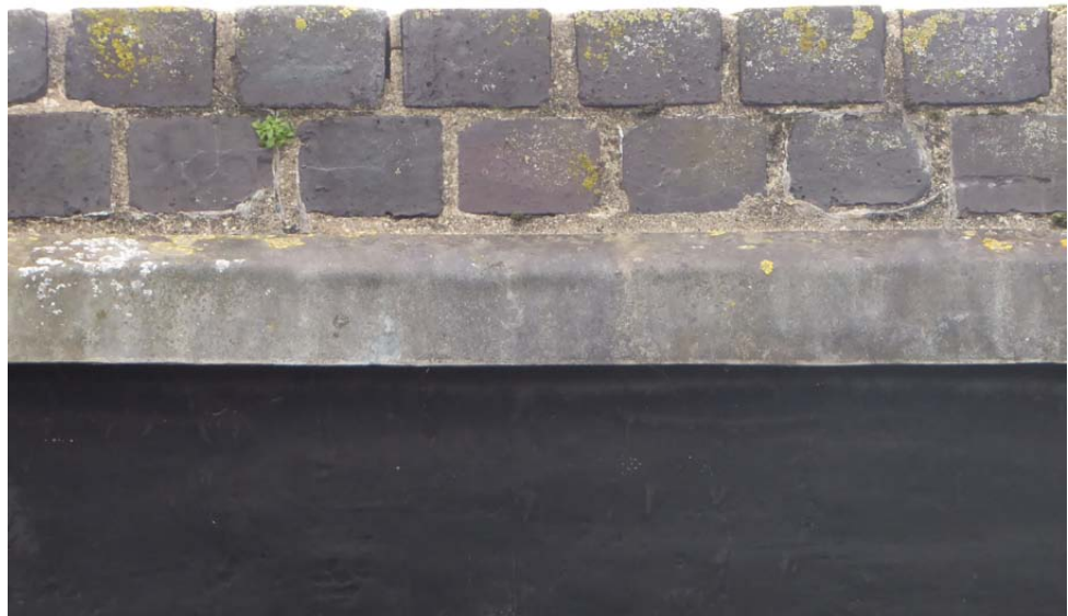
View of top of walls with two brick courses over a lead flashing
