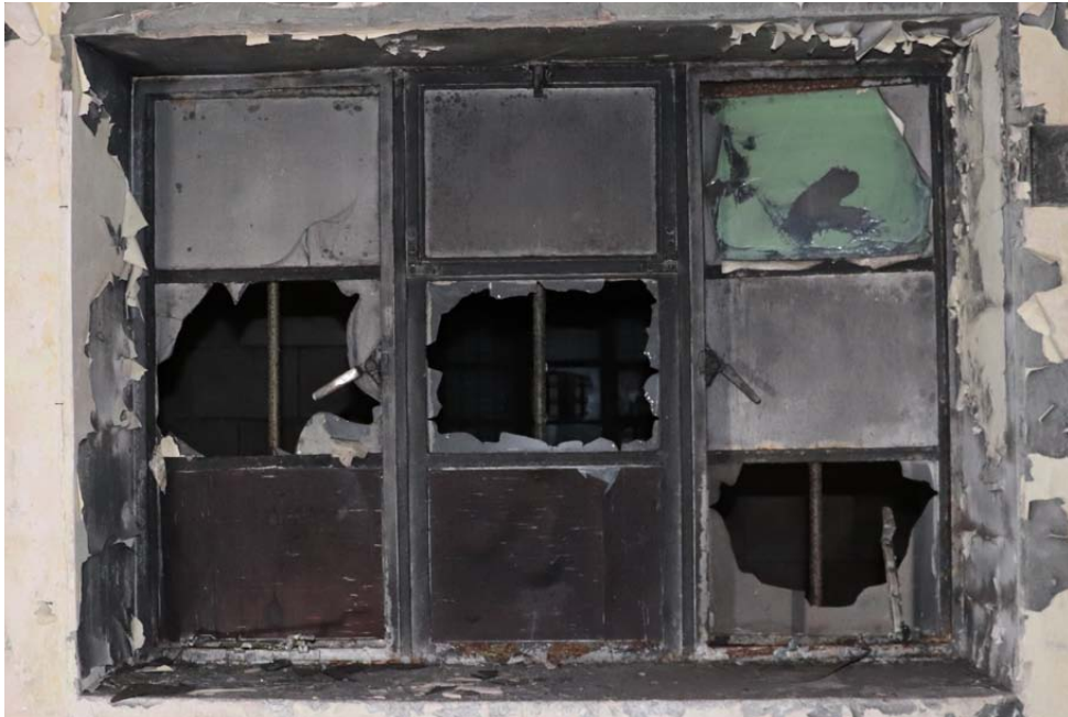
View of window in east wall
