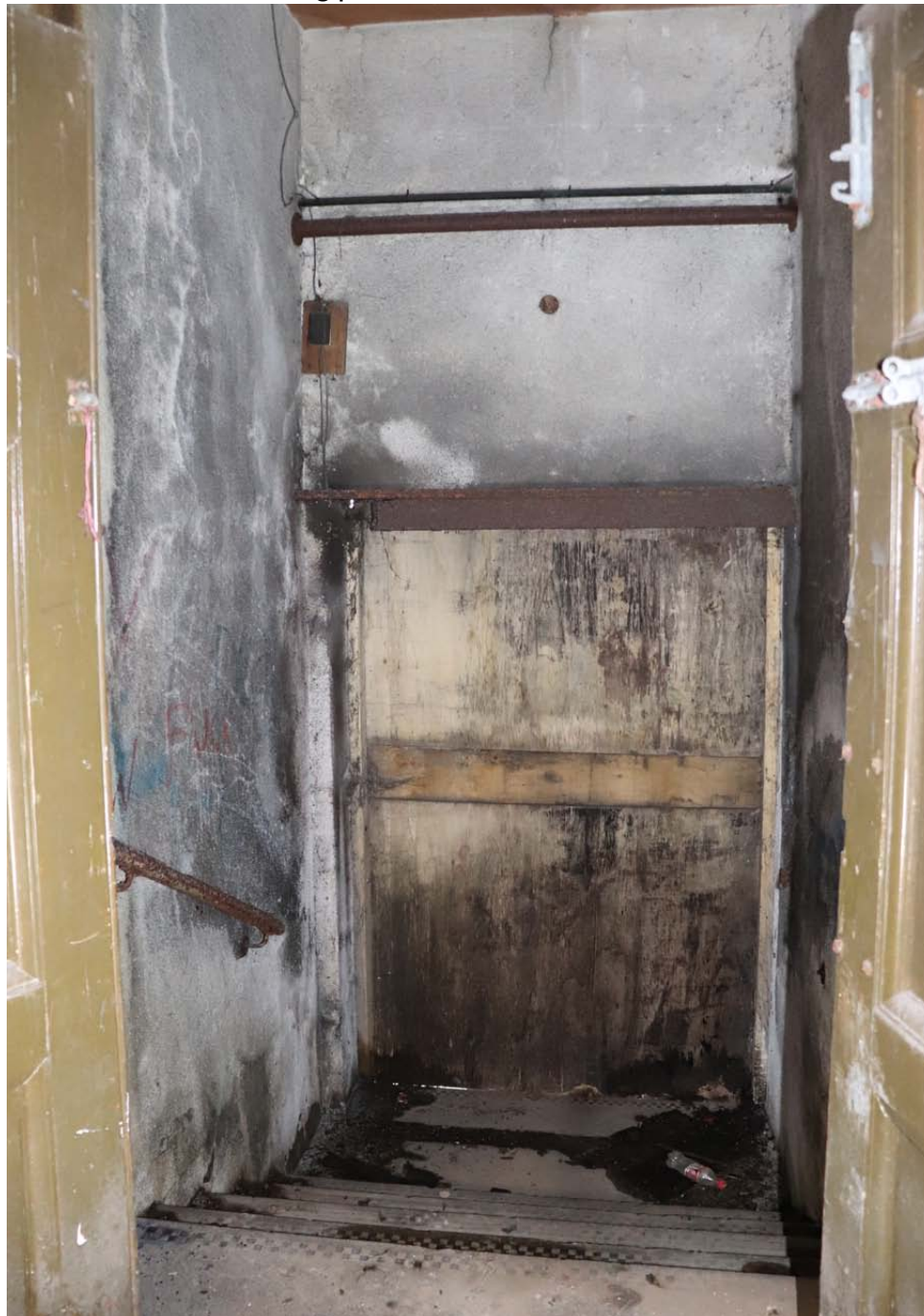
View of external door at base of steps
