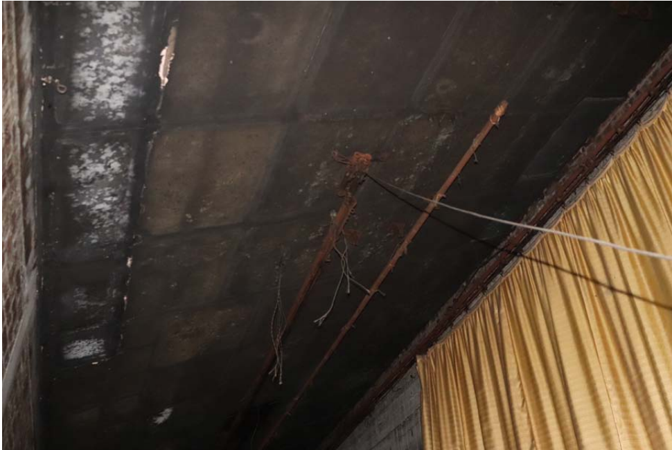
View of black painted soffit boarding
