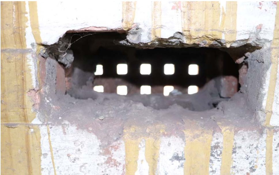
View of vent within brickwork of wall
