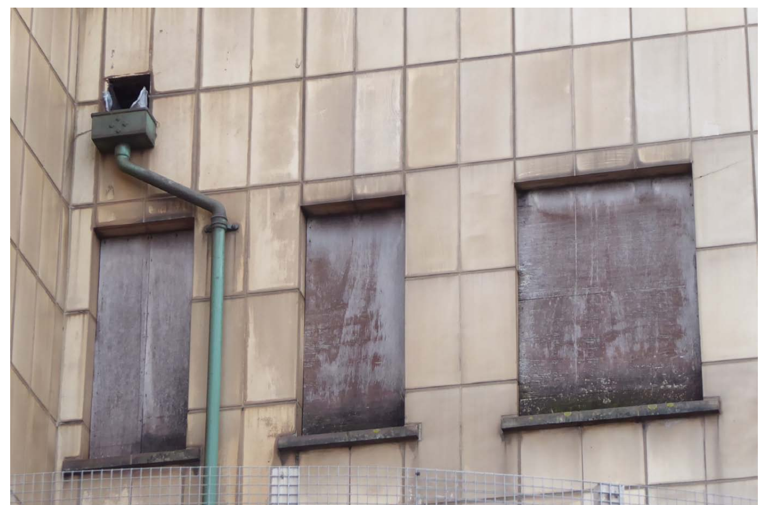
View of the three windows to the left hand side, facing west
