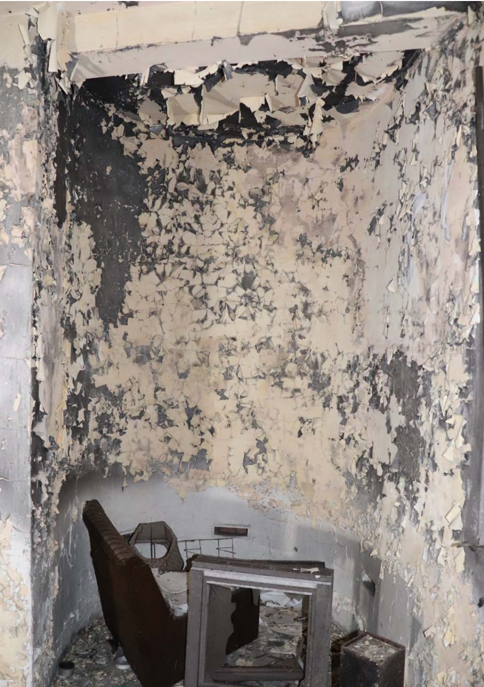
View rounded apse-like recess in south wall
