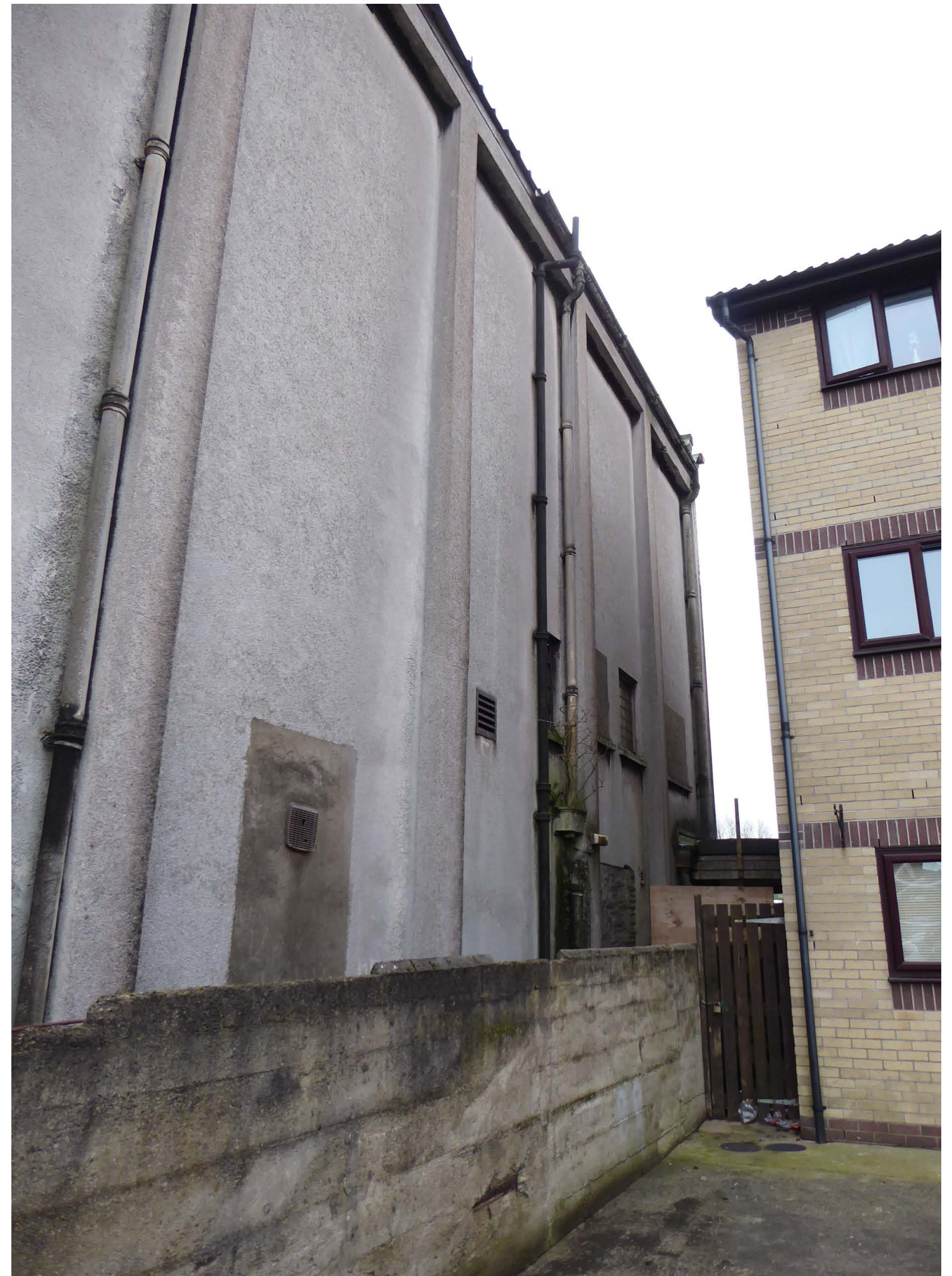
View of Right of Way with Plaza to the left and Eagle Mews housing to the right
