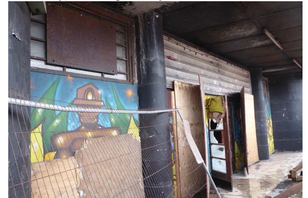
G Timber-framed Entrance Doors to be Retained & Restored
