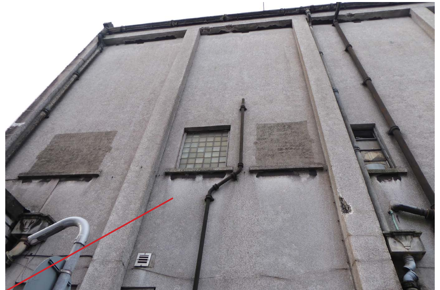
View of windows (and blocked up windows) at high level
