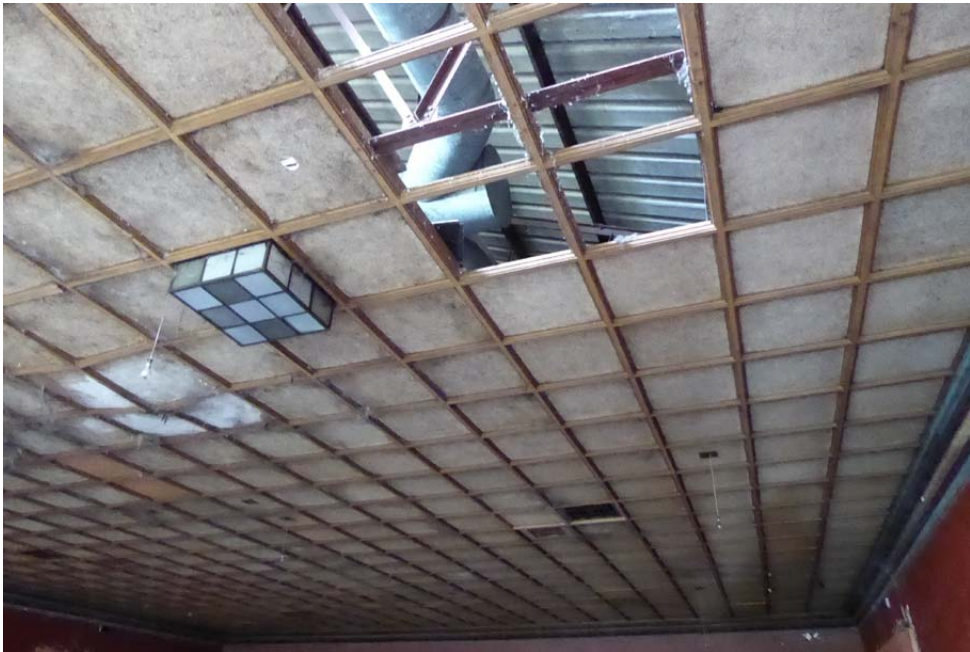
View of the ceiling looking northwards
