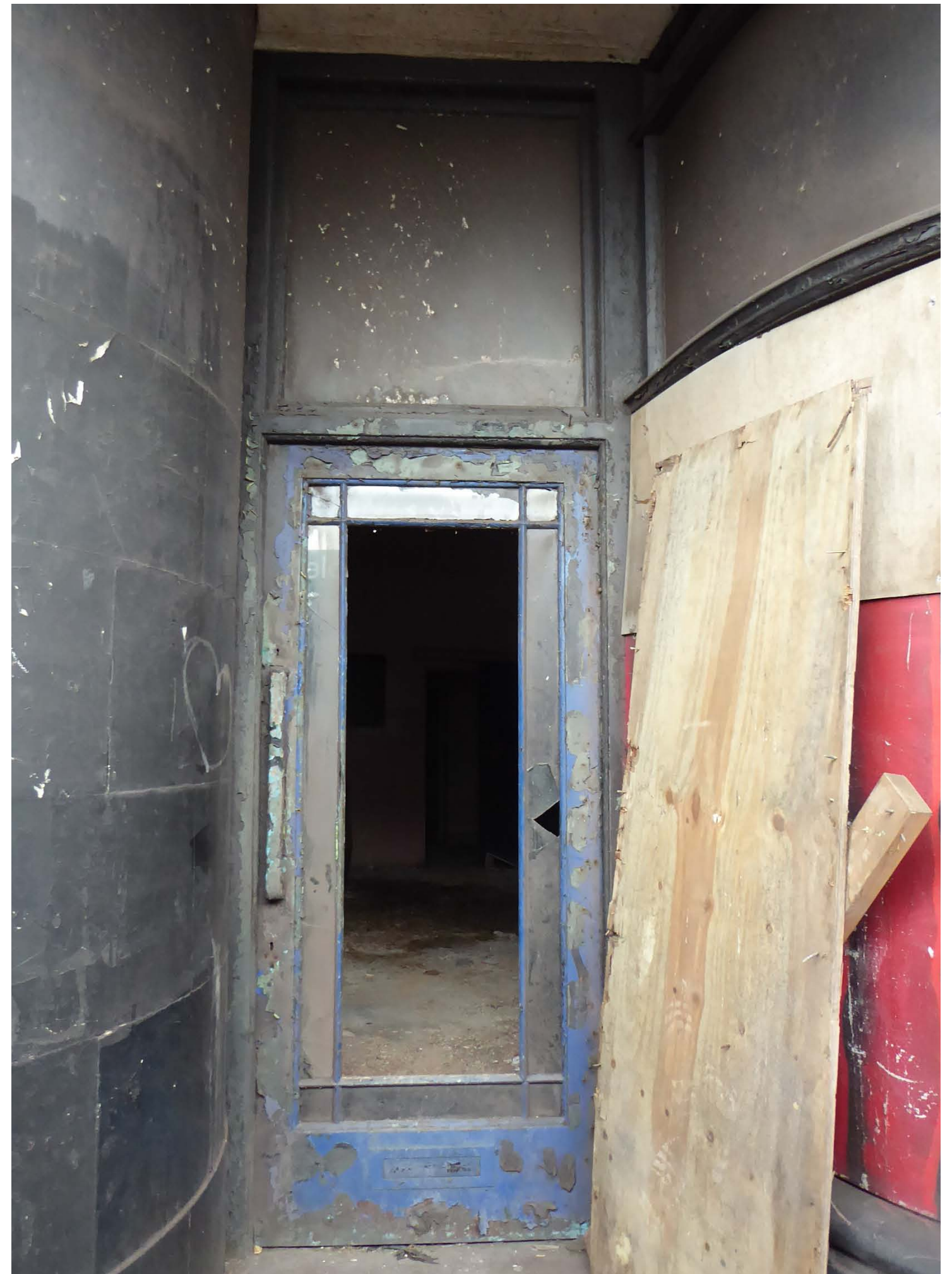
View of glazed door and overpanel to single door to right hand (larger) retail unit
