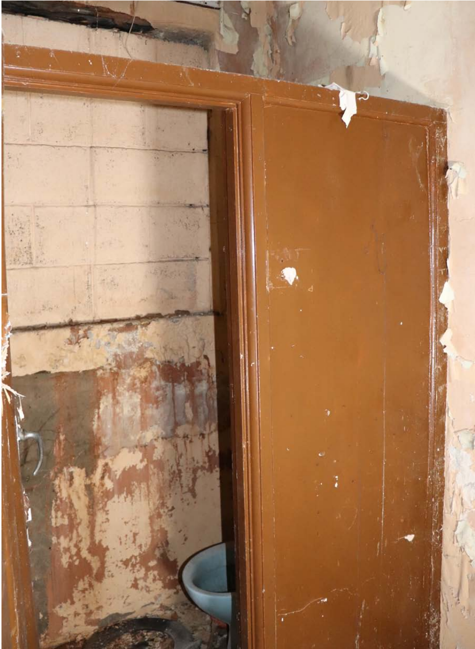
Further view of Timber Cubicle Partition
