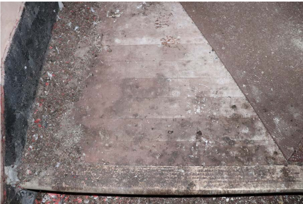
View of timber board flooring at top of stairs underneath carpet
