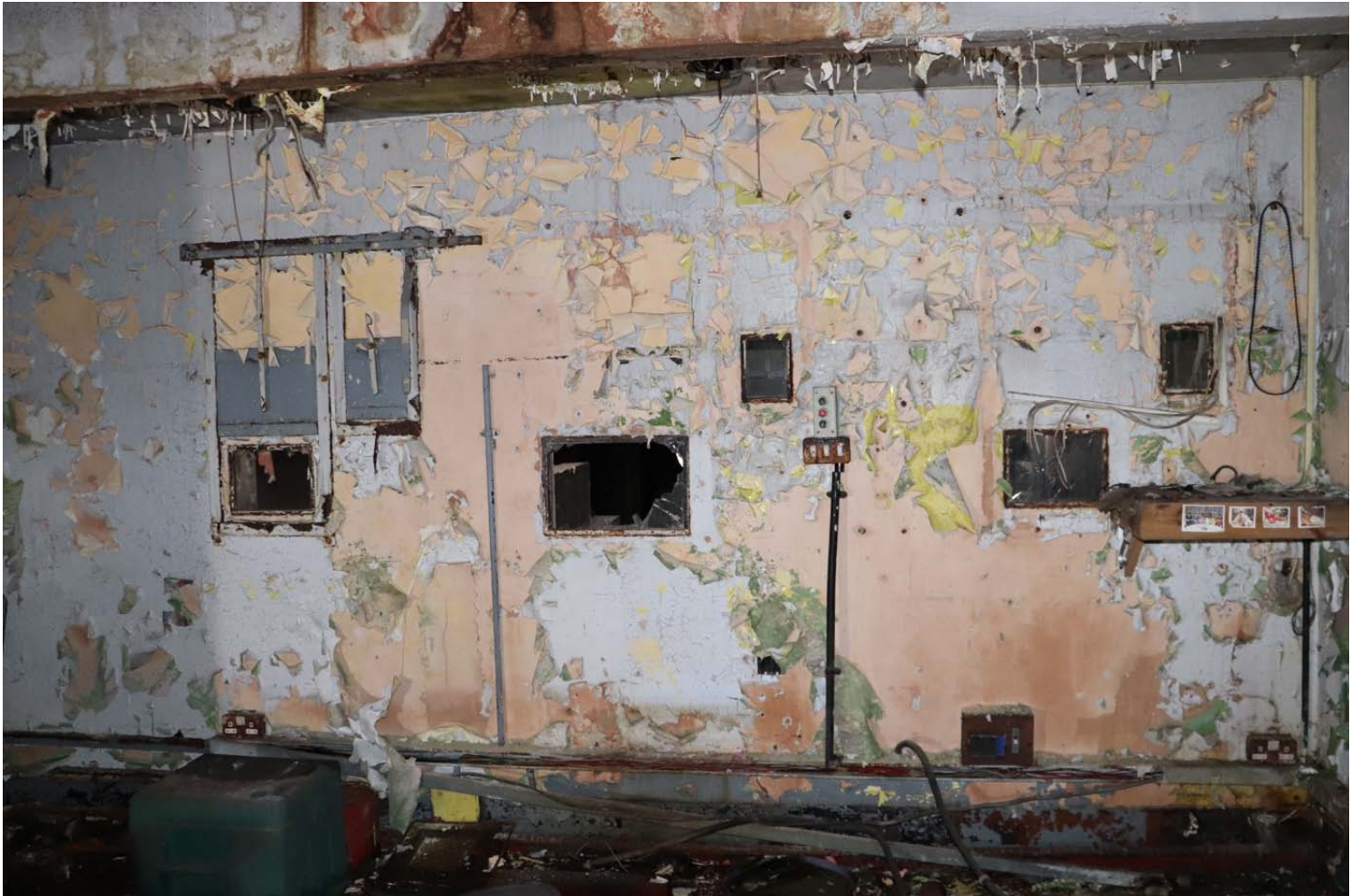
View of glazed projection openings as seen straight on
