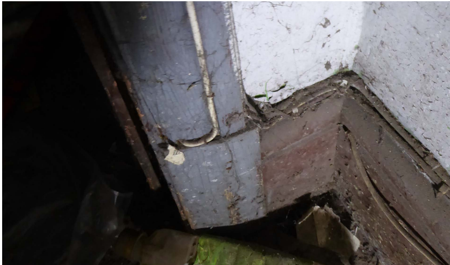
View of profiles of skirting and door architrave in the space
