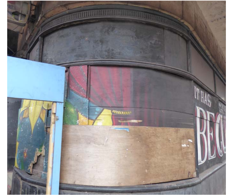
F Thick Shopfront Glazing to be Replicated
