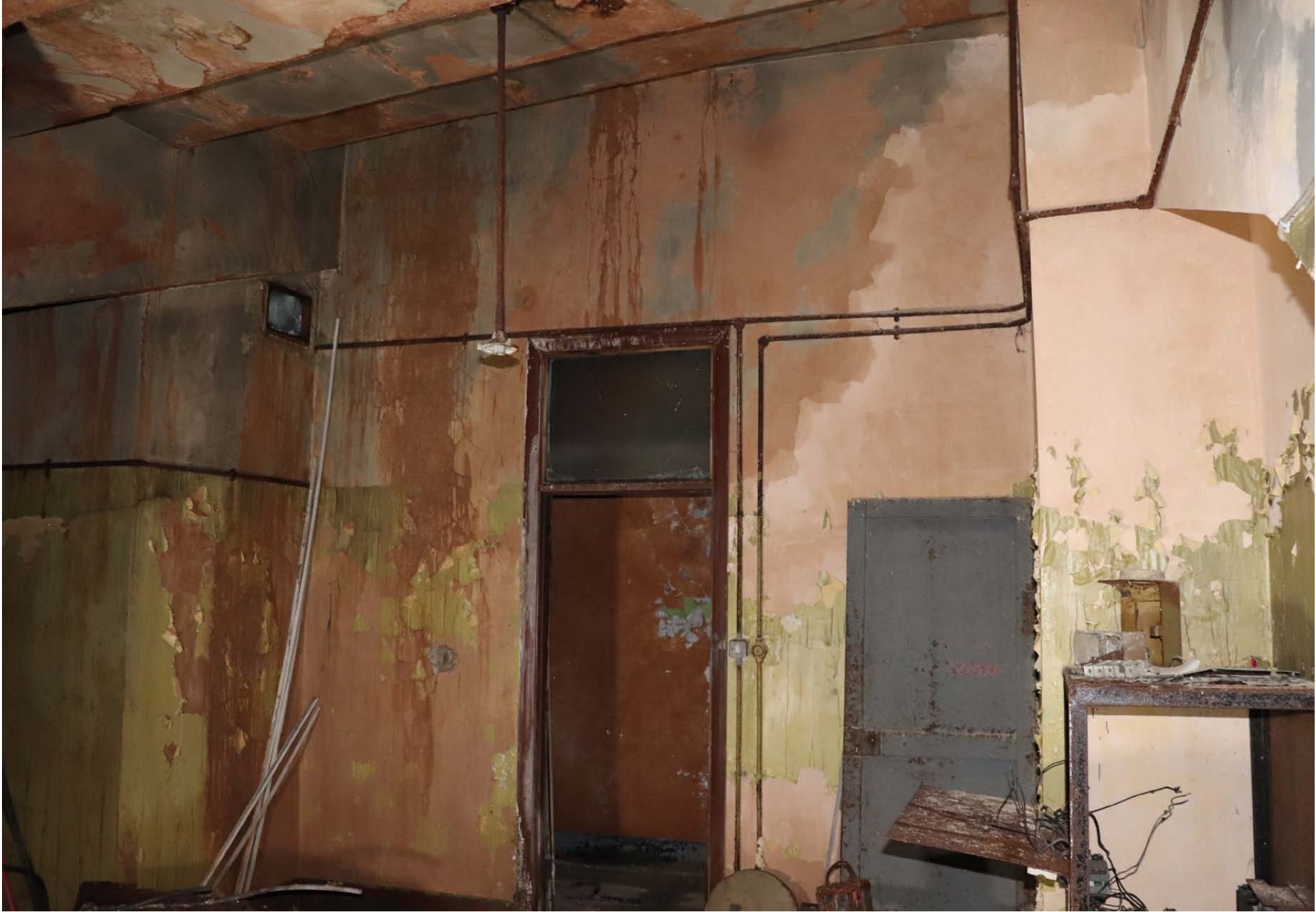
View of south wall with entrance to room
