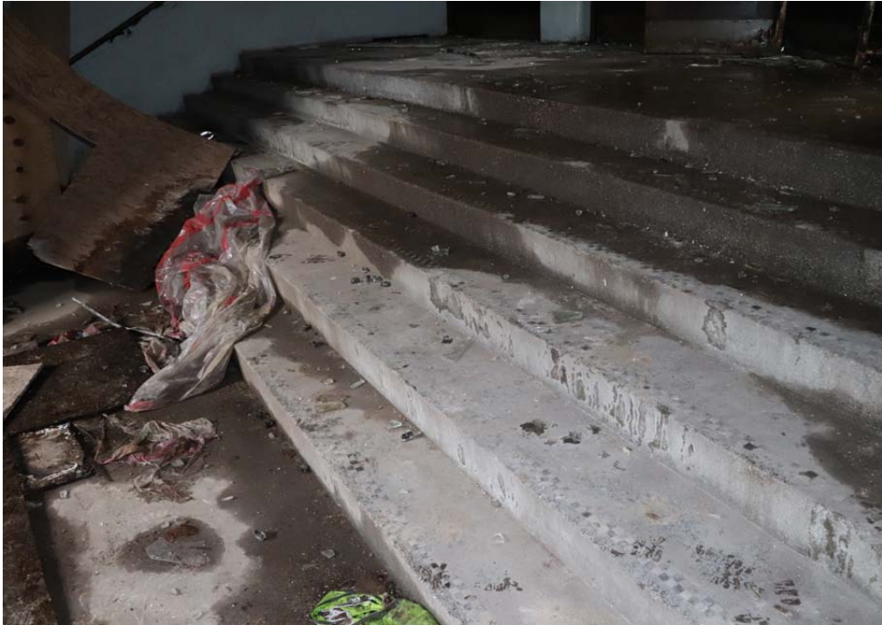
View of the run of 6no. terrazzo steps
