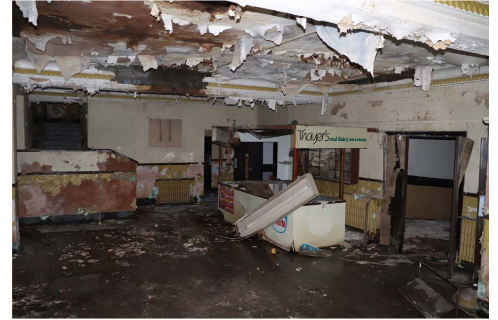
View of the Foyer looking towards the east
