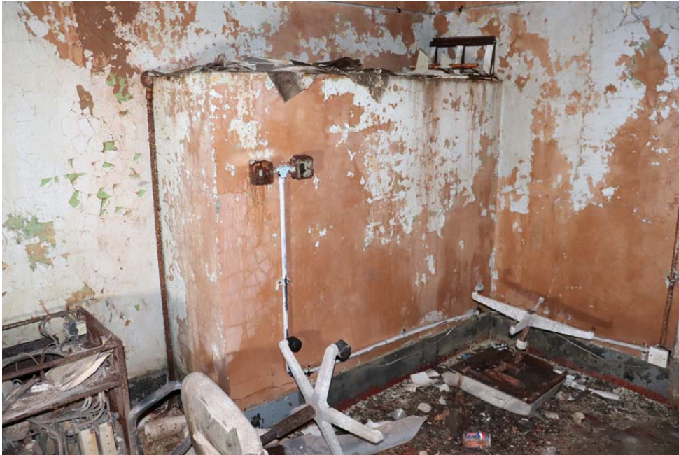
Boxed out masonry construction providing headroom to staircase
