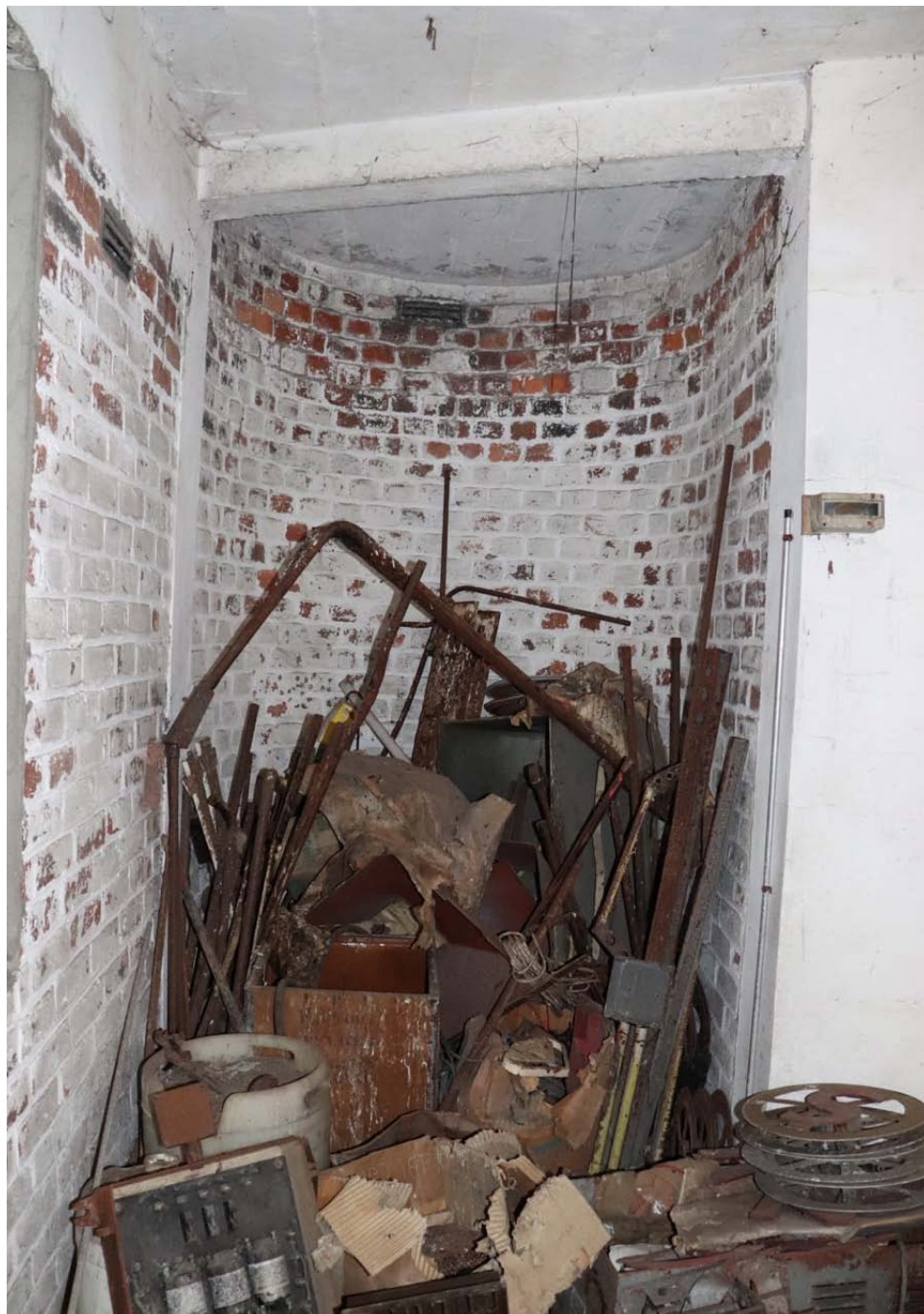
View of the brick formed curved turret end to the south east corner
