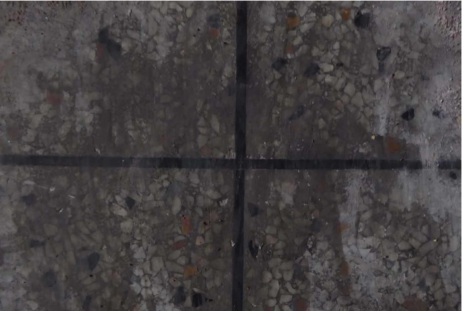
View the grey insitu terrazzo with separating strips between bays
