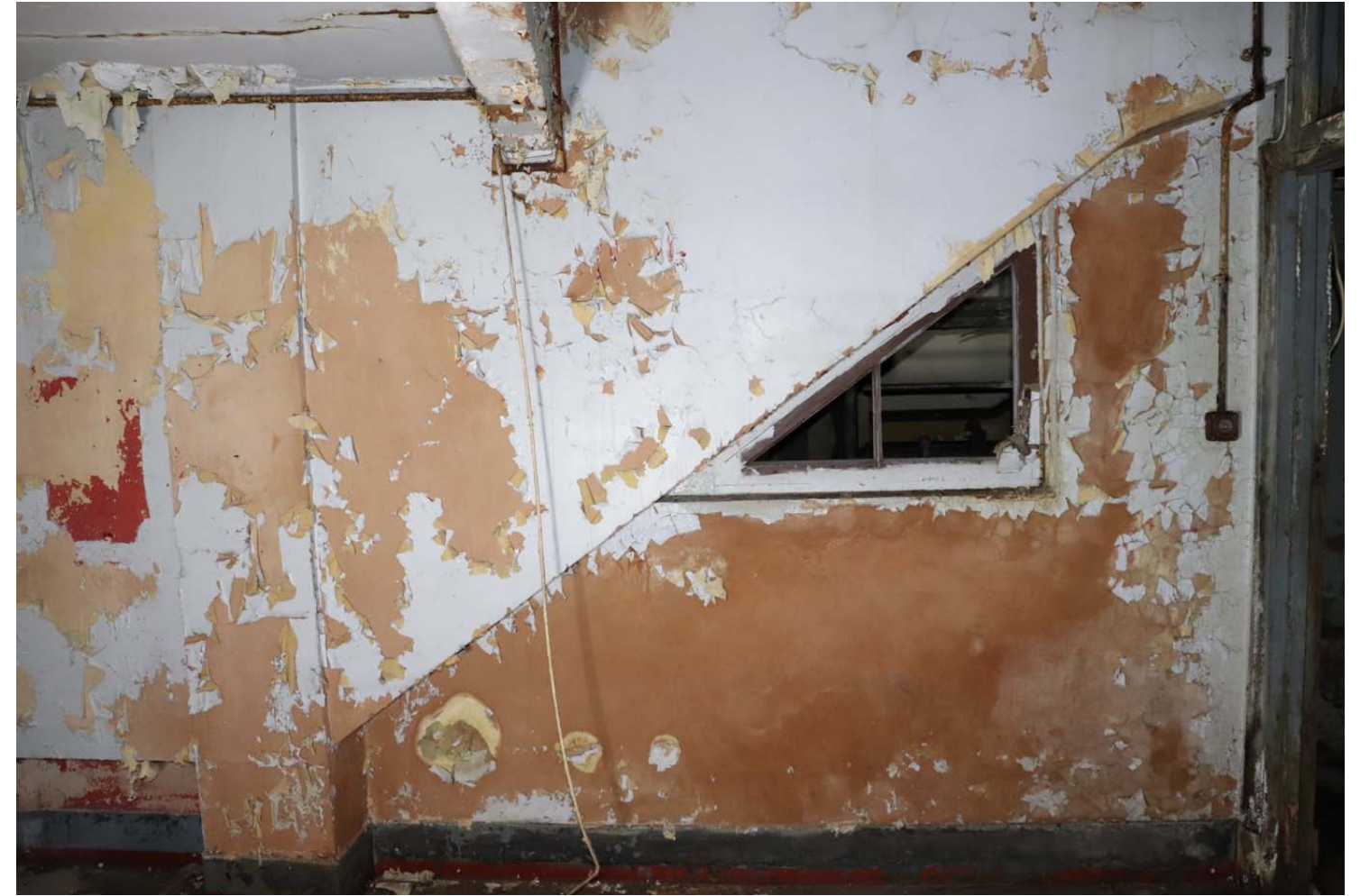
View of east wall to space showing raking concrete 'beam' to seating above
