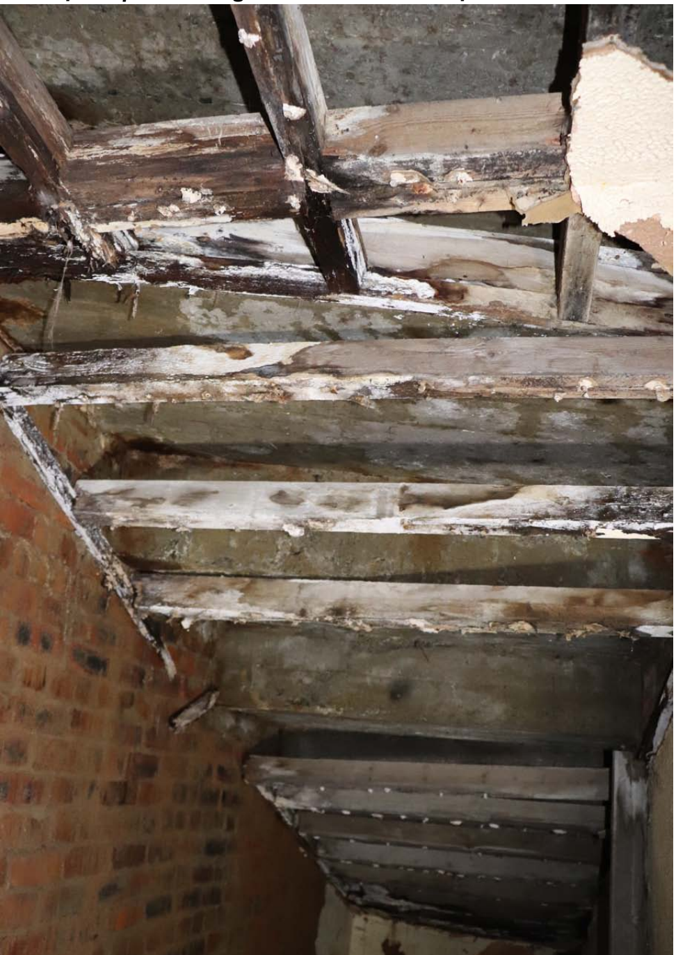
View of underside of internal flight
