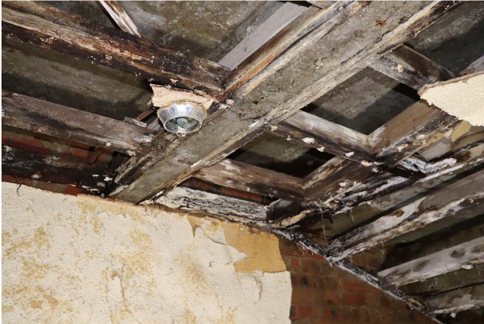
View of underside of upper landing
