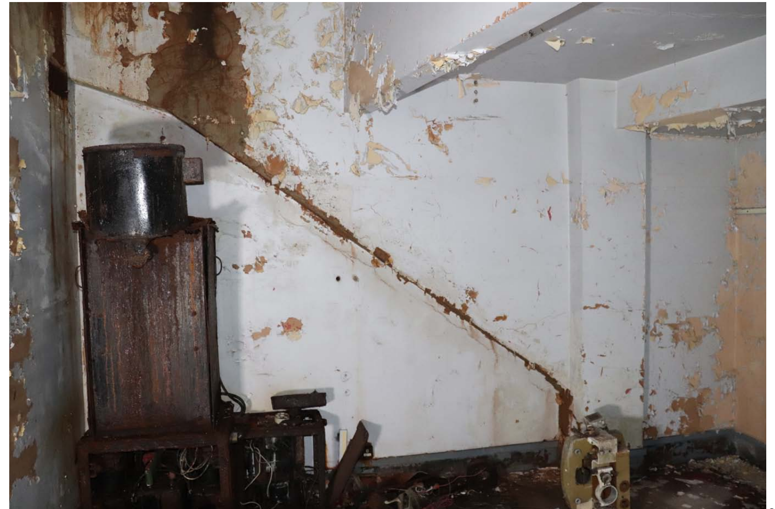
View of west wall to space showing raking concrete 'beam' to seating above
