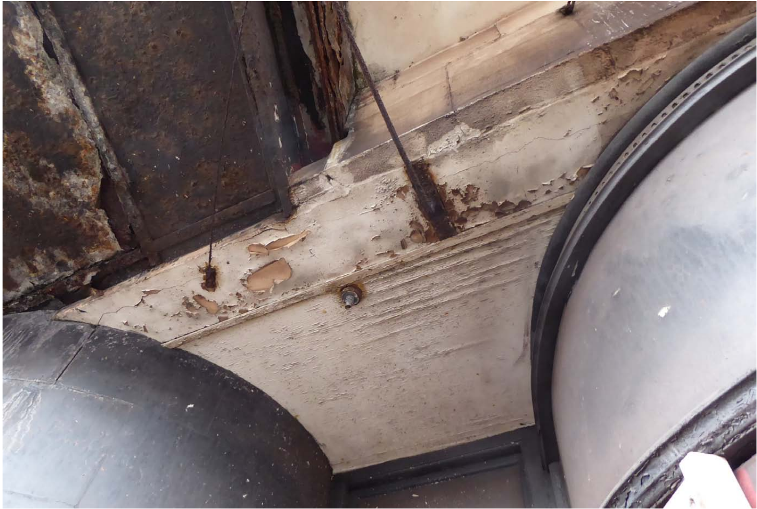
View of head of glazed overpanel to door to right hand (larger) retail unit with faience facing
