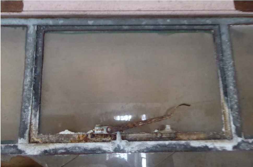
View of example of top-hinged toplight to windows
