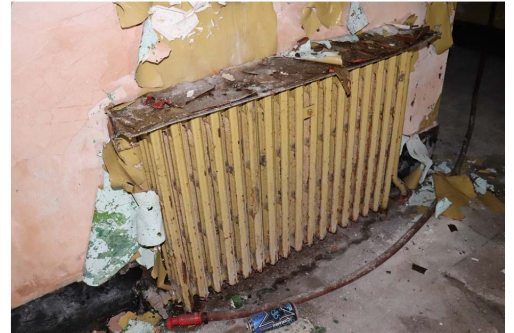
View of cast iron radiator with timber shelf
