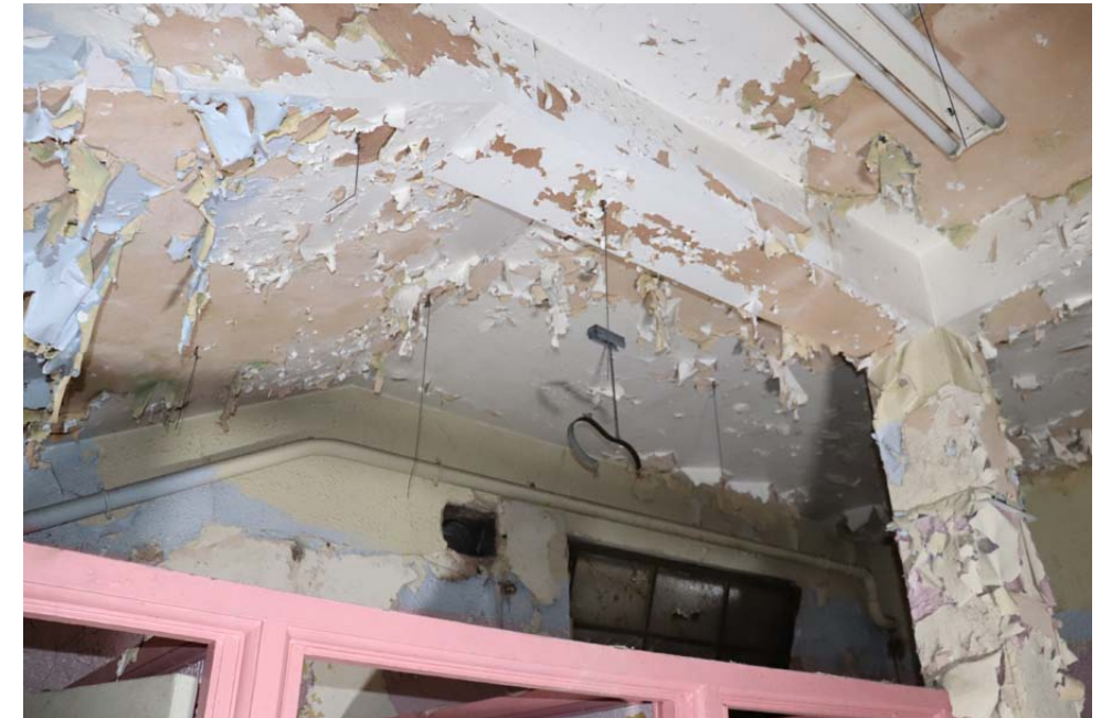
View of the Ceiling, downstand beam and column
