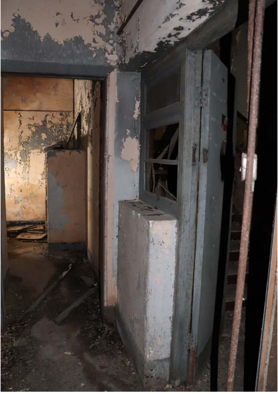
View up corridor towards masonry construction over staircase
