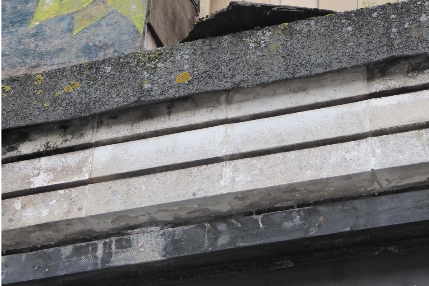
View of the 2no.rebates in the canopy edging providing an articulated profile
