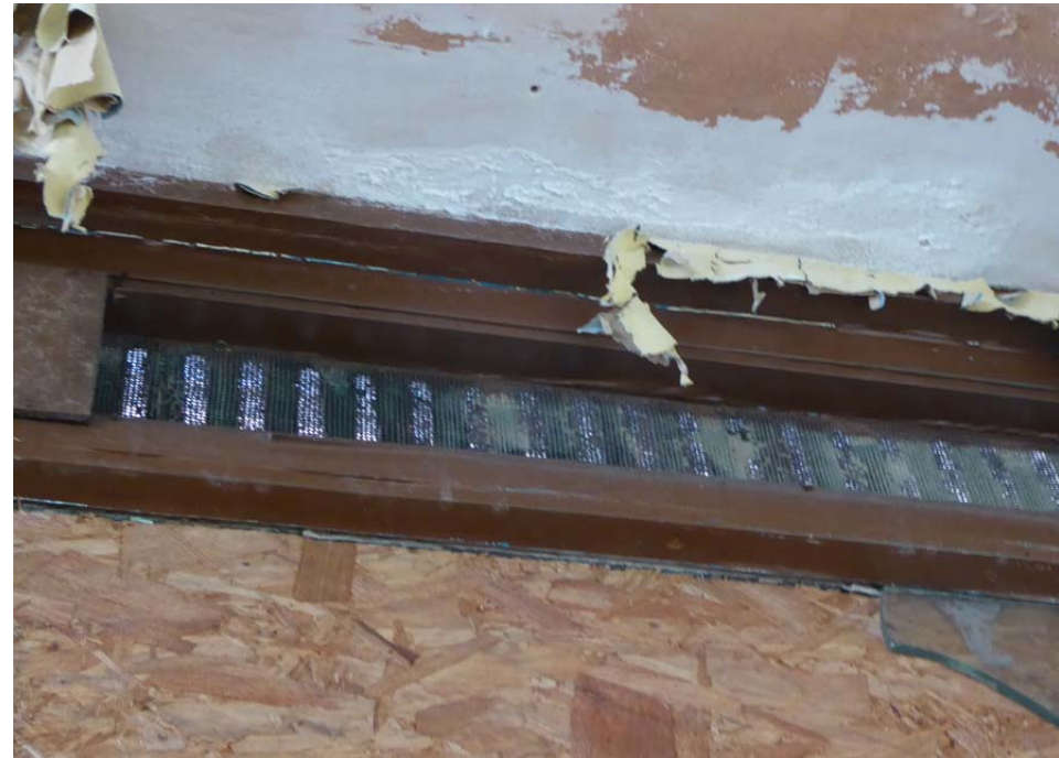
View of Vented Strip to top of Glazing - in this area, the vent is open
