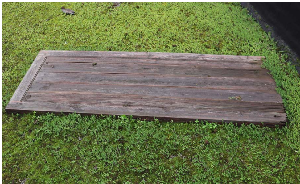
View of timber door which used to enclose box construction to ladder
