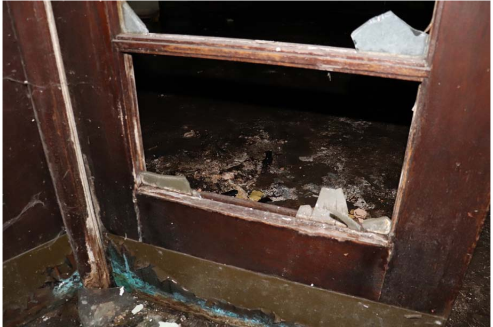
View of base of one door with glazing beads and kickplate
