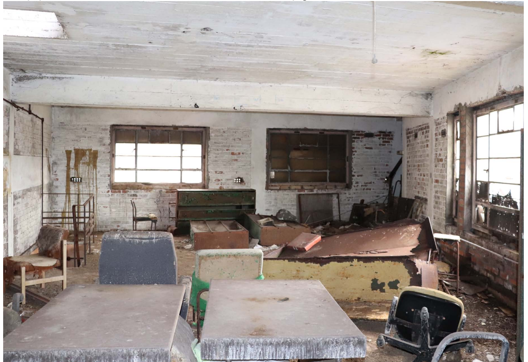
View of the east elevation of the room
