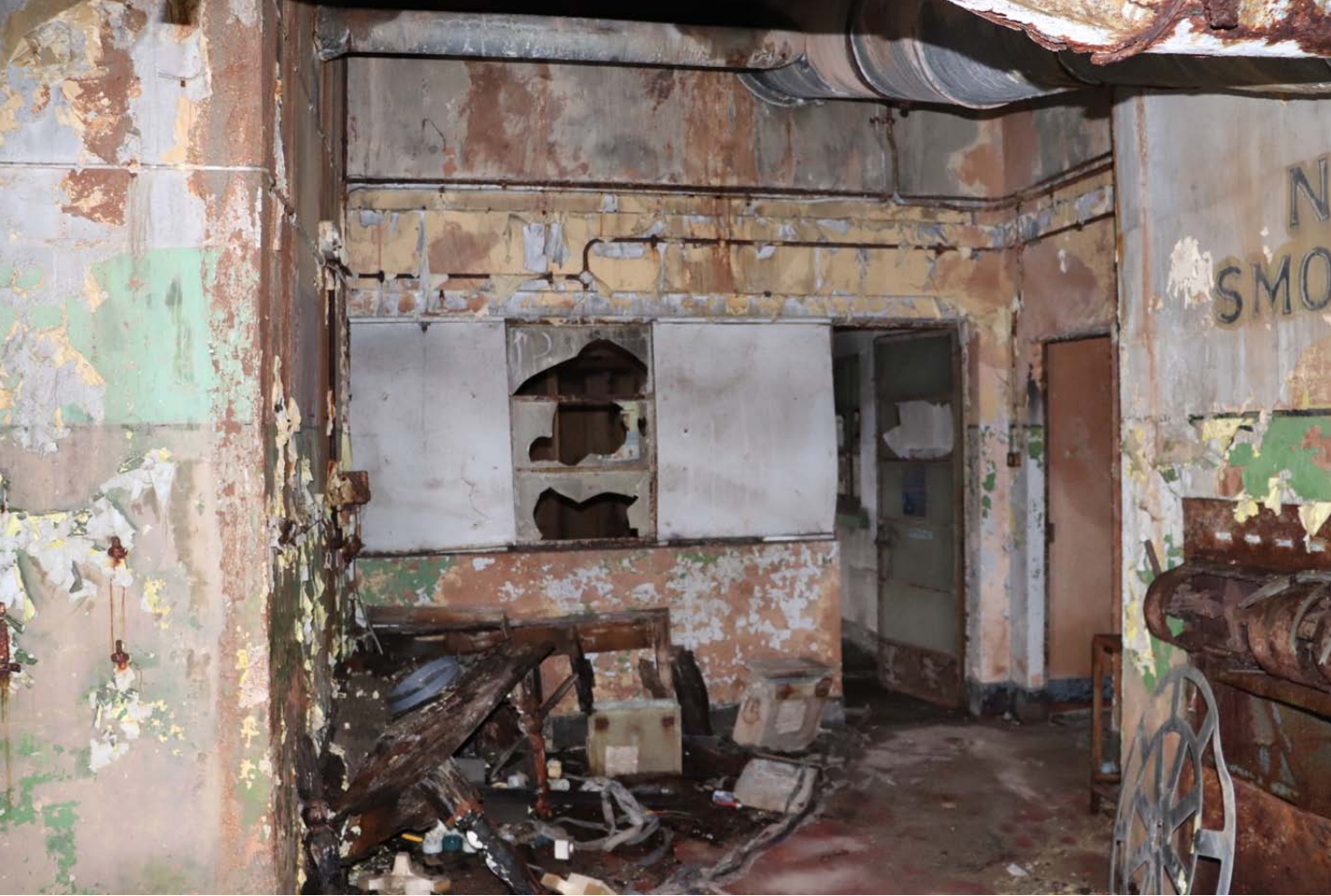
View of south wall
