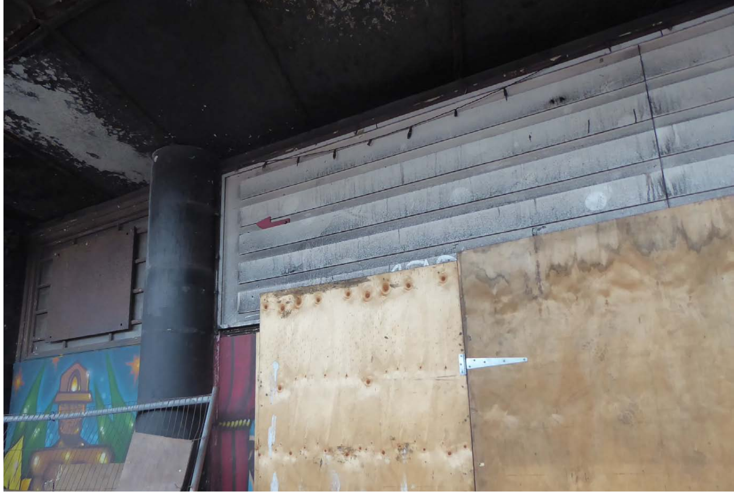
View of left hand side of louvres & overhead panel over the top of the bank of main entrance doors & screen
