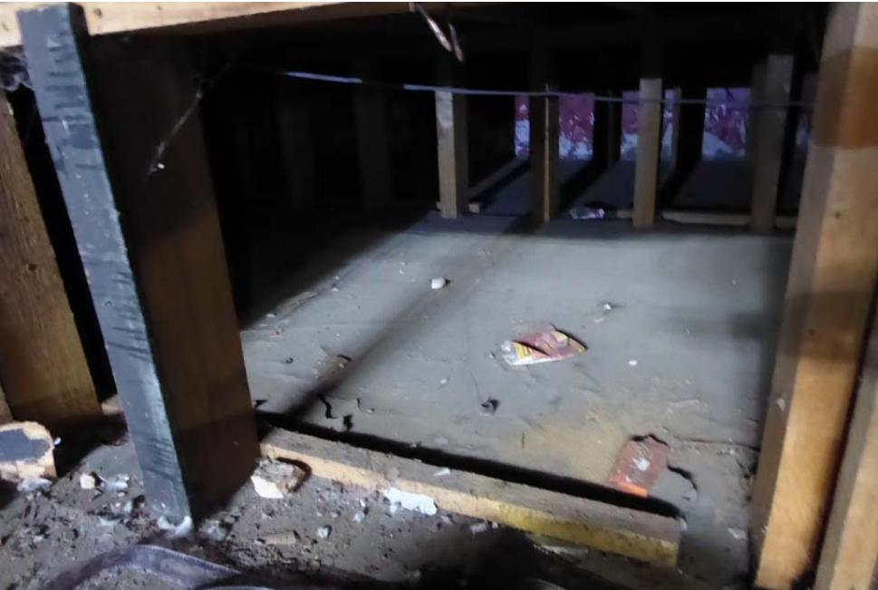
View of underside construction of timber stage
