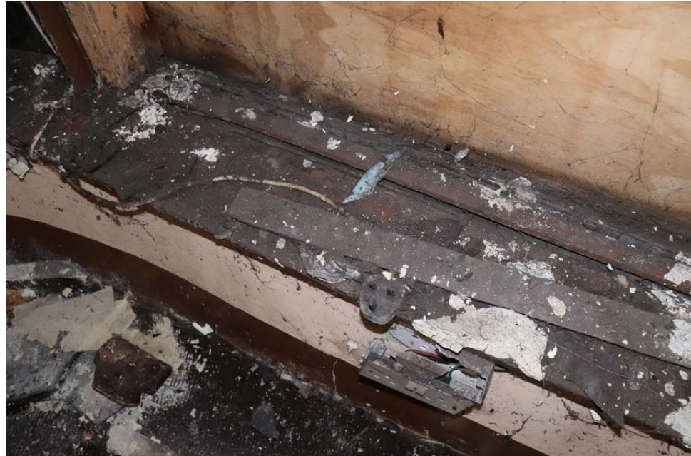
View of Timber Cill to Glazing
