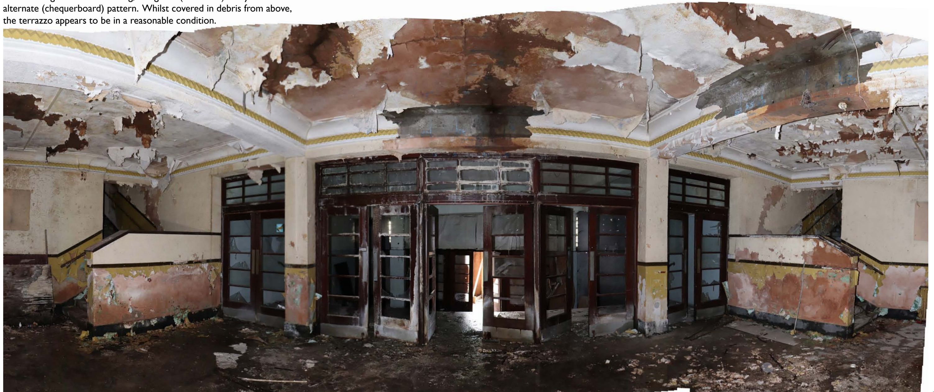
View of the Foyer looking towards the bank of doors to the south with the inner lobby beyond
