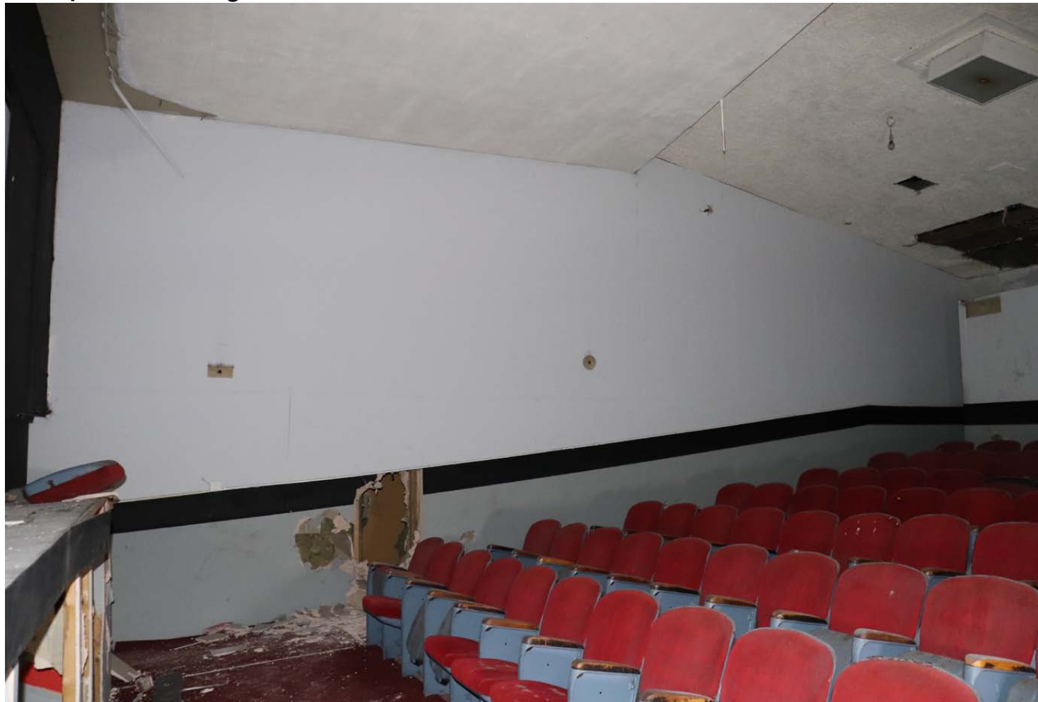
View of Cinema looking east
