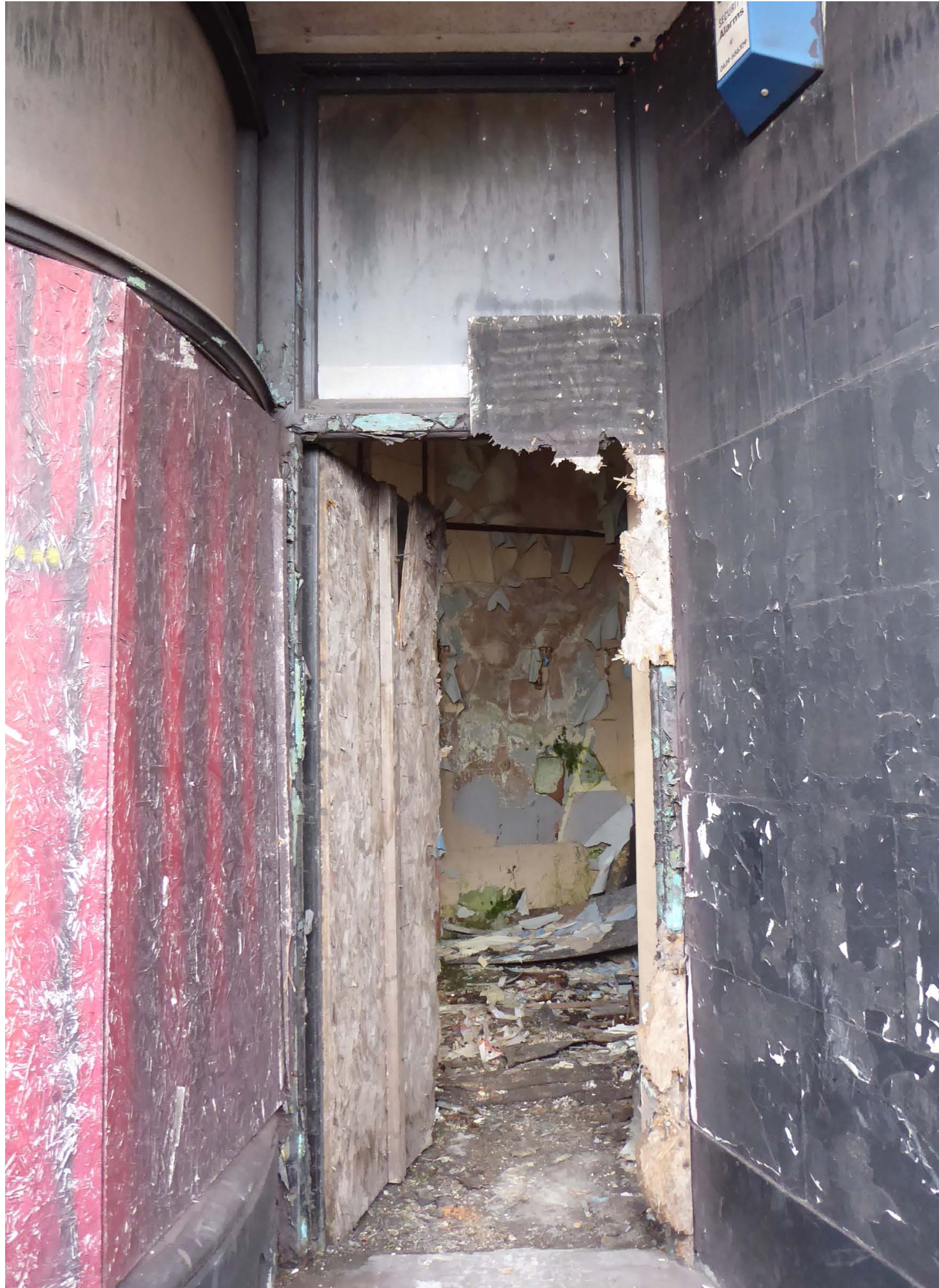
View of glazed door and overpanel to single door to left hand (smaller) retail unit
