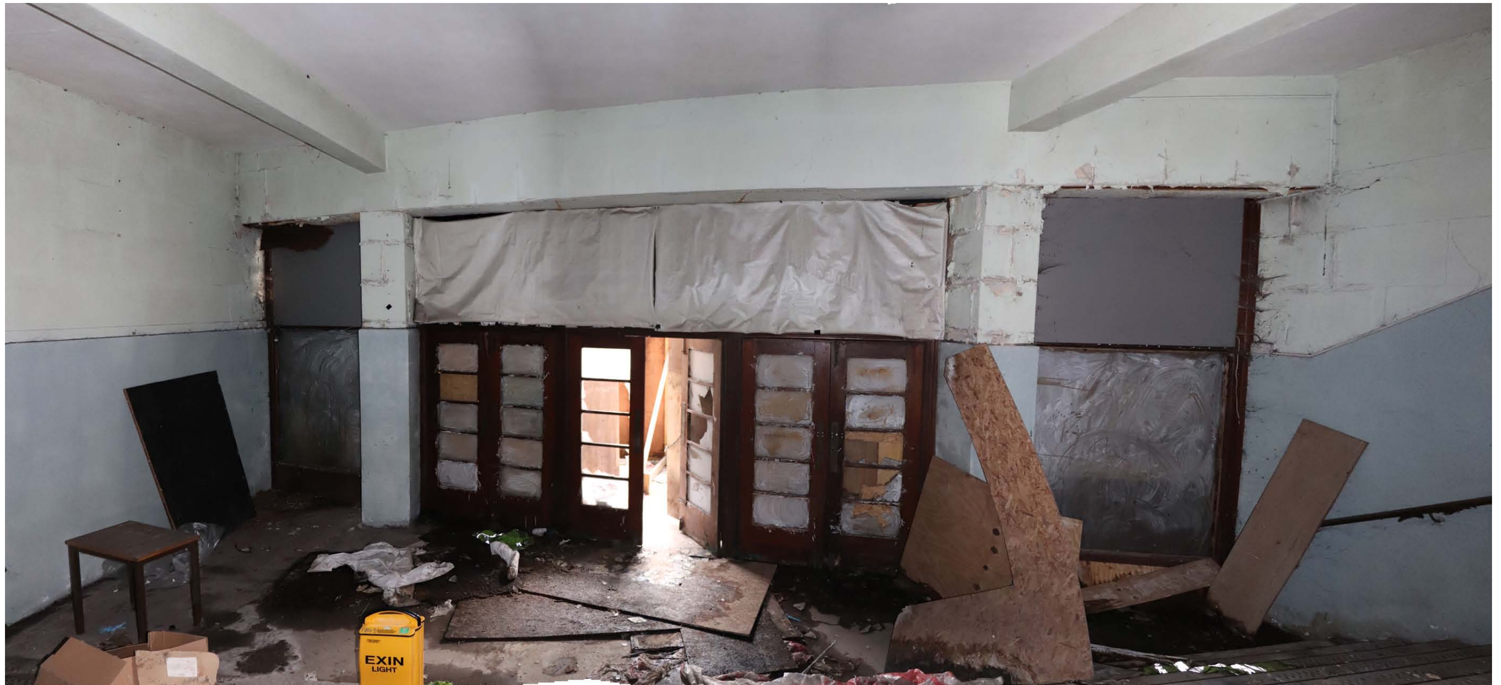
View, from top of steps, of bank of Timber-Framed Glazed Entrance Doors with 3no. sets of double doors in centre, between the 2no. columns, and a wide timber-framed glazed screen to each side of the columns
