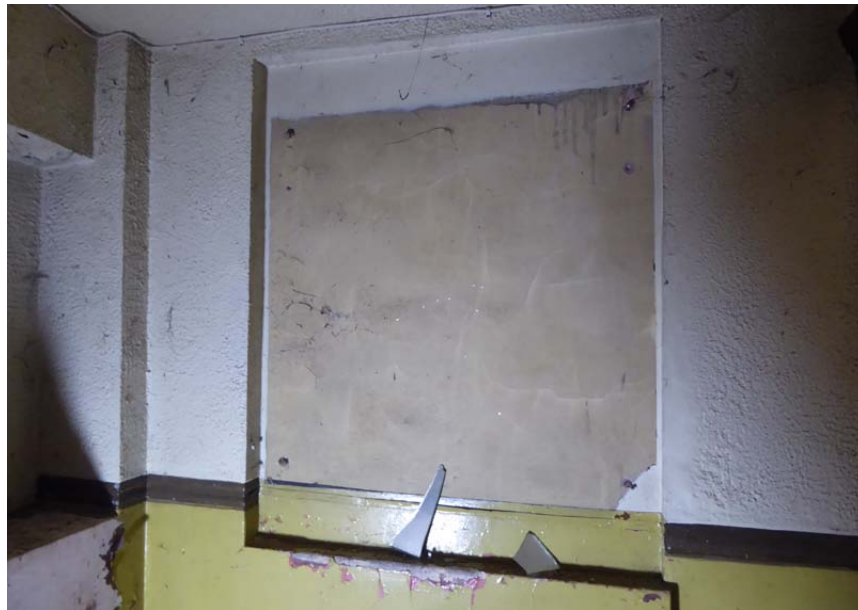
View of blocked up opening to stair landing
