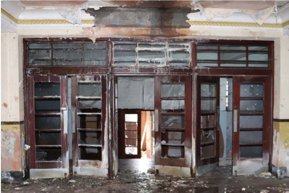
View of central bank of 3no. sets of doors
