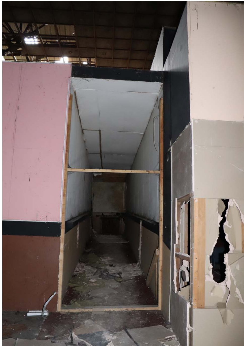
View of central Corridor as seen from main Auditorium space
