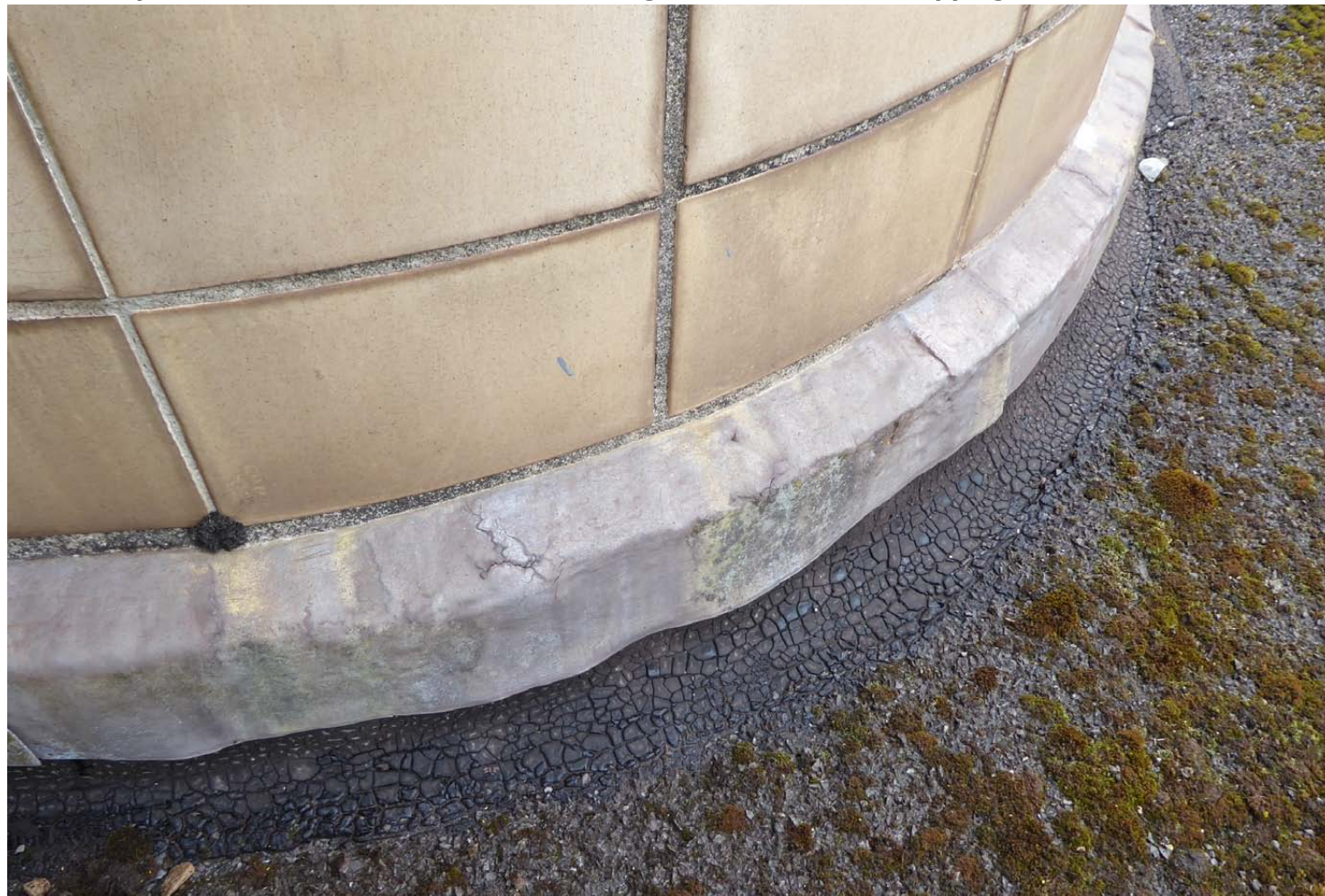
View of the base of the faience tiling to the asphalt roof to the canopy with a lead dressing
