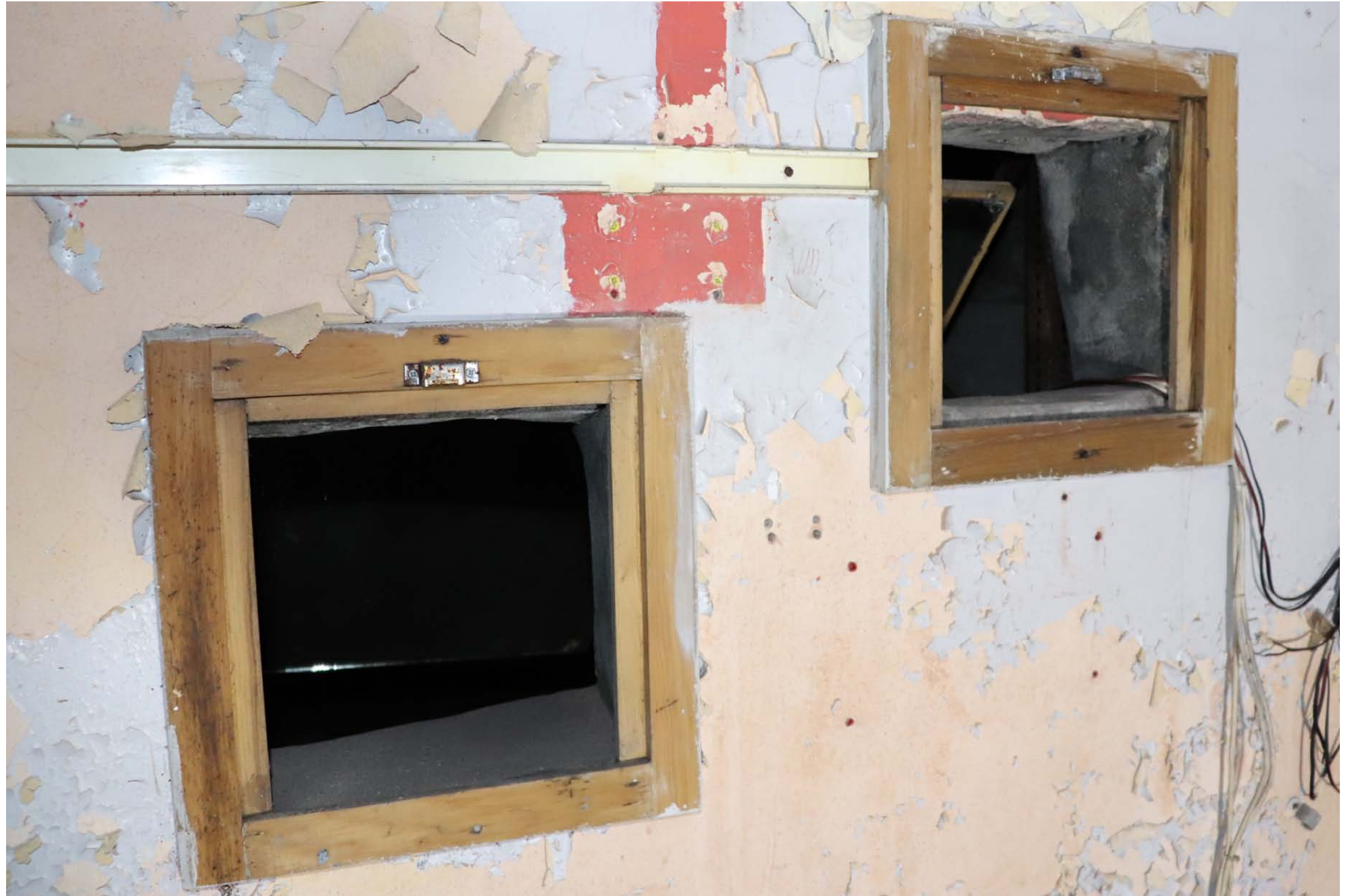
View of the 2no. projection windows in the north wall
