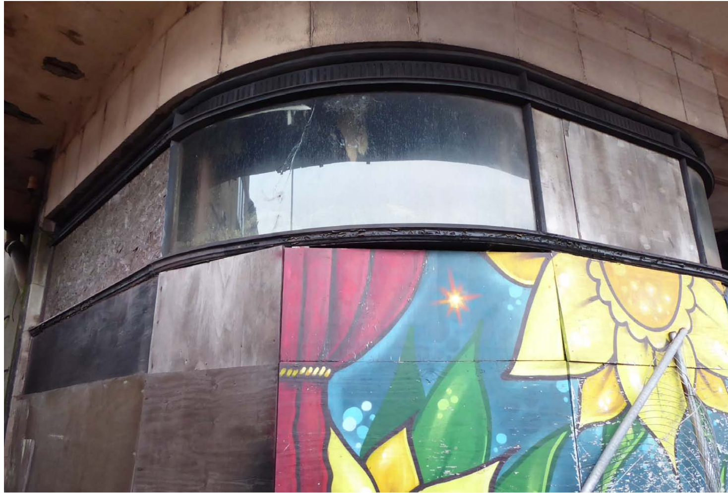
Views of top of curved frontage to timber-framed glazing to the smaller (left-hand) Retail unit, showing curved glass to corners & straight glass to ends and sides, with middle sections boarded up due to loss of glass
