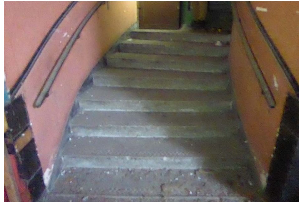
View of the Steps leading up to the final exit doors
