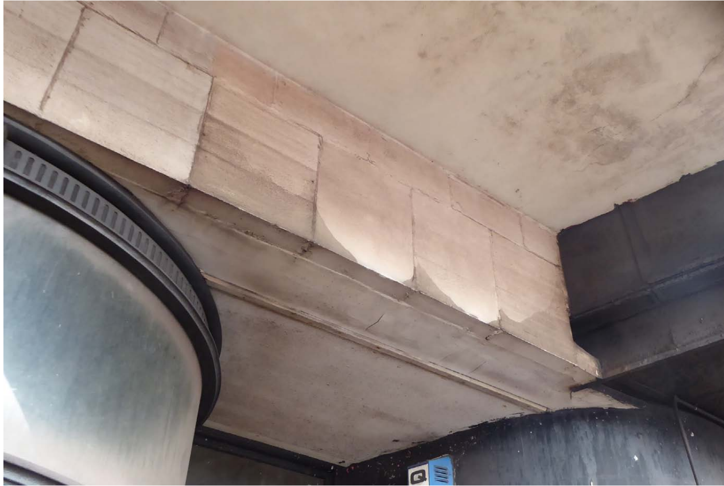
View of head of glazed overpanel to door to left hand (larger) retail unit with faience facing
