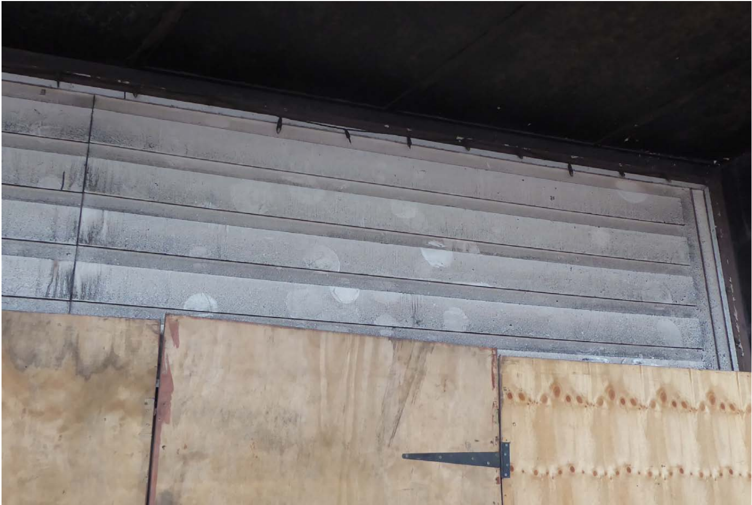
View of louvres over the top of the bank of main entrance timber doors
