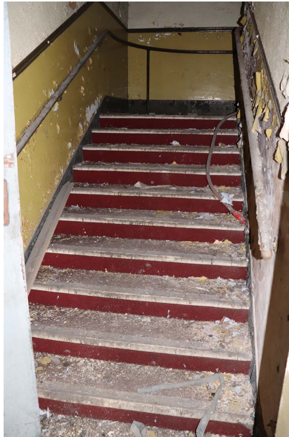
View of lower flight of stair looking up
