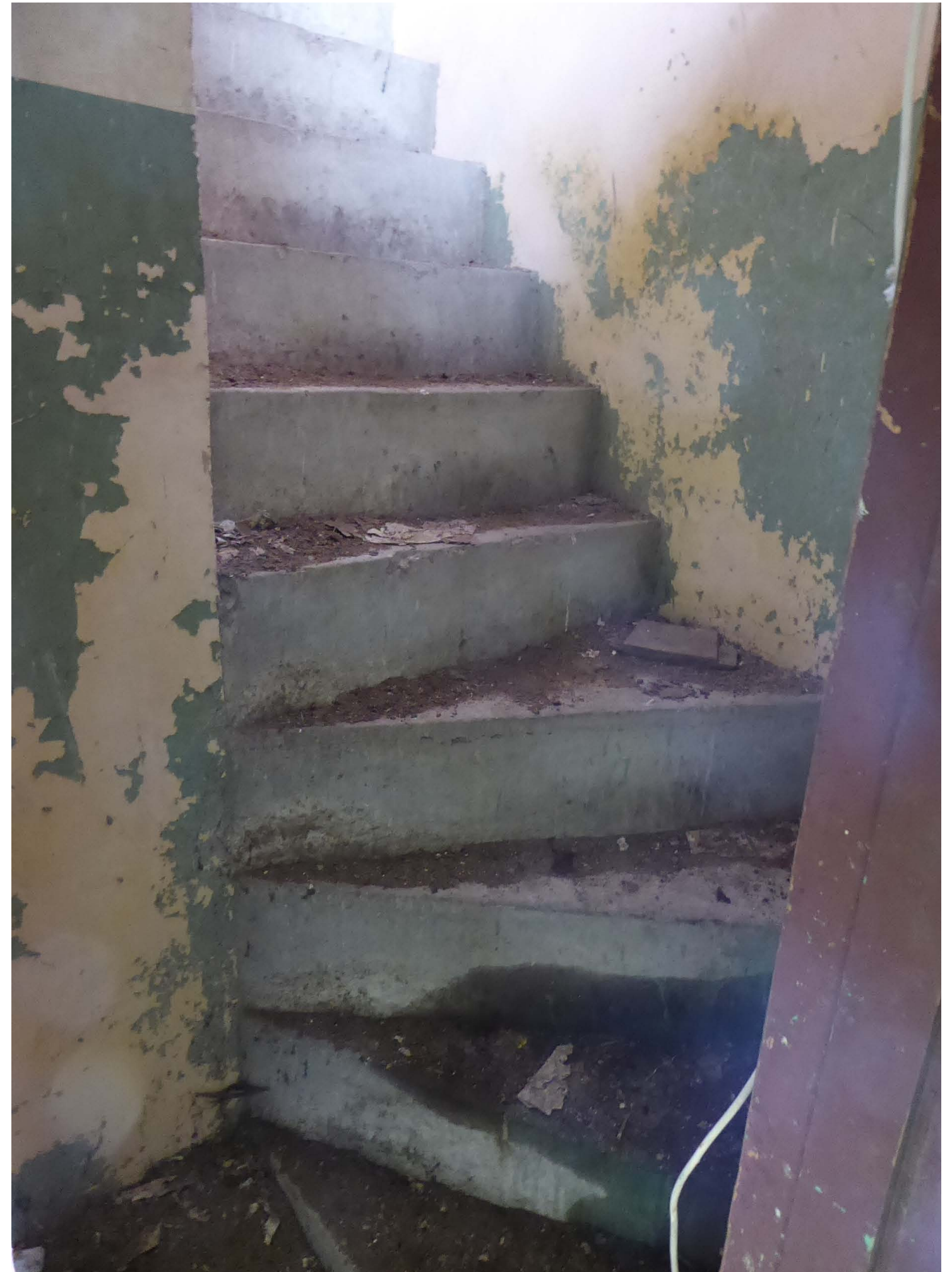
View of spiral concrete staircase leading from first floor to second floor
