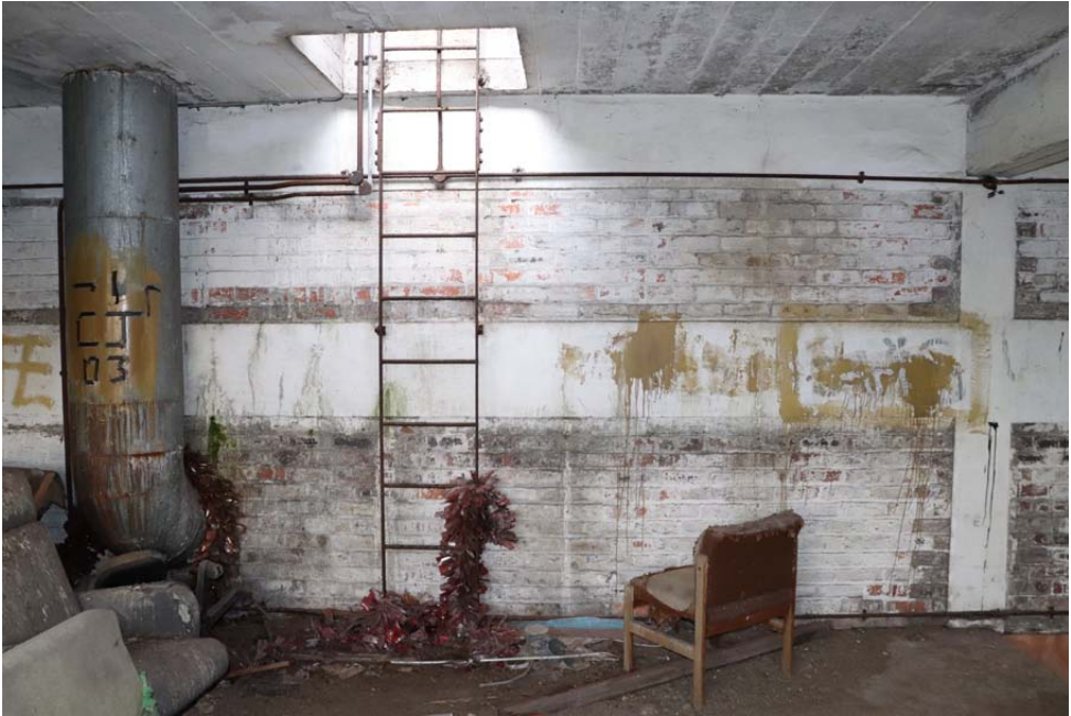
View of steel ladder to access roof & galvanised steel duct
