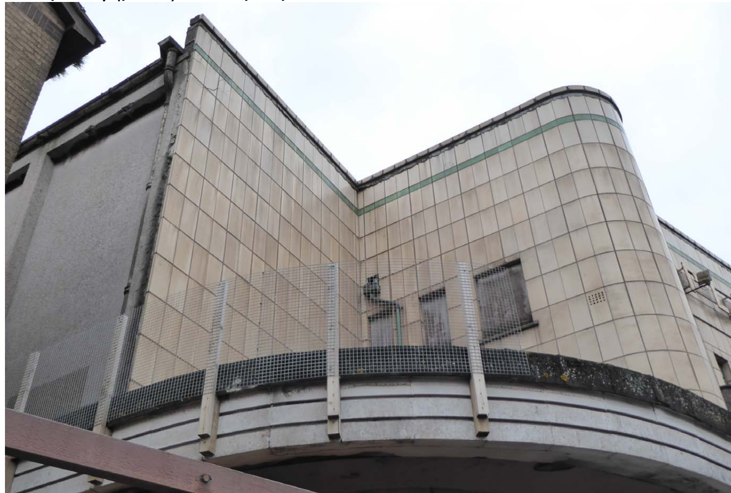
View of the left hand side (faience) section of the front elevation
