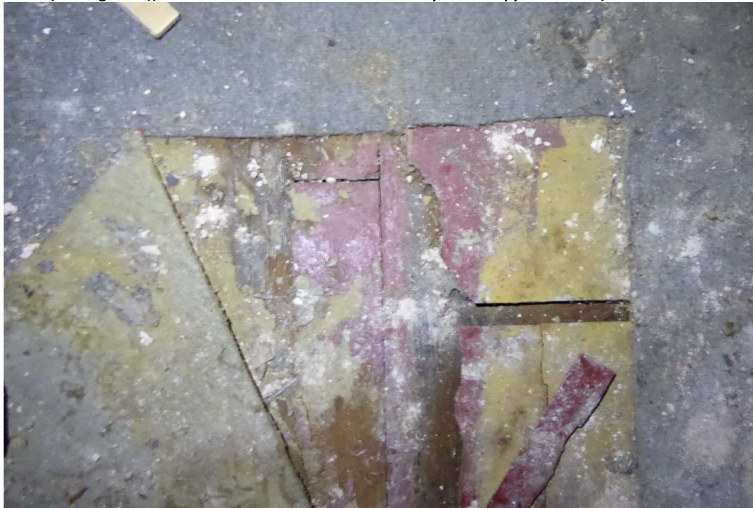
View of timber flooring with linoleum floor covering and then carpeting on top
