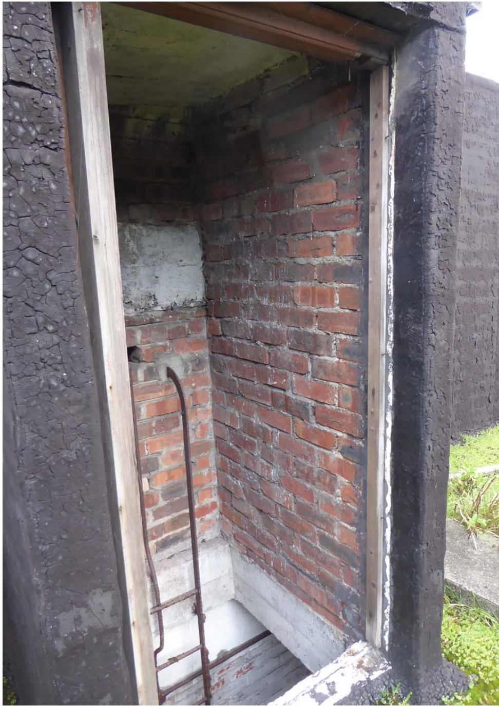
View of interior of box construction to ladder access
