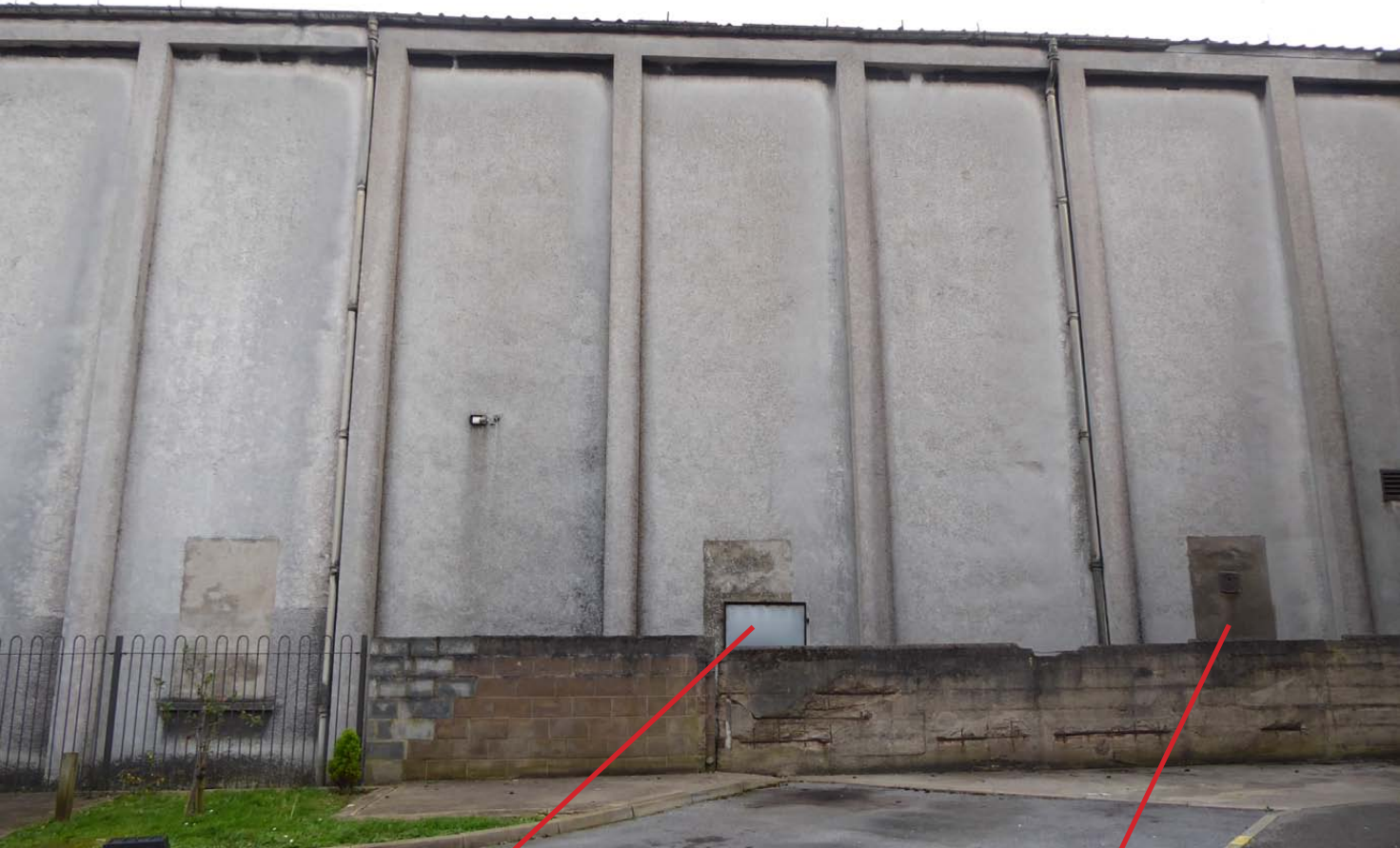
View of the blocked & boarded up windows and exit door to the central section of the west side elevation
