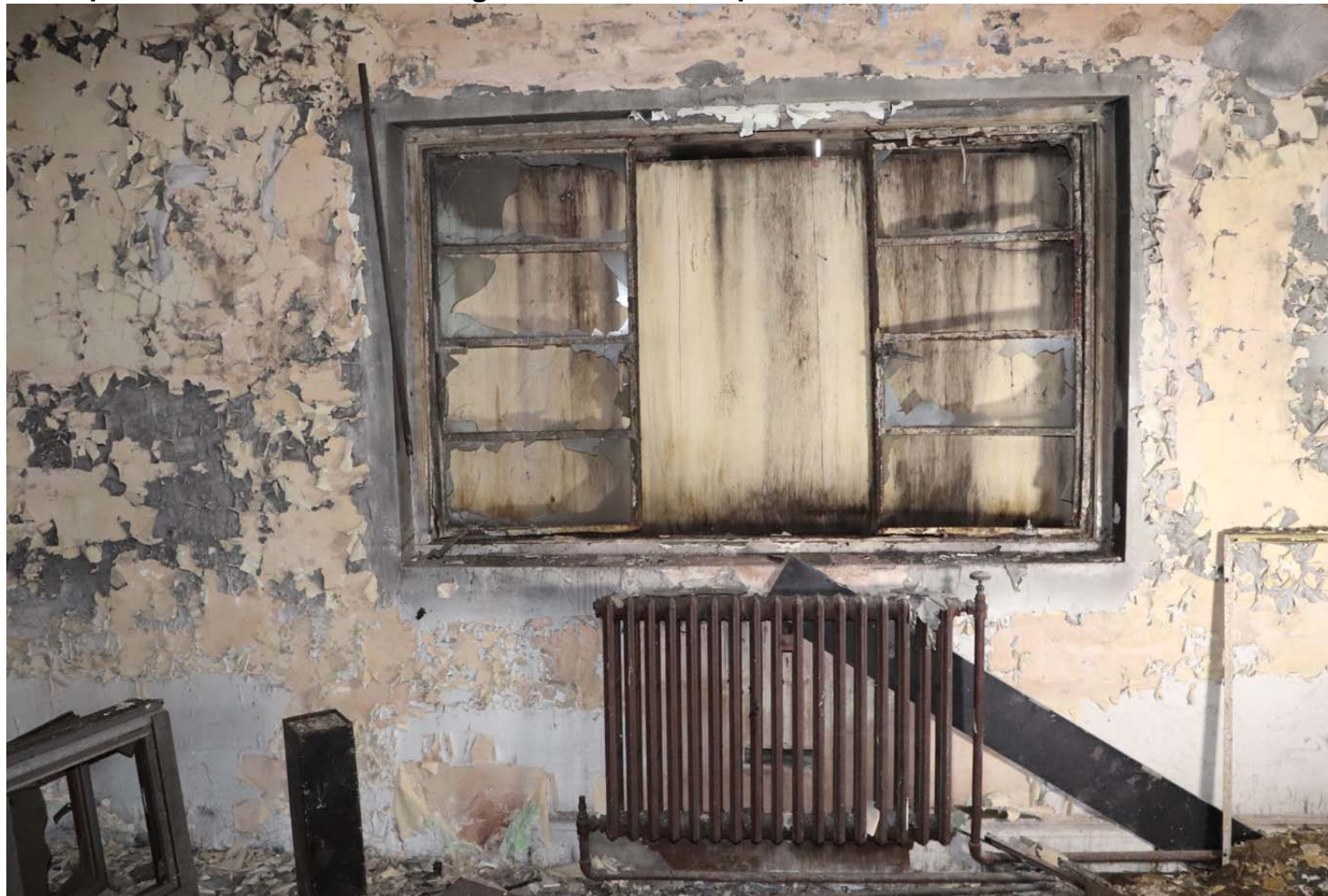
View of west wall with window to the exterior
