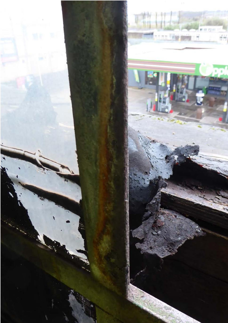
View of example of mullion to transom joint to windows
