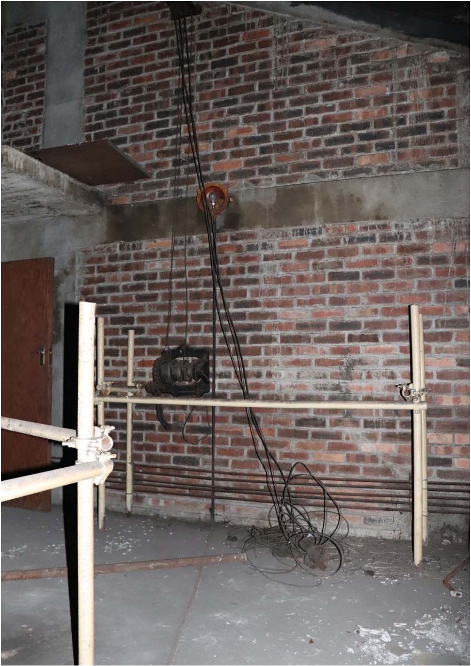
View of brickwork within concrete frame to raised section
