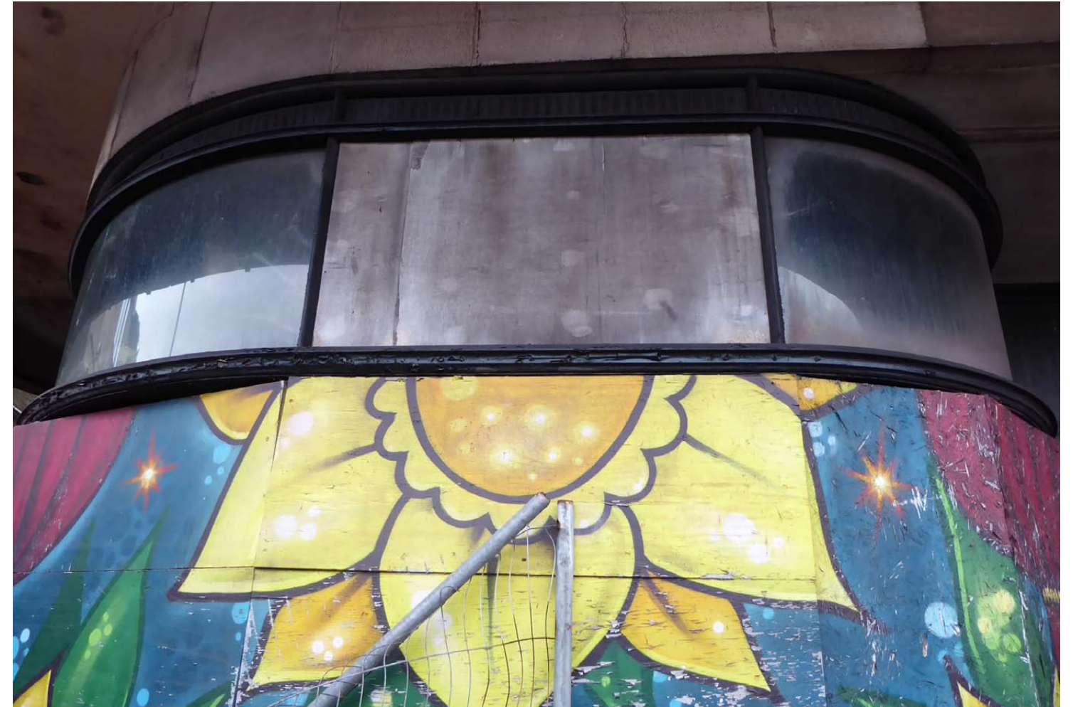
Views of top of curved frontage to timber-framed glazing to the smaller (left-hand) Retail unit, showing curved glass to corners & straight glass to ends and sides, with middle sections boarded up due to loss of glass
