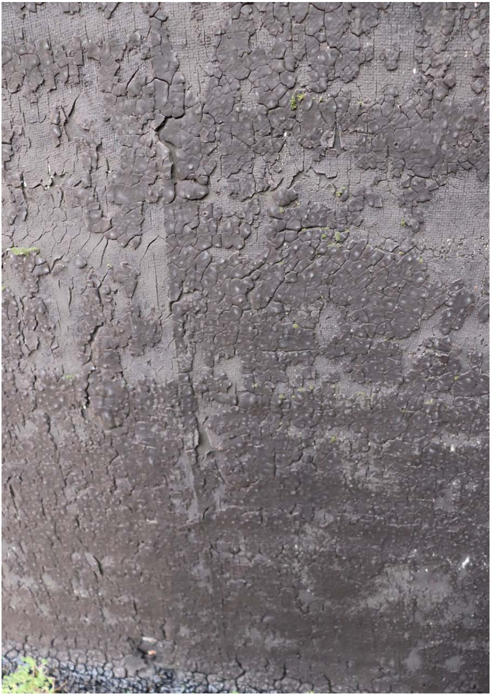
View of the bitumen coating to the wall
