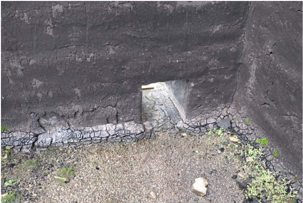
View of ne of the two drainage outlets from the roof
