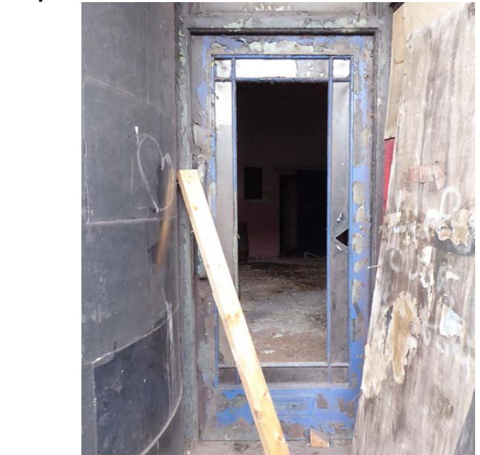
H Timber-framed Shop Doors to be Retained & Restored
