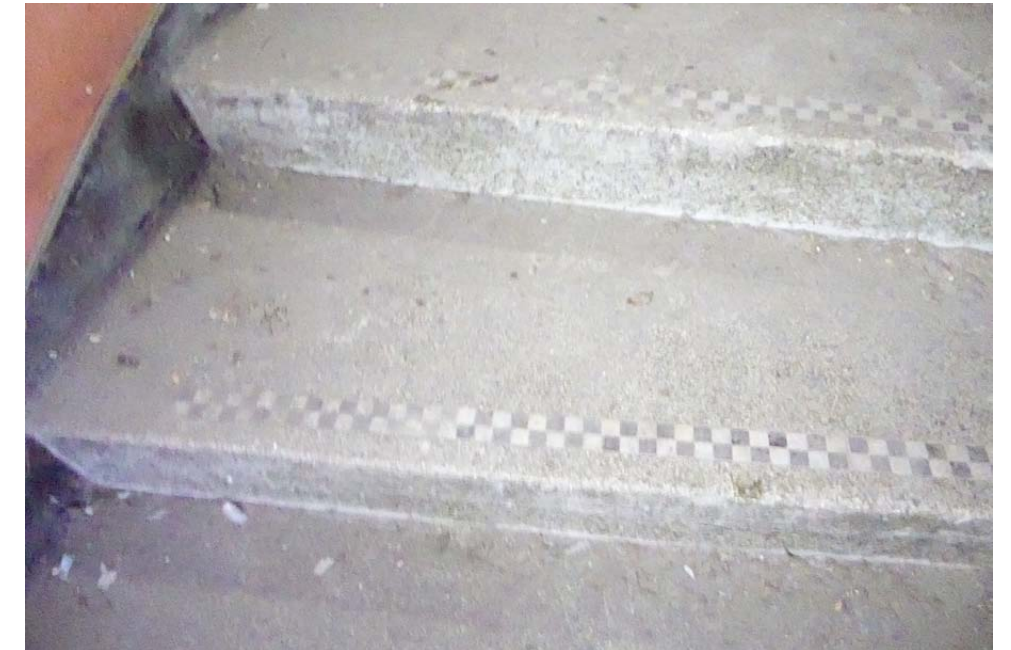
View of terrazzo steps with black & white checkerboard nosings
