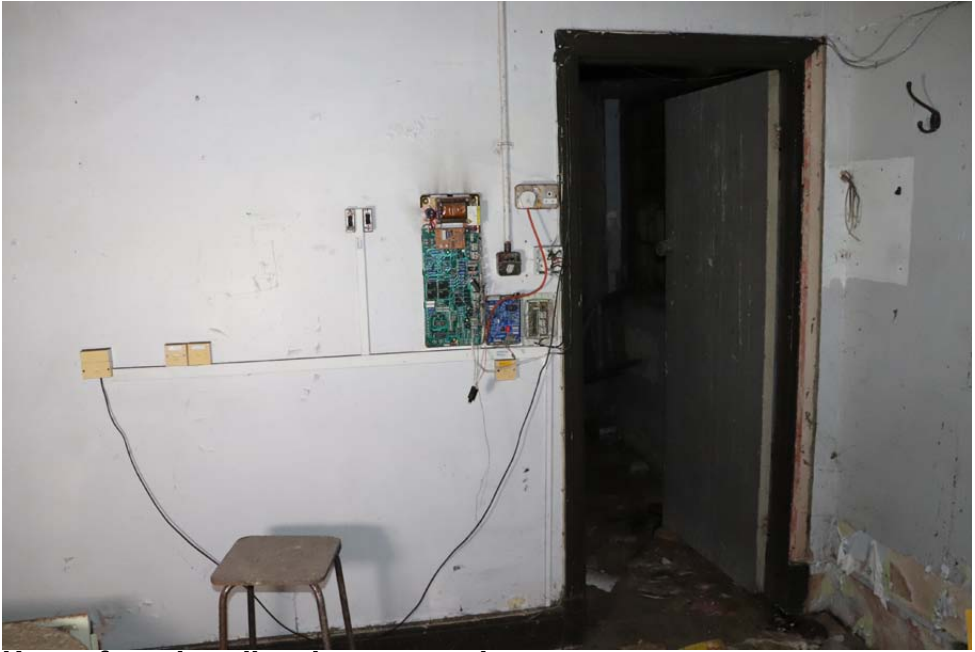
View of north wall with entrance door
