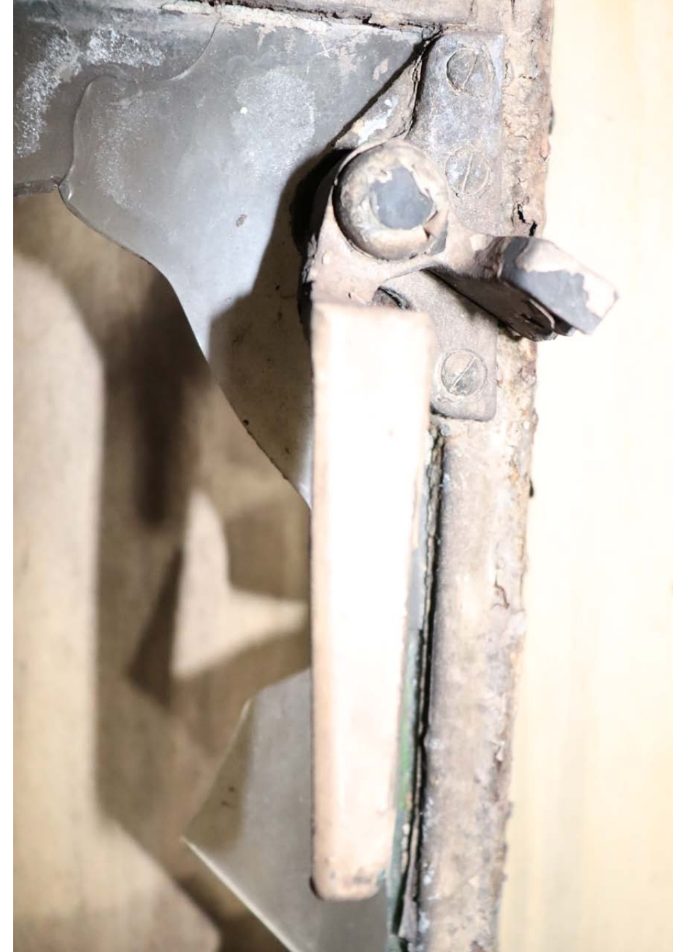
View of two-point cockscur fastener
