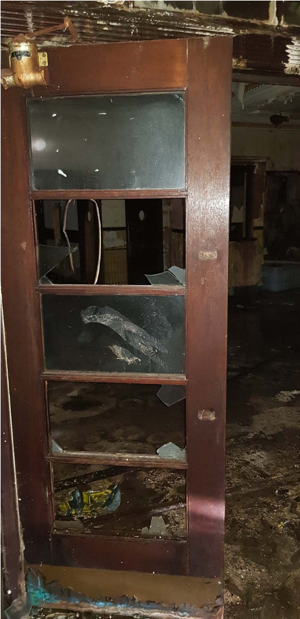
View of one leaf of doors with 5no. glazed panes & brass kickplate
