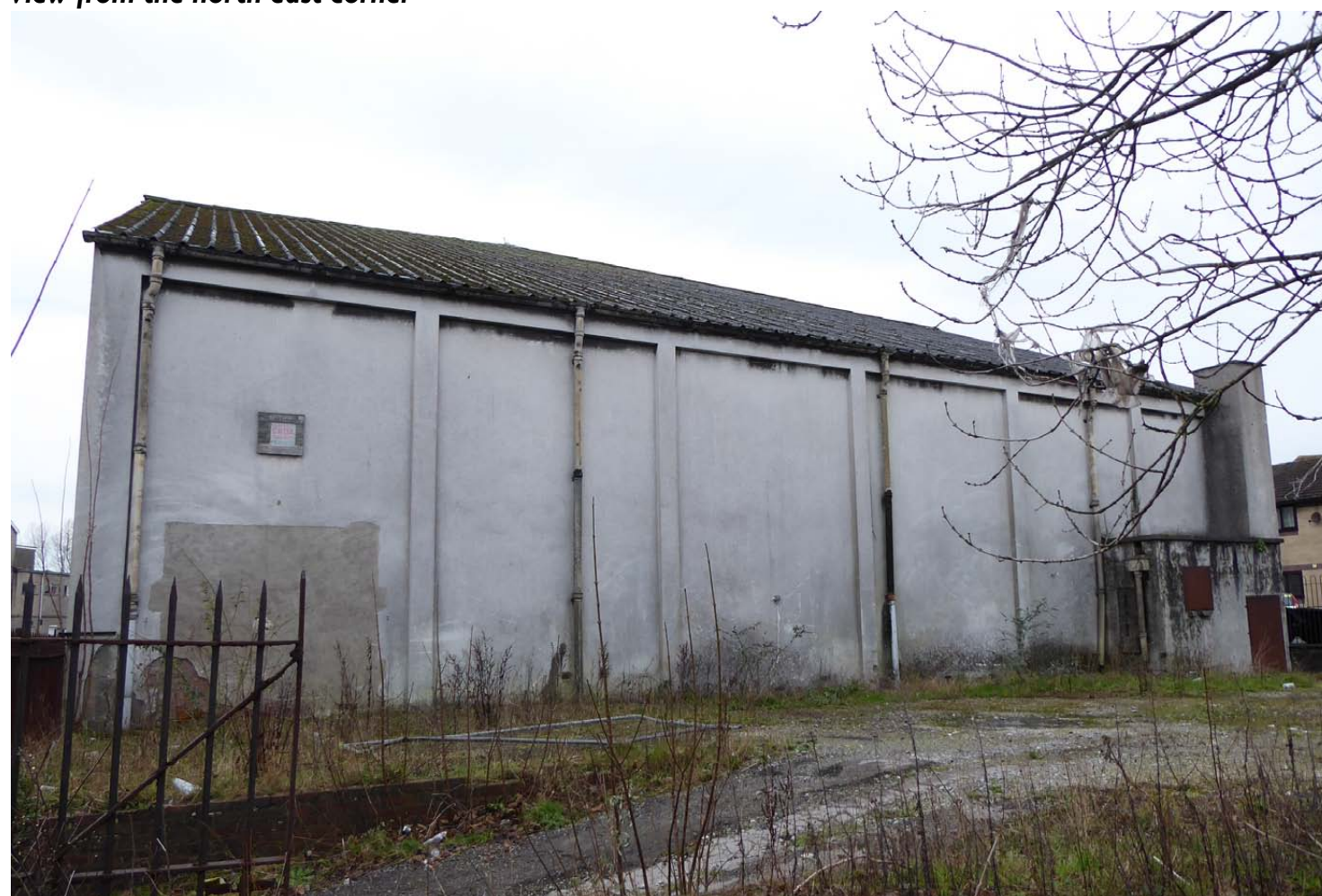
View of the rear (south) elevation
