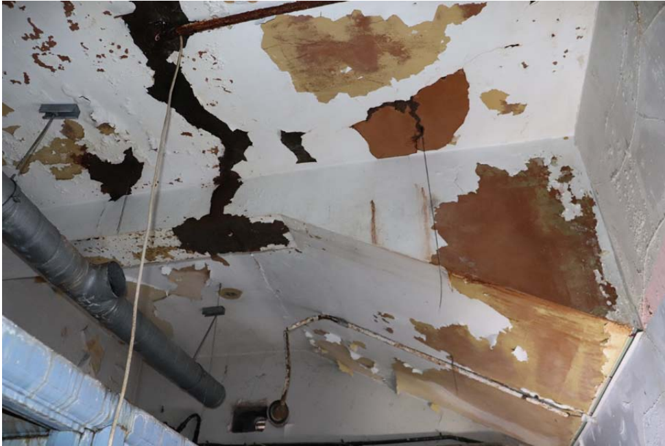
View of the sloping soffit of the staircase within the toilets
