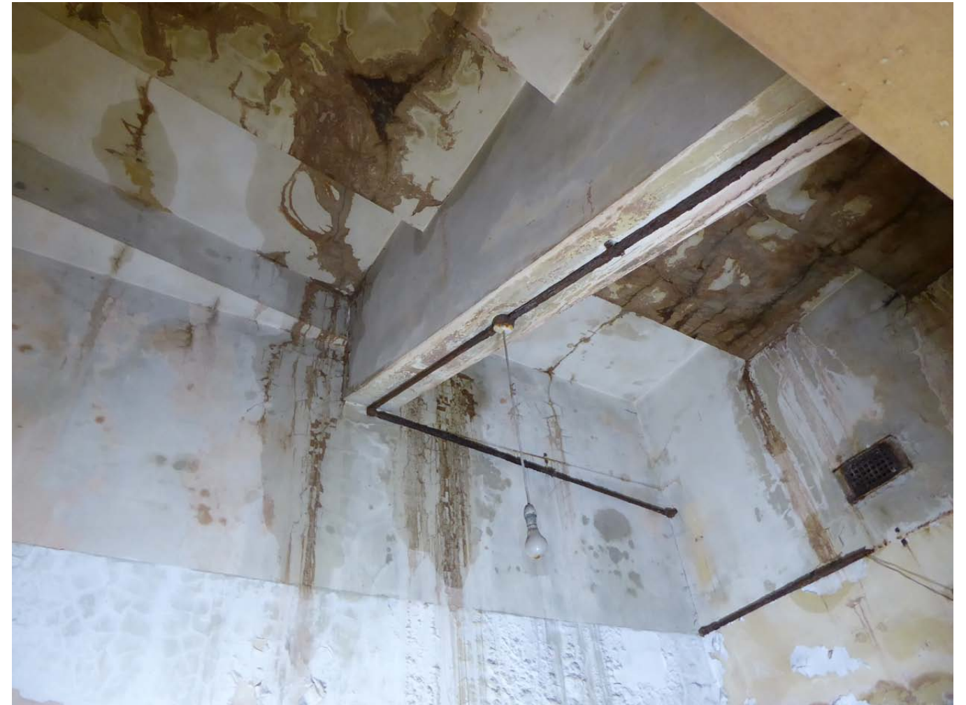
View of top of the raking concrete 'beam' with the flat concrete seating
