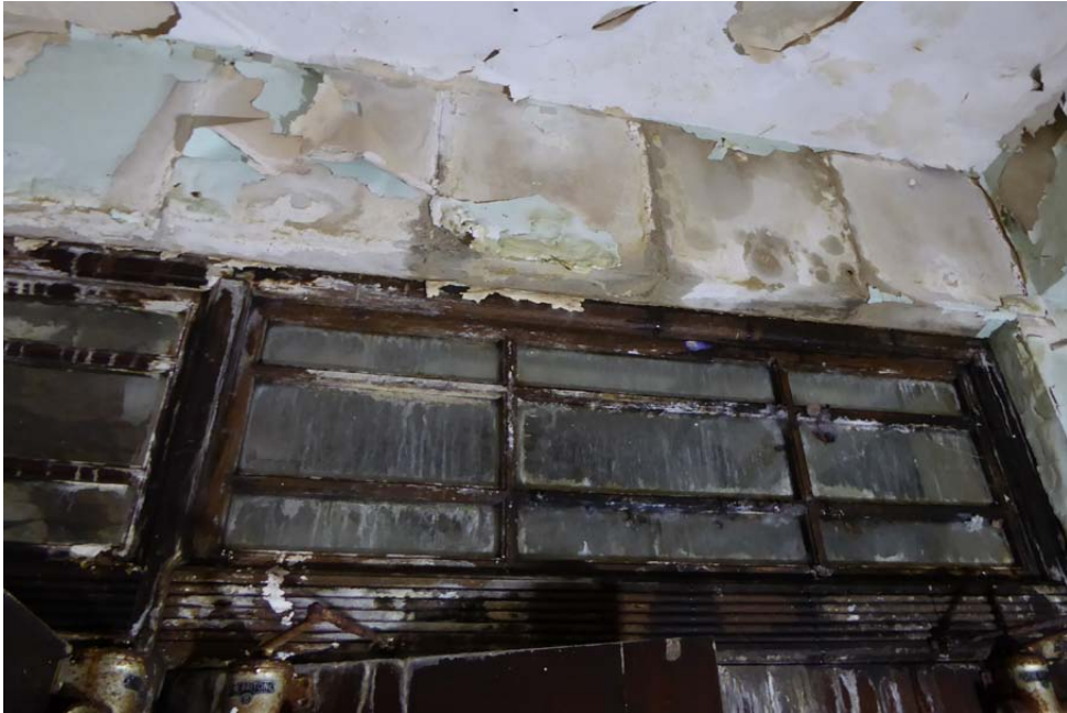
View of timber-framed glazed overpanels
