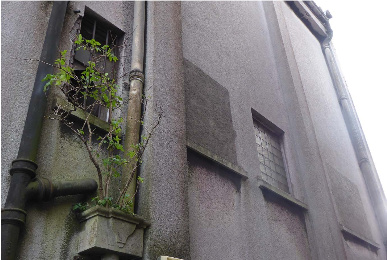
View of the windows and blocked up windows to the upper right hand side of the west side elevation
