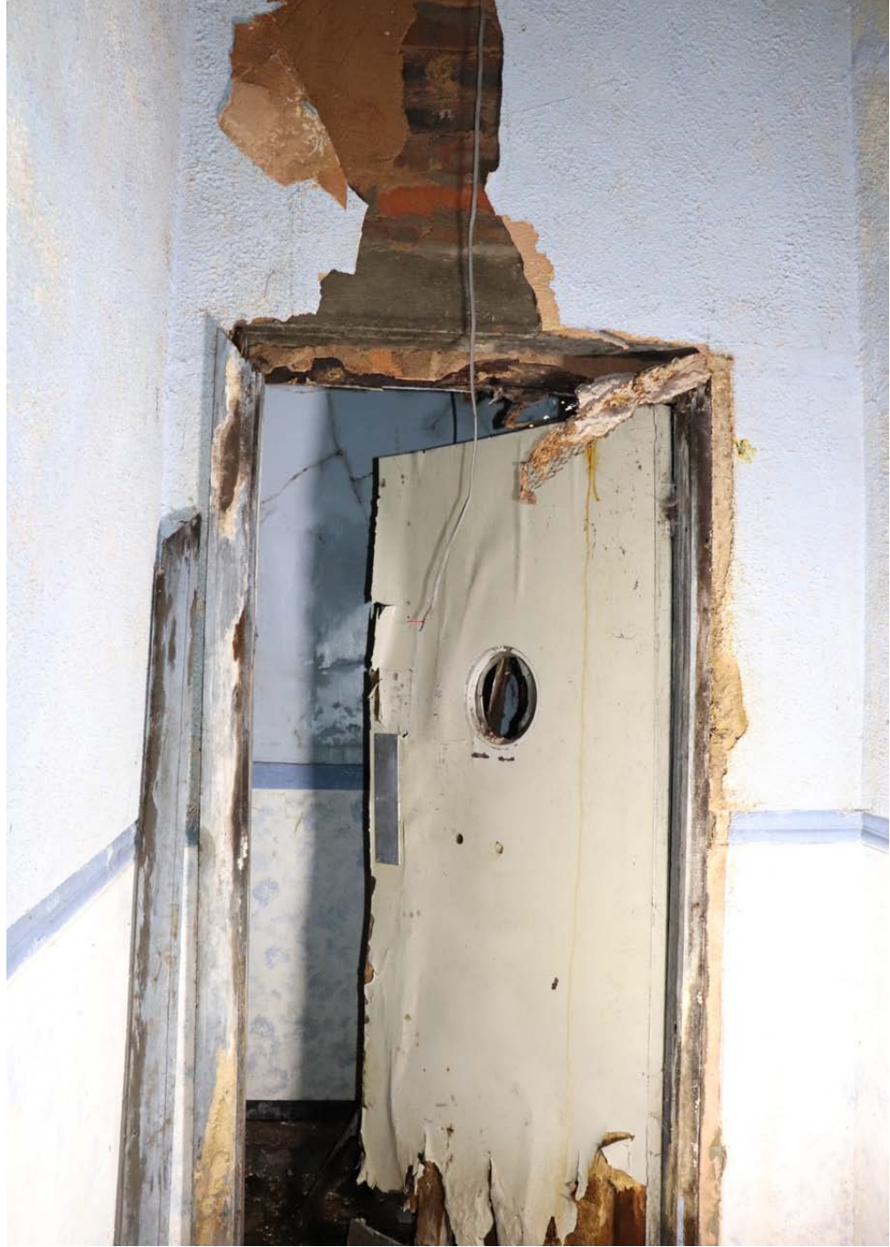
View of the door to the toilets from within the lobby
