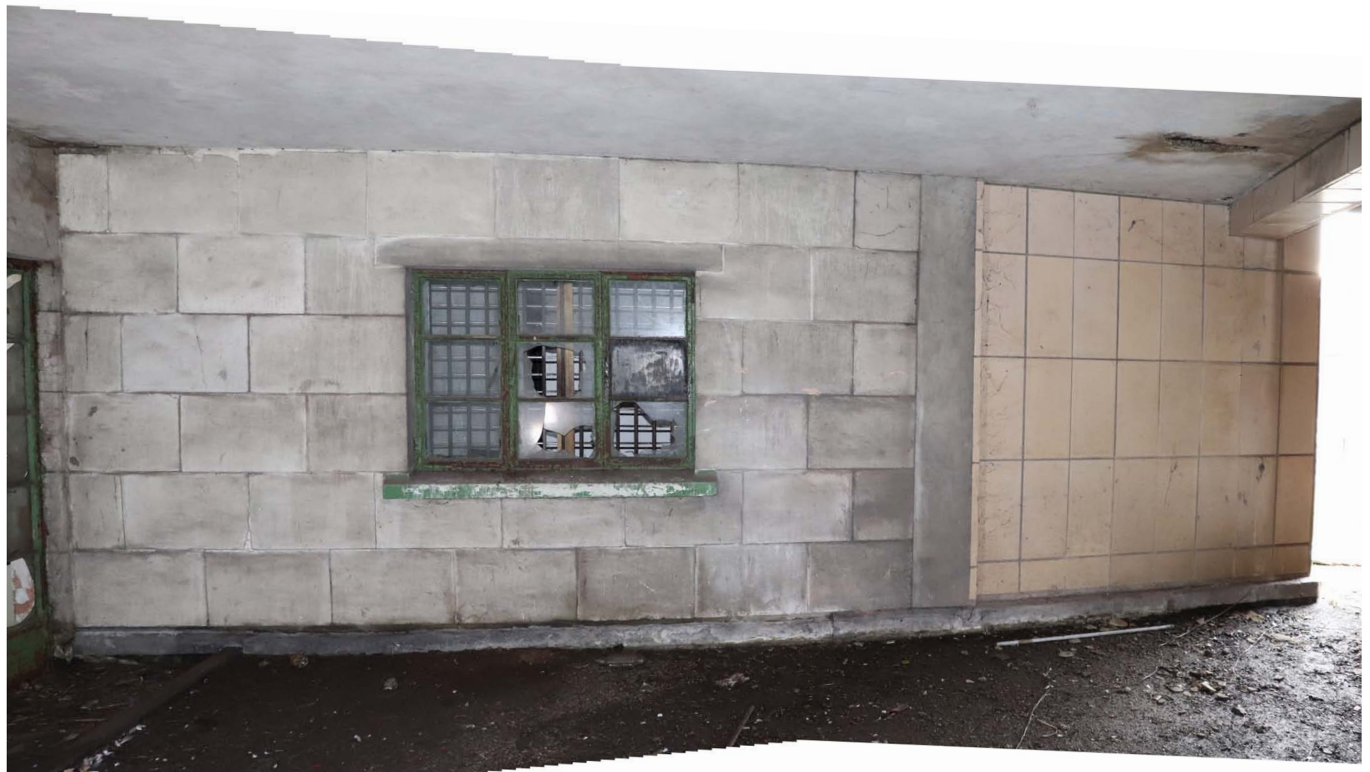
View of east elevation to open space with the masonry block facade, with its metal-framed window, leading to faience cladding
