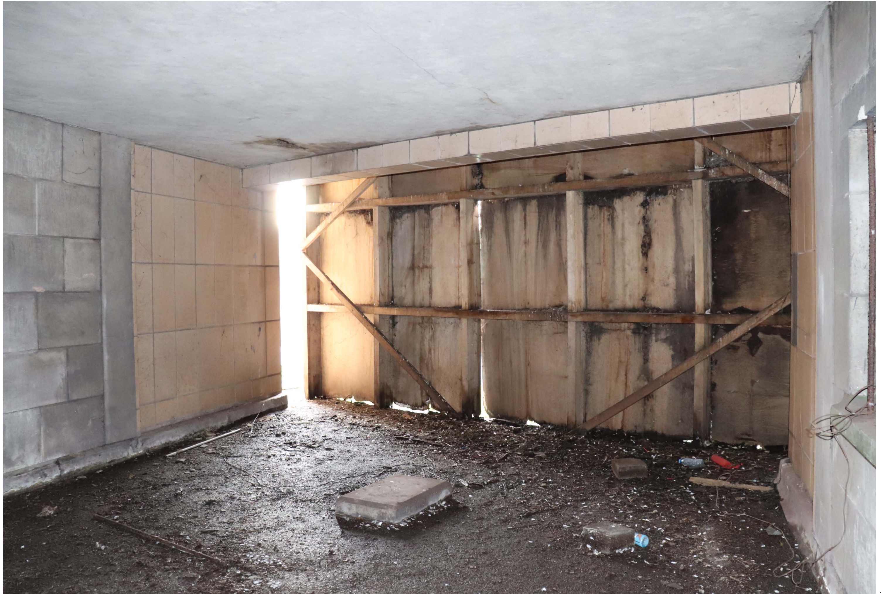
F13 - Central Roofed Recess - View looking out to large opening, now boarded up
