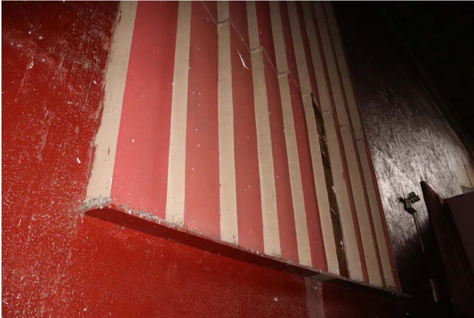
View of underside of acoustic reflector panels to either side of stage
