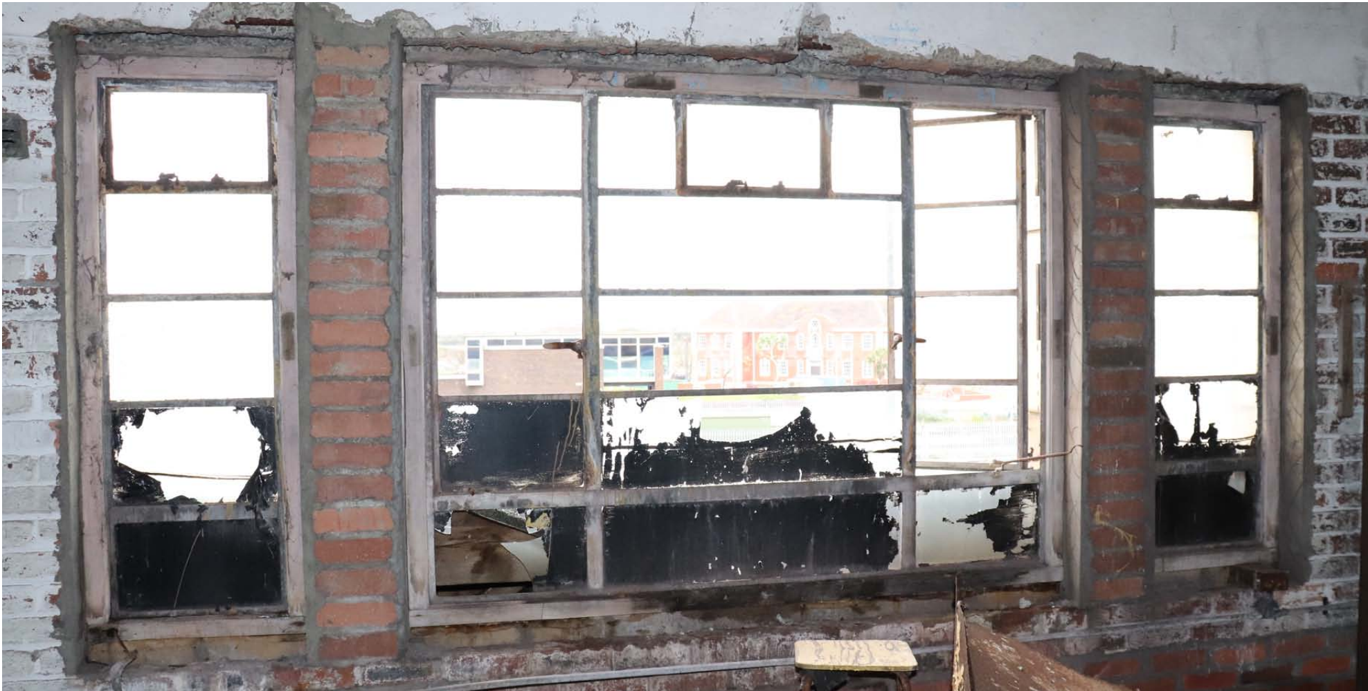
View of the large tripartite windows to the centre of the south elevation
