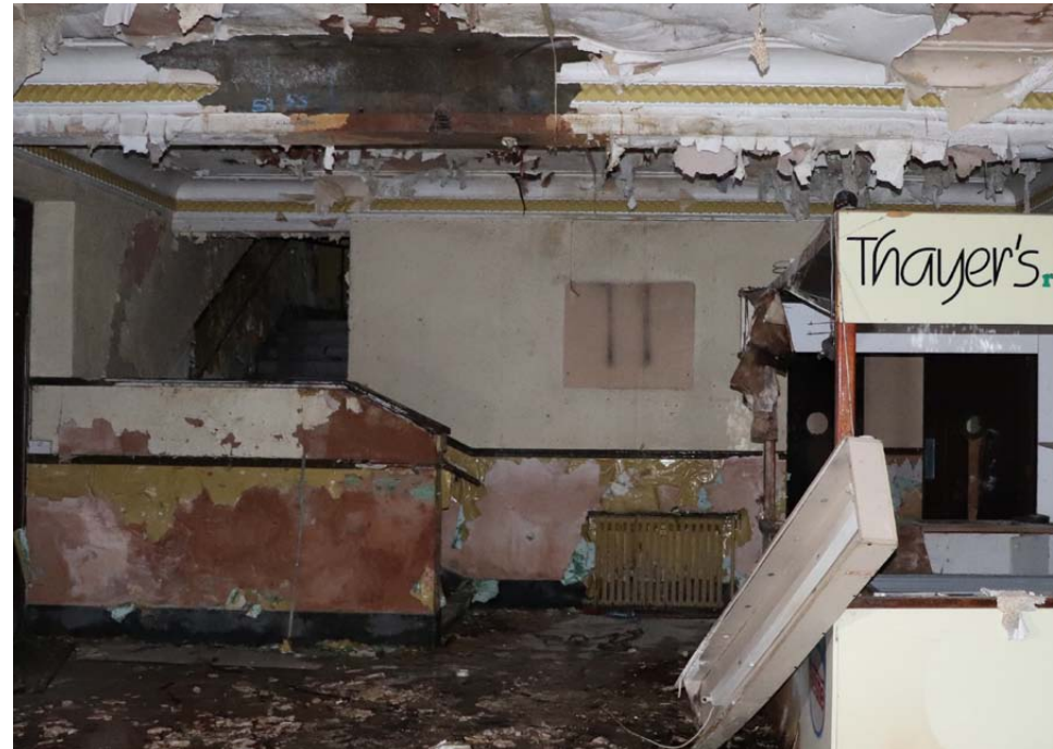
View of the Foyer looking towards the west staircase and toilets
