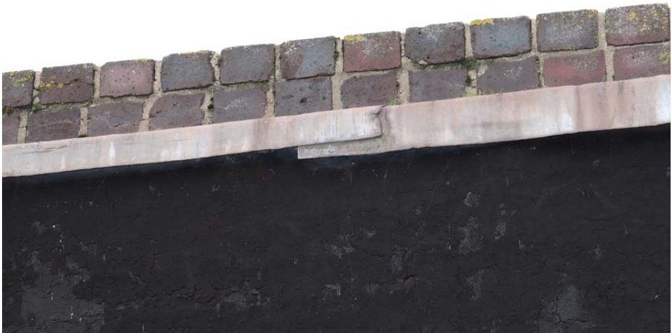
View of top of walls with two brick courses over a lead flashing
