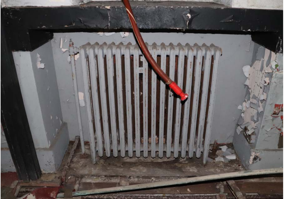
View of cast iron radiator at rear of space
