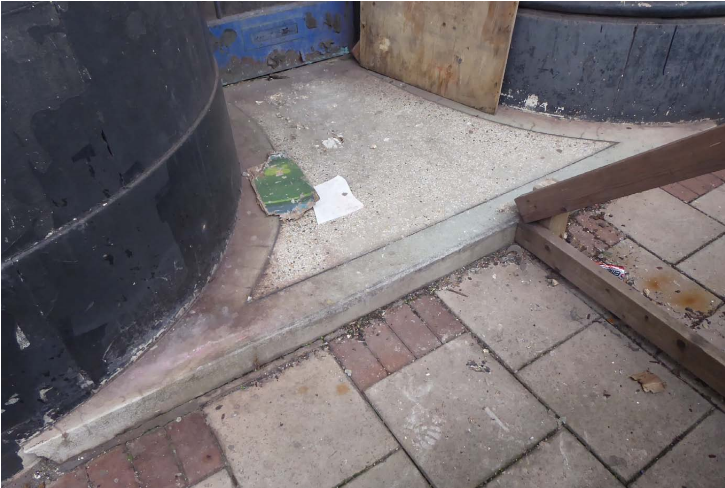
View of terrazzo threshold to right hand (larger) retail unit
