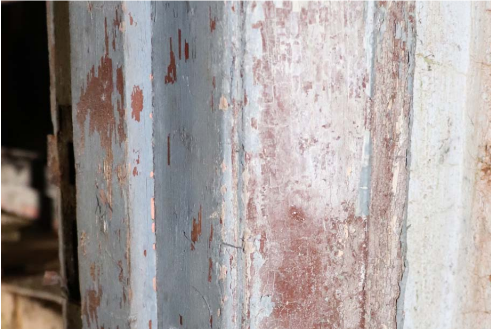
View of profile of architrave to doors in the space
