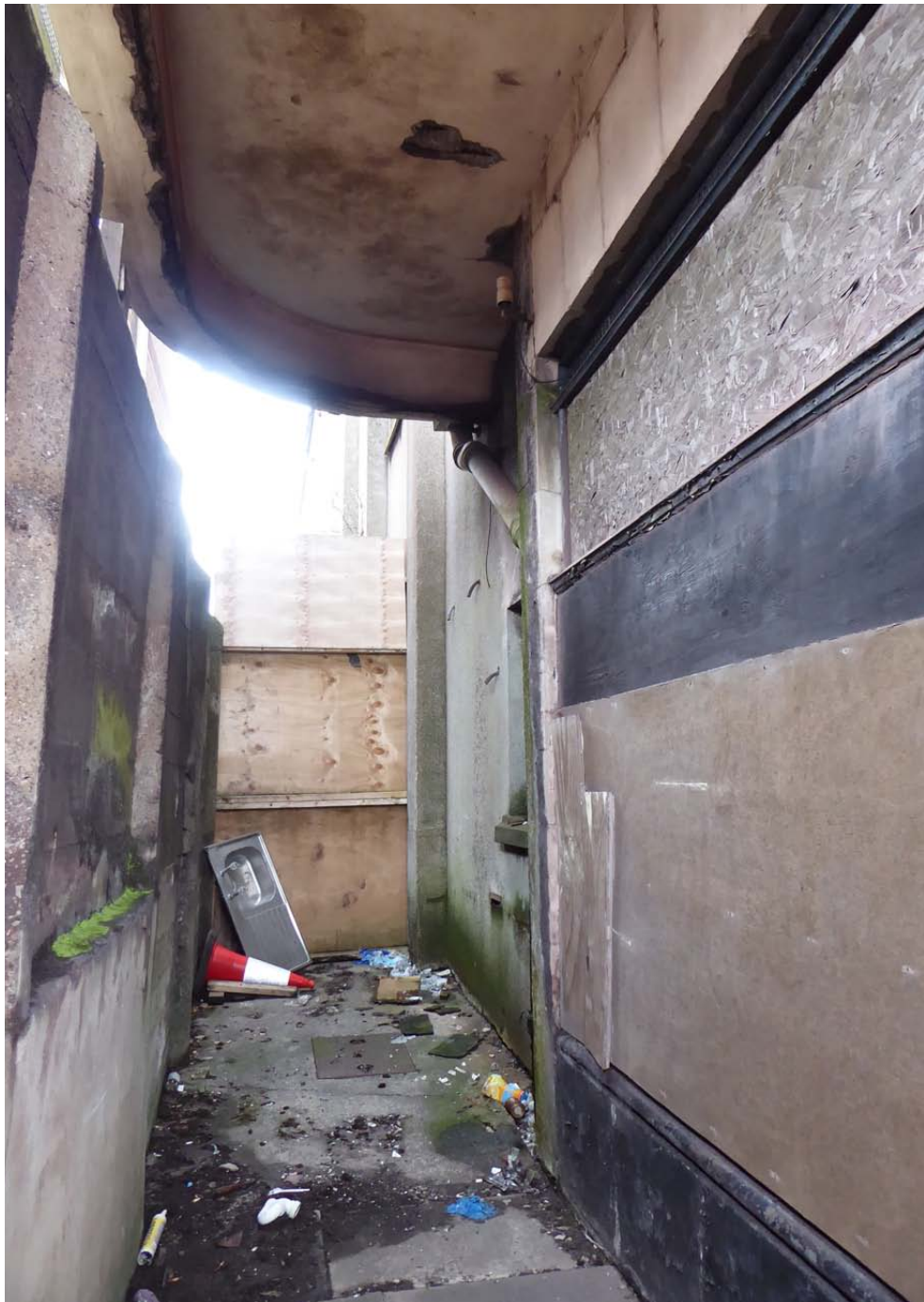
View of the west side of the frontage with the Retail unit to the right
