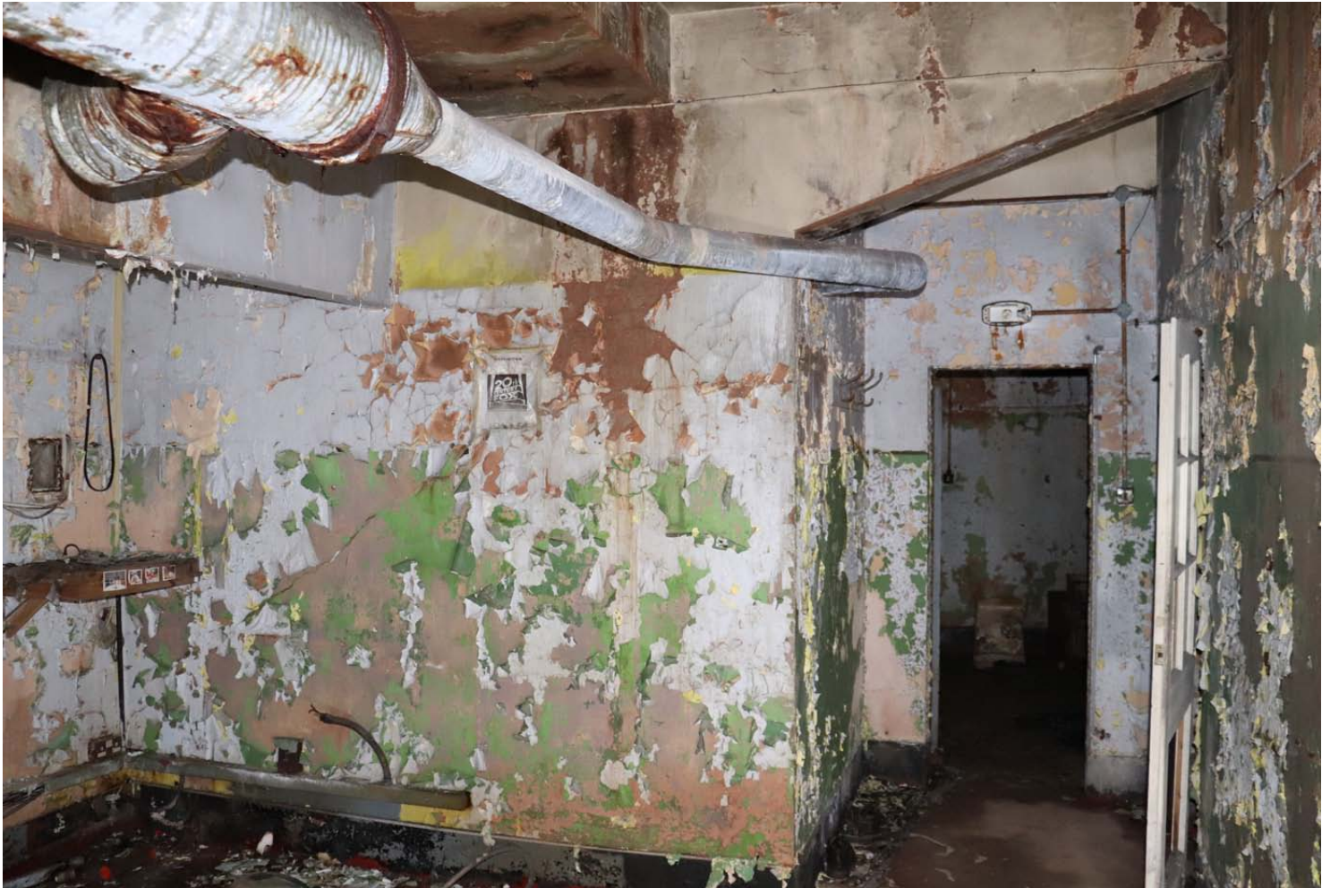
View of east wall
