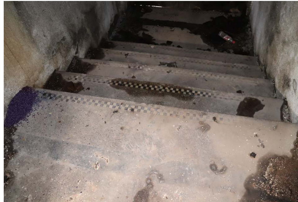
View of terrazzo steps with black and white chequerboard nosings
