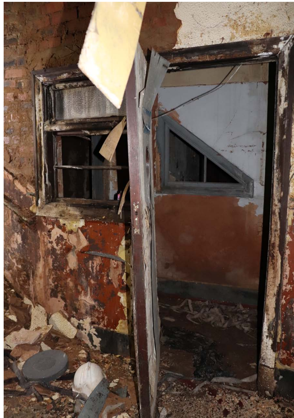
View from stair landing looking towards projection room
