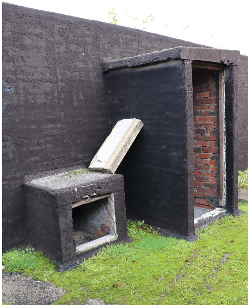
View of box construction to ladder access & duct vent - from side
