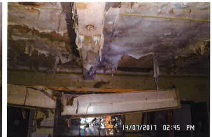
Foyer area ceiling, July 2017
