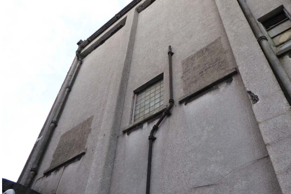
R Existing Masonry Infills to be Replaced
