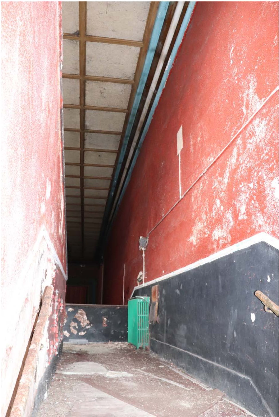
View at top of stairs leading to vomitory to auditorium balcony
