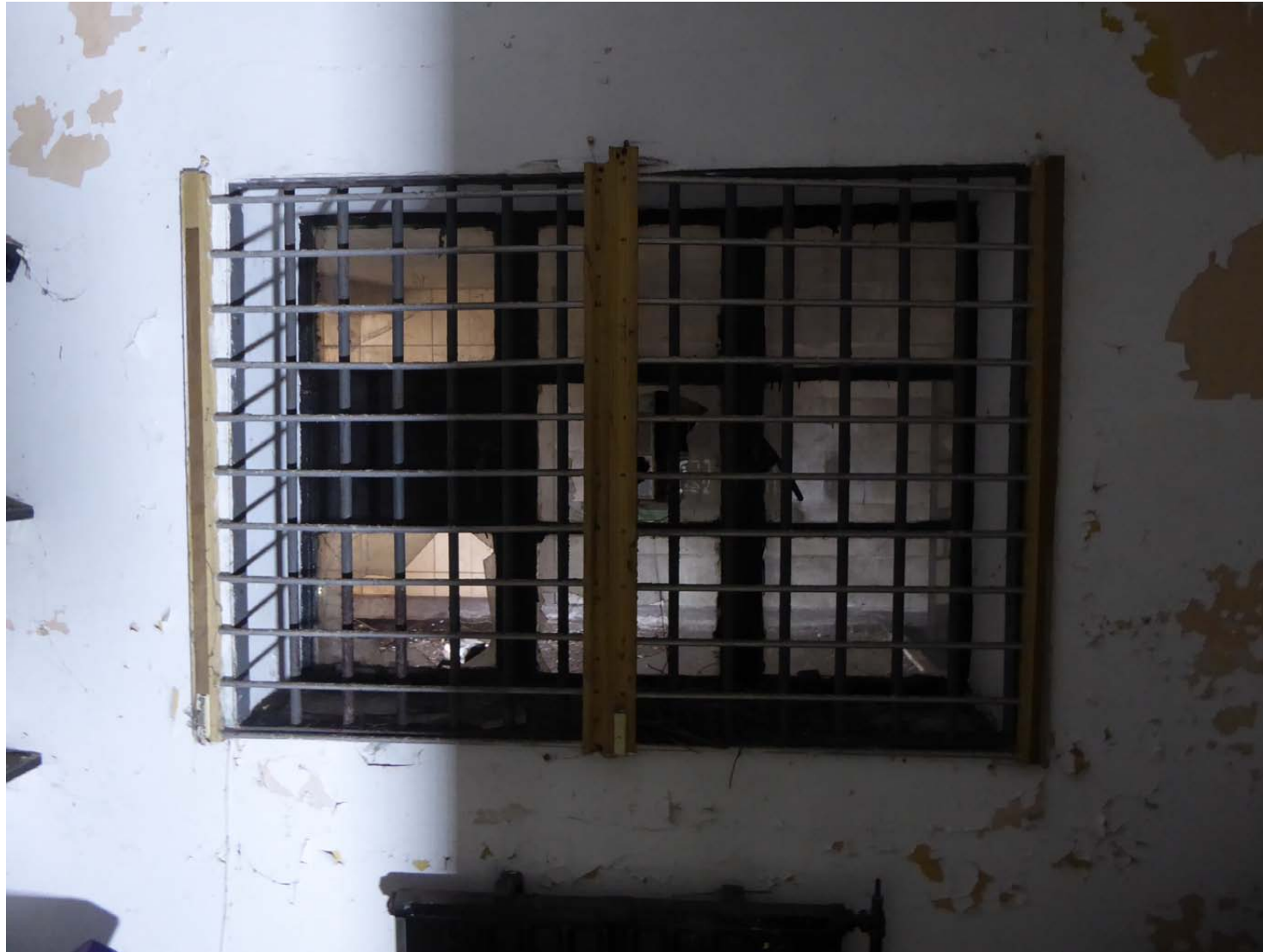
View of west wall with window looking out to recessed roof area
