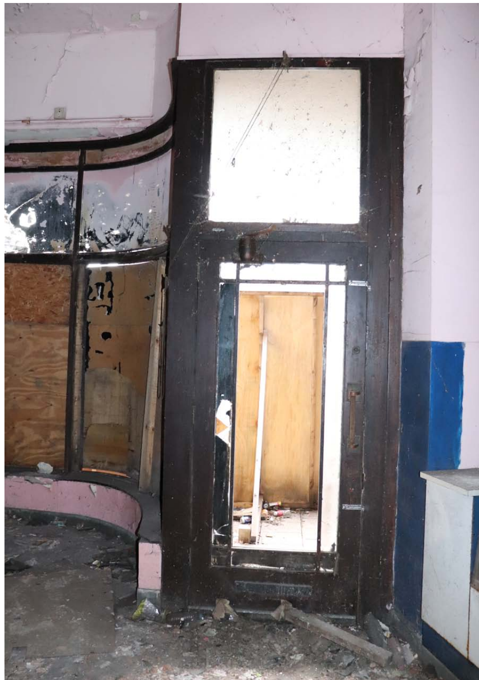
Timber-framed Glazed External Door with perimeter glazed panes
