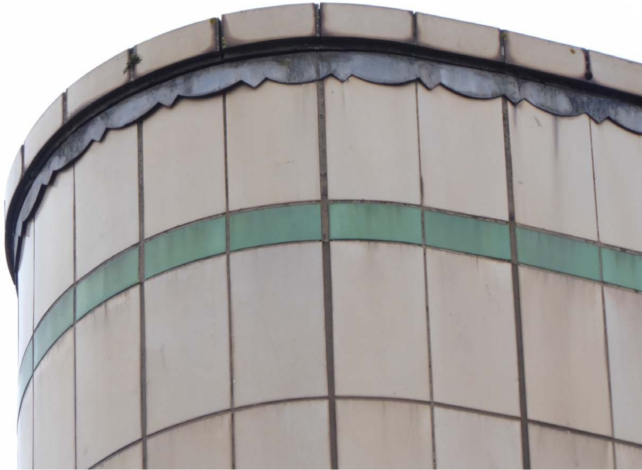
View of top of curved end with ornate lead dressing and faience brick capping
