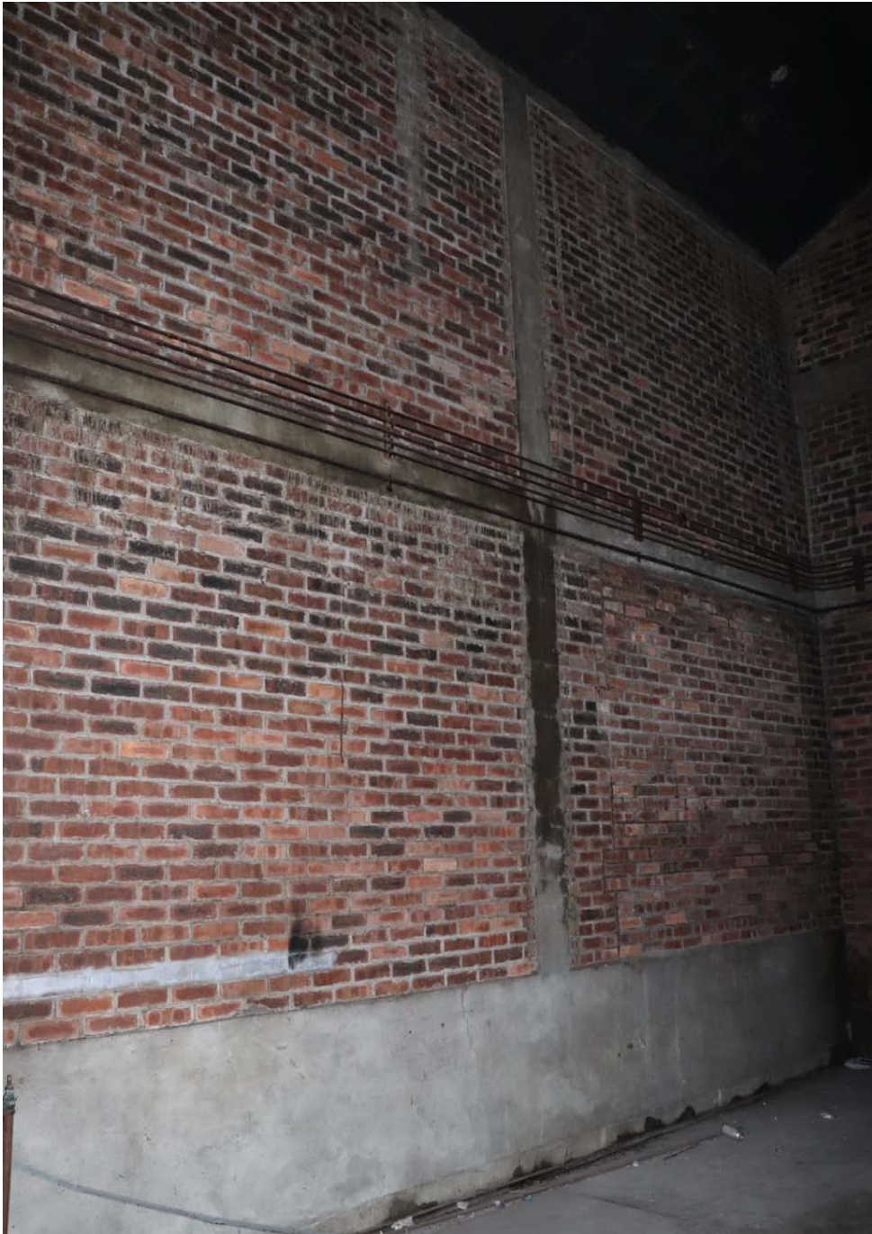
View of brick rear wall to stage within a concrete frame
