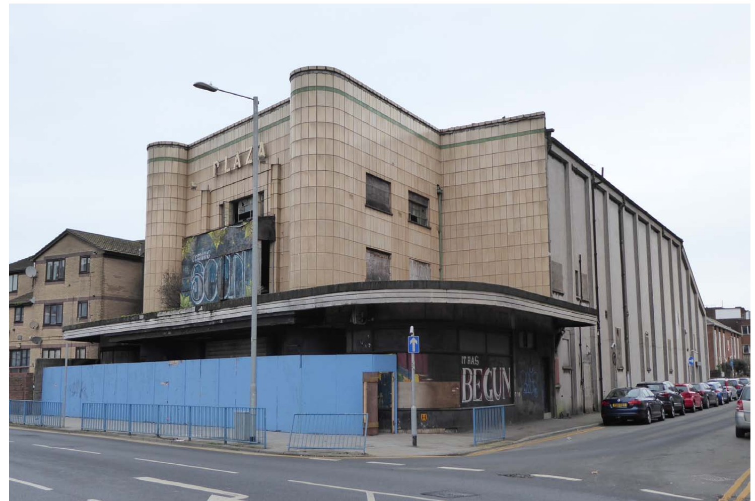
View of the Plaza from the south
