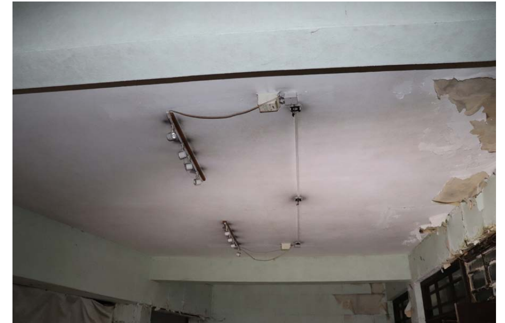
View of Painted Plastered Ceiling
