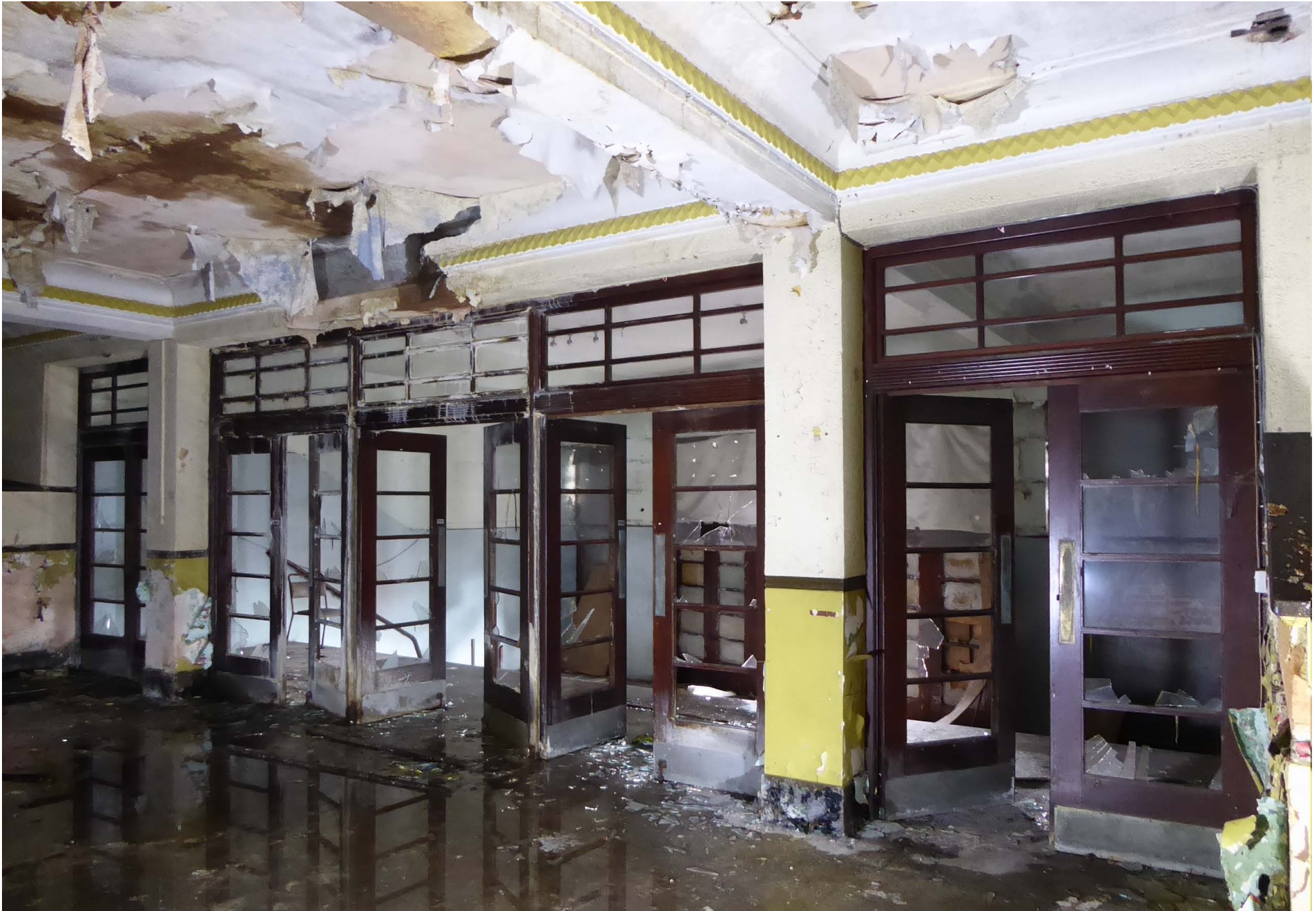
View of full extent of 5no. sets of doors
