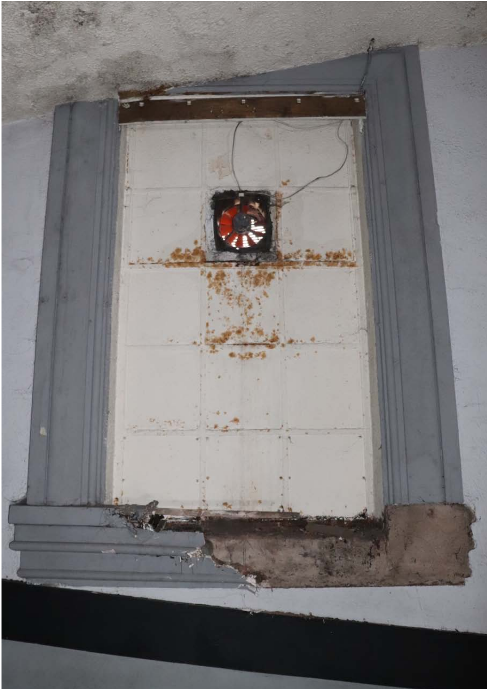
View of blocked up window on west elevation
