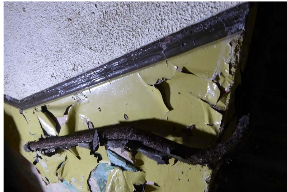
View of dado profile in plaster with handrail below
