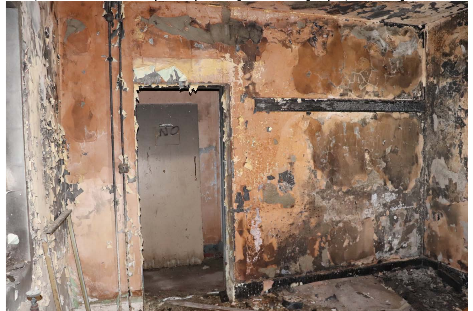
View of north wall with entrance door to room
