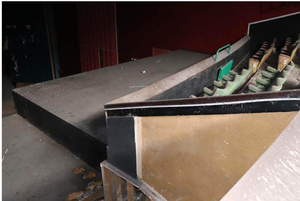
View of timber construction over the top of the east cinema below
