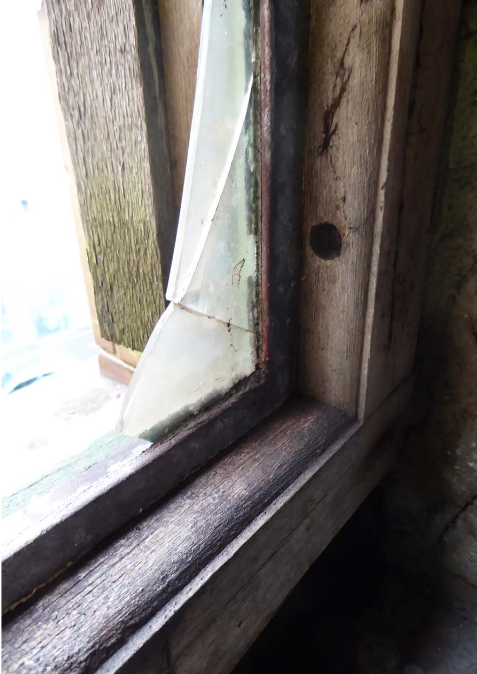
View of example of timber sub-frame to windows
