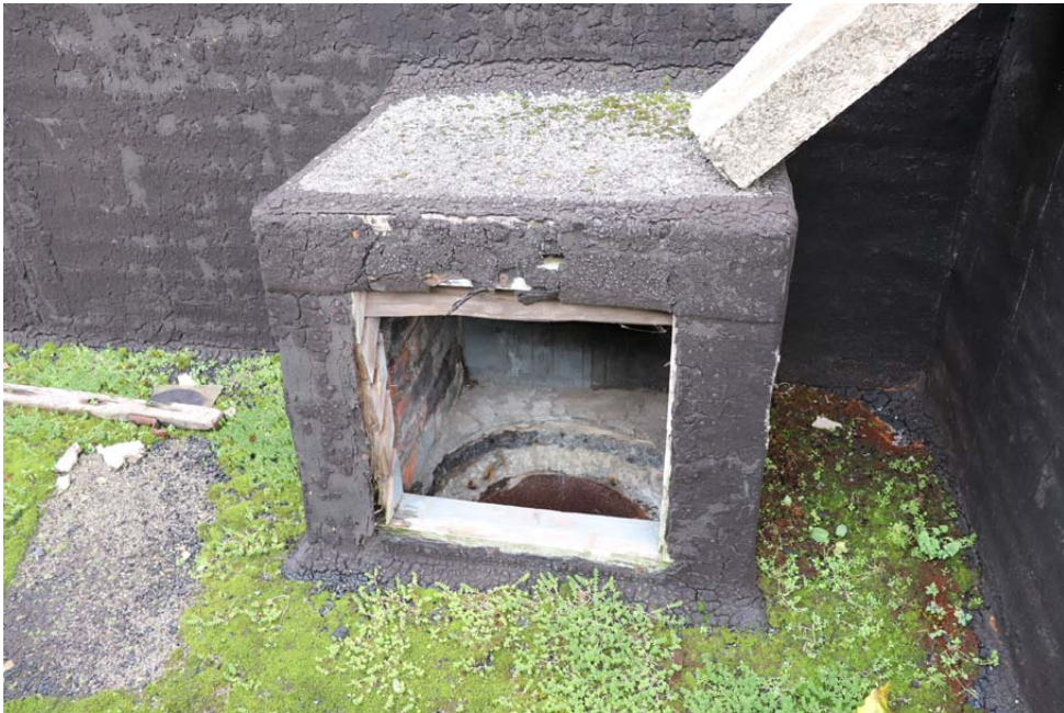
View of box construction to duct vent
