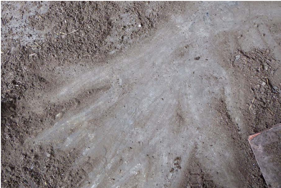
View of concrete floor
