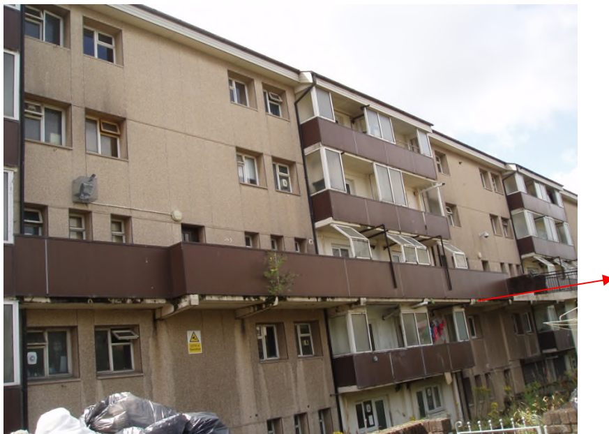
The rear of the building showing location of roost
