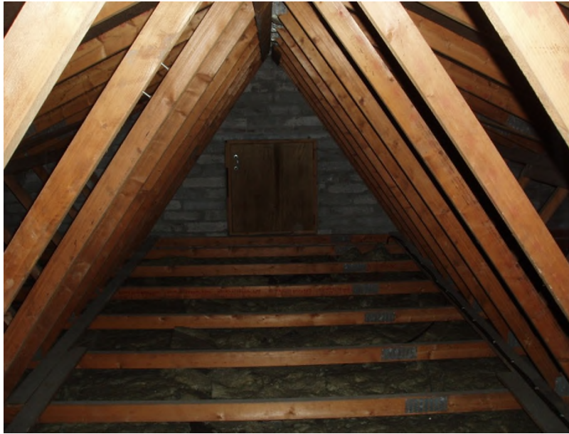
Inside the double itch loft space, built over the original flat roof structure
