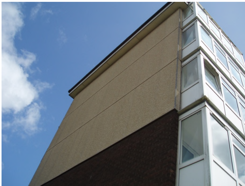
A view of the western gable showing cladding and tight soffits
