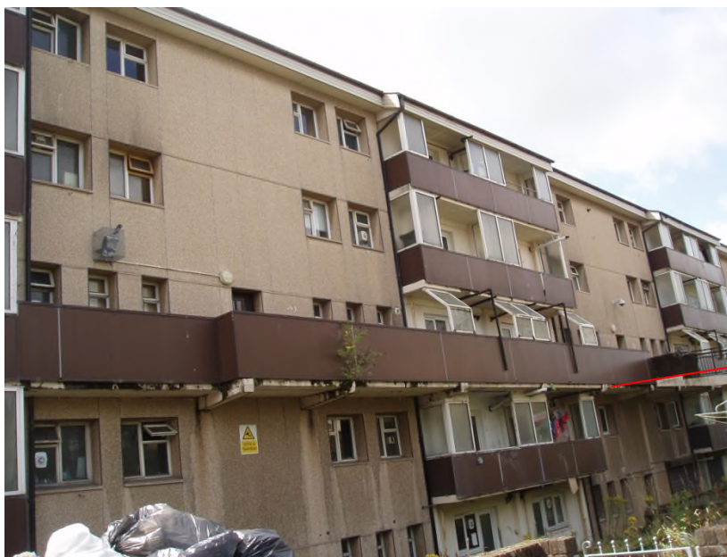
The rear of the building showing location of roost
