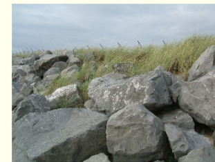
4577 North Westerly View
