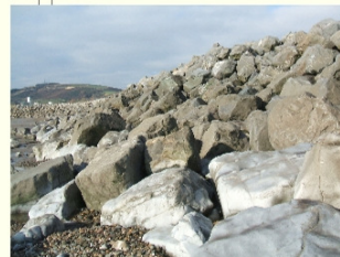
4594 North Westerly View
