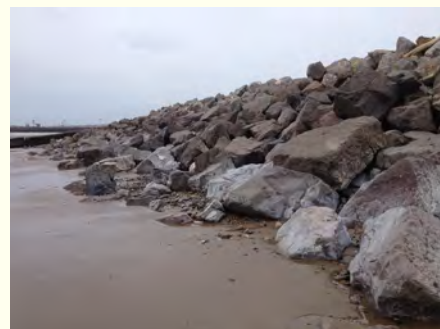
IP10 - South Westerly View
