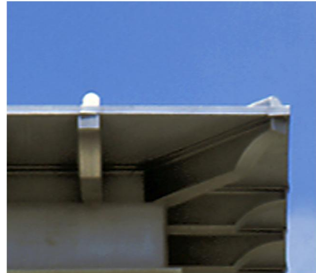
Image of Metal Cladding to Roof
