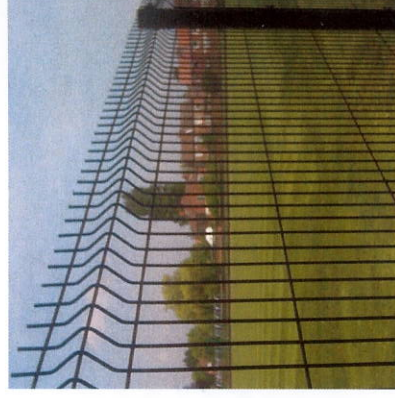
Welded mesh fence
