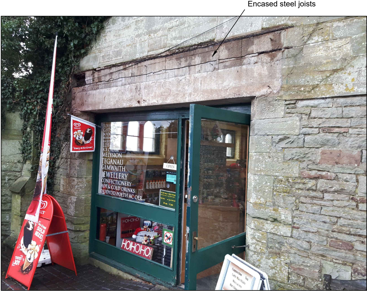
View on Shop Front
