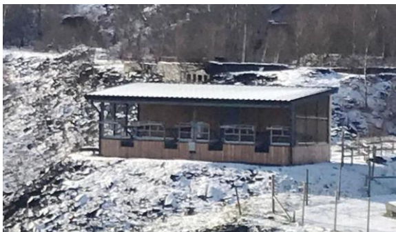
Similar dispatch platform (but at ground level, without supporting steel legs)
