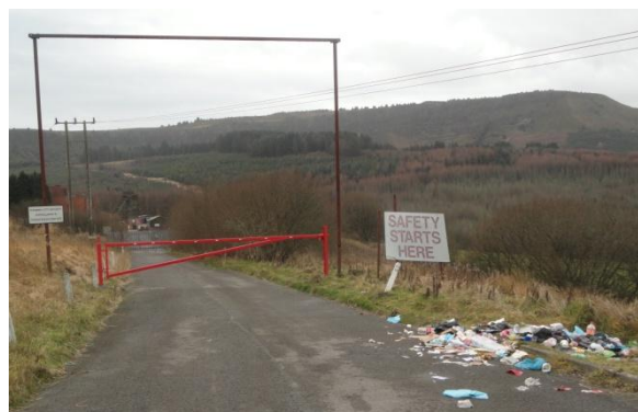
Existing access road to Tower Colliery
