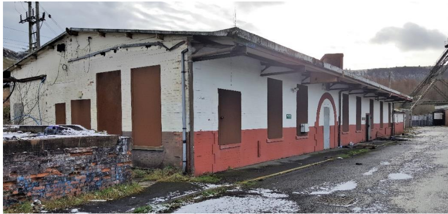
Figure 3.8 - Lamp Room / Office
