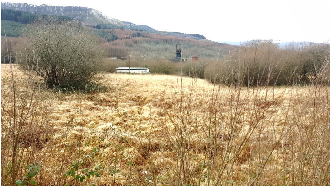
Figure 3.1 – view of Pithead from north-east
