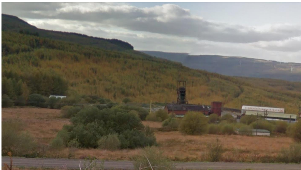
Figure 6.10 Part of application site at Tower Colliery from the east
