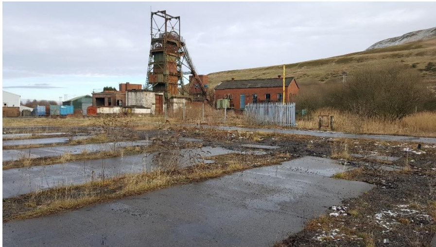
Figure 6.9 Listed buildings as viewed from southwest
