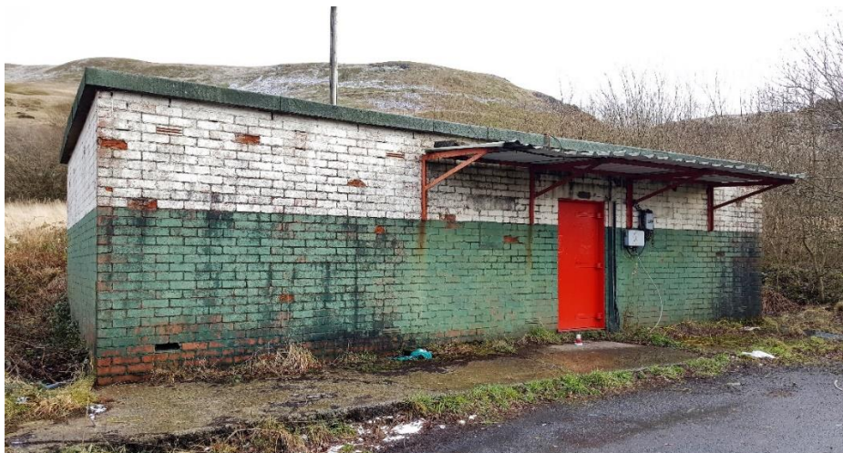
Figure 3.7 - Powder (Explosives) Room
