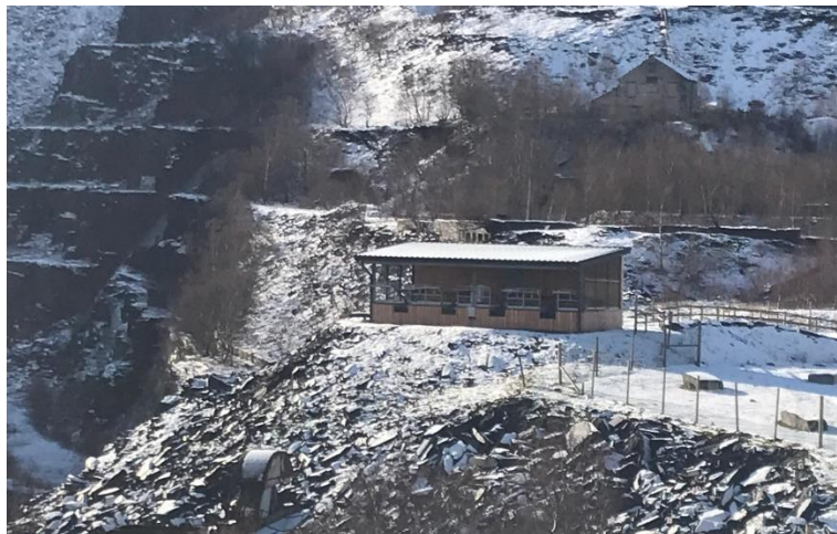
Figure 4.3 Example of zip wire despatch platform
