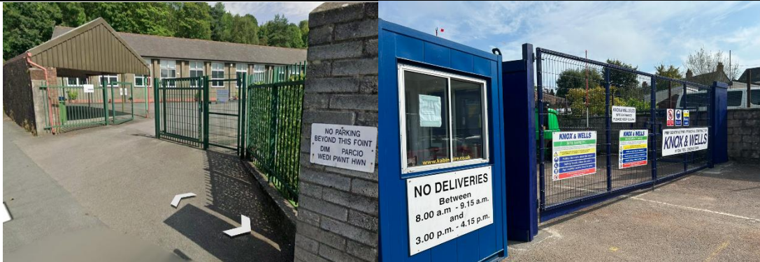
Existing gated access to YGG Tregelles (Pre-Demolition)
