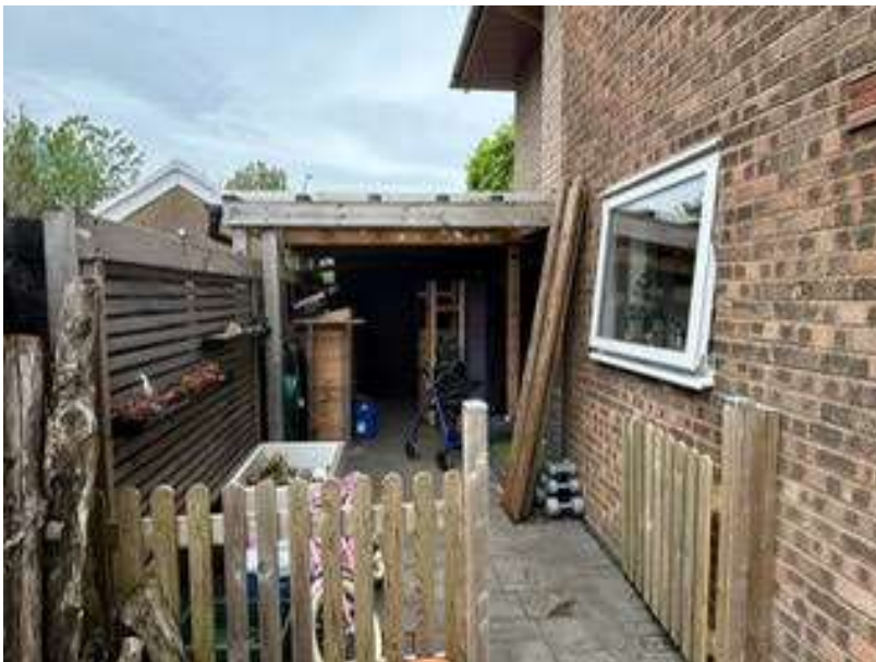
Closer view of existing extension to be replaced and where new roof canopy will be sited. Timber panelled and blockwork boundary to left side can be seen.
