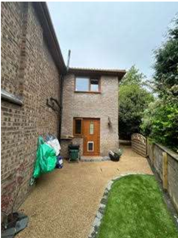
View of right side of property with blockwork boundary wall, small lawn and hard-surfaced area leading to the rear garden area.
