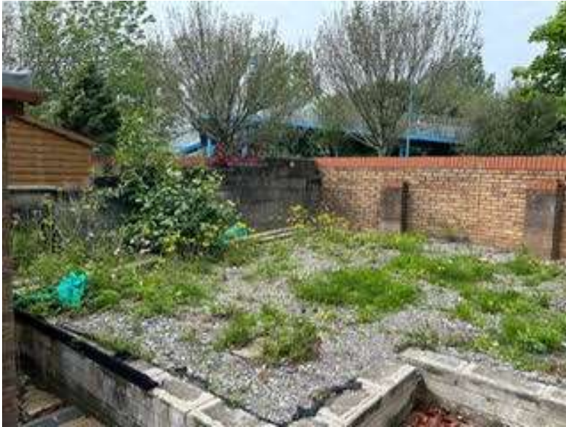
View of rear boundary area with brickwork and blockwork boundary walls and existing raised area.
