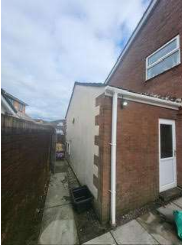
Close up view of existing garage, off which the new rear extension will be sited.
