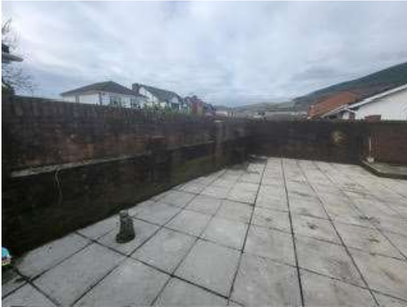
View of rear of plot including brickwork/blockwork rear boundary wall
