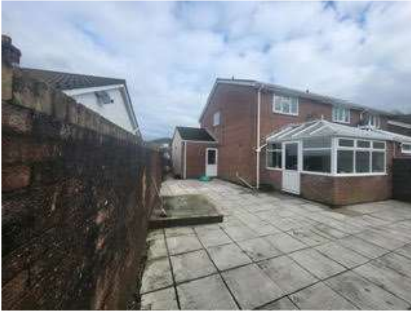
Further view of rear/side elevations including existing conservatory extension and large patio area
