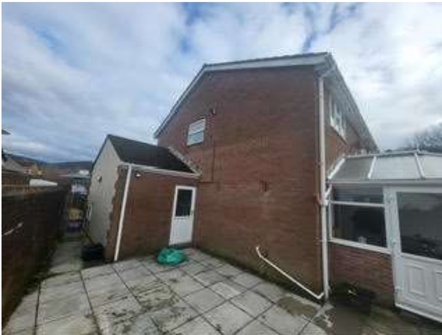
View of rear/side elevation and where the rear extension will be sited over the existing patio area
