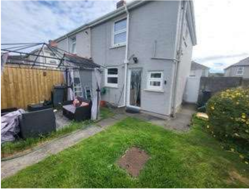
View of rear elevation and where the two storey and single storey extensions will be sited. Concrete path can be seen around the property and small patio area adjacent the rear elevation.
