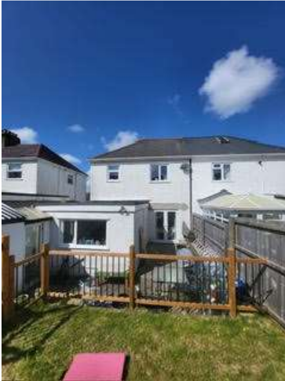
View of rear of property with existing rear extension and area to the right where the proposed extended rear extension will be sited. Existing raised lawn area can be seen in the foreground.
