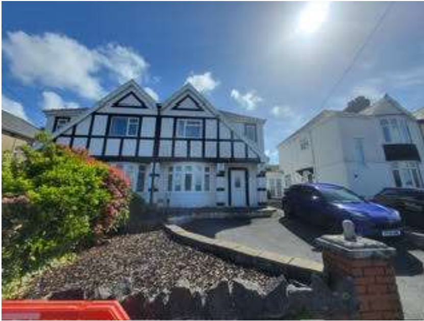
View of front elevation showing existing tarmac driveway and raised bedding area.
