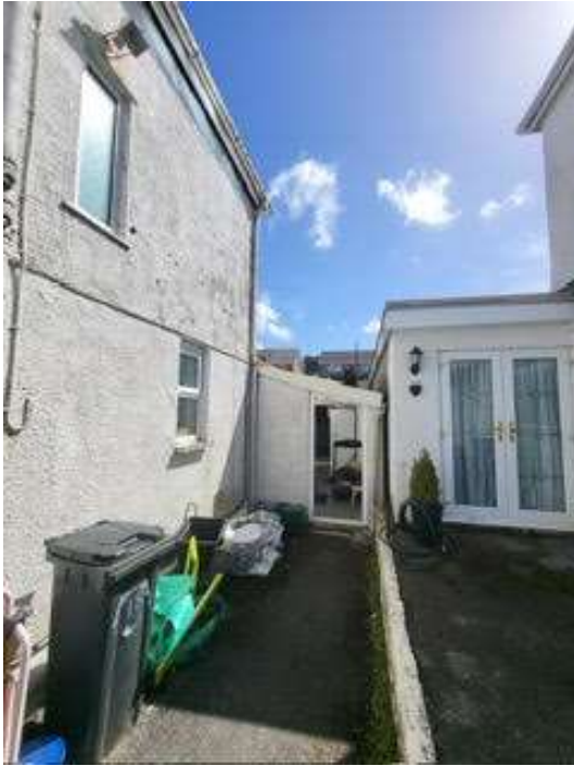
View of existing side extension to be replaced and tarmac area leading to the side access.
