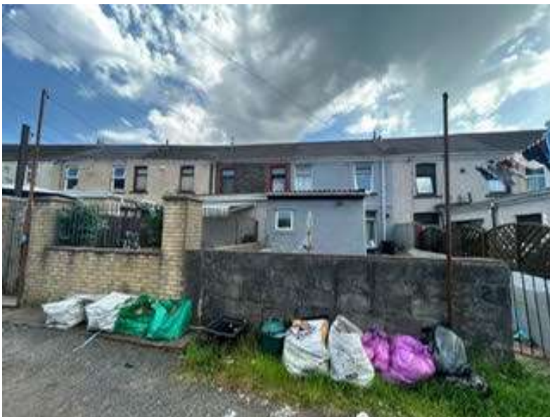
View from lane of the rear elevation
