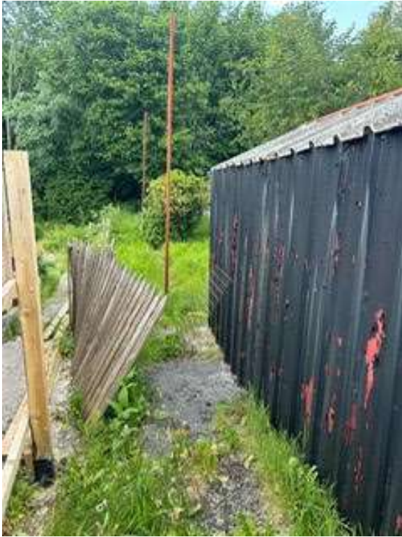
Further view of rear garden area with detached metal clad garage and lawn with tree line
