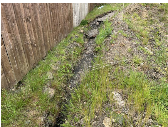
Figure 10 - Dry ditch onsite on western boundary.
