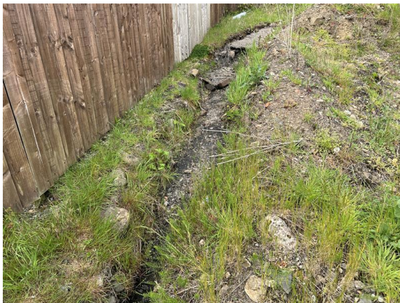
Figure 9 - Dry ditch onsite on western boundary.
