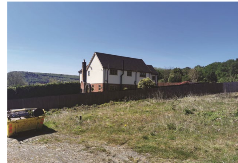
Large detached house to west of the site
