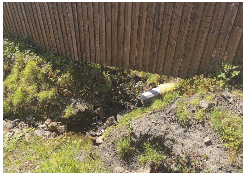
Existing pipe entering site, western boundary
