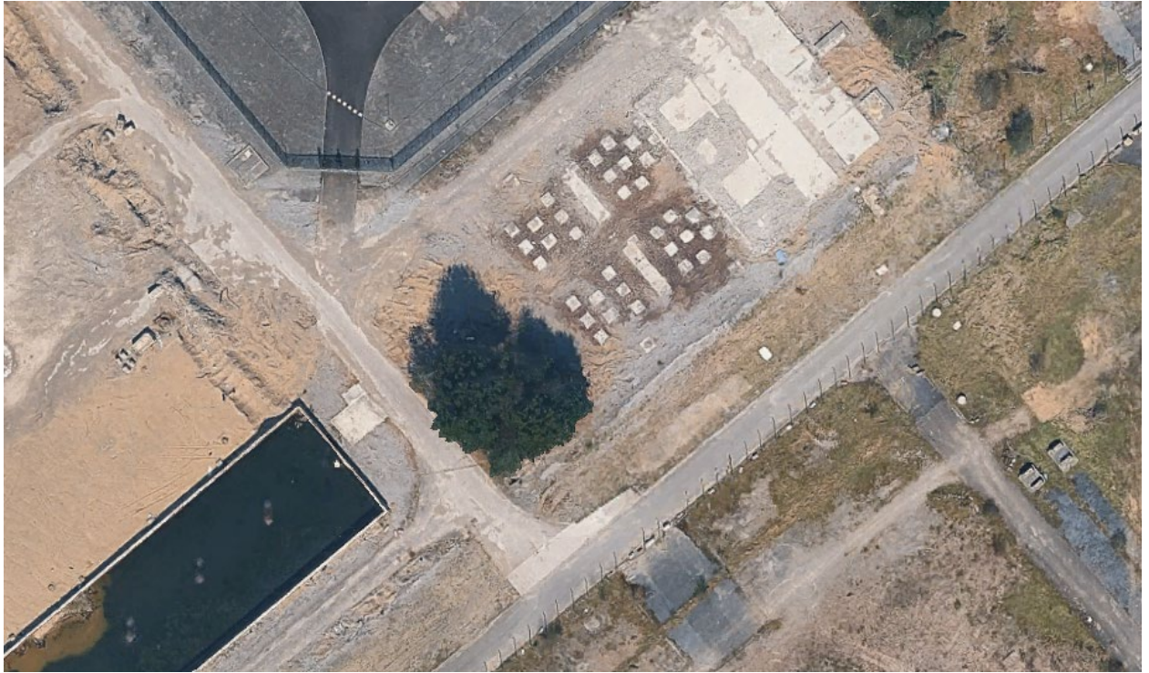
Figure 1 Group of trees to the south of the substation
